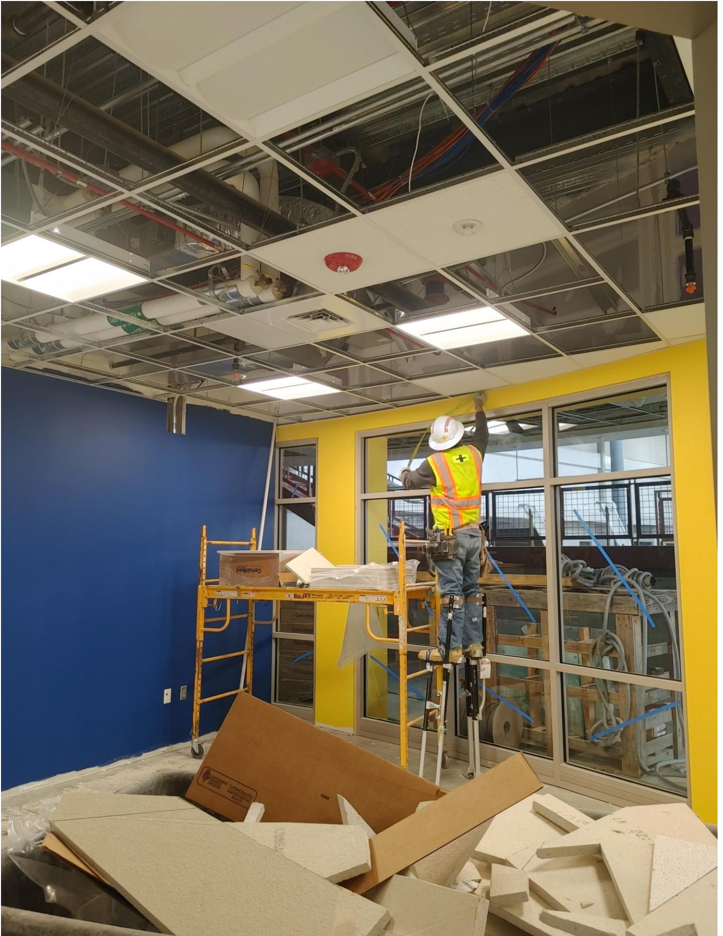
Photo 3 - Acoustical Tile being installed in Area A.
