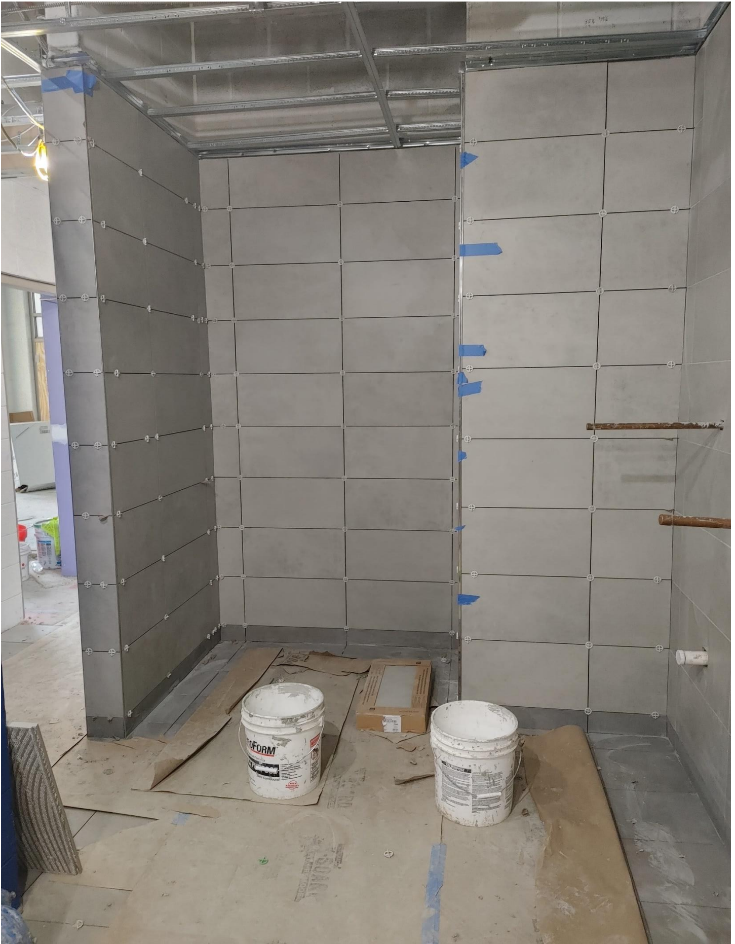
Photo 11 - Wall tile has been set in Boys Toilet E103.
