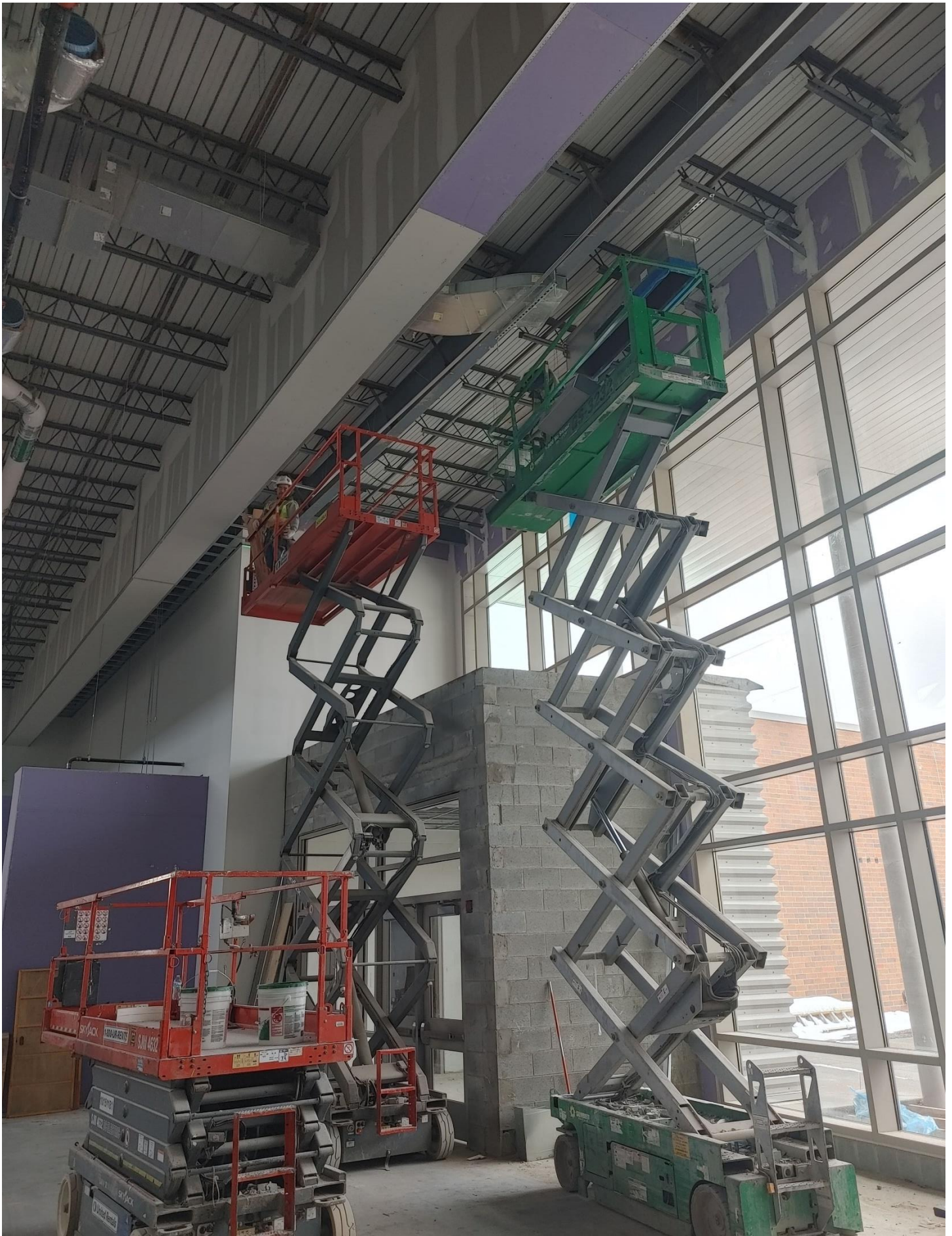
Photo 2 - Acoustical Ceiling Grid and HVAC Duct is being installed.
