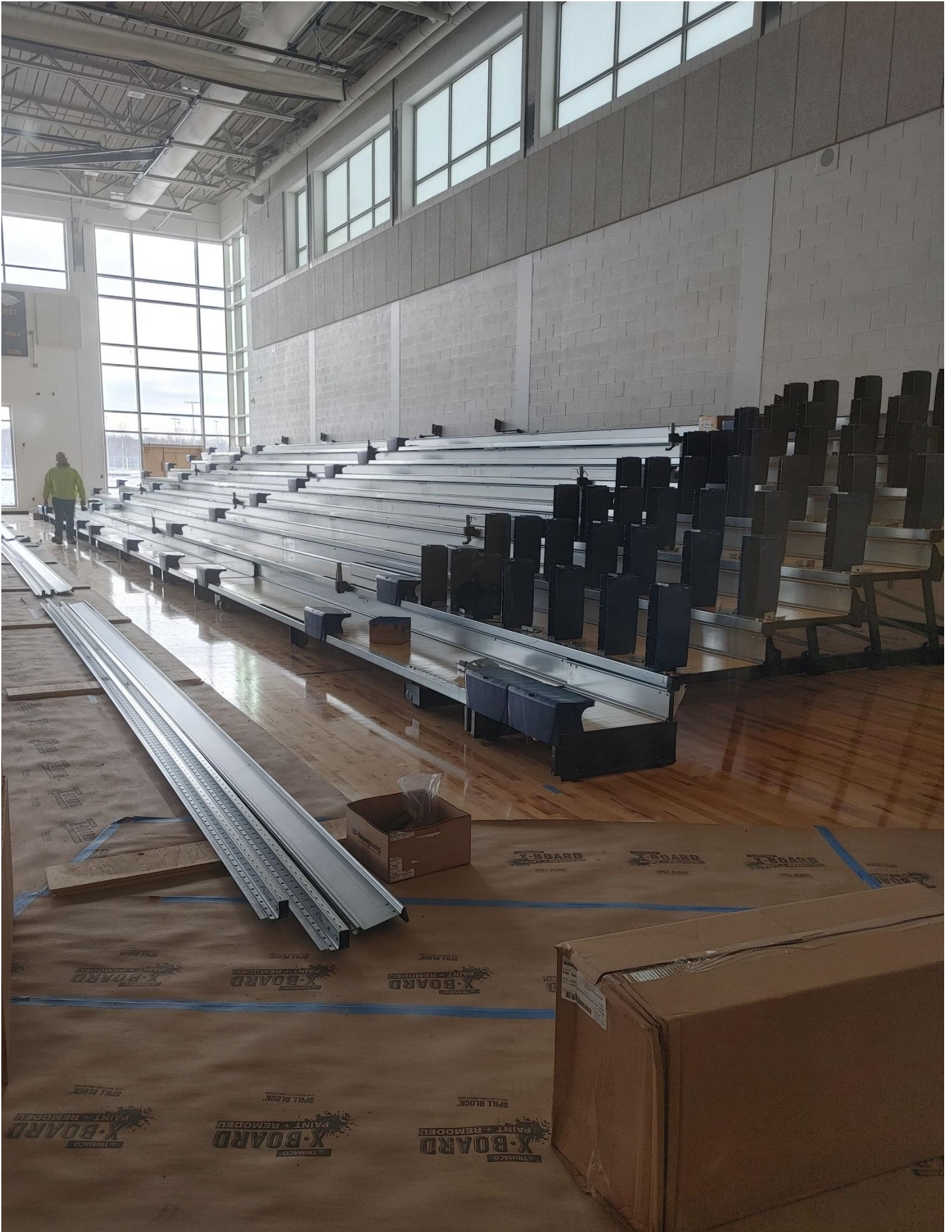
Photo 12 - Bleachers are being constructed in Gym.
