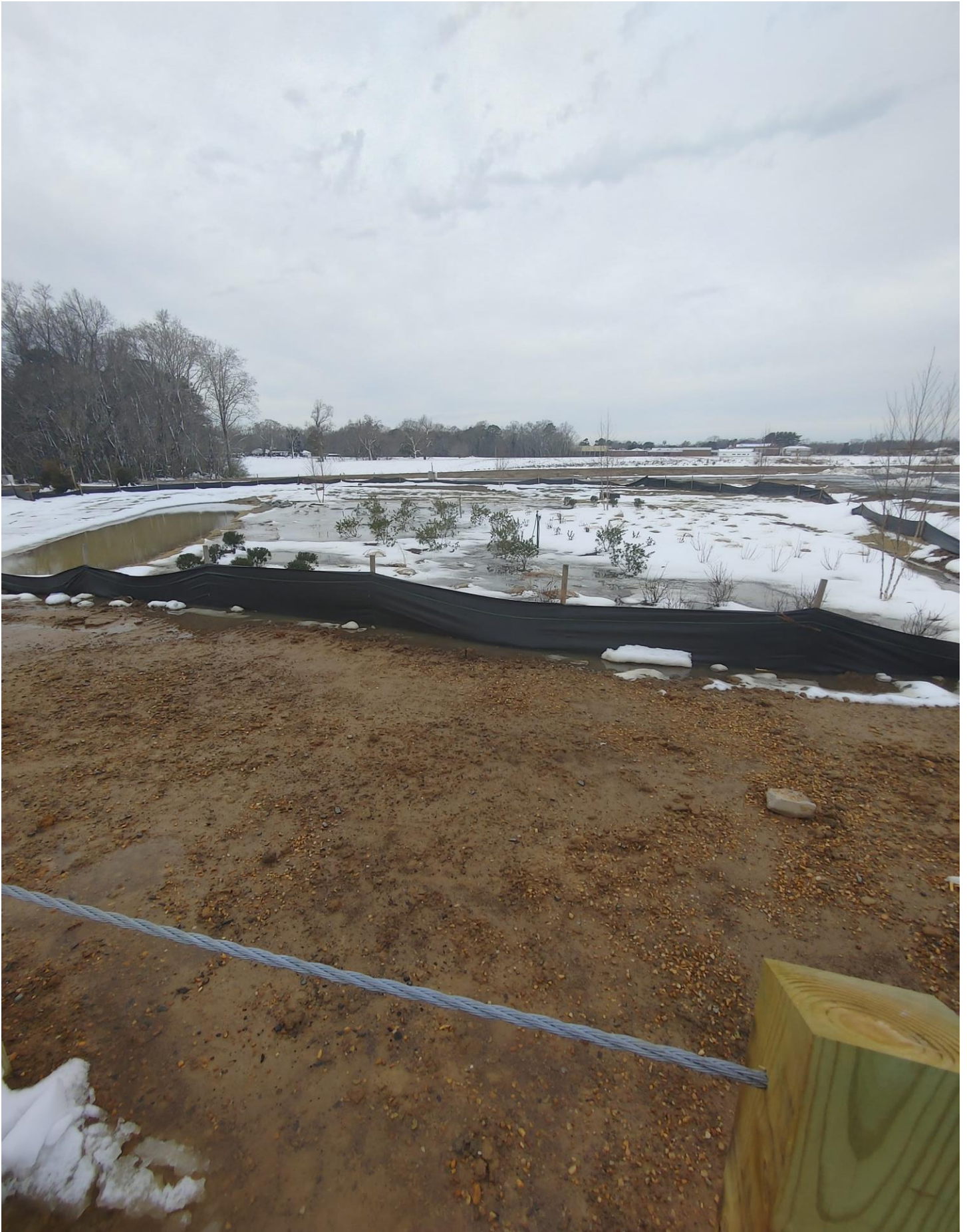
Photo 17 - Retention Pond on Westside of Bus loop.
