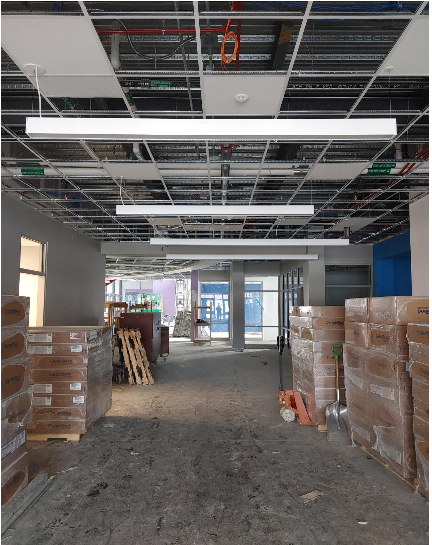
Photo 1 - Lights have been installed in Corridor A13 near the main entrance.
