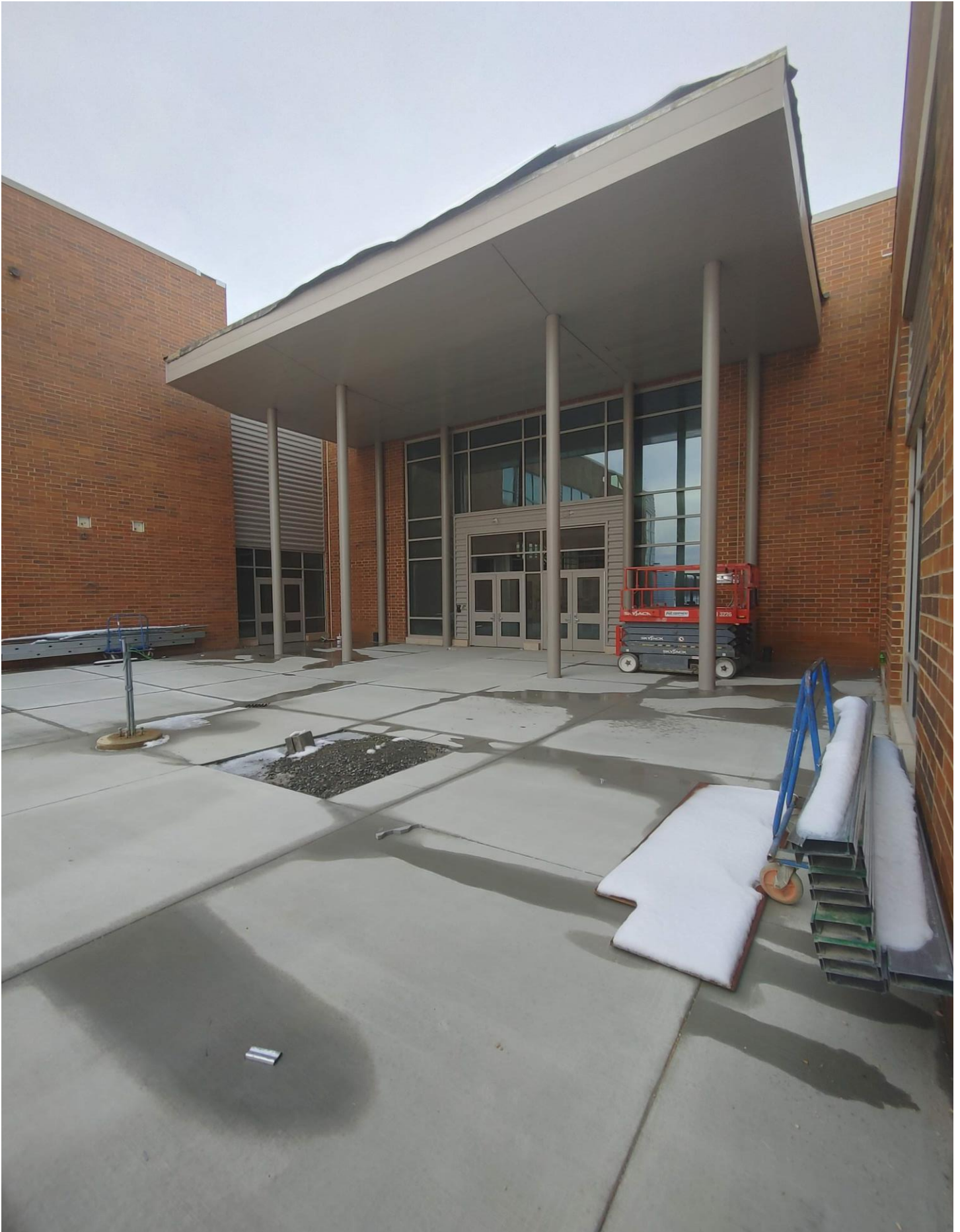
Photo 9 - Rear Canopy and columns of Area C have been painted.
