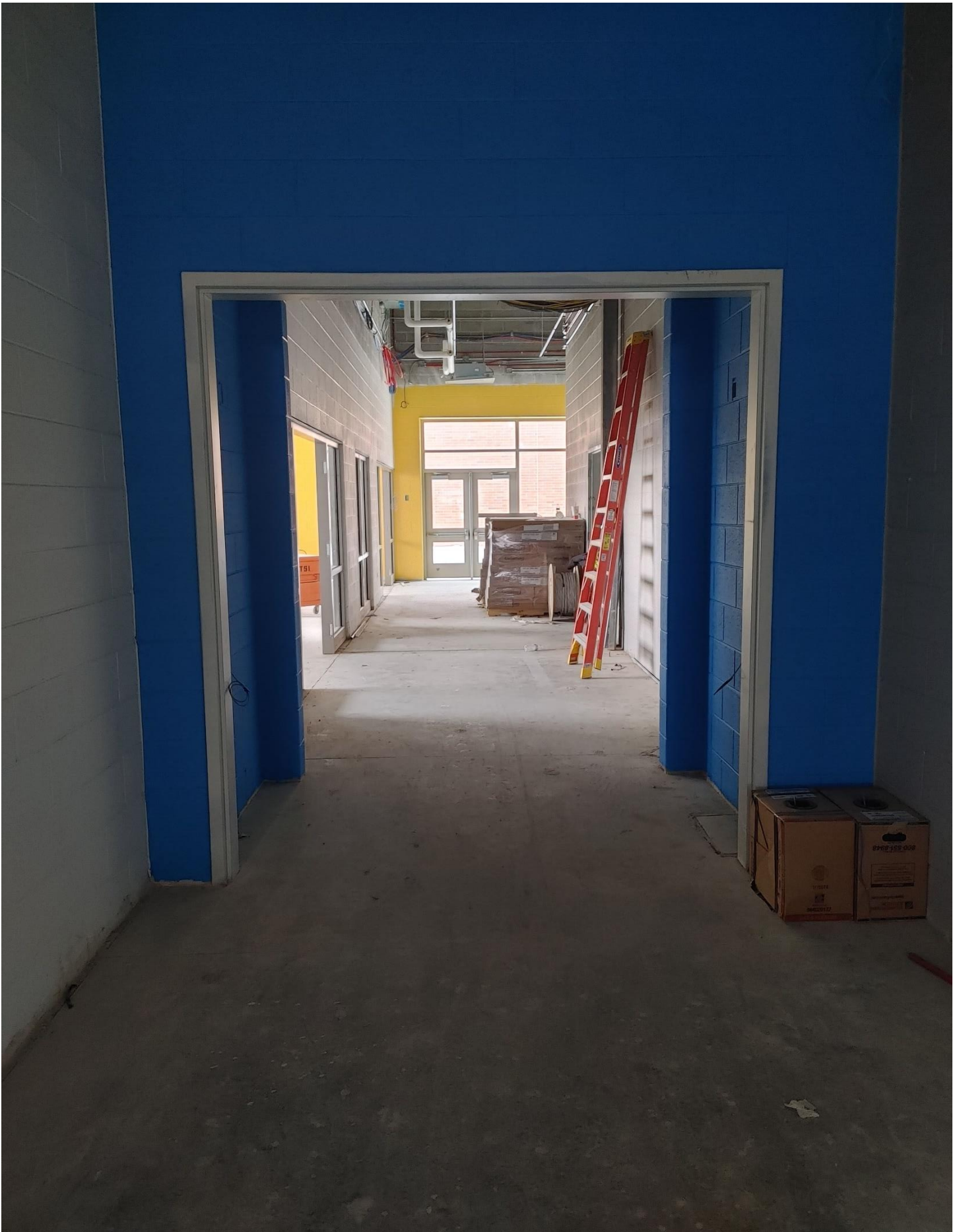
Photo 8 - Frame D12 has been installed.
