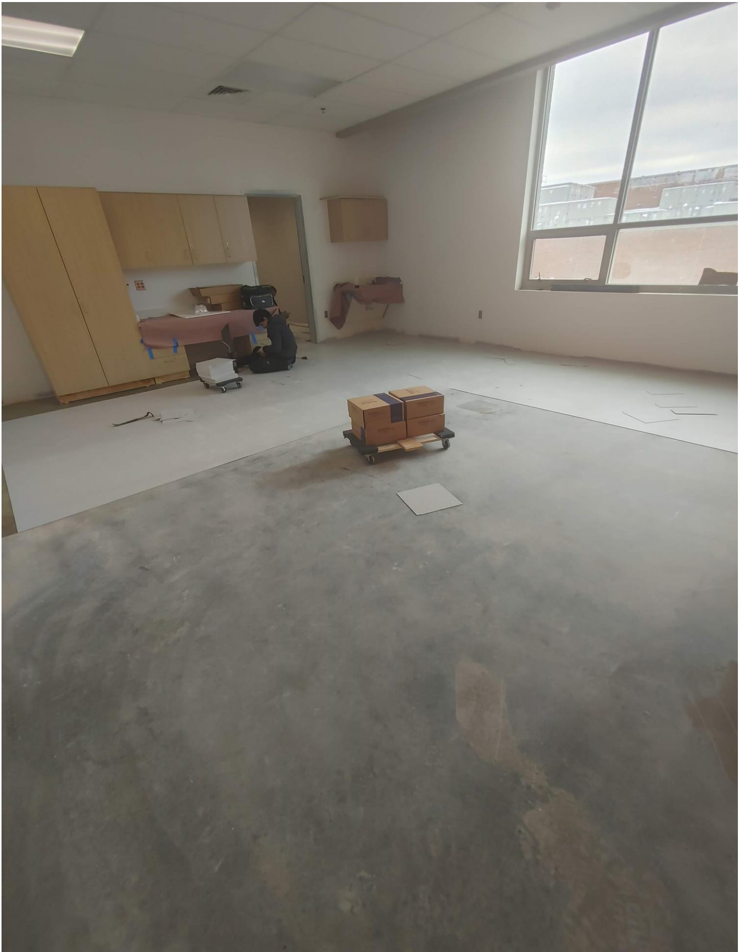
Photo 15 - VCT is being laid in Area B
