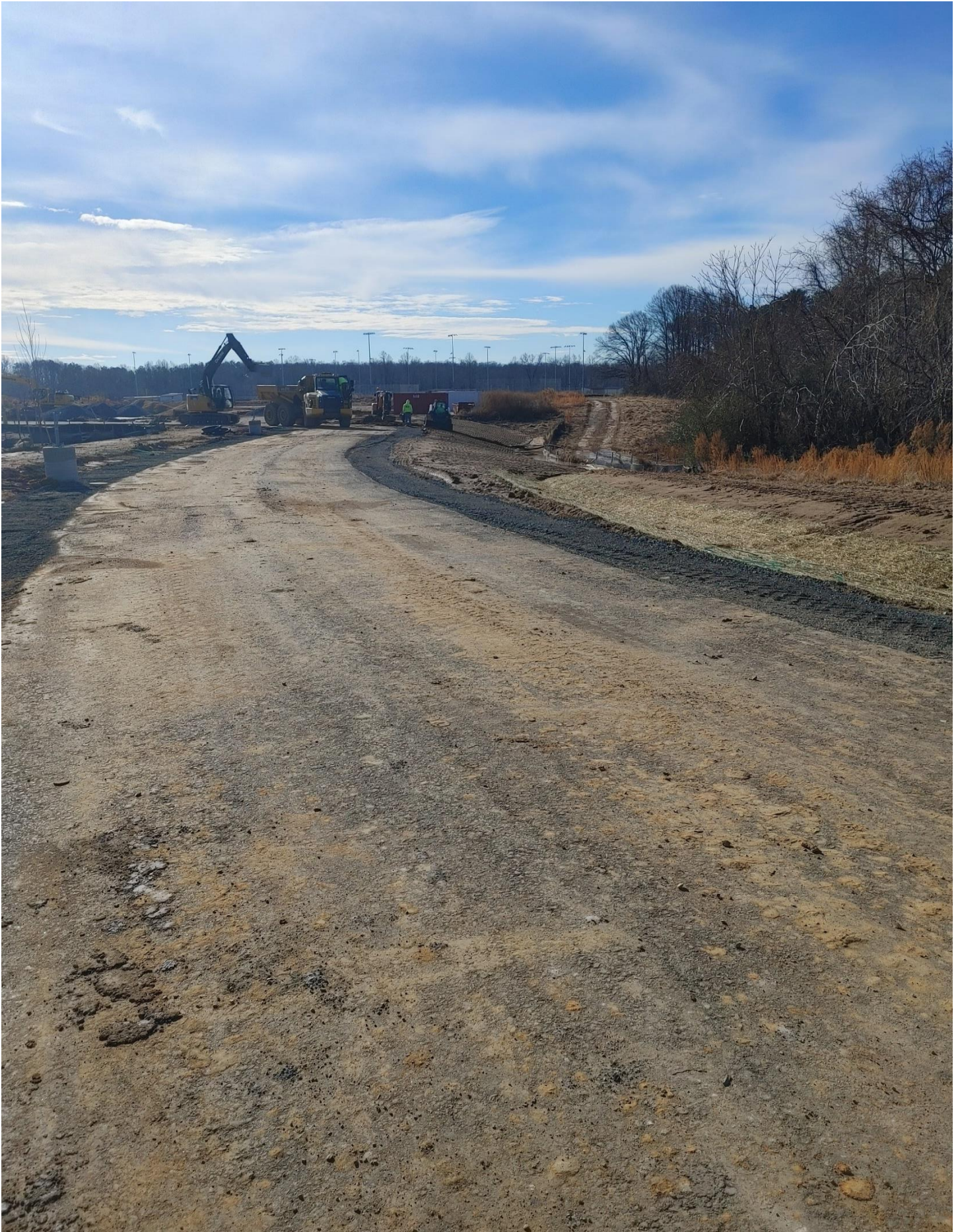
Photo 15 - Ditch and Bank Grading is occurring on West side of site
