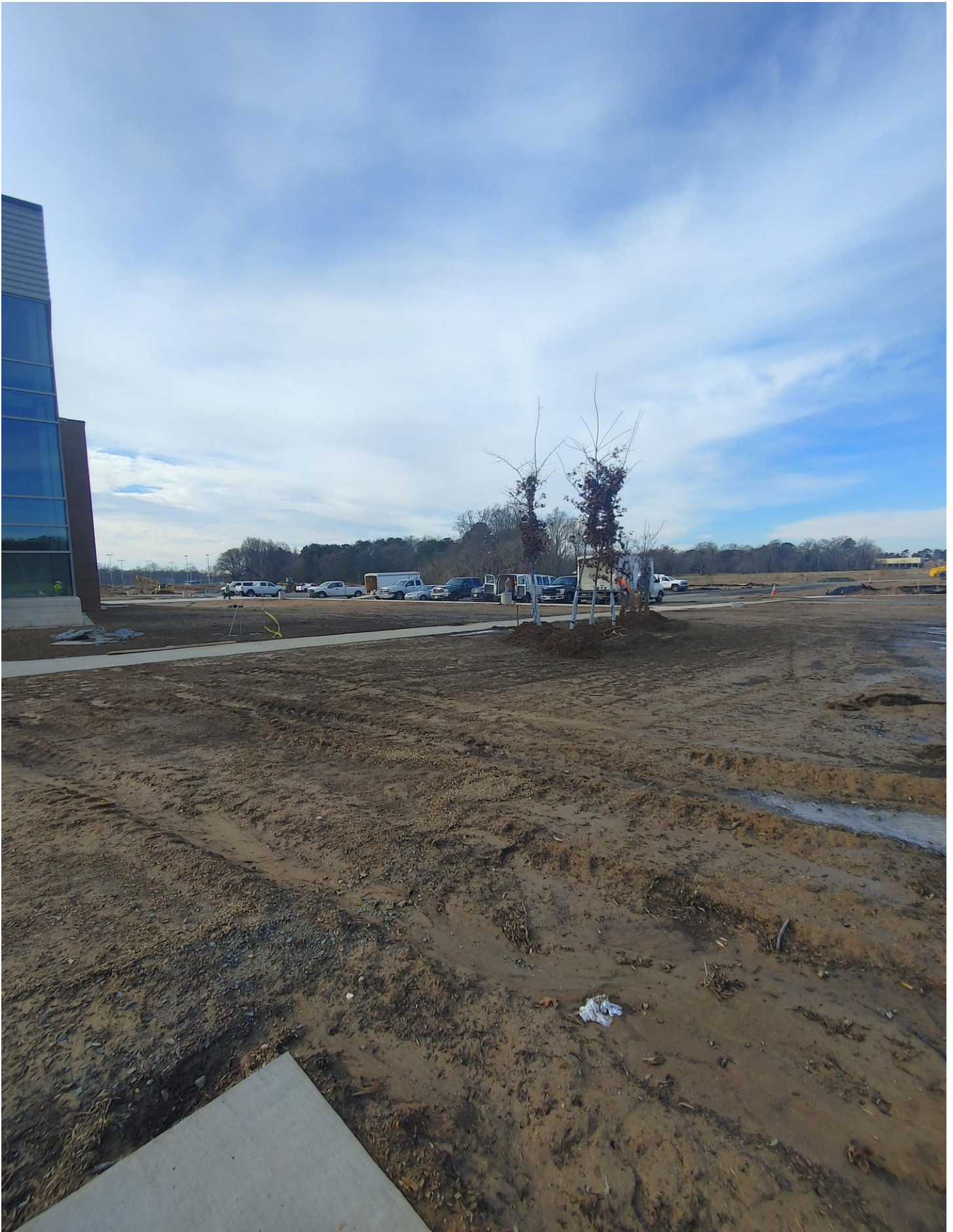
Photo 12 - Northwest Corner of Site
