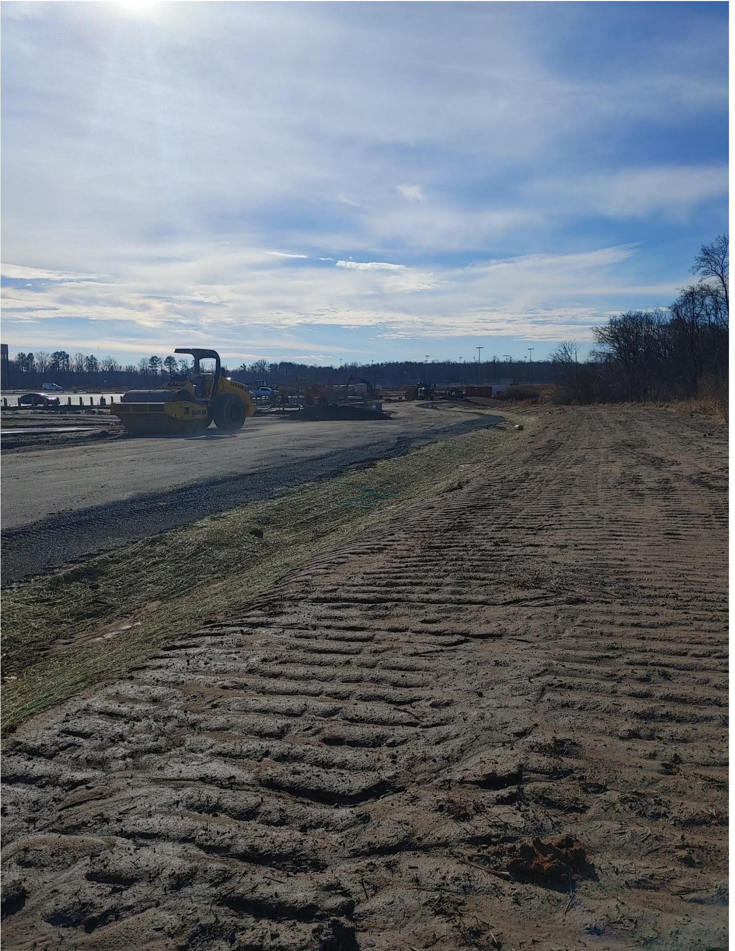
Photo 13 - Bus Entrance shoulder work and ditch grading is ongoing.
