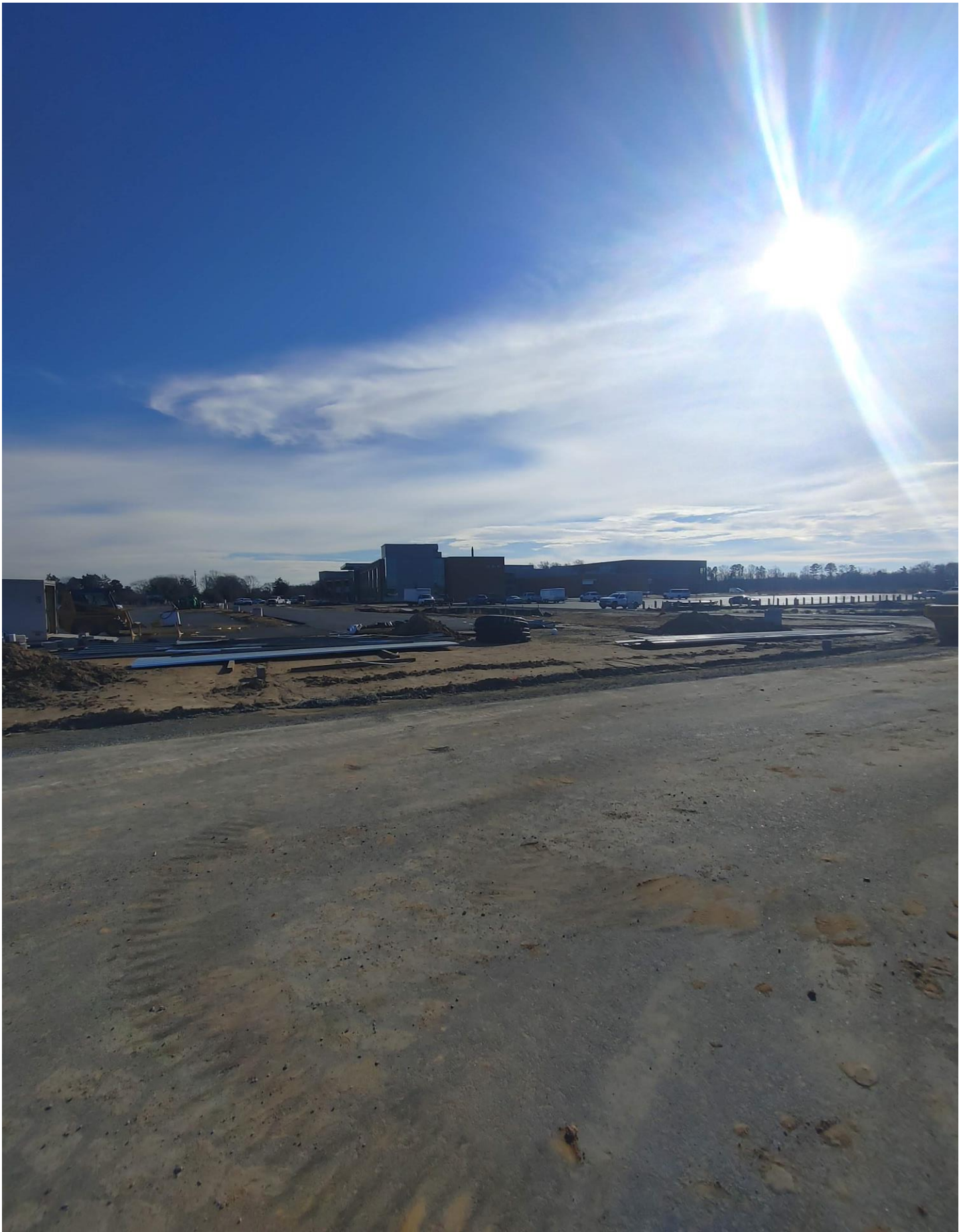
Photo 14 - West side of School
