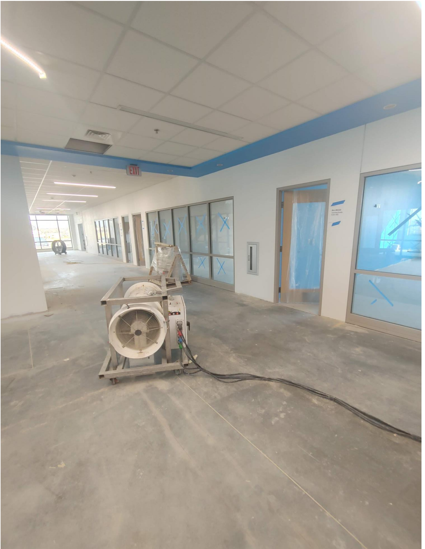
Photo 10 - Doors have been hung in Area B, 1st floor.
