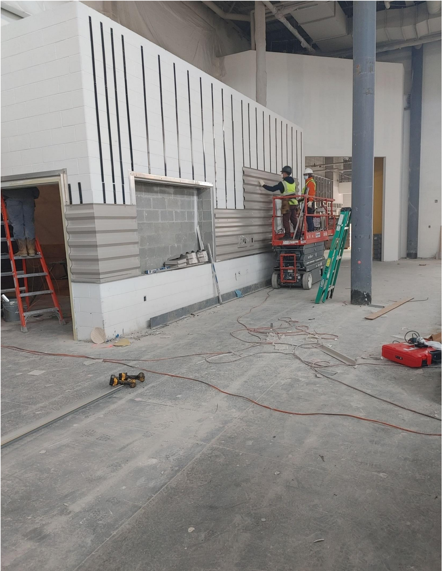
Photo 3 - Metal Panels are being installed outside of Ticket Office.
