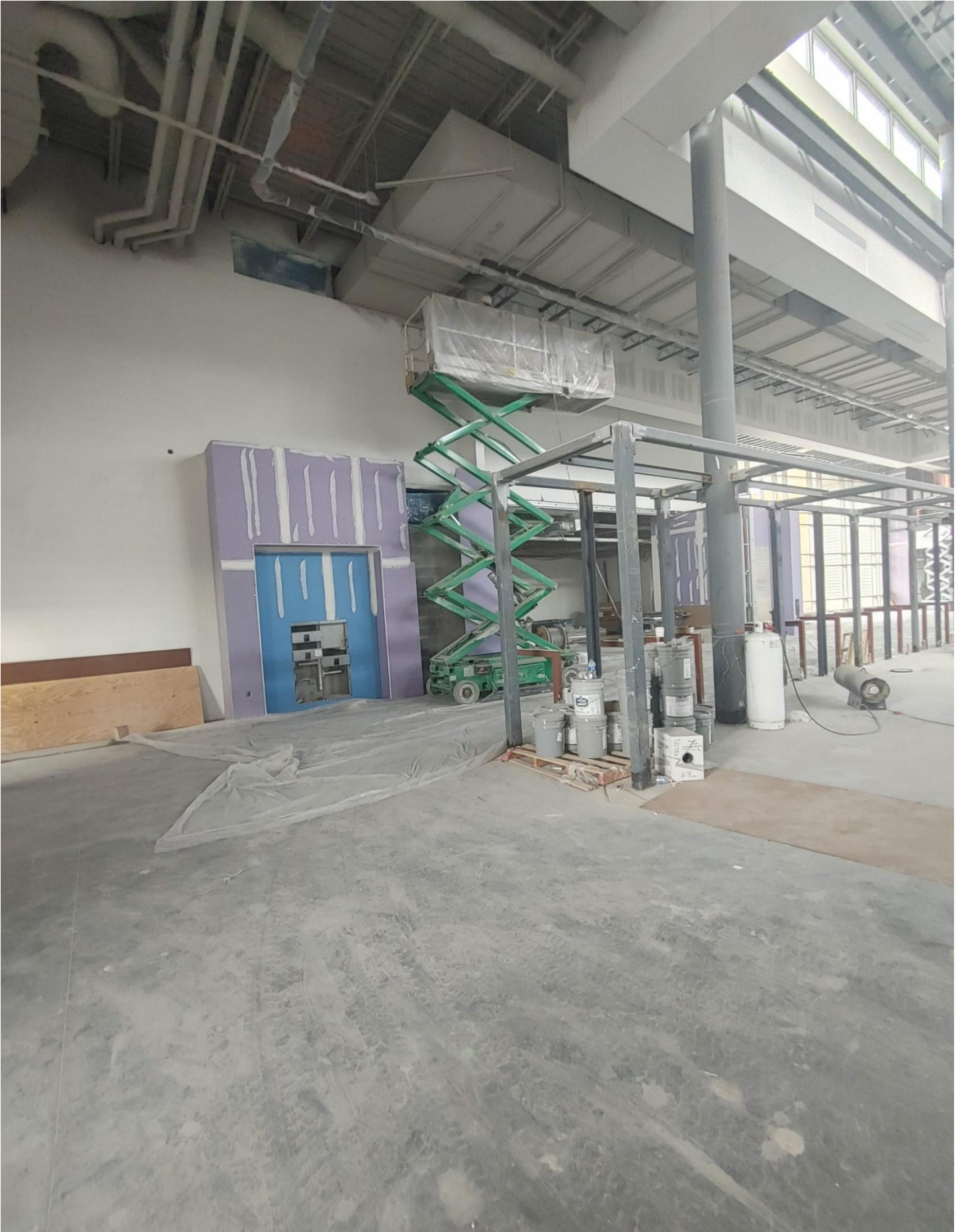
Photo 4 - Painters are painting walls in Area C
