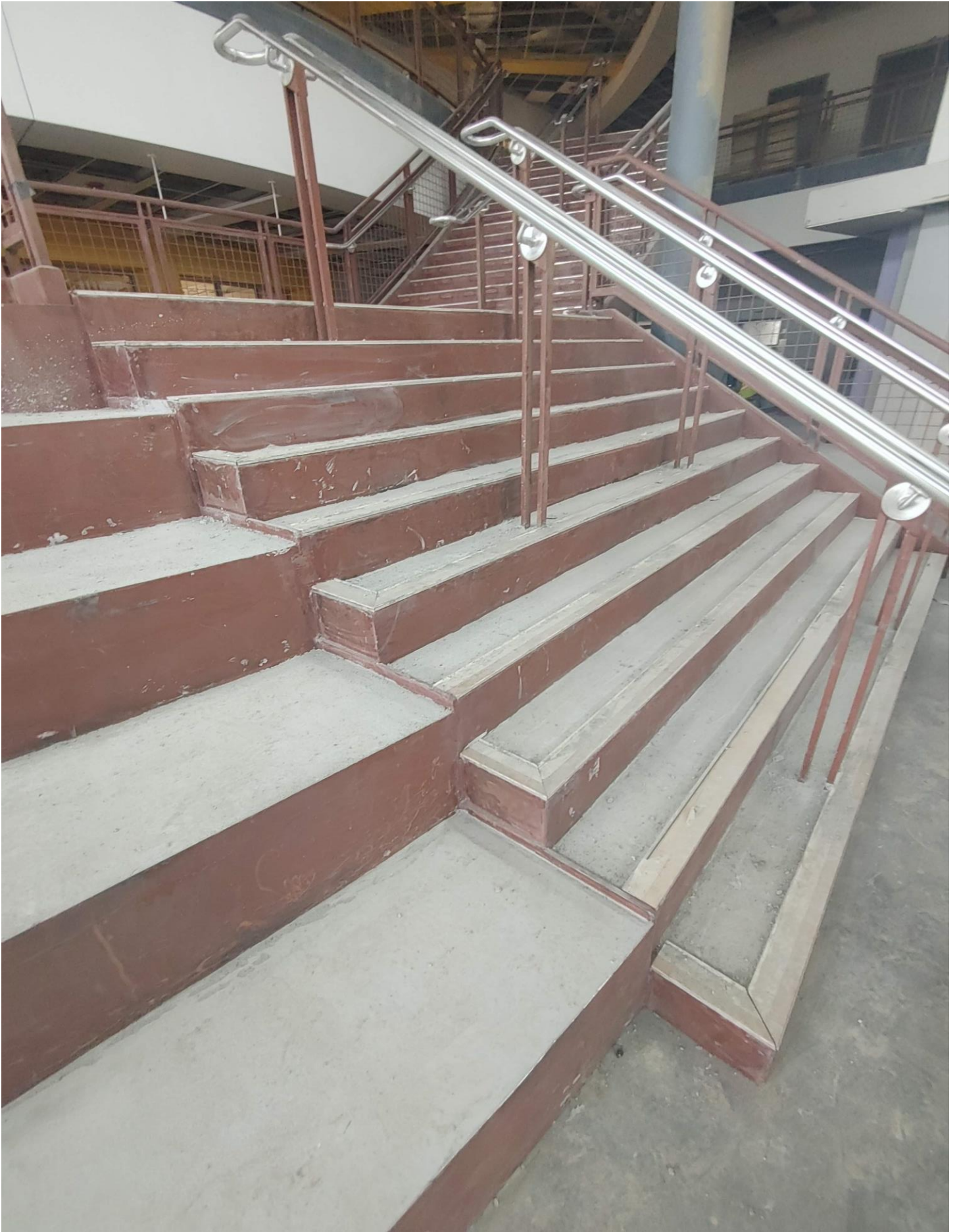
Photo 2 - Grand Staircase Treads have been poured
