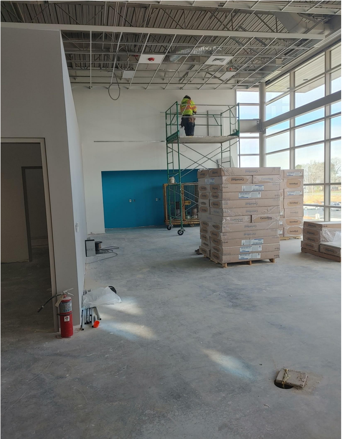
Photo 6 - Acoustical Panels are being installed in Area A, A220
