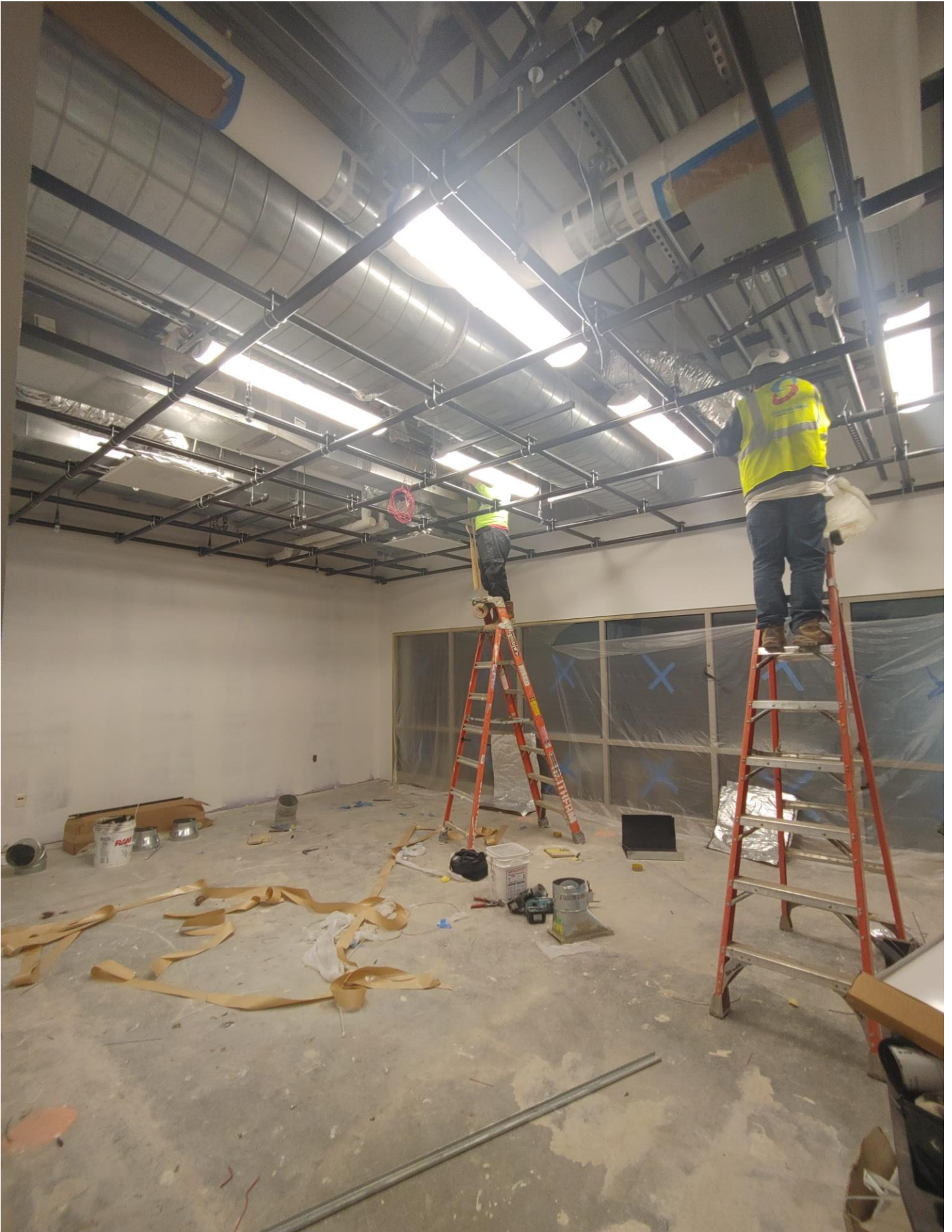
Photo 8 - Work progressing in room A221, TV Studio/Video Production
