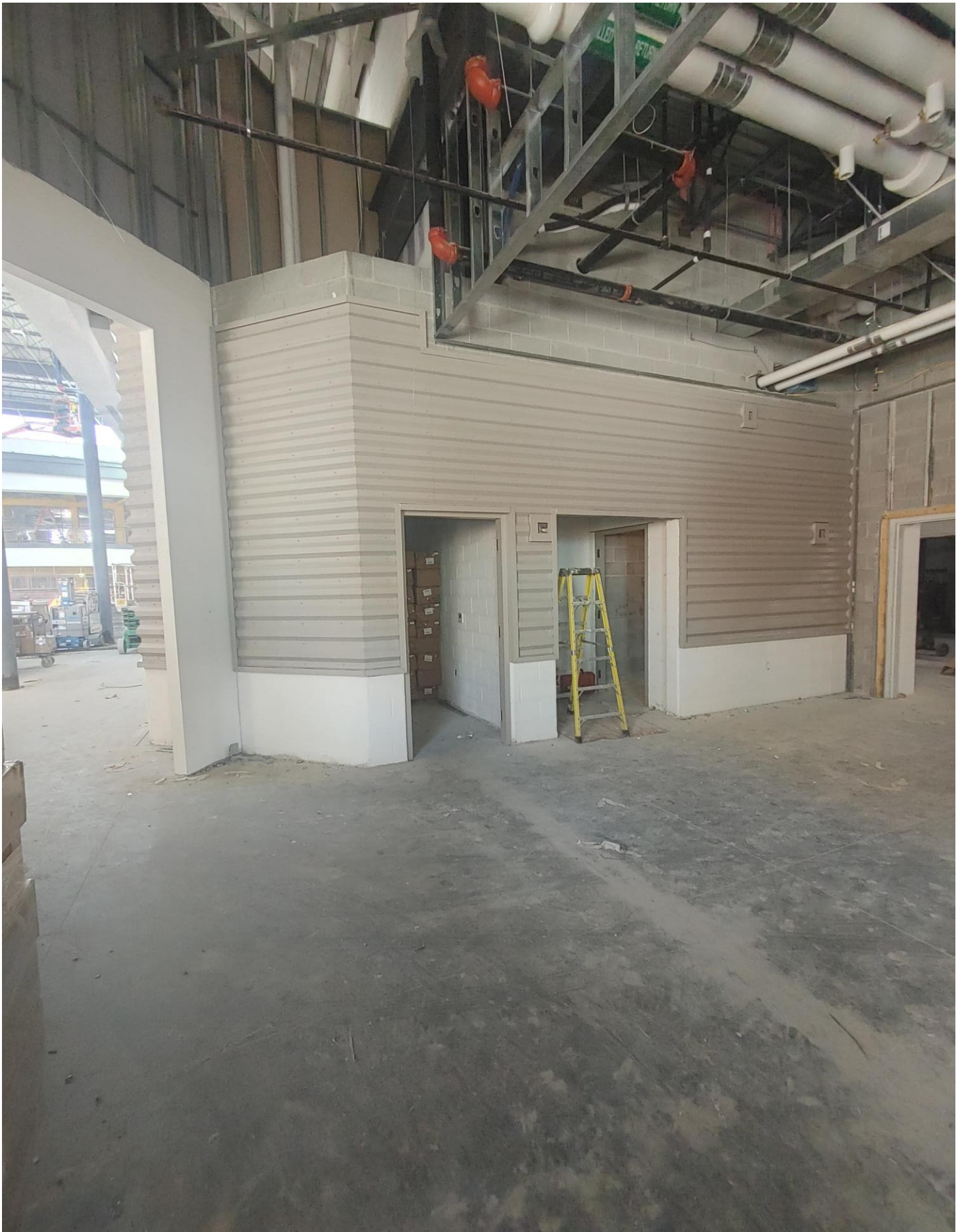
Photo 5 - Metal Wall completed outside of D104 and D117
