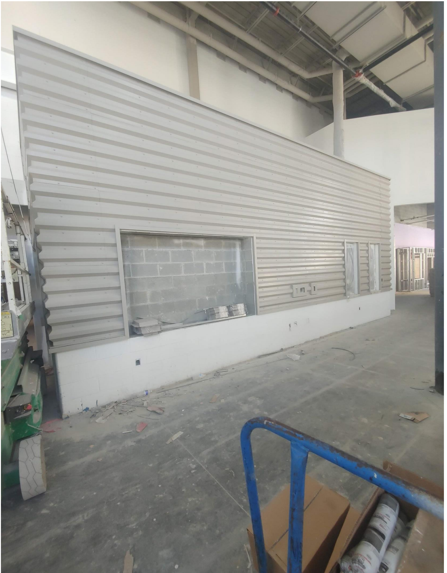
Photo 4 - Metal wall has been completed in Area C
