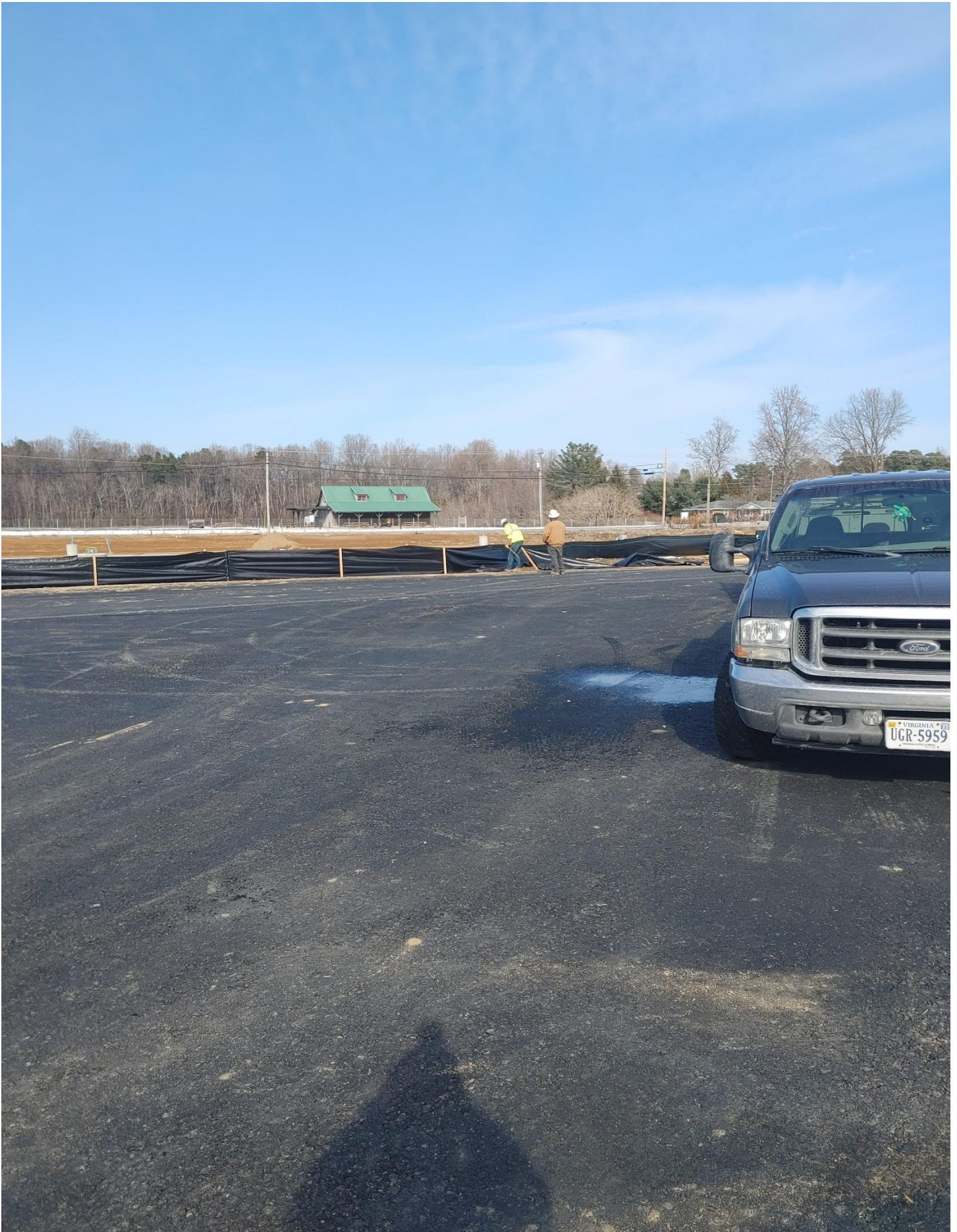
Photo 10 - Silt Fence is being erected around the site.
