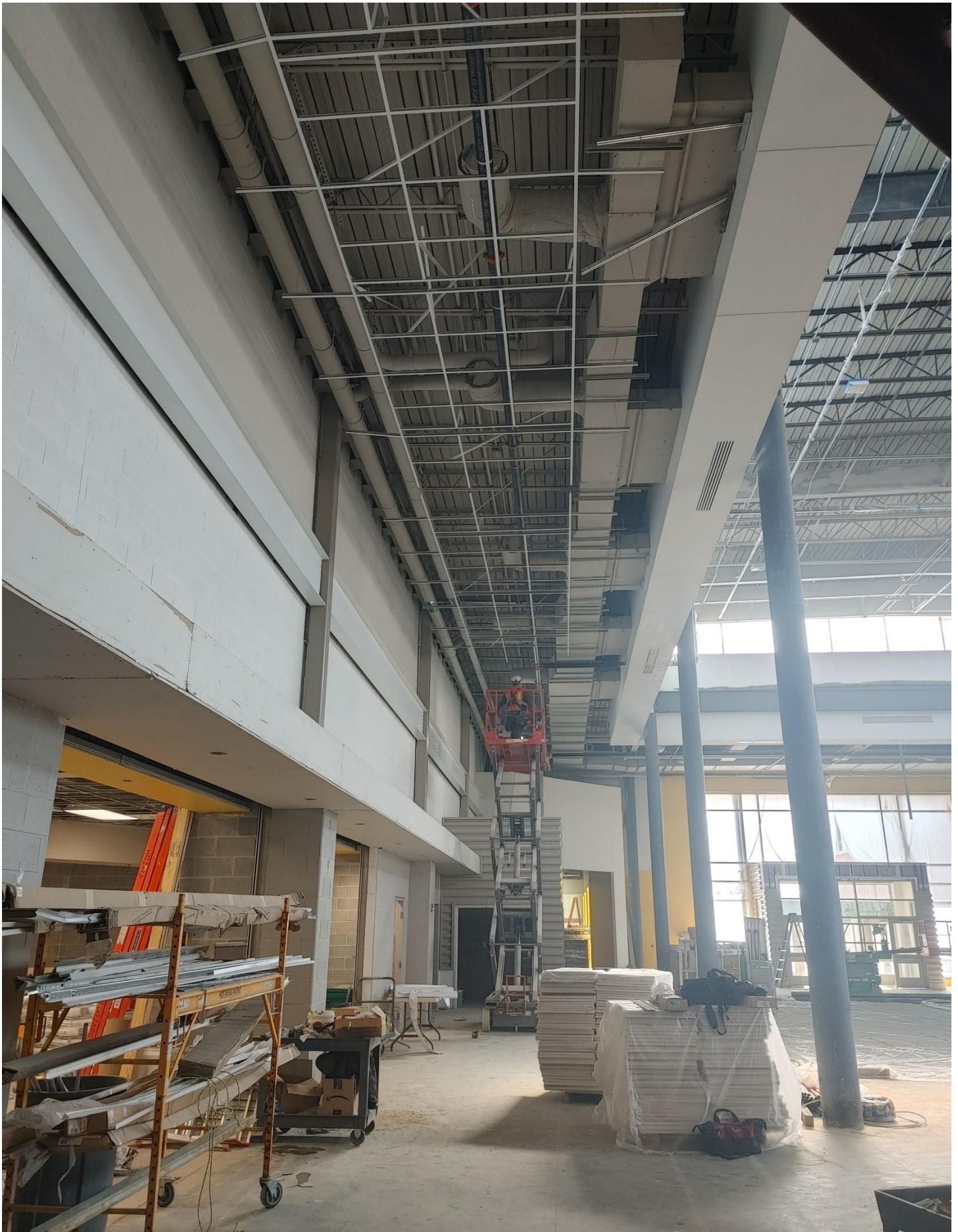
Photo 1 - Acoustical Cloud Ceiling is being installed in Area C
