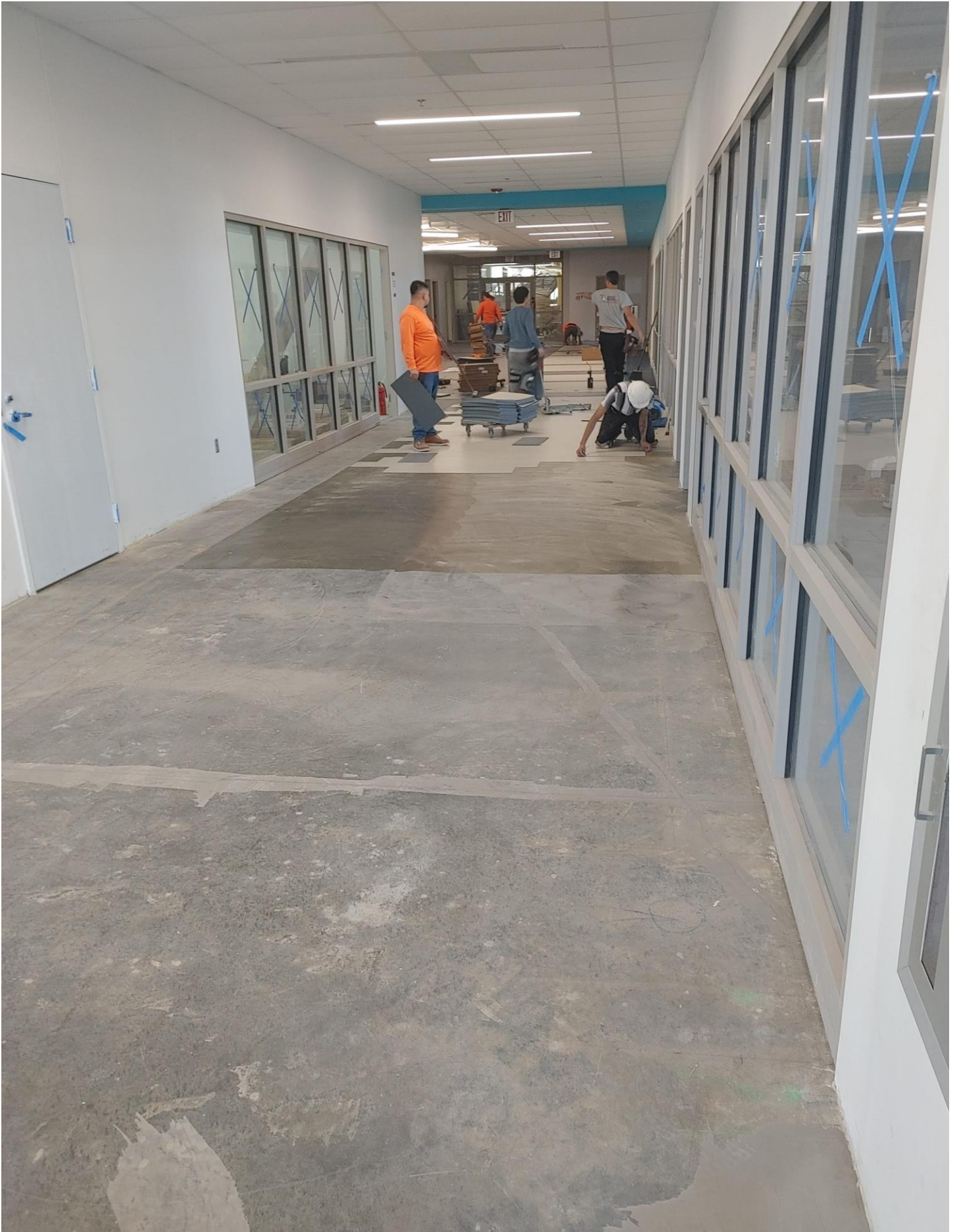
Photo 9 - VCT is being laid in A10 Design Commons
