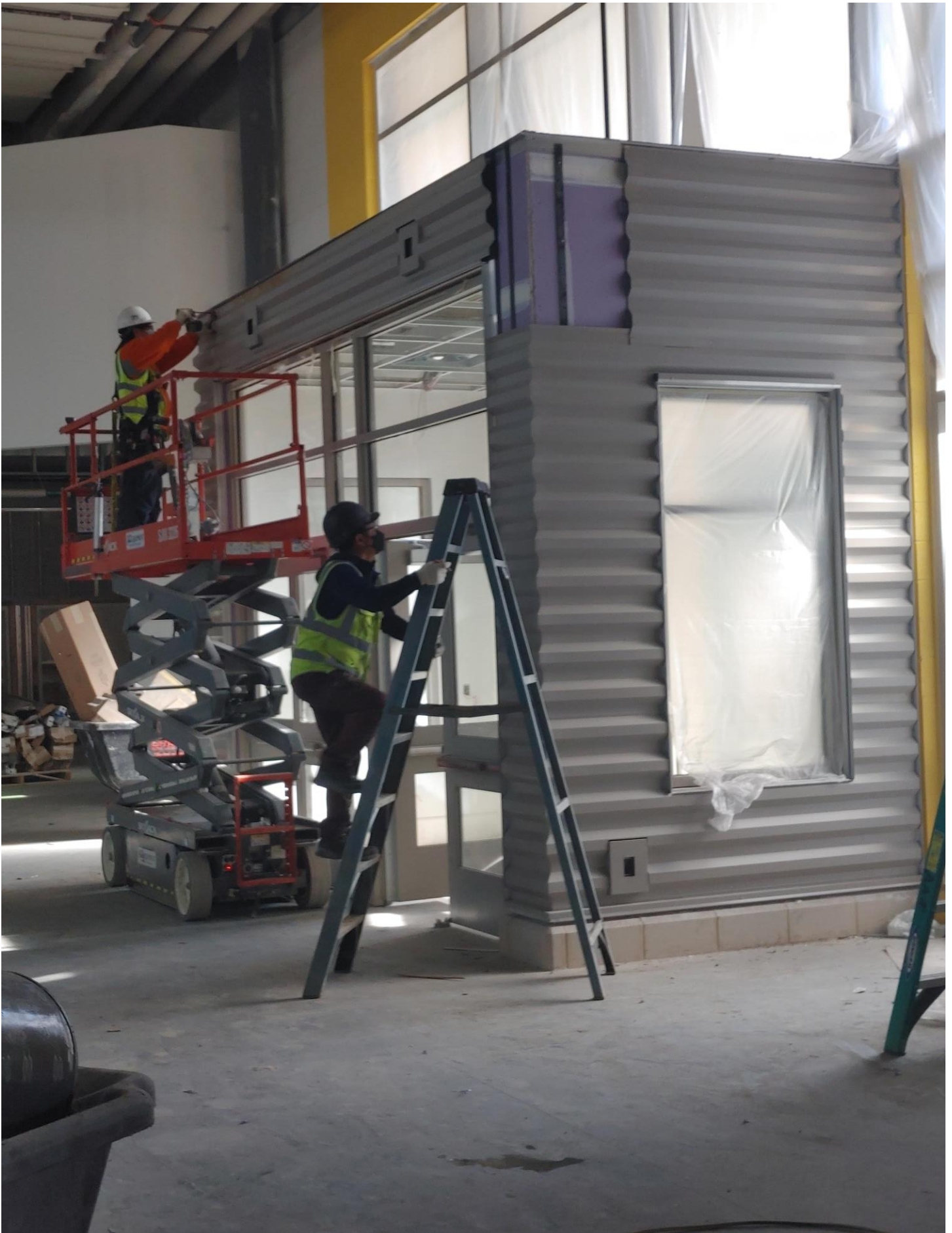
Photo 6 - Metal Panels are being installed in Area C.
