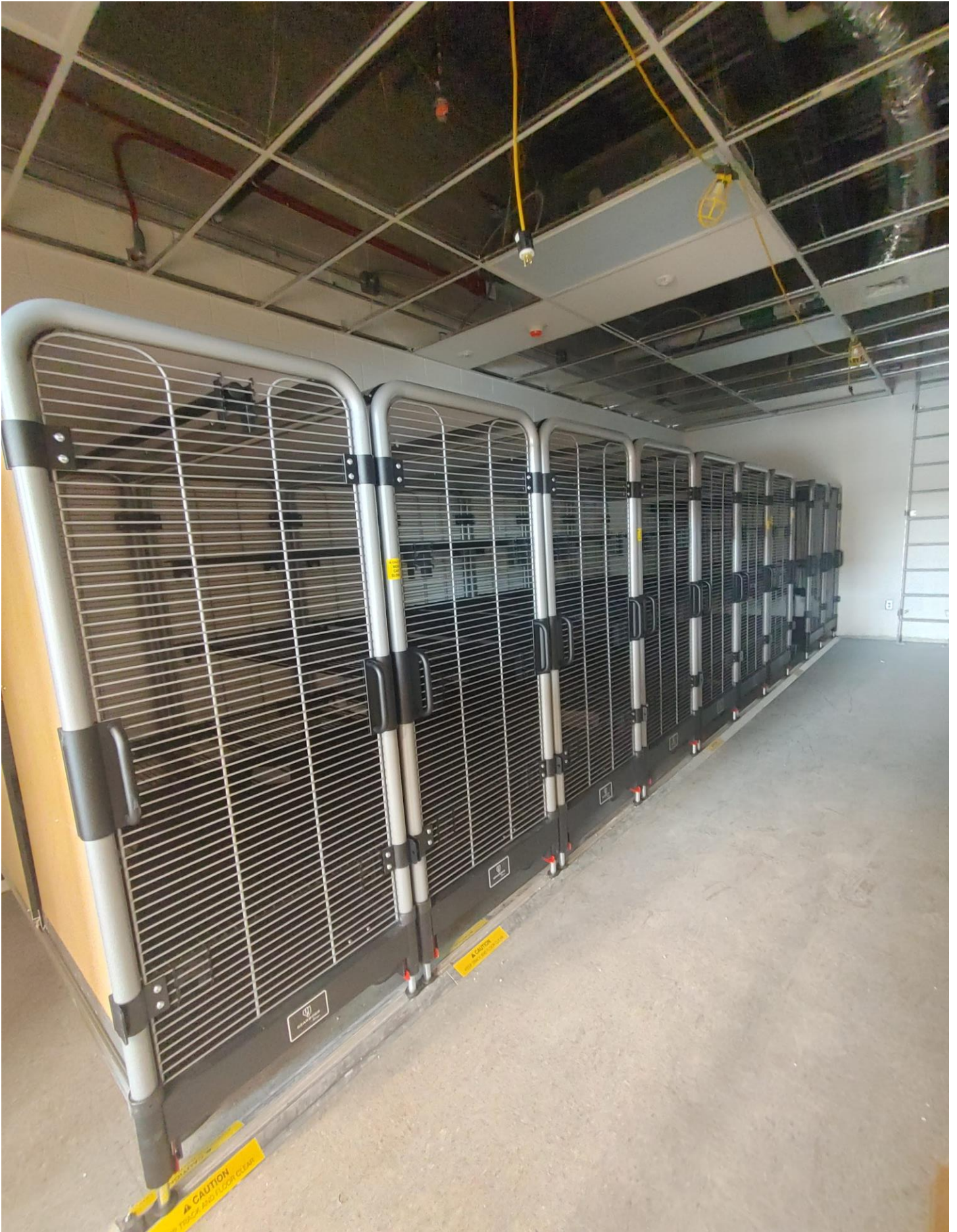
Photo 5 - Equipment Cages have been installed in Room E130
