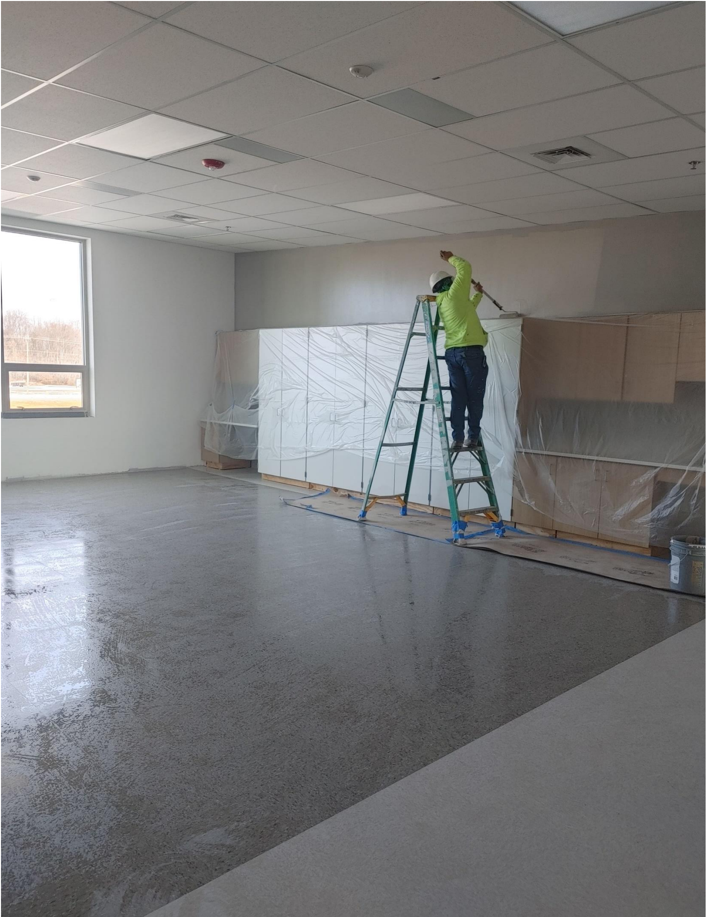
Photo 3 - Painter is painting in Area B
