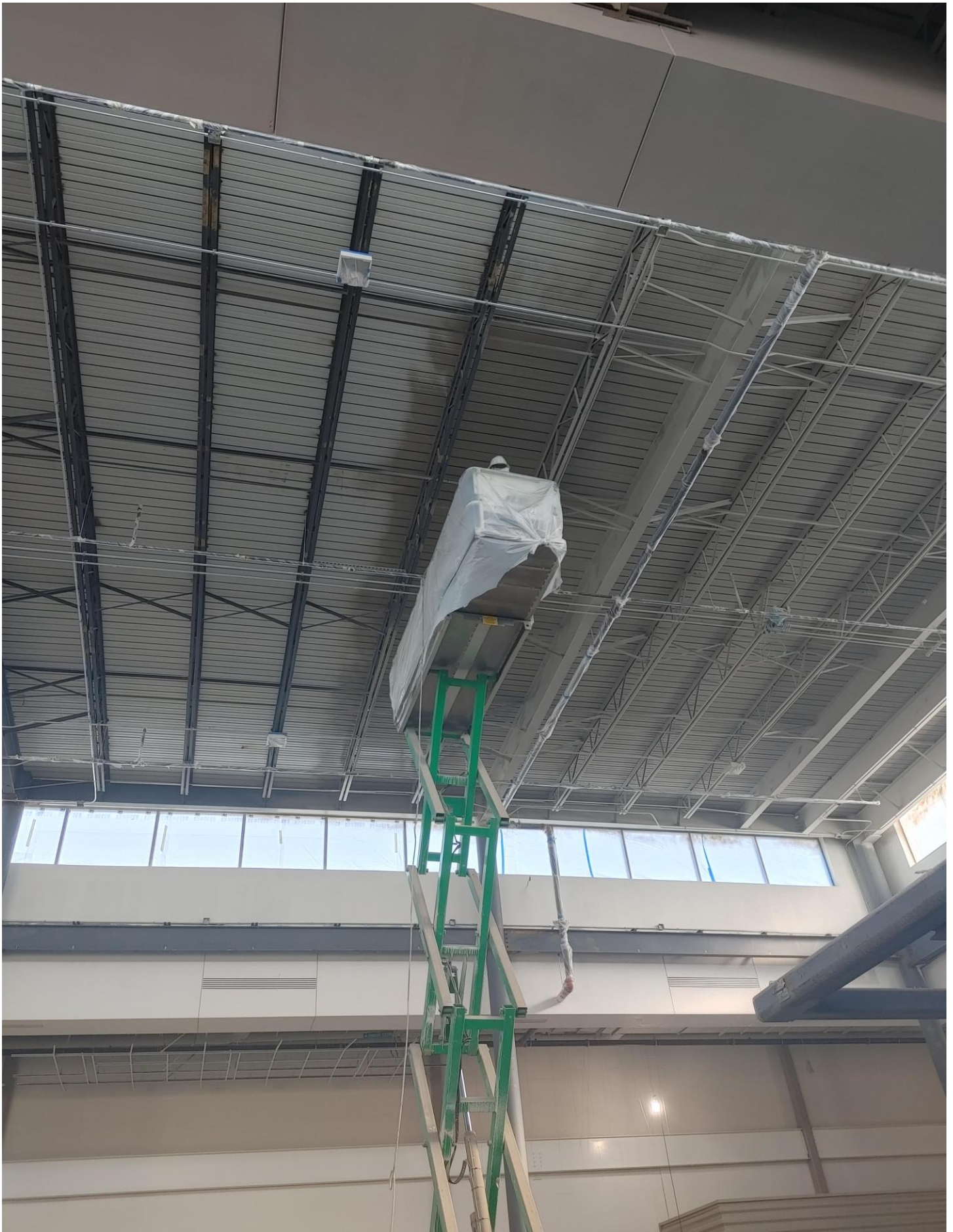
Photo 4 - Roof Deck is being painted in Area C.
