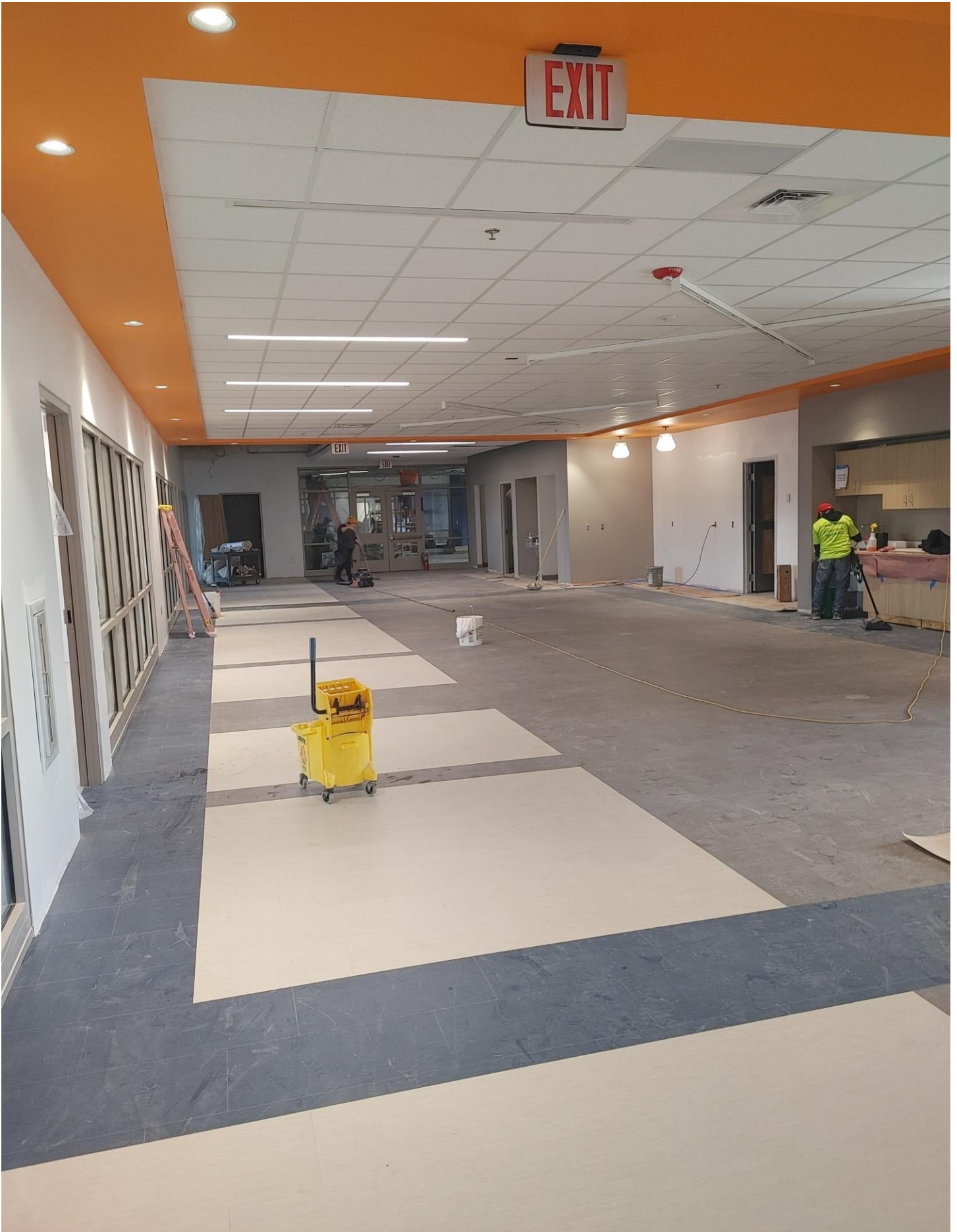
Photo 2 - 1st Floor, Area B, Room B10 - Design Commons
