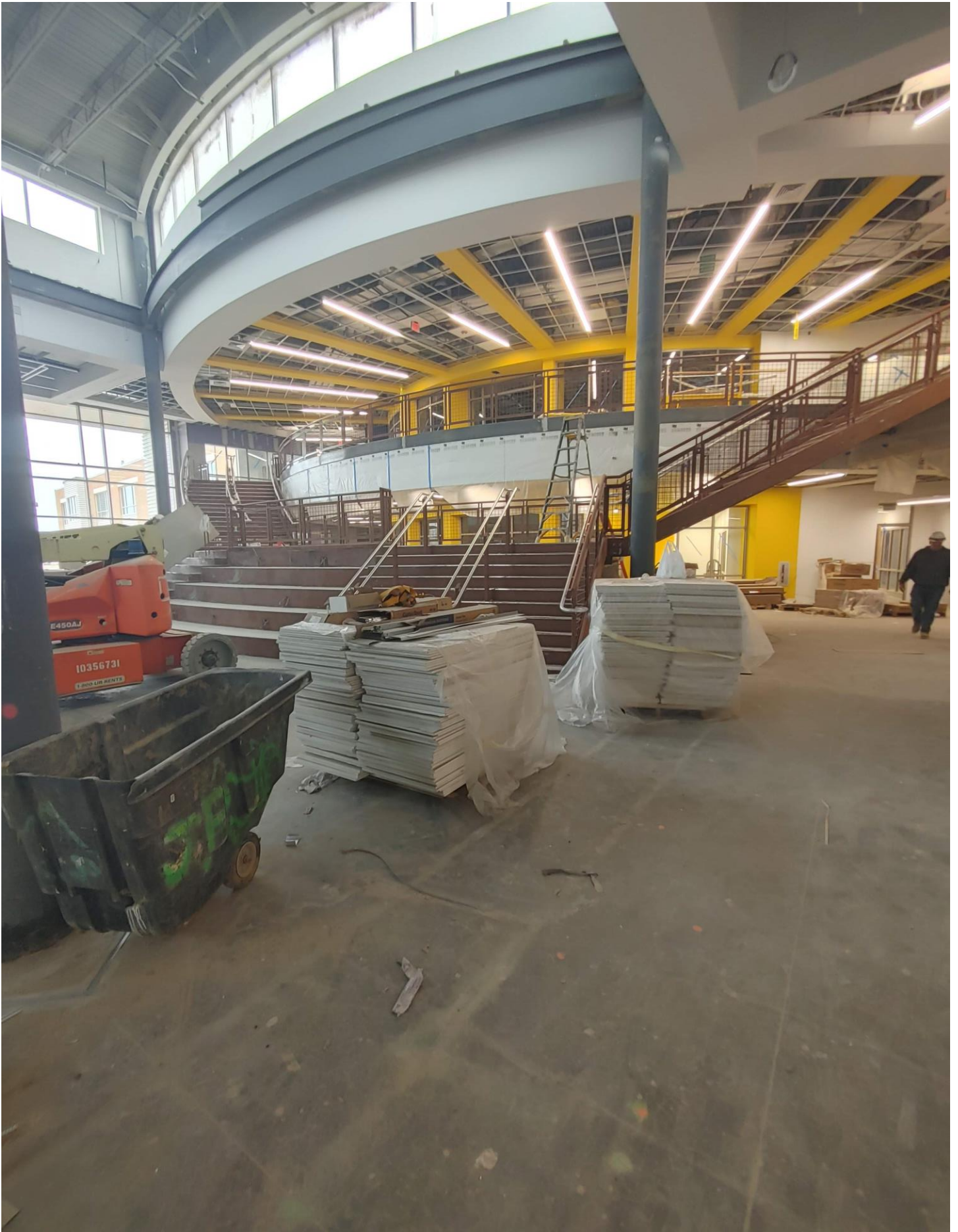
Photo 2 - Grand Staircase being prepped and painted
