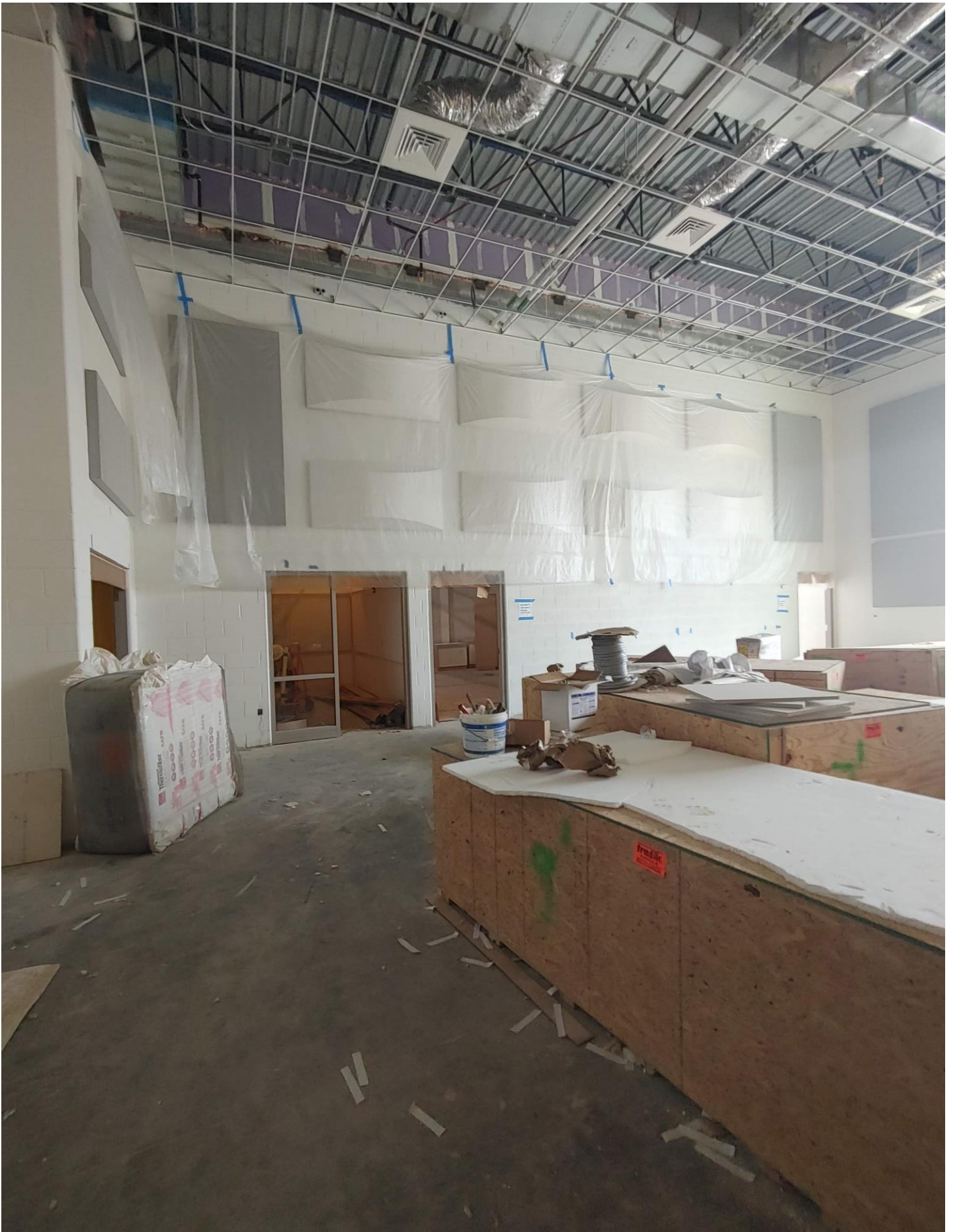
Photo 6 - Acoustical Panels have been hung on the East wall of D122
