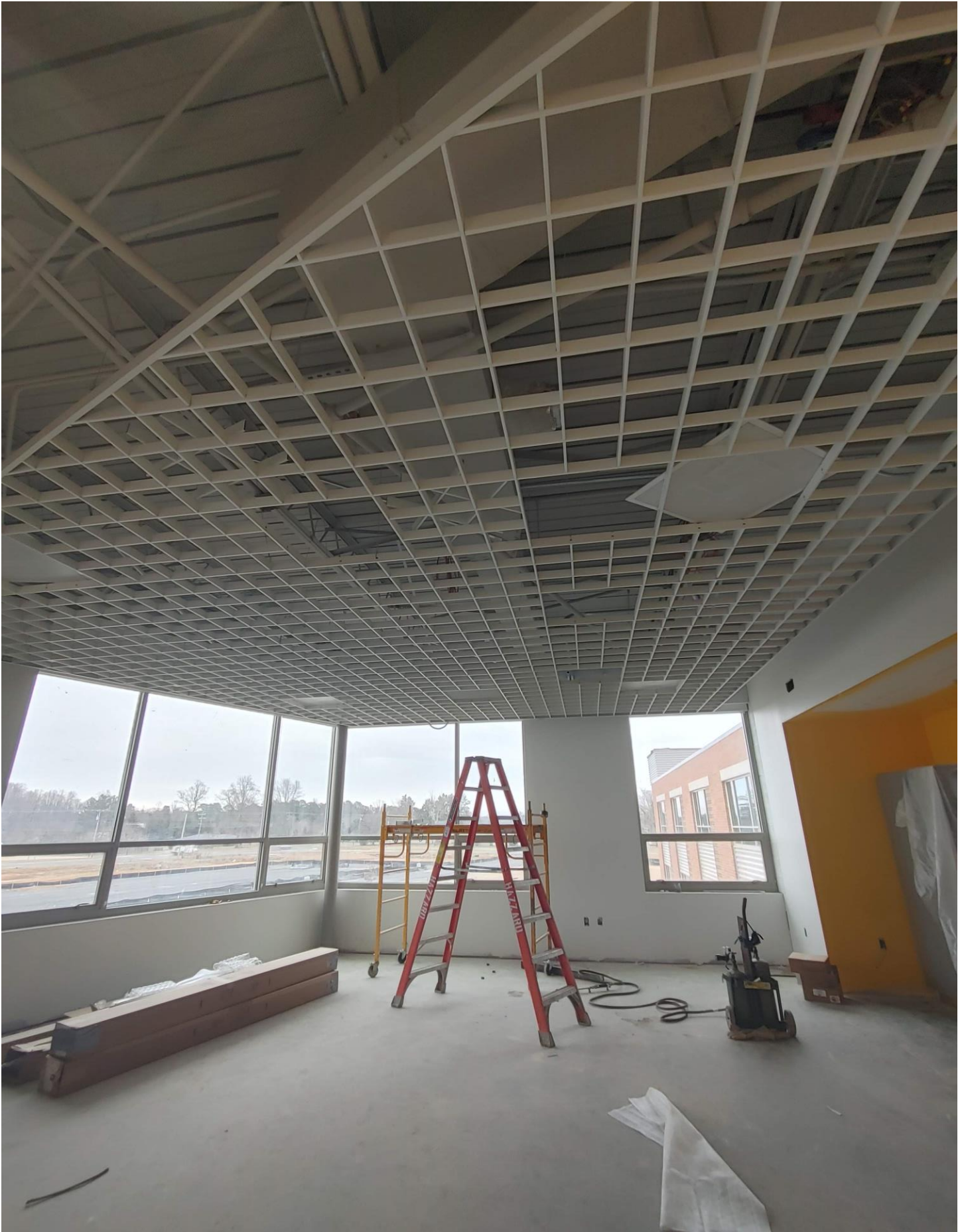
Photo 12 - Open Grid Ceiling in Room A224 has been installed.
