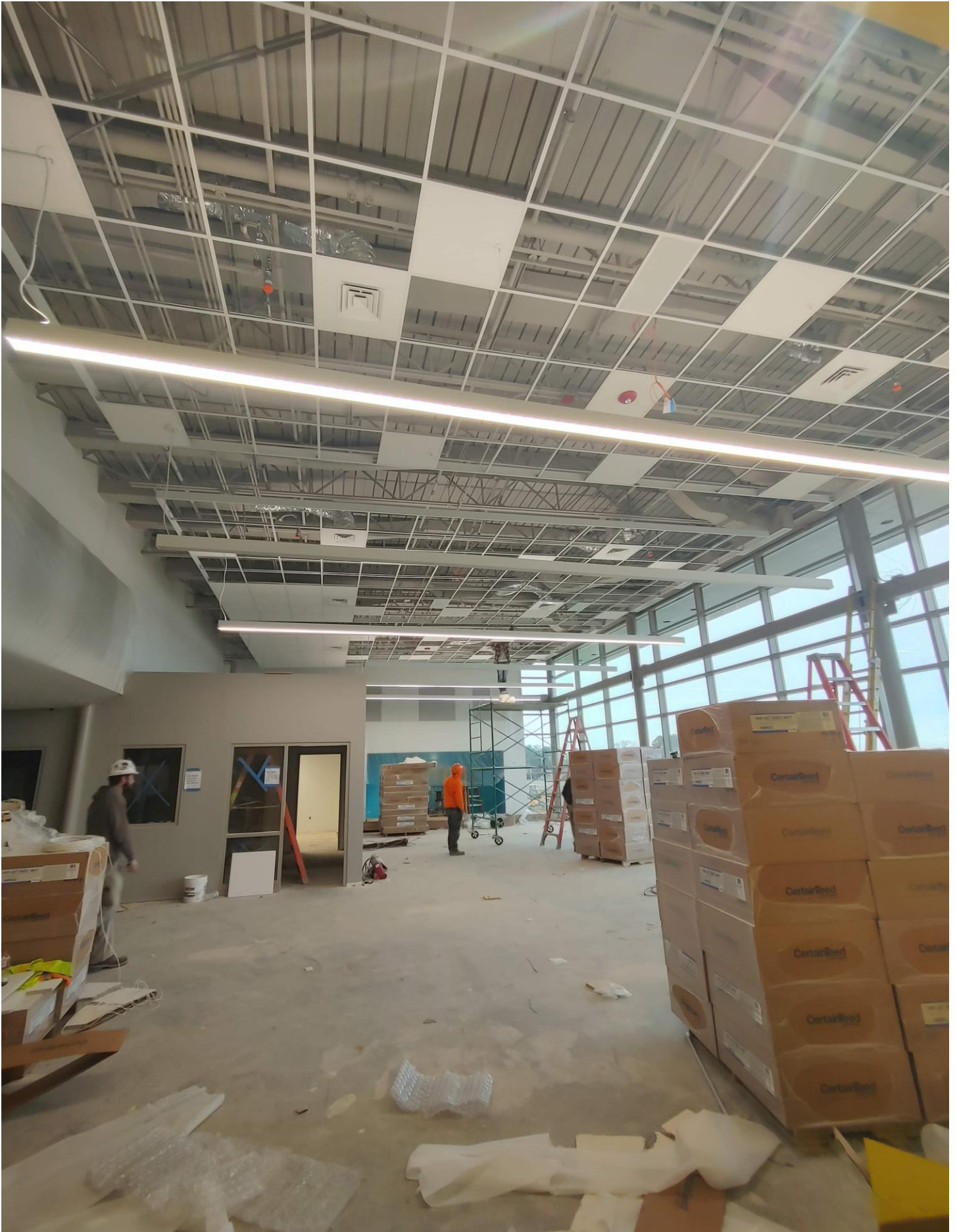
Photo 13 - Lights have been installed in Room A220
