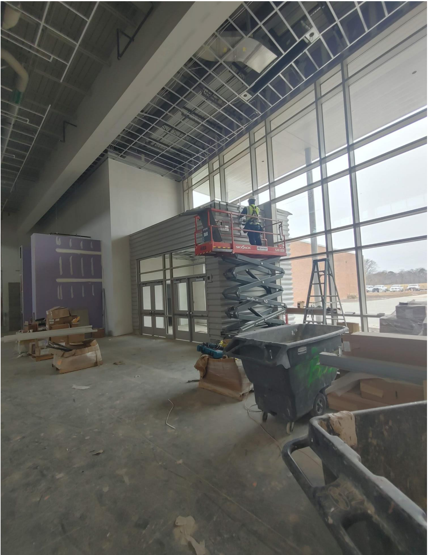
Photo 3 - Metal Panels are being installed on Vestibule C10
