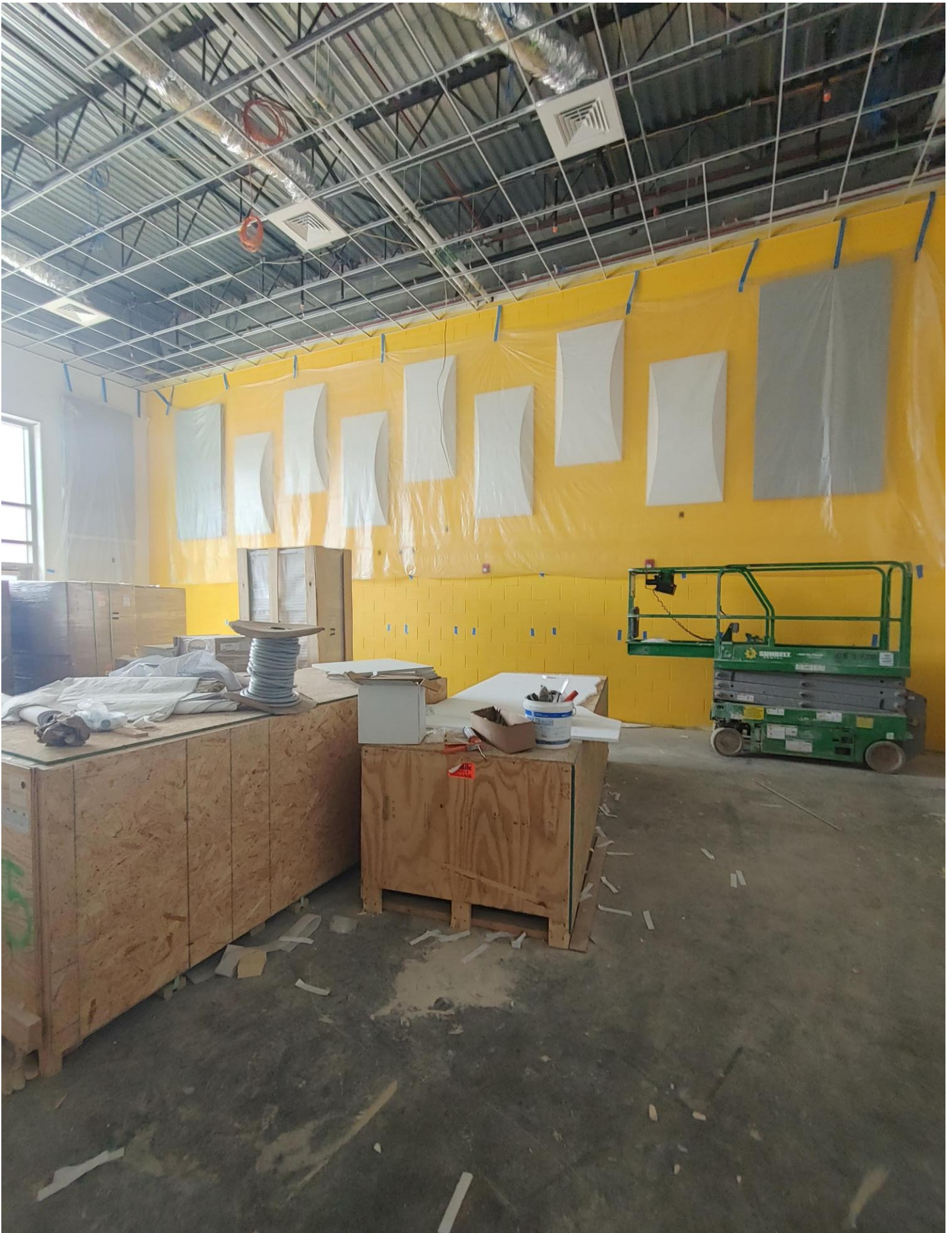
Photo 5 - Acoustical Panels have been installed on the west wall of D122
