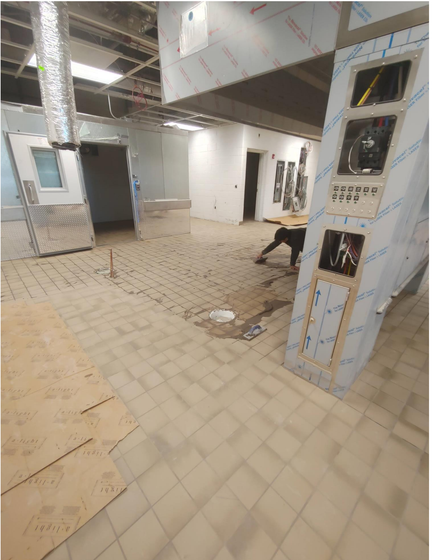
Photo 8 - Floor tile is being grouted in the Kitchen
