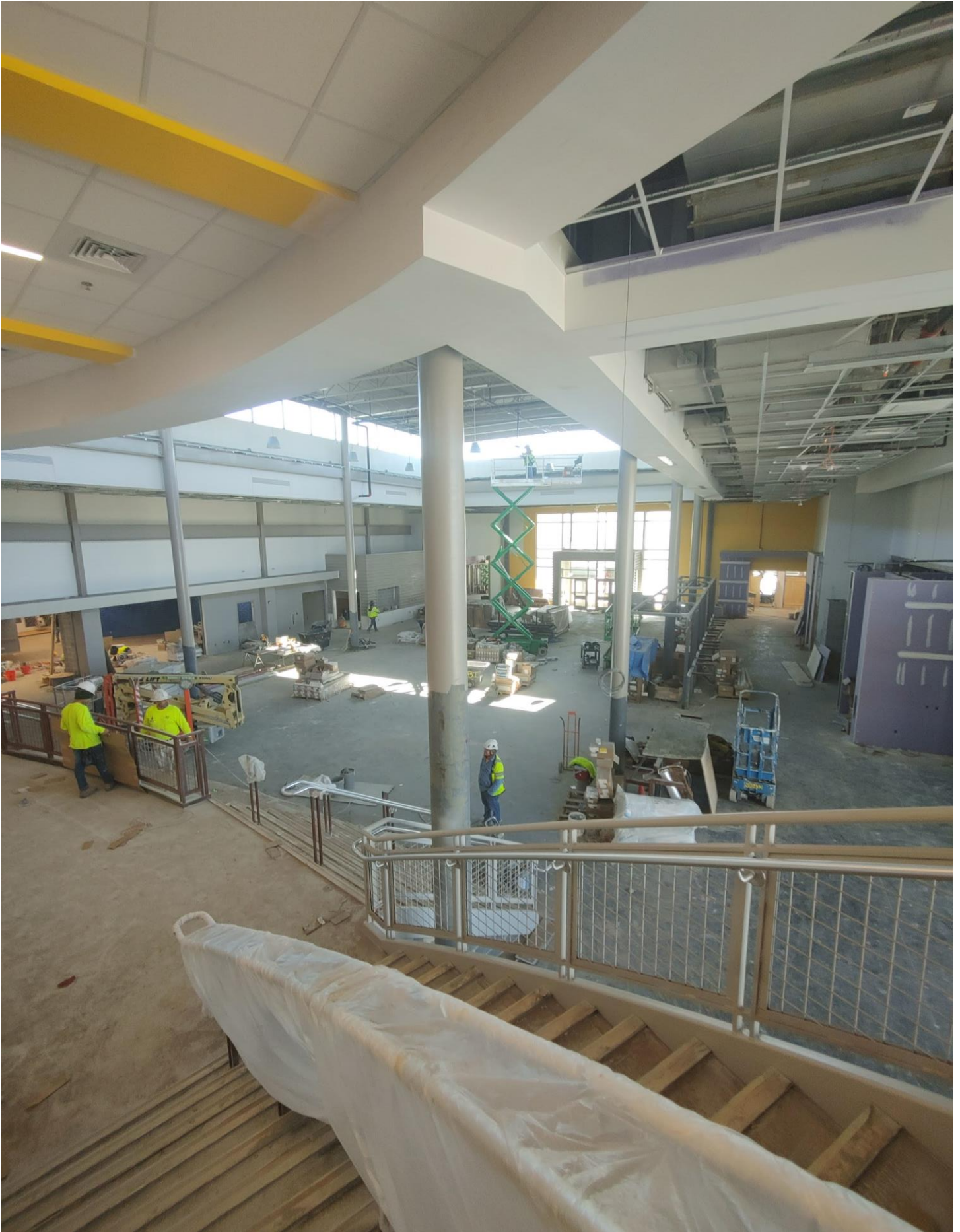
Photo 6 - Grand Staircase is being painted
