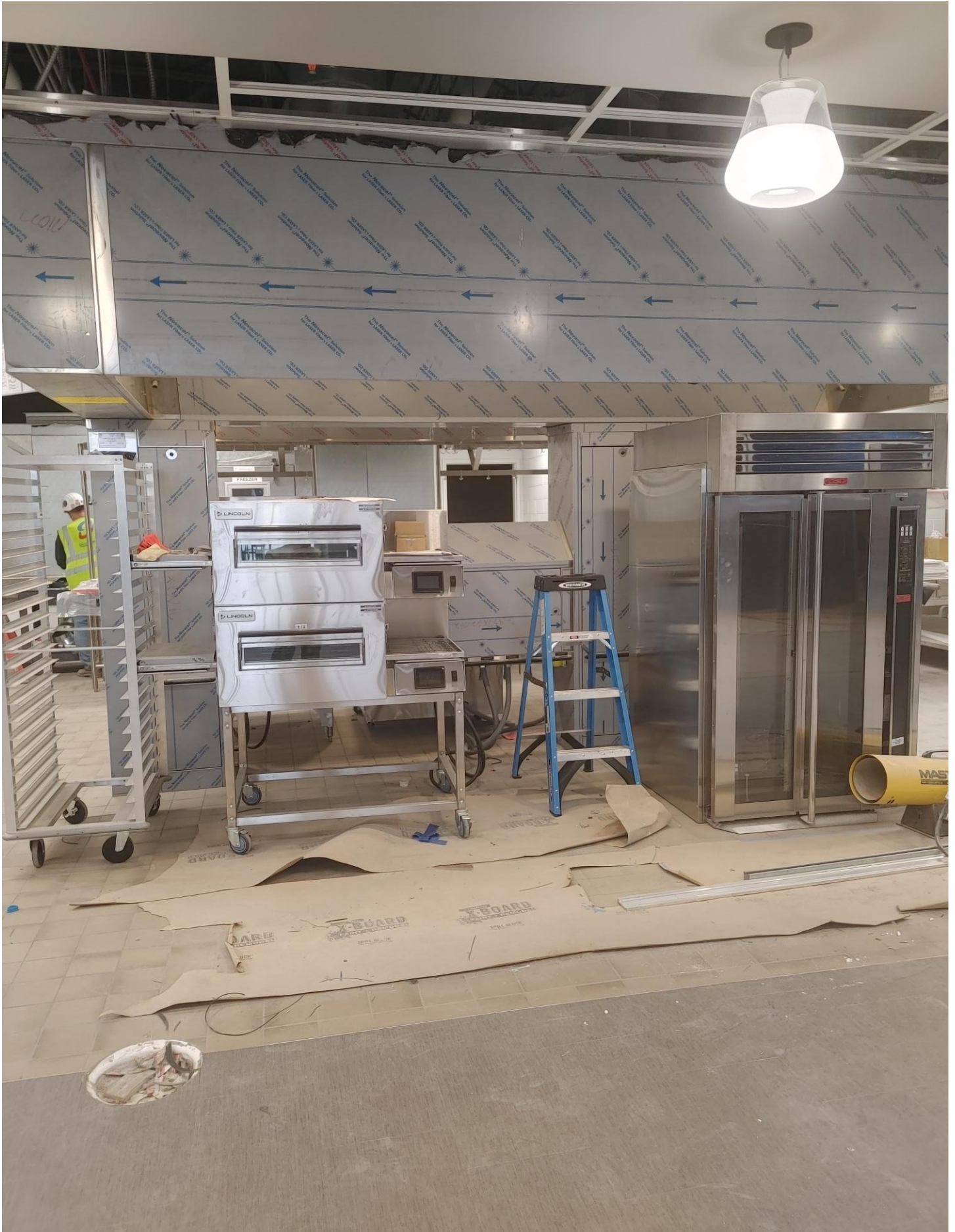
Photo 2 - Kitchen Equipment is being installed
