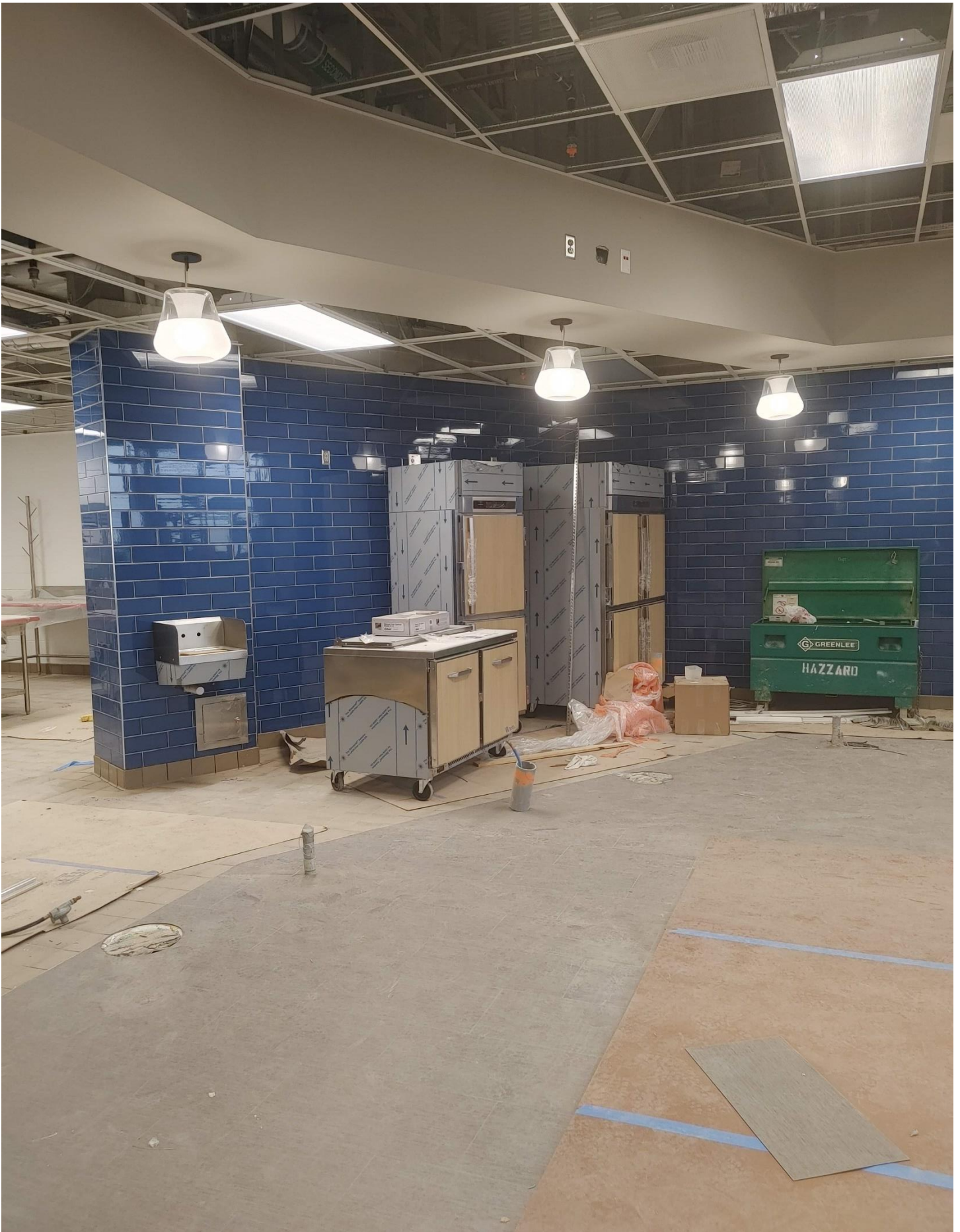
Photo 3 - Kitchen Equipment is being installed
