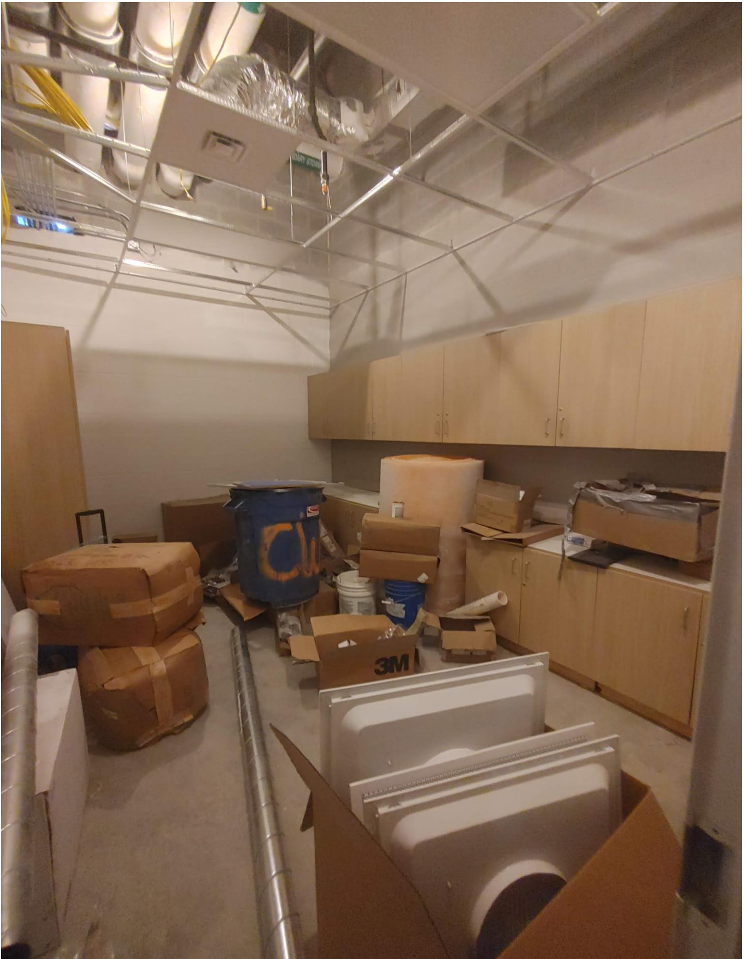
Photo 7 - Cabinetry has been installed in Room D153
