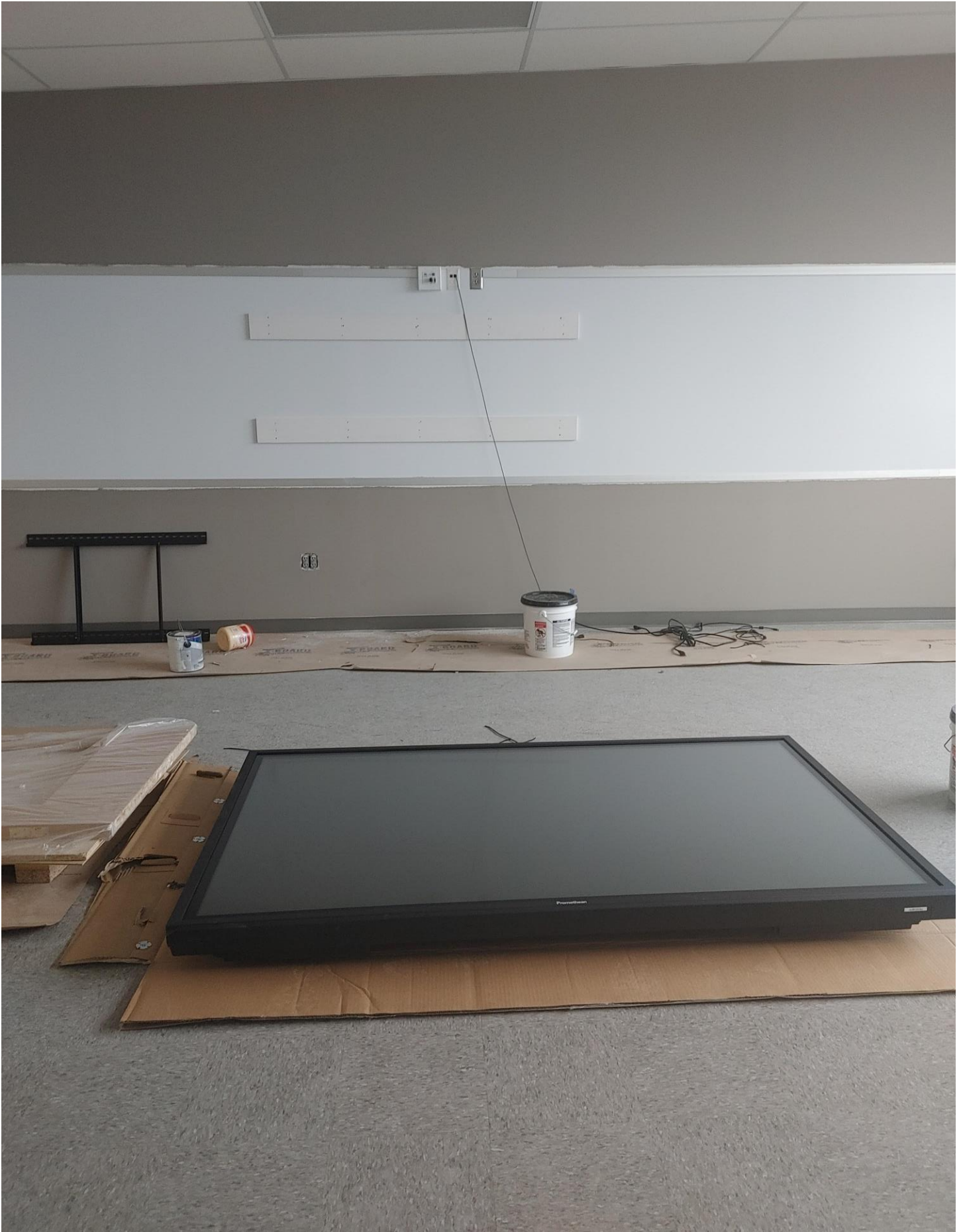
Photo 11 - Promethean Board stage and waiting to be hung on 2x4" mounting brackets
