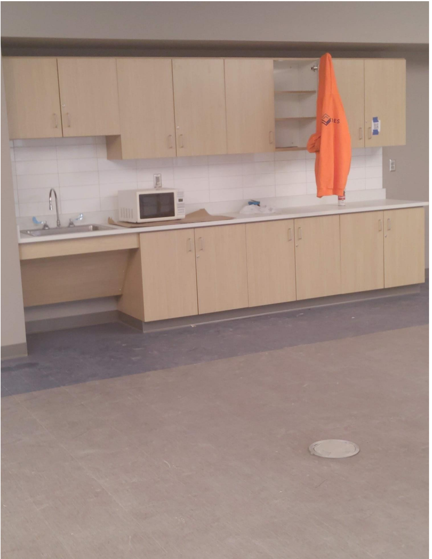
Photo 12 - Tile Backsplash has been laid in B10
