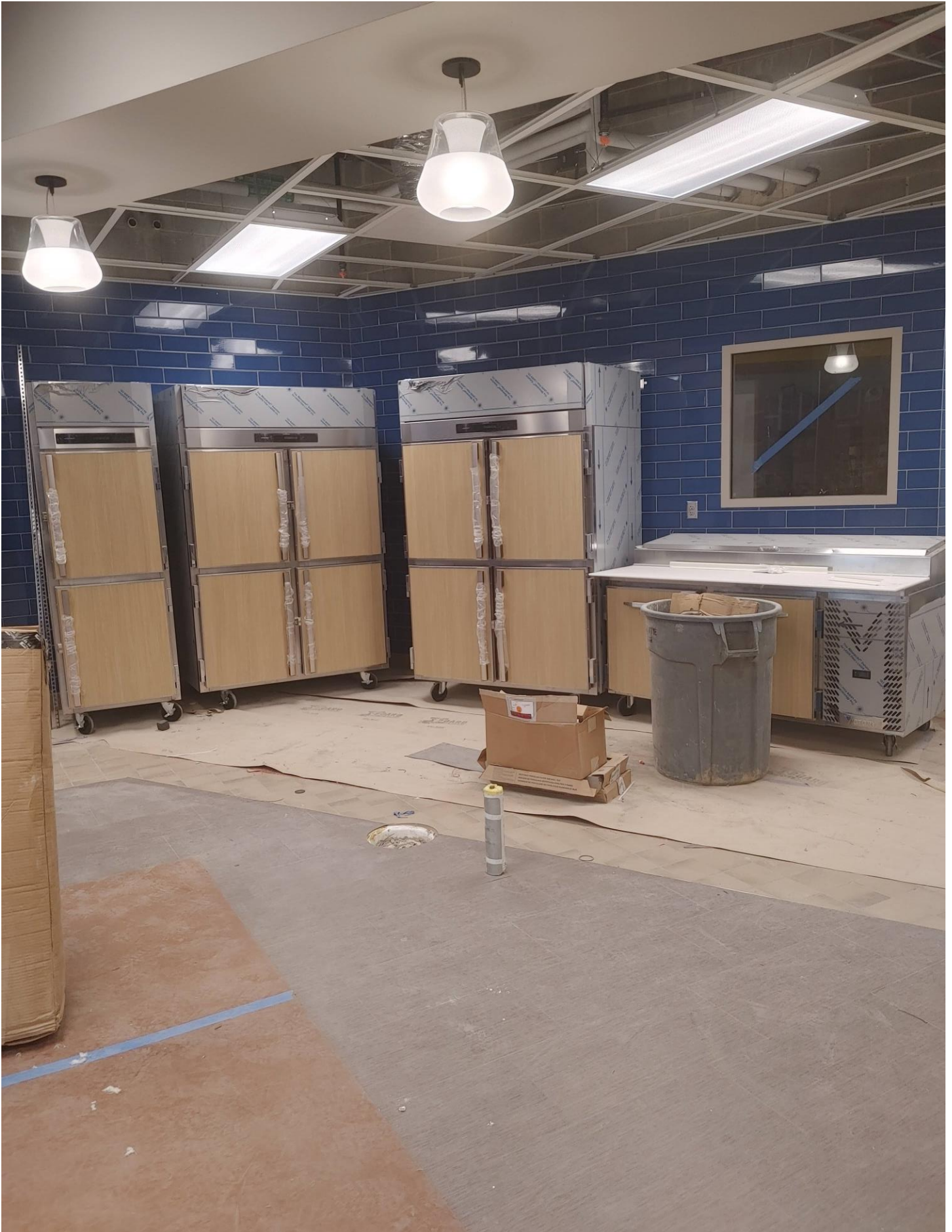
Photo 1 - Kitchen Equipment is being installed
