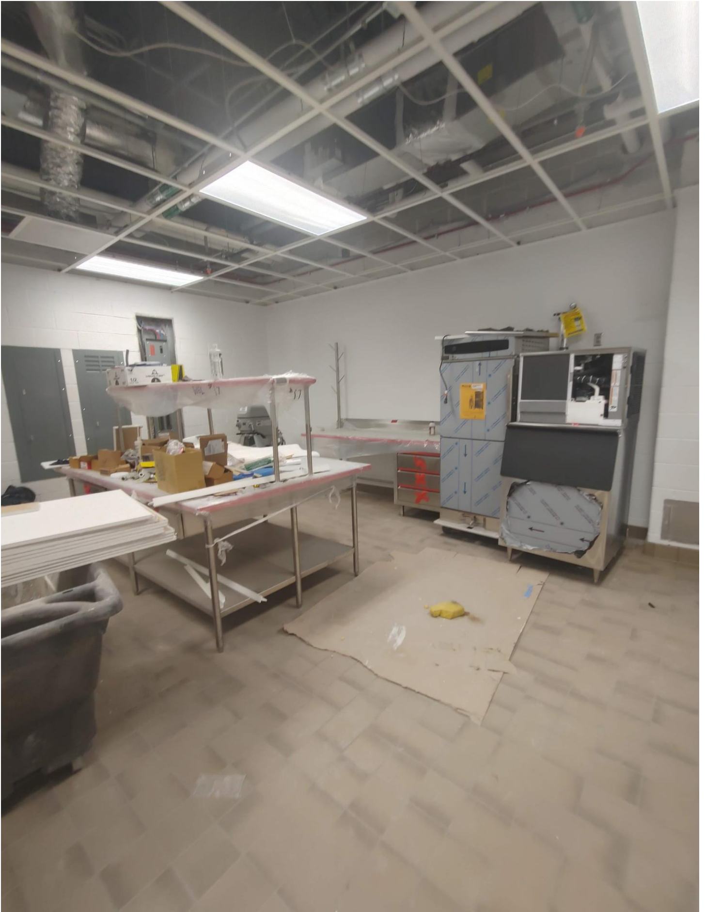
Photo 4 - Kitchen Equipment is being installed
