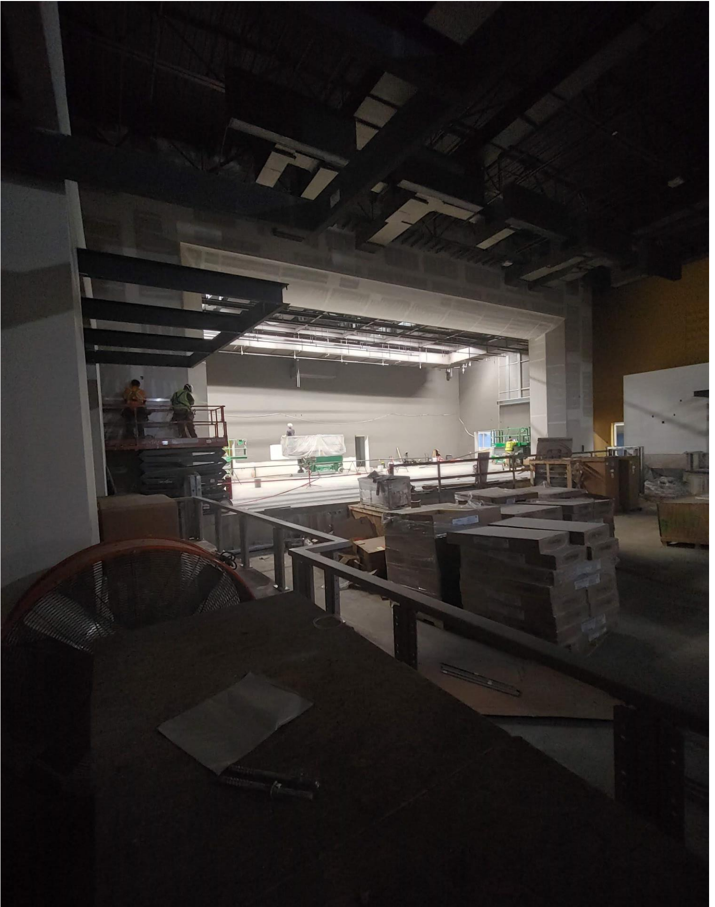
Photo 8 - Walls being finished and Painted in the Auditorium
