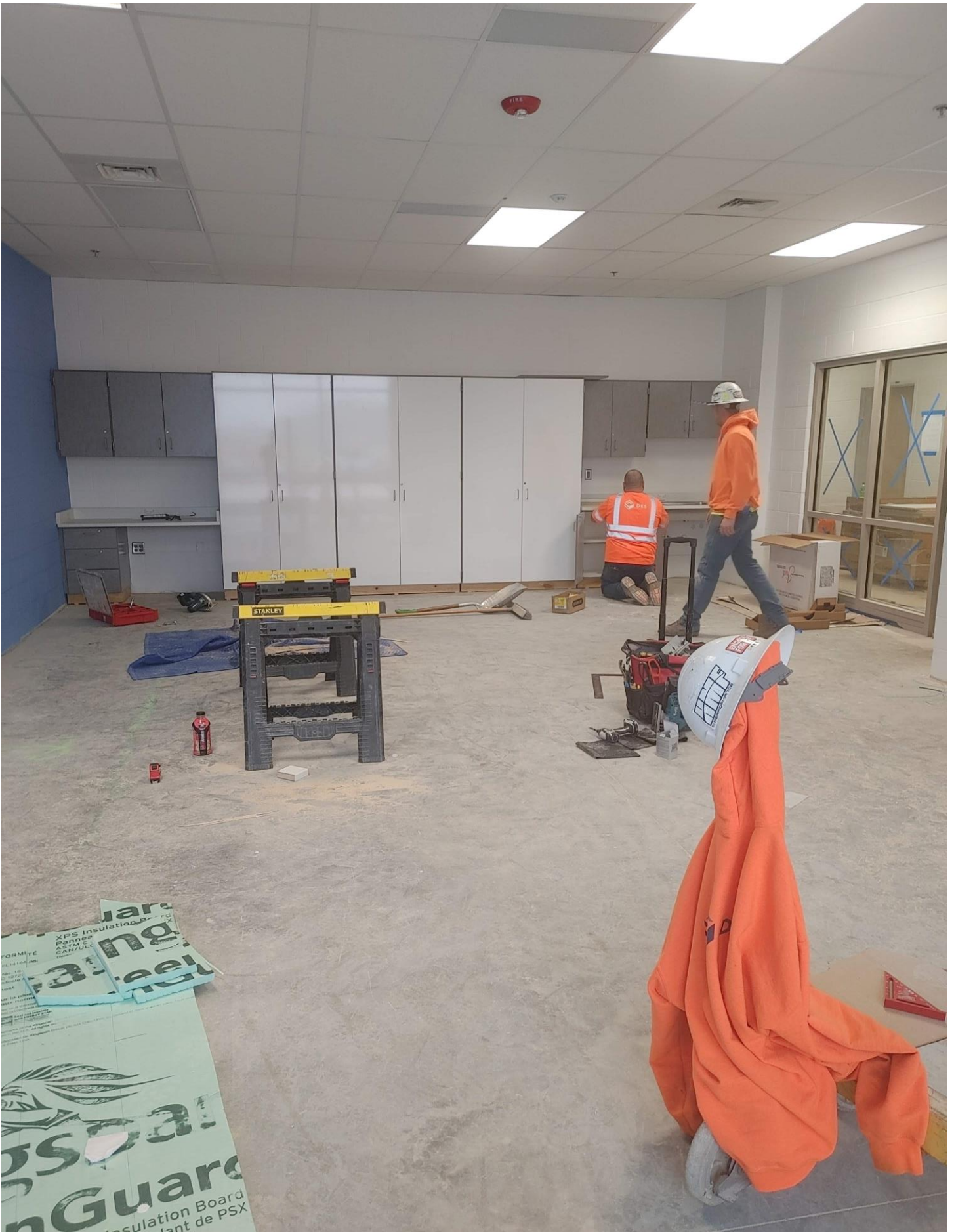
Photo 10 - Cabinetry is being installed in Room E132
