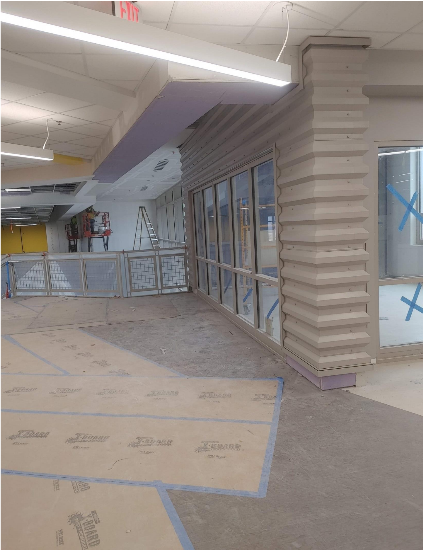
Photo 14 - Ceiling being finished in Area C
