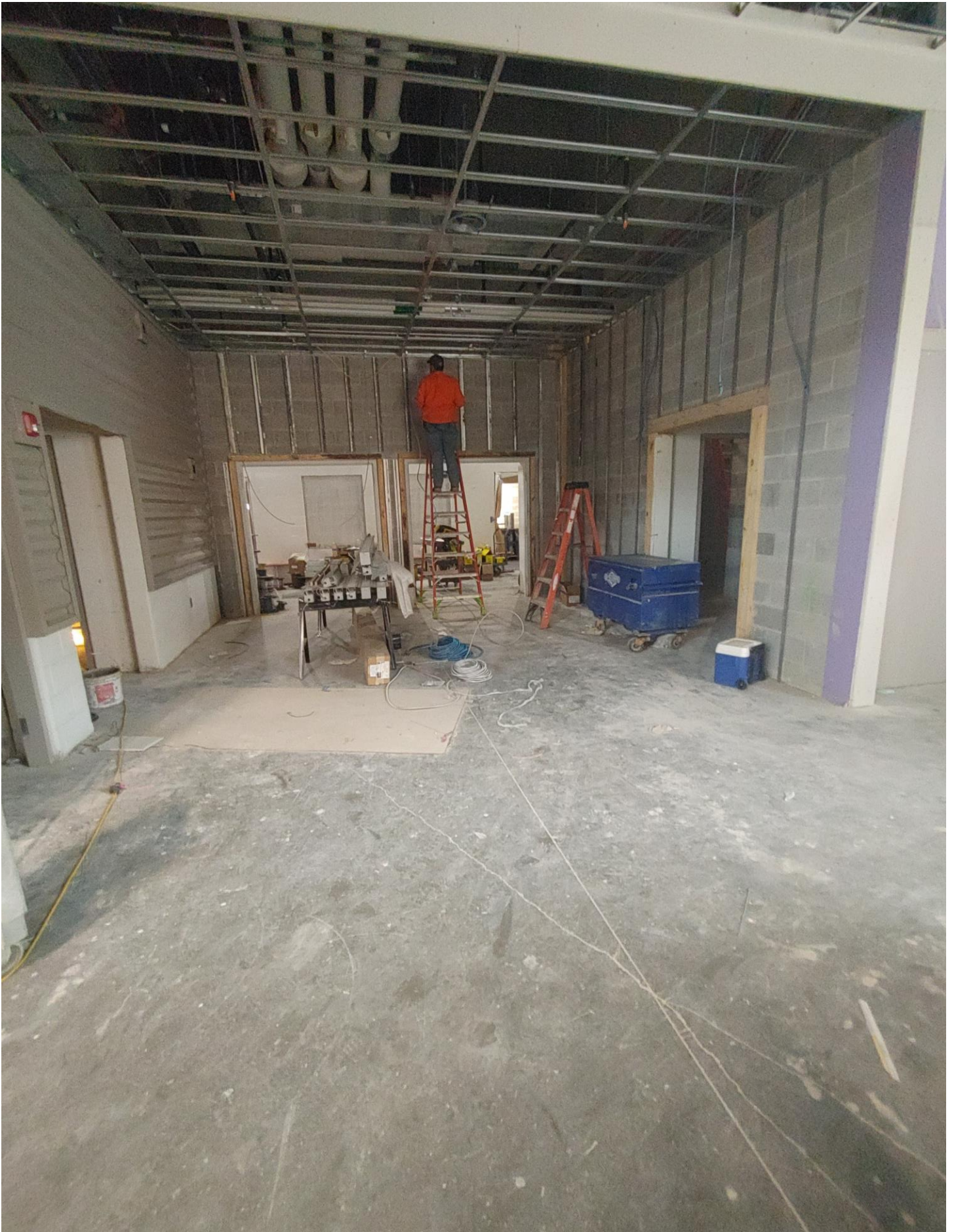
Photo 9 - Entrance to Auditorium
