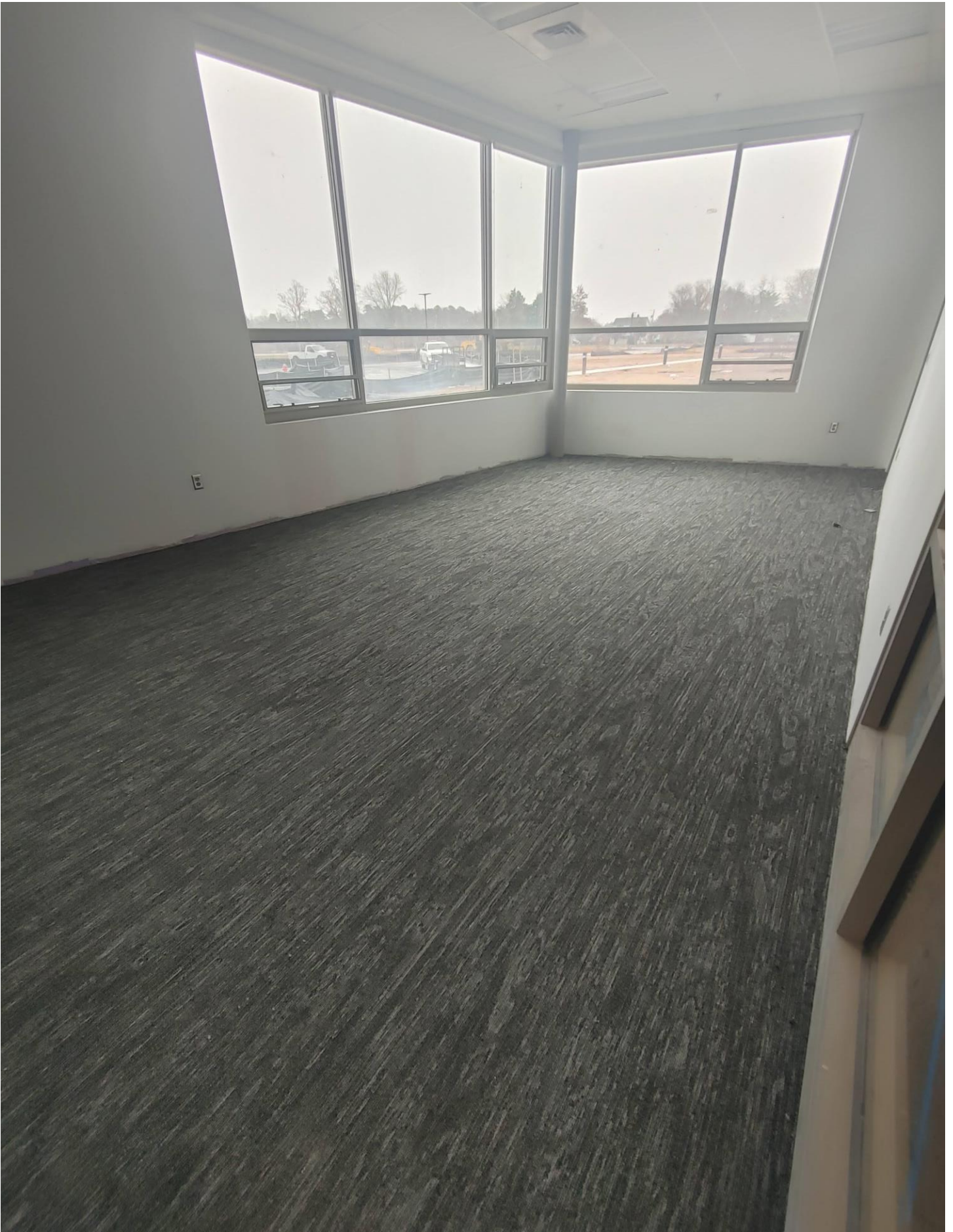
Photo 3 - Carpet has been installed in the Administrative Office area.
