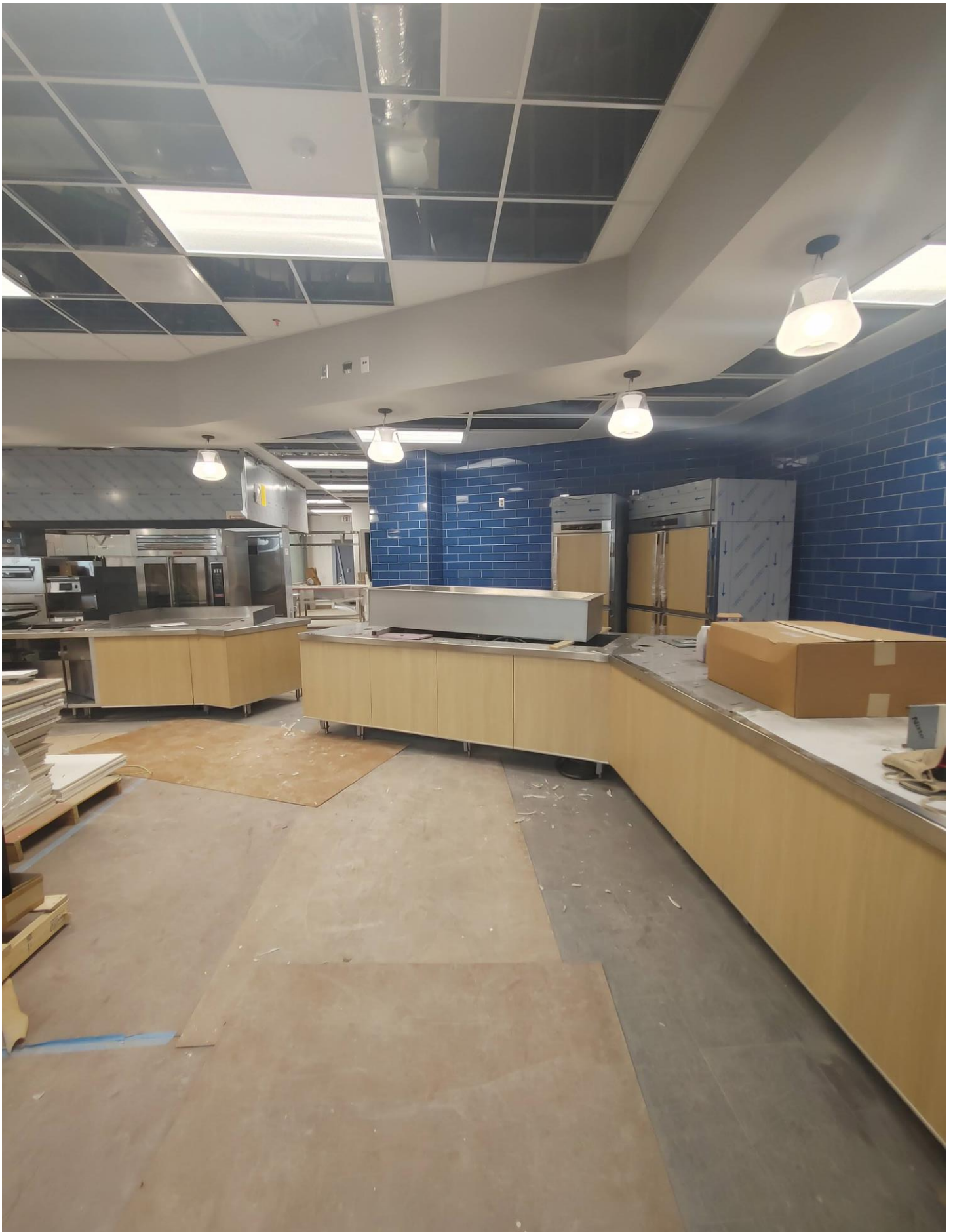
Photo 2 - Equipment continues to be installed in the Kitchen
