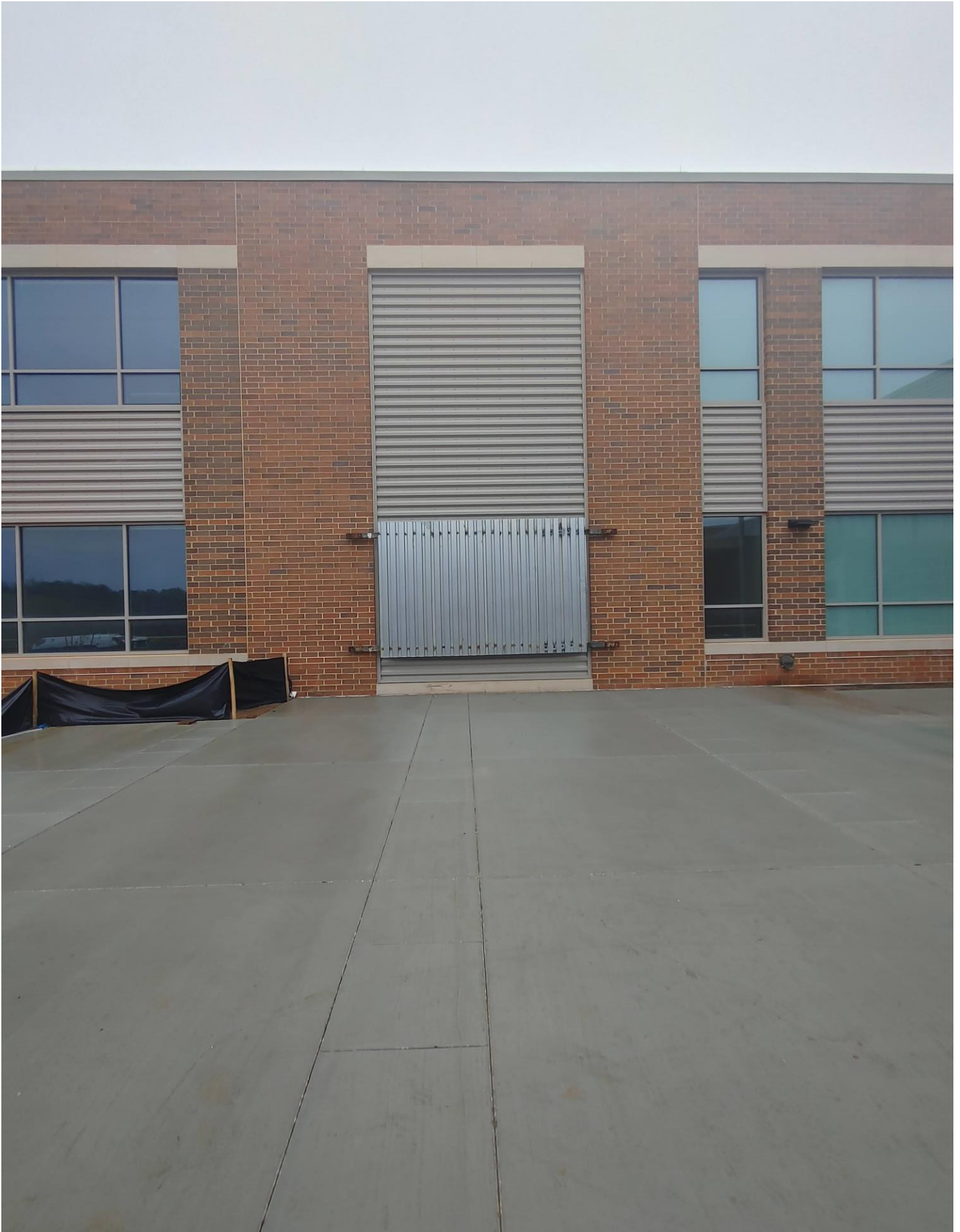
Photo 1 - Galvanized Panel installed - Student Entrance area.
