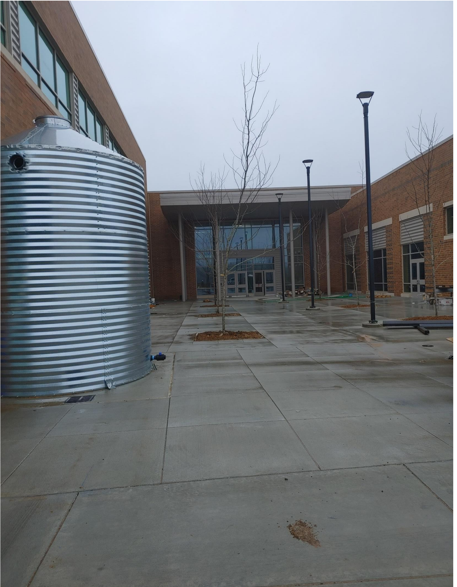
Photo 15 - Light poles installed and trees planted on South Entrance
