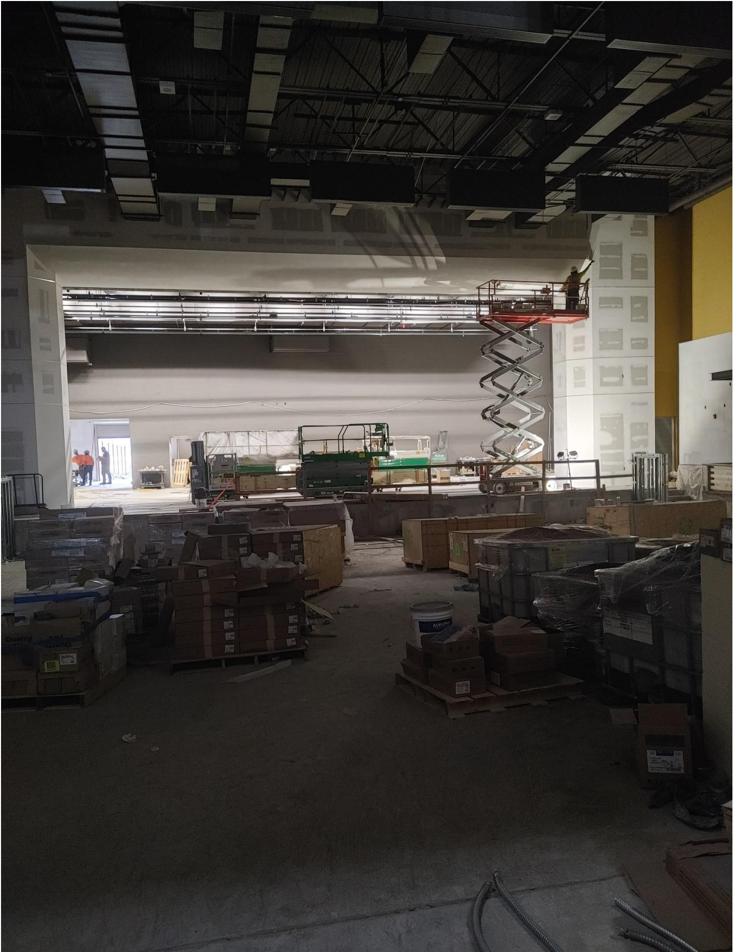
Photo 10 - Shetrock is being finished in Auditorium
