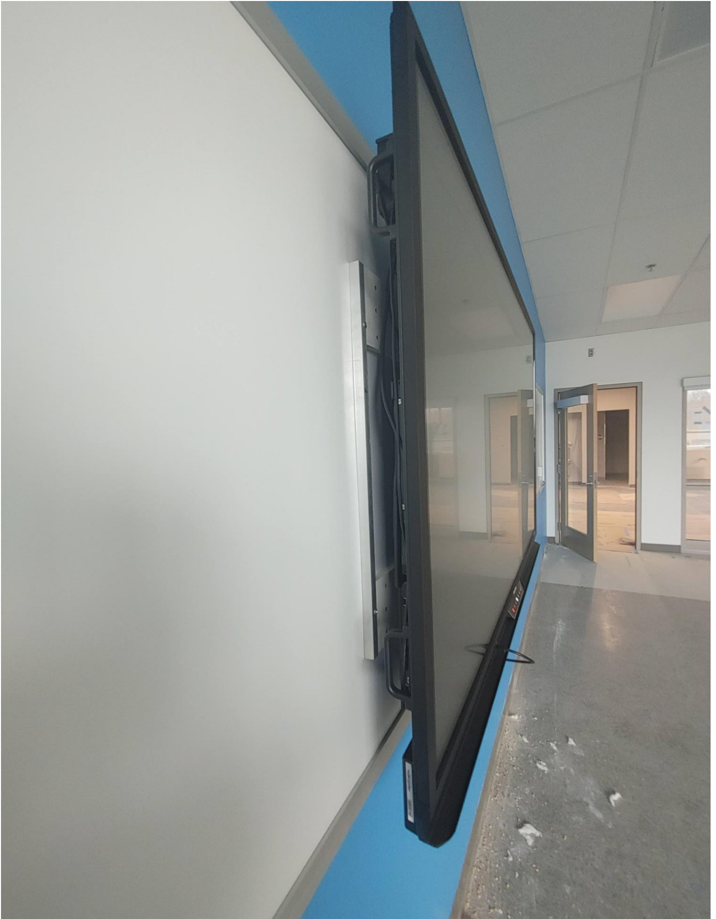
Photo 5 - Promethean Board has been mounted.
