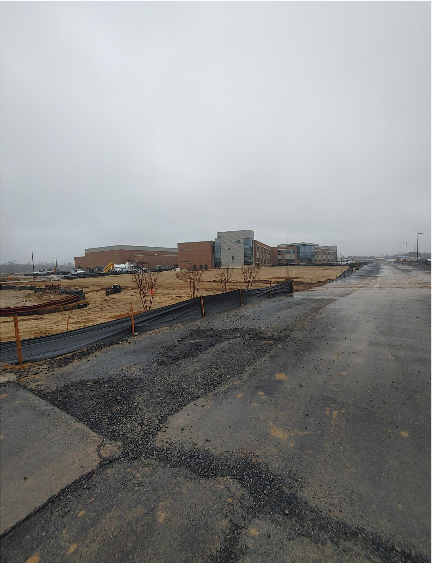
Photo 18 - Northeast view of site
