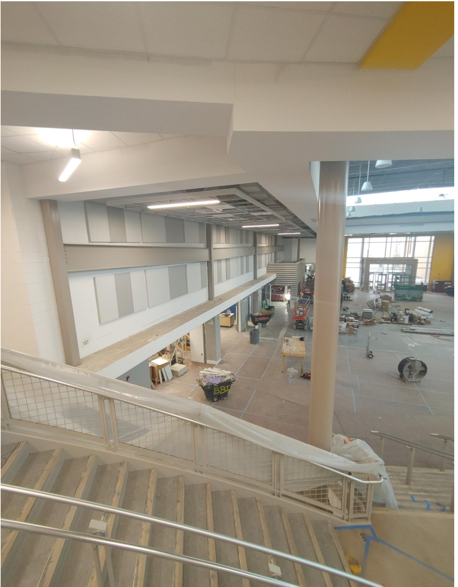
Photo 8 - Acoustical Panels hung in Area C
