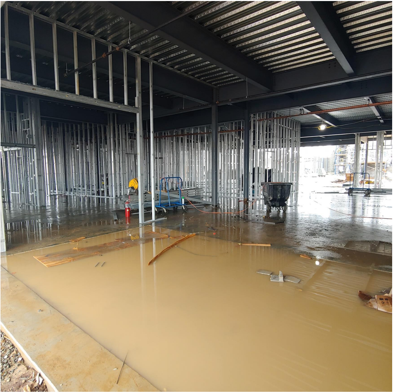
Photo 4 - Framing continues in the Administrative Office area of Area A
