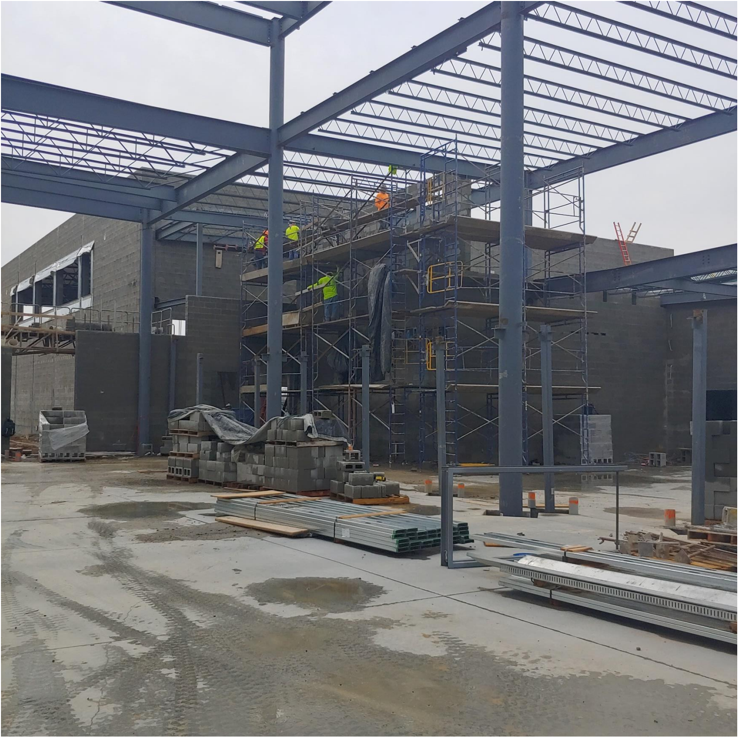
Photo 6 - Block being laid in Area D
