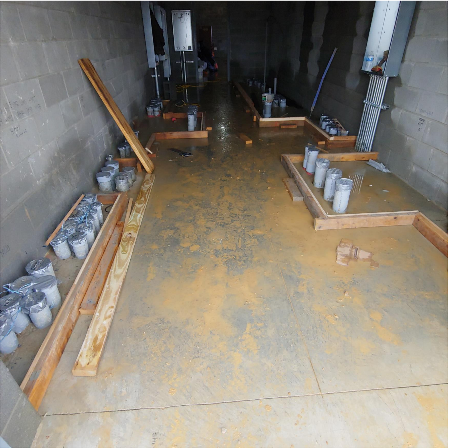
Photo 8 - Forms being constructed in electrical room for raised slabs
