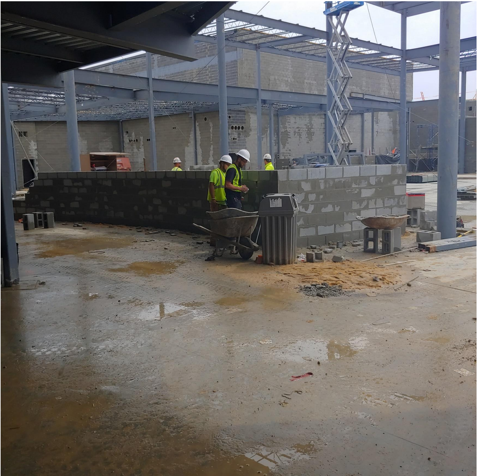
Photo 5 - Stair #3 being constructed
