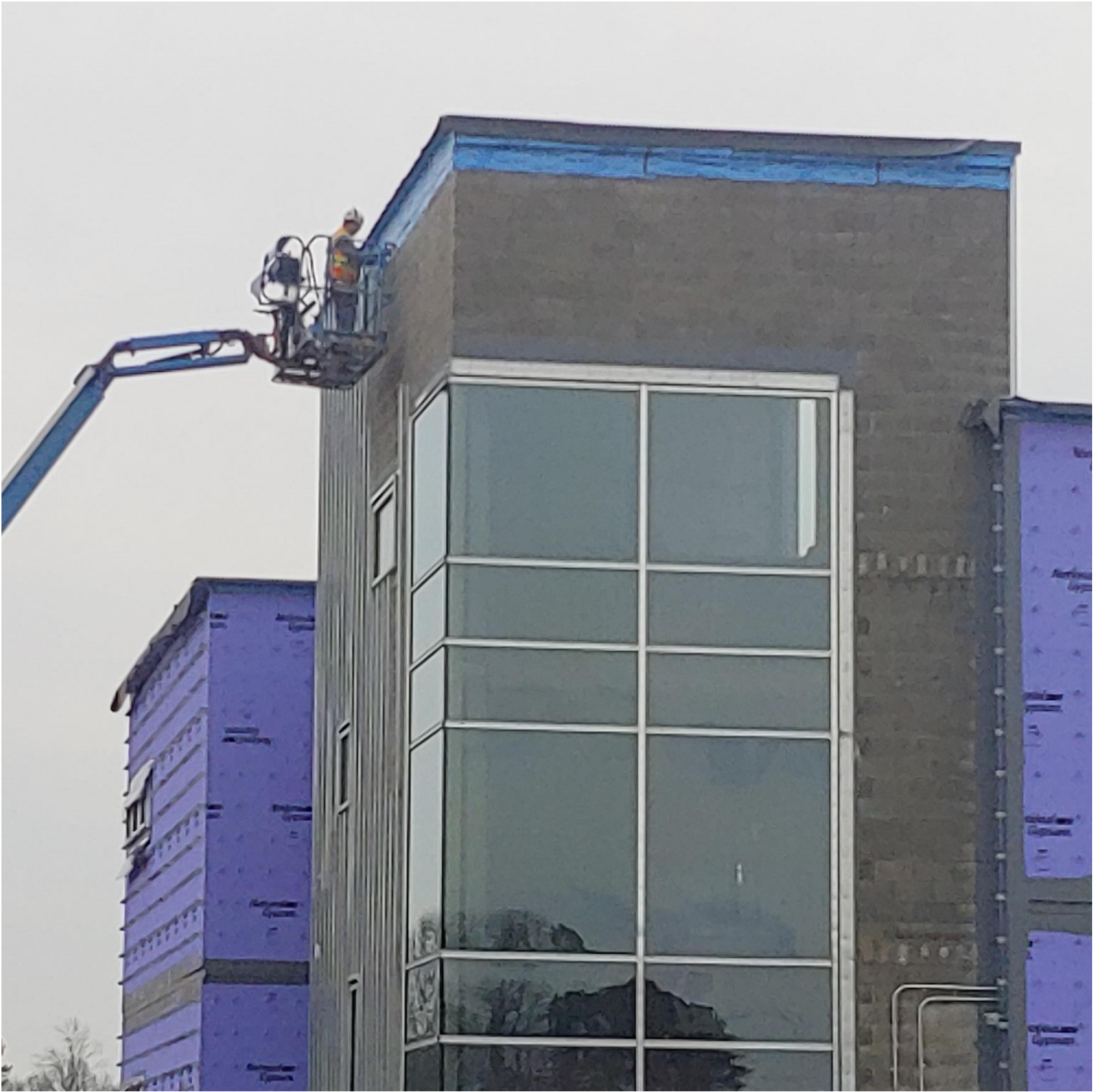
Photo 2 - Flashing being installed - Stairwell #1
