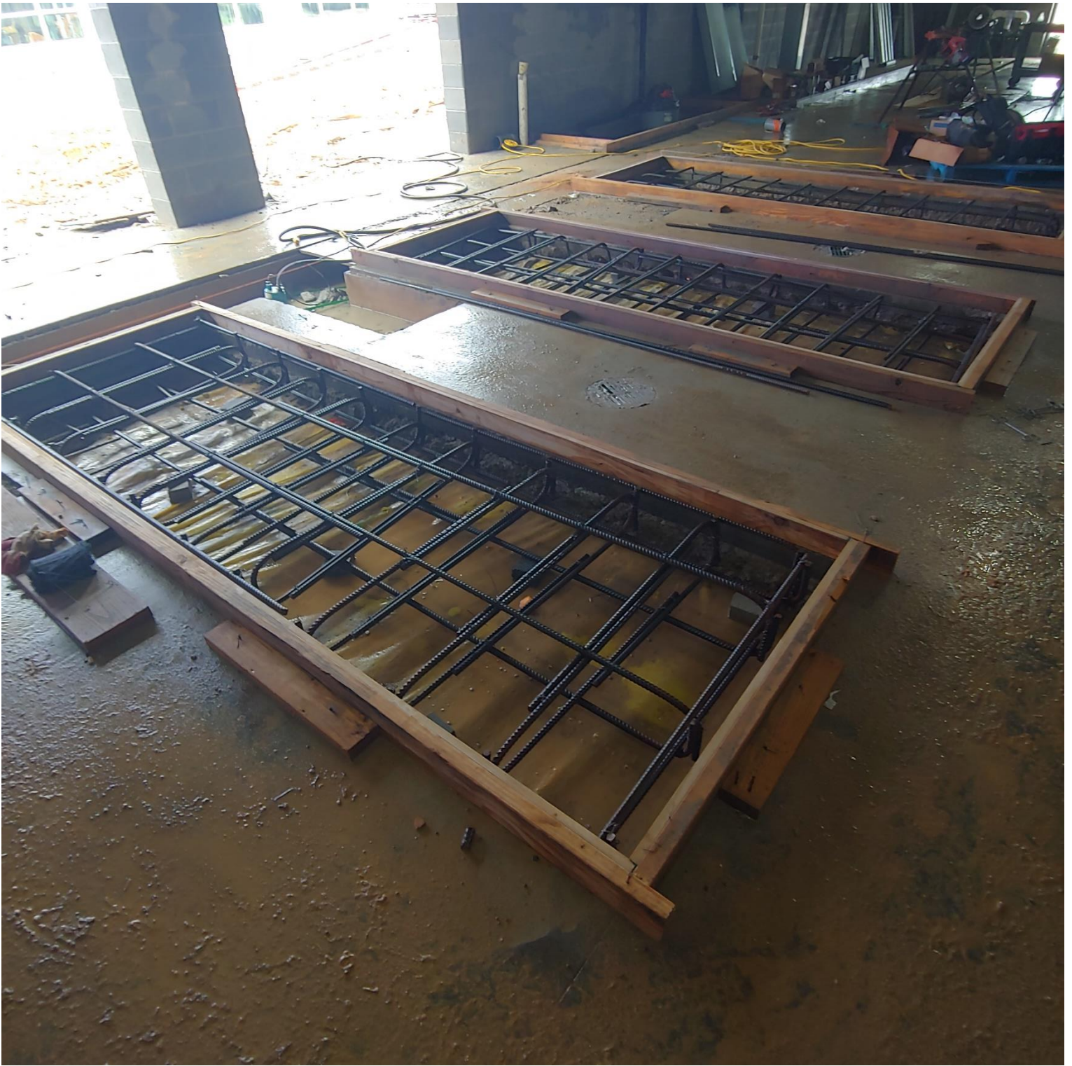
Photo 7 - Steel set in forms for concrete in Mechanical room
