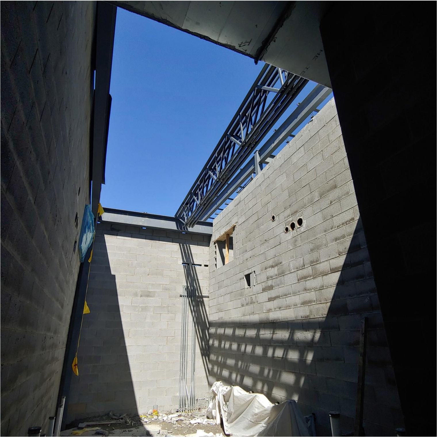
Photo 2 - Trusses staged above room E104
