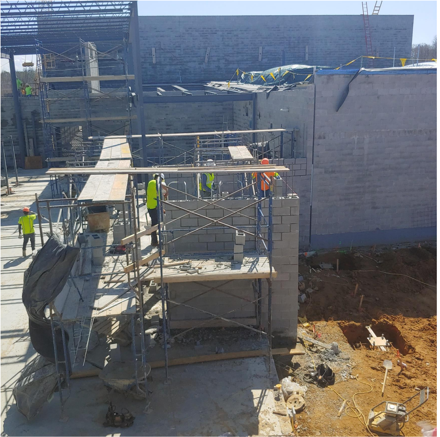
Photo 8 - Block being laid in Vestibule C10
