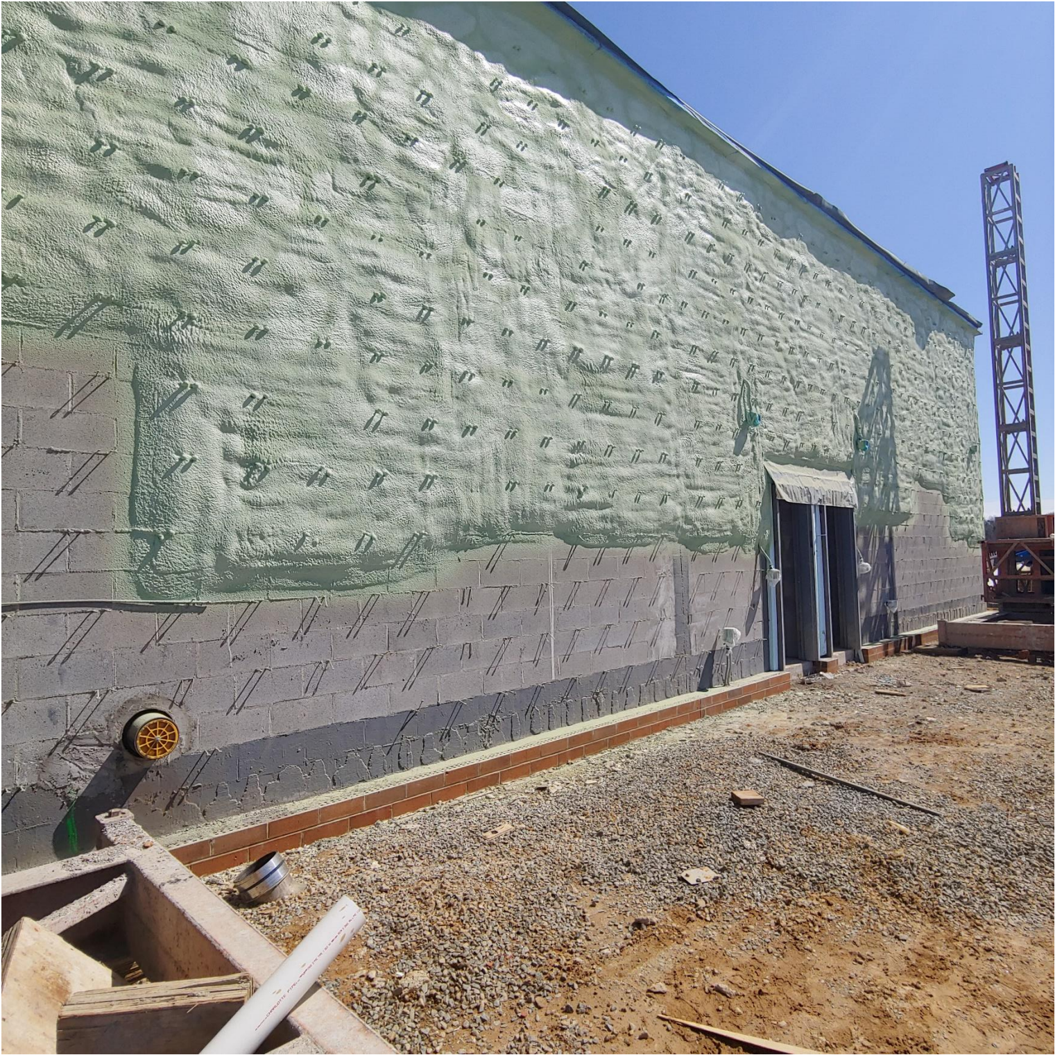
Photo 3 - Exterior wall of Area E receiving spray foam
