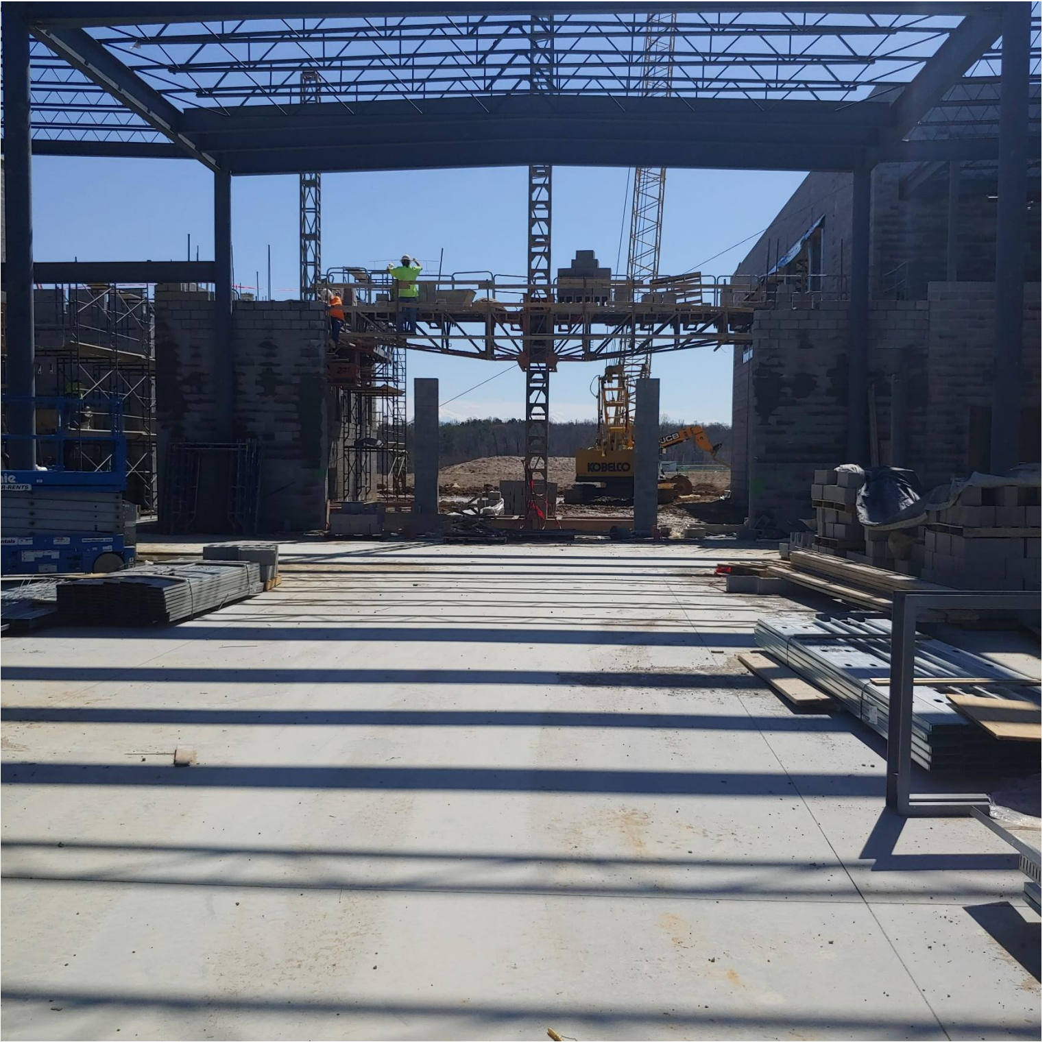
Photo 1 - Block being laid on the South Wall of Area C
