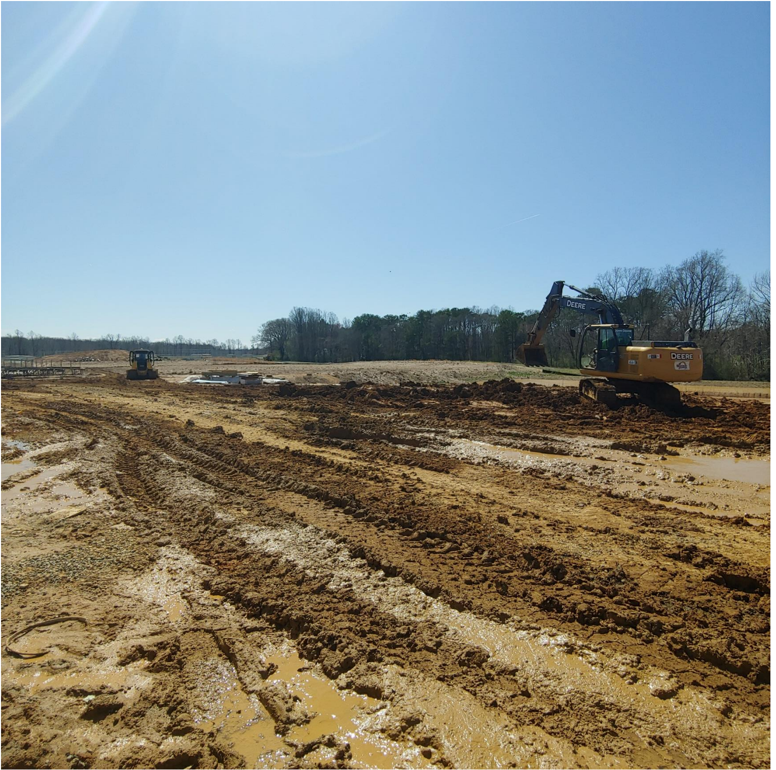
Photo 4 - Dozer and Excavator dressing up the Westside of the site.
