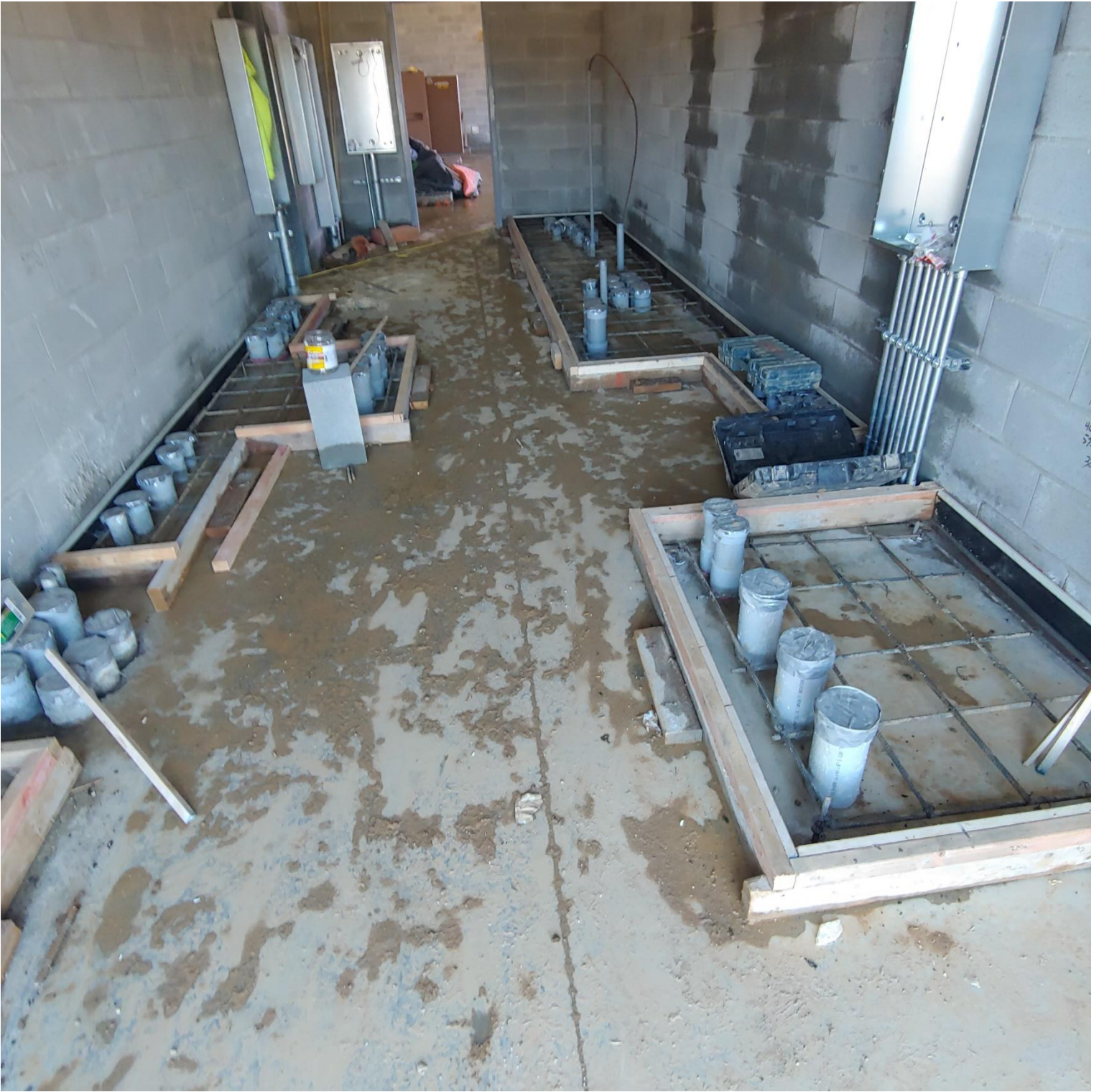
Photo 6 - Concrete Forms completed in Electrical Room D158
