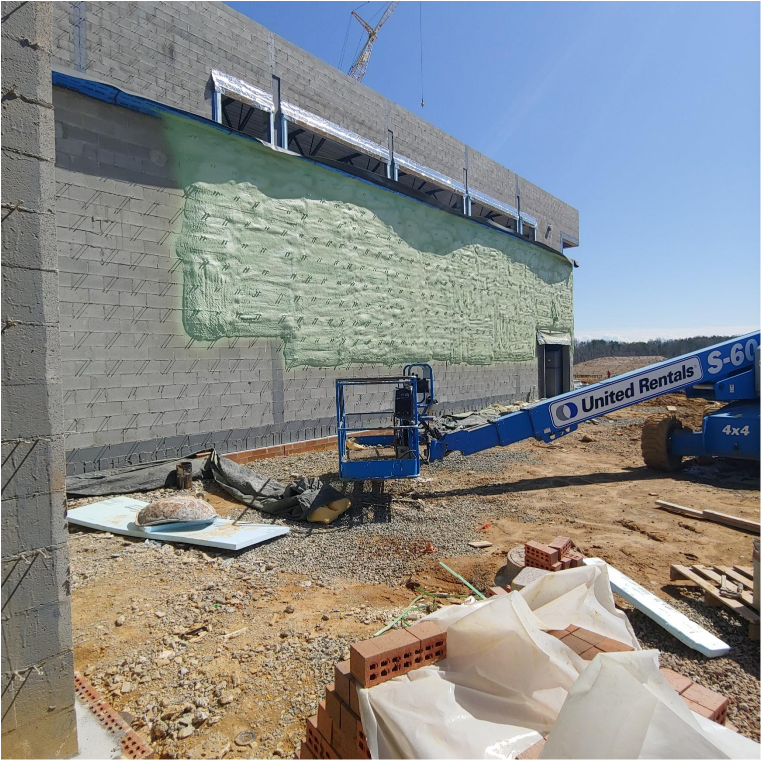
Photo 5 - Westside exterior wall of Gym receiving Spray Foam
