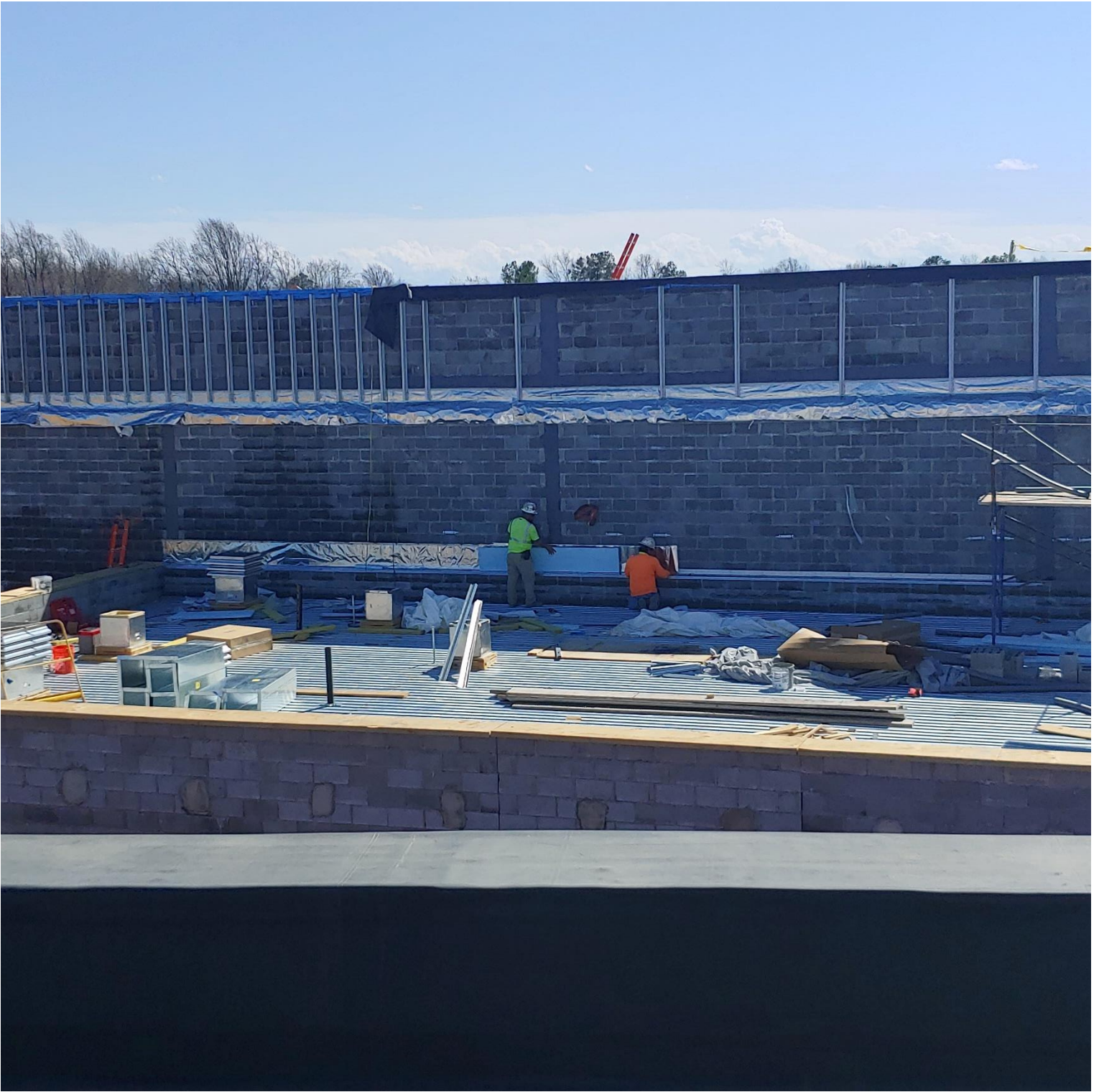
Photo 9 - Flashing being installed along the low roof of Area D
