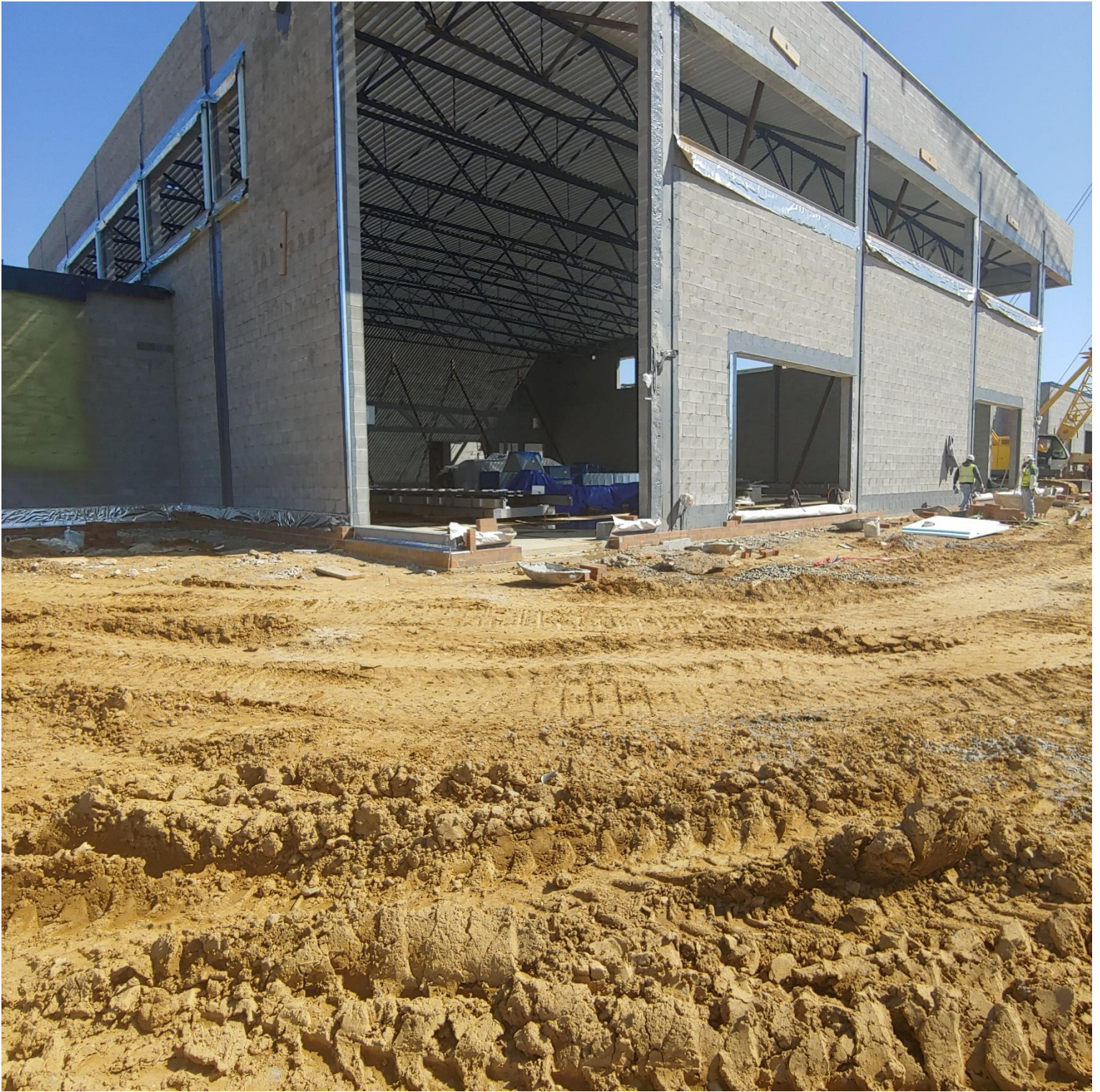
Photo 8 - Brick being laid on the Southside of Area E
