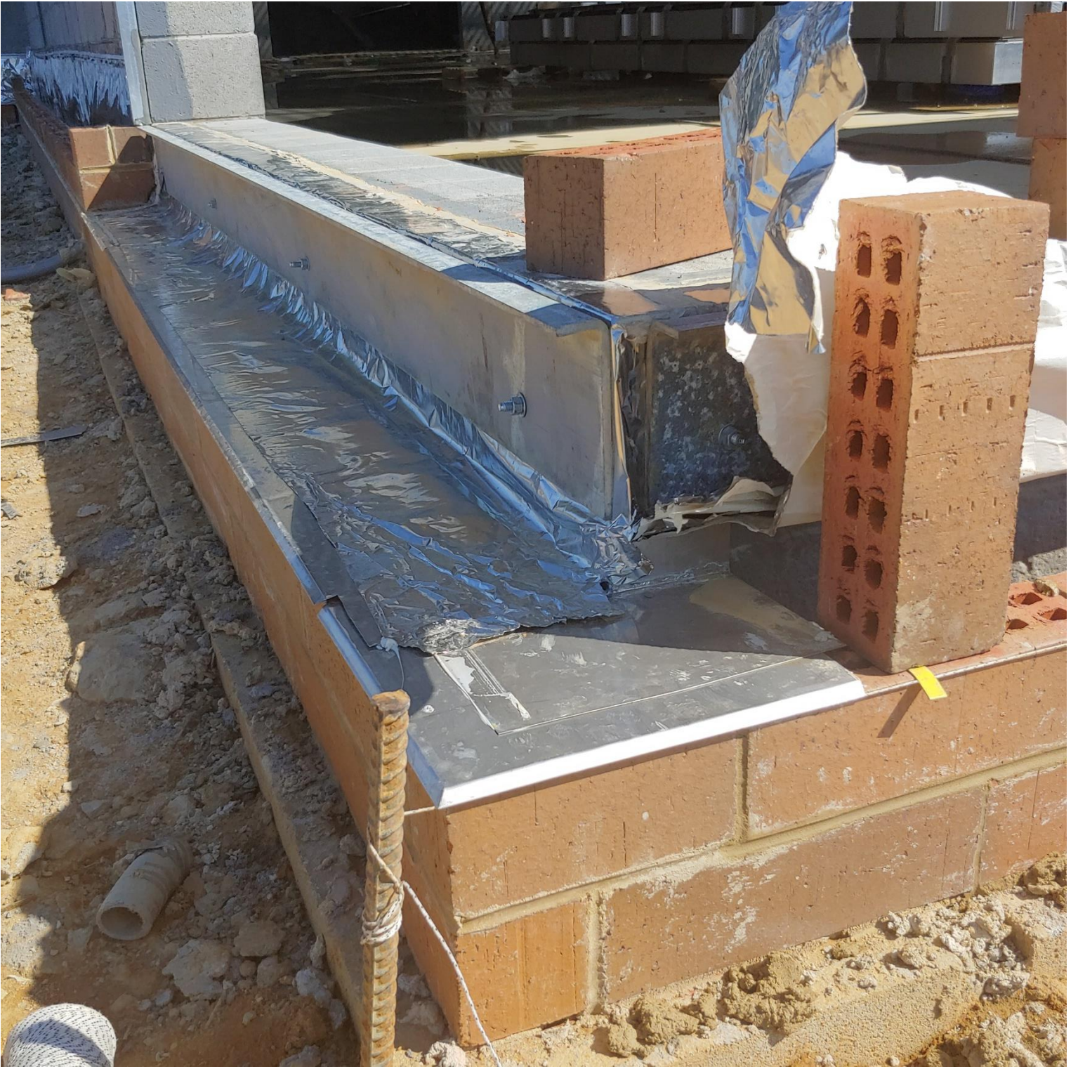
Photo 9 - Flashing installed on the Southwest Corner of Area E
