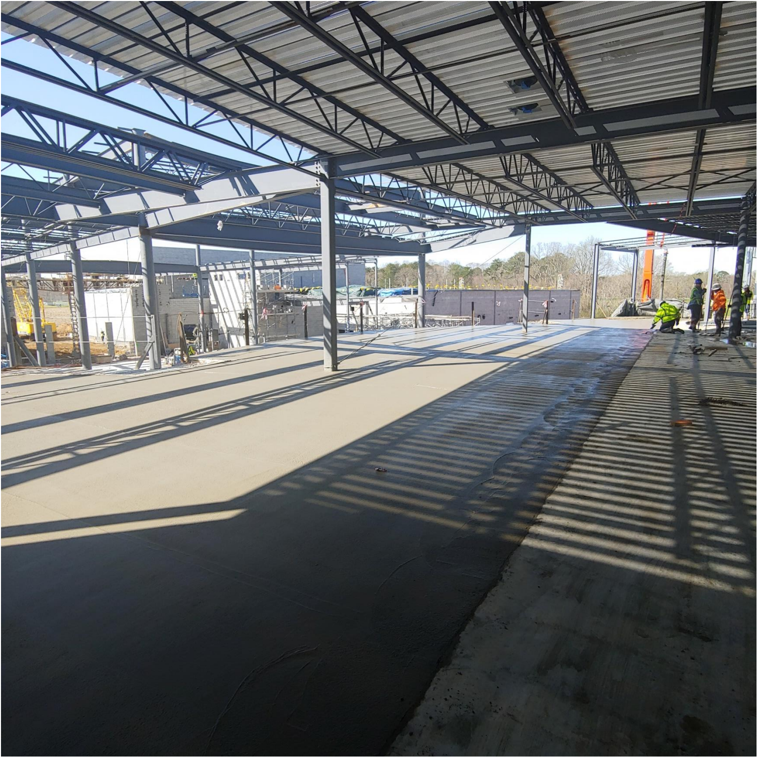
Photo 2 - Concrete slab poured on the 2nd floor of Area A
