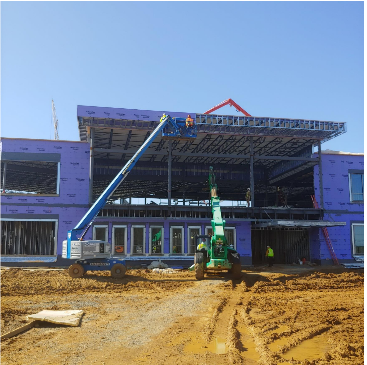
Photo 1 - Gyp Board Being Installed on the Northside of Area A
