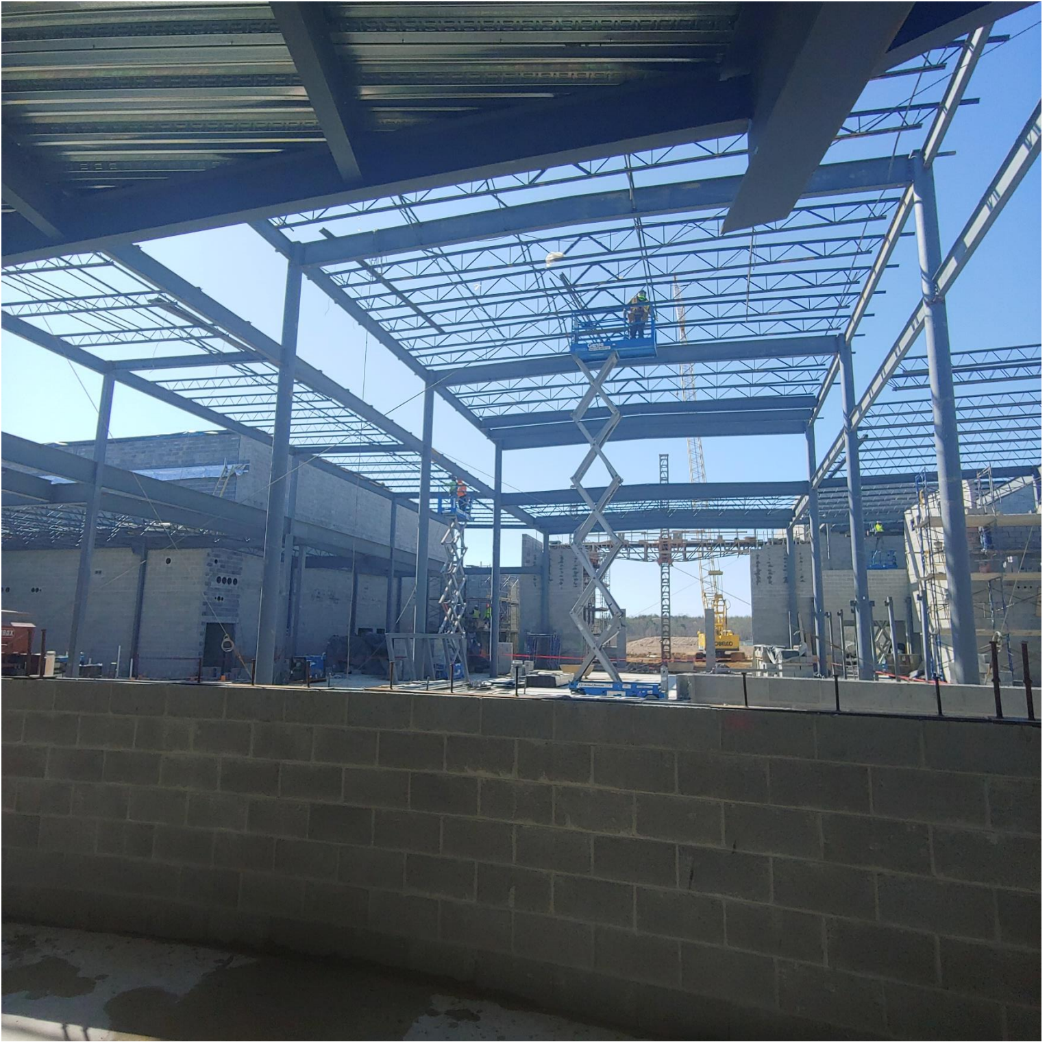
Photo 3 - Steel being welded in Area C
