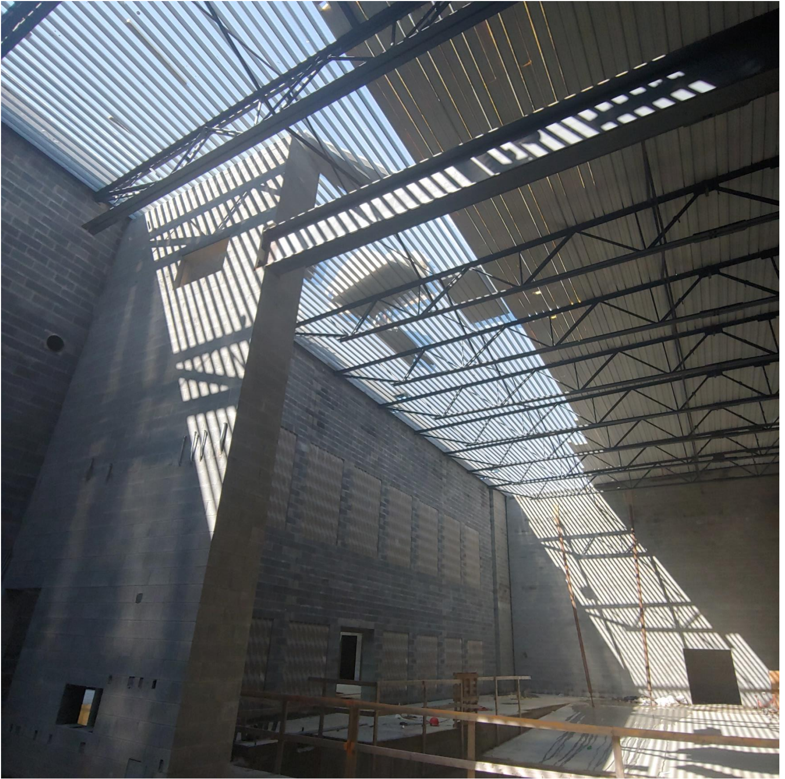
Photo 5 – Foam Board being installed above Auditorium
