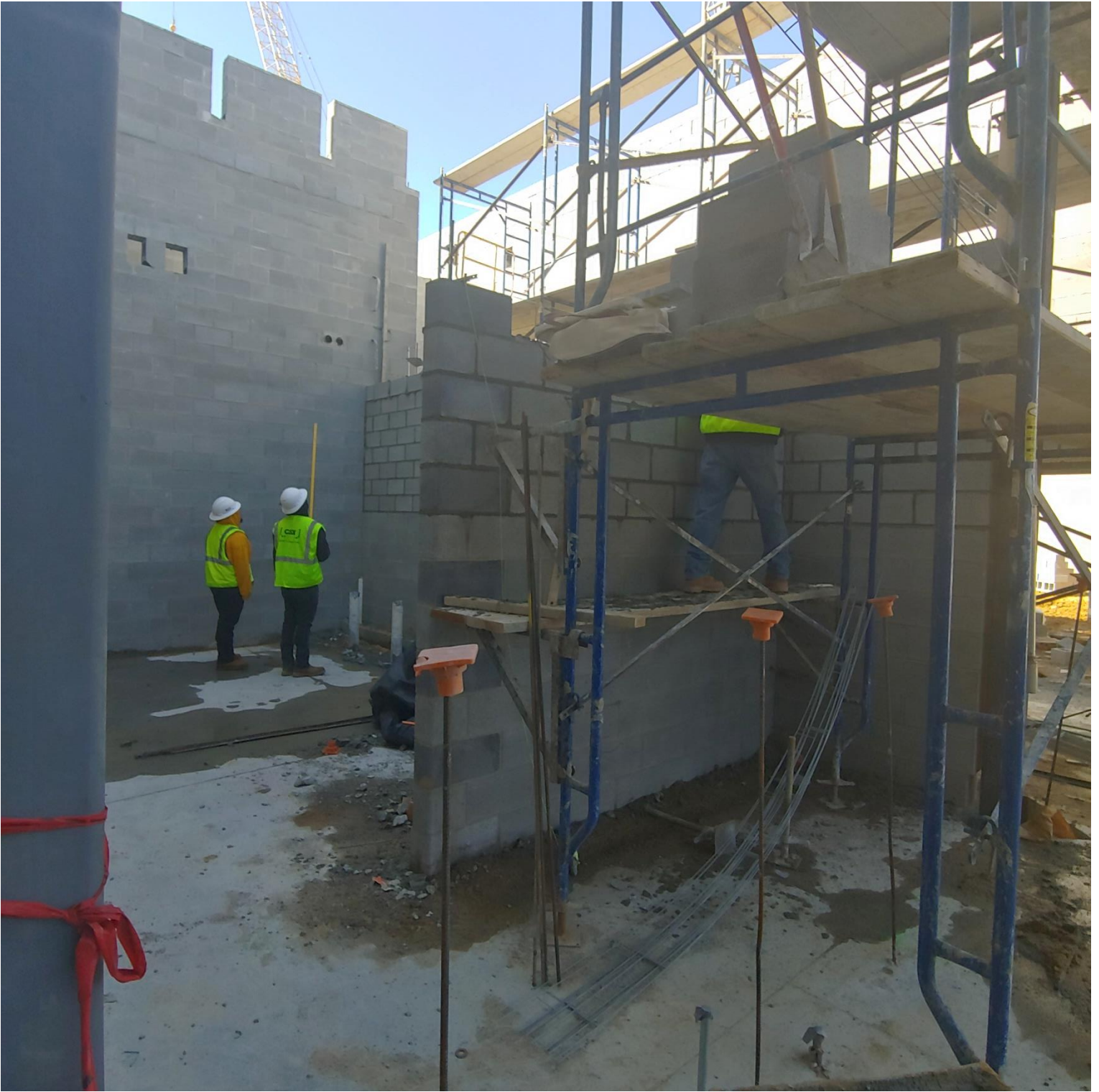
Photo 6 - Block being laid in D103
