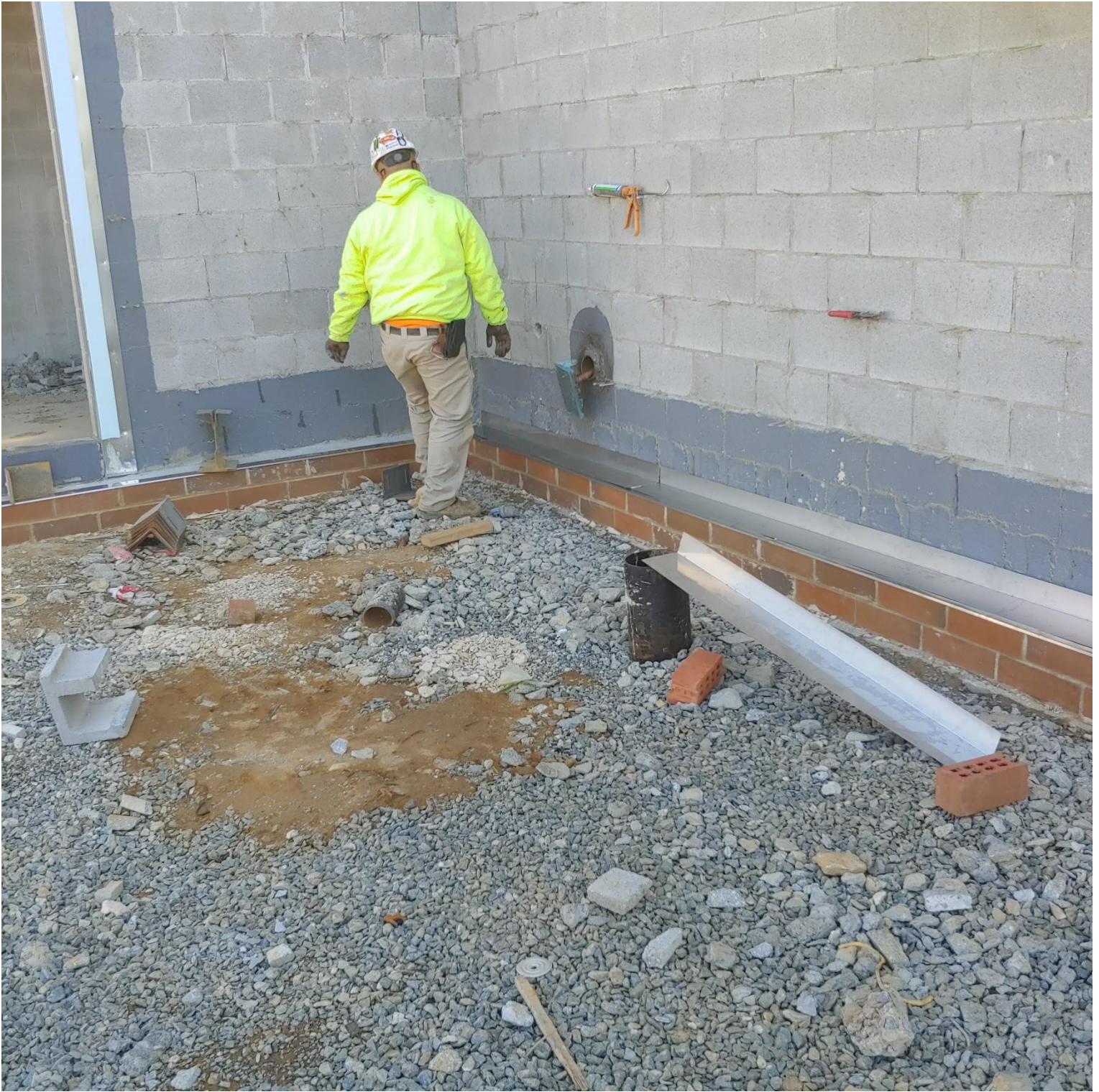
Photo 10 - flashing being installed on the Southwest corner of Vestibule E10
