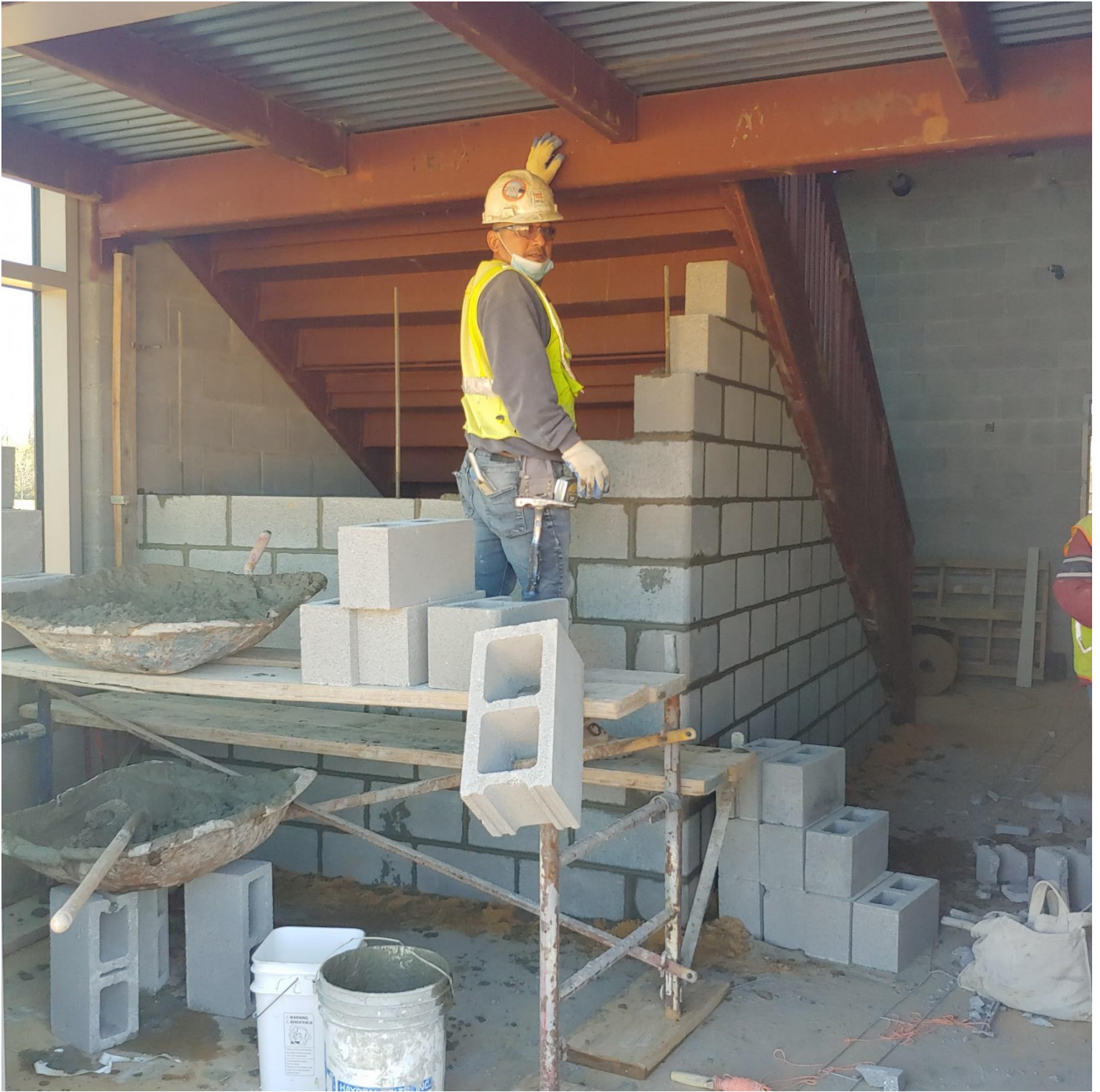
Photo 6 - Block being laid under the Stairs in Stairwell #1
