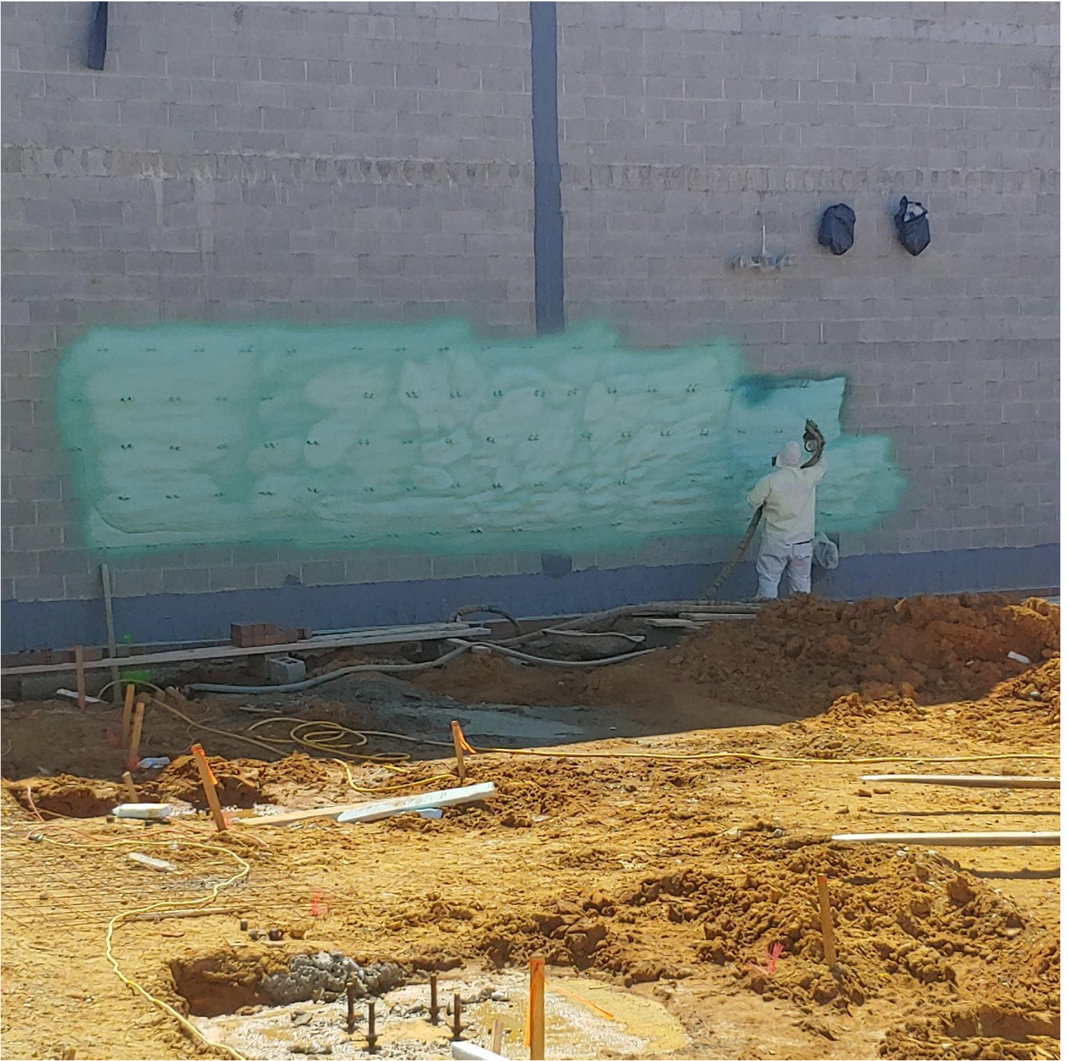
Photo 2 - Foam being applied to the North wall of Area E.
