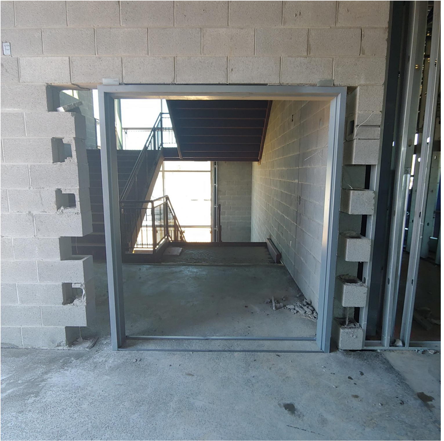
Photo 8 - Door frame has been set on the 2nd floor of Stairwell #2
