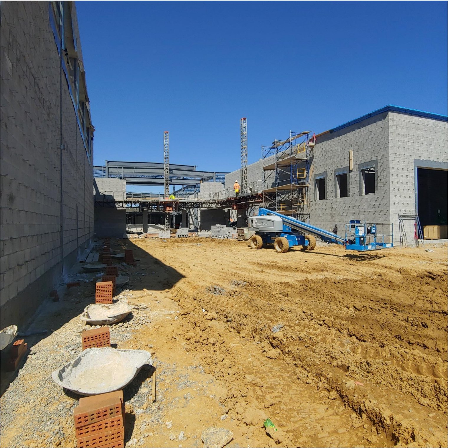
Photo 4 – Masons laying block on the Westside of Area D.
