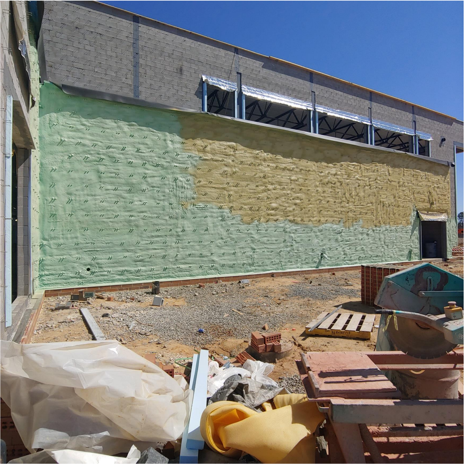
Photo 3 – A section on the Westside of Gym, Area E has been Spray Foamed.
