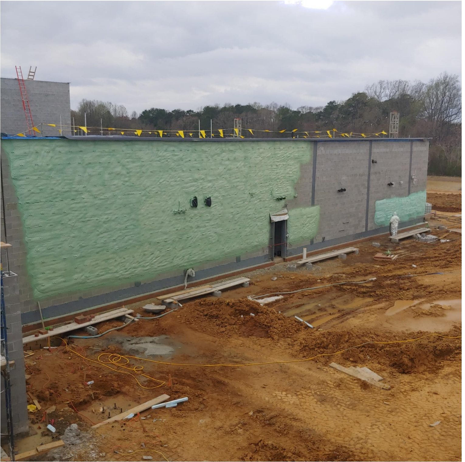
Photo 1 Spray Foam being applied to the Northside of Area E
