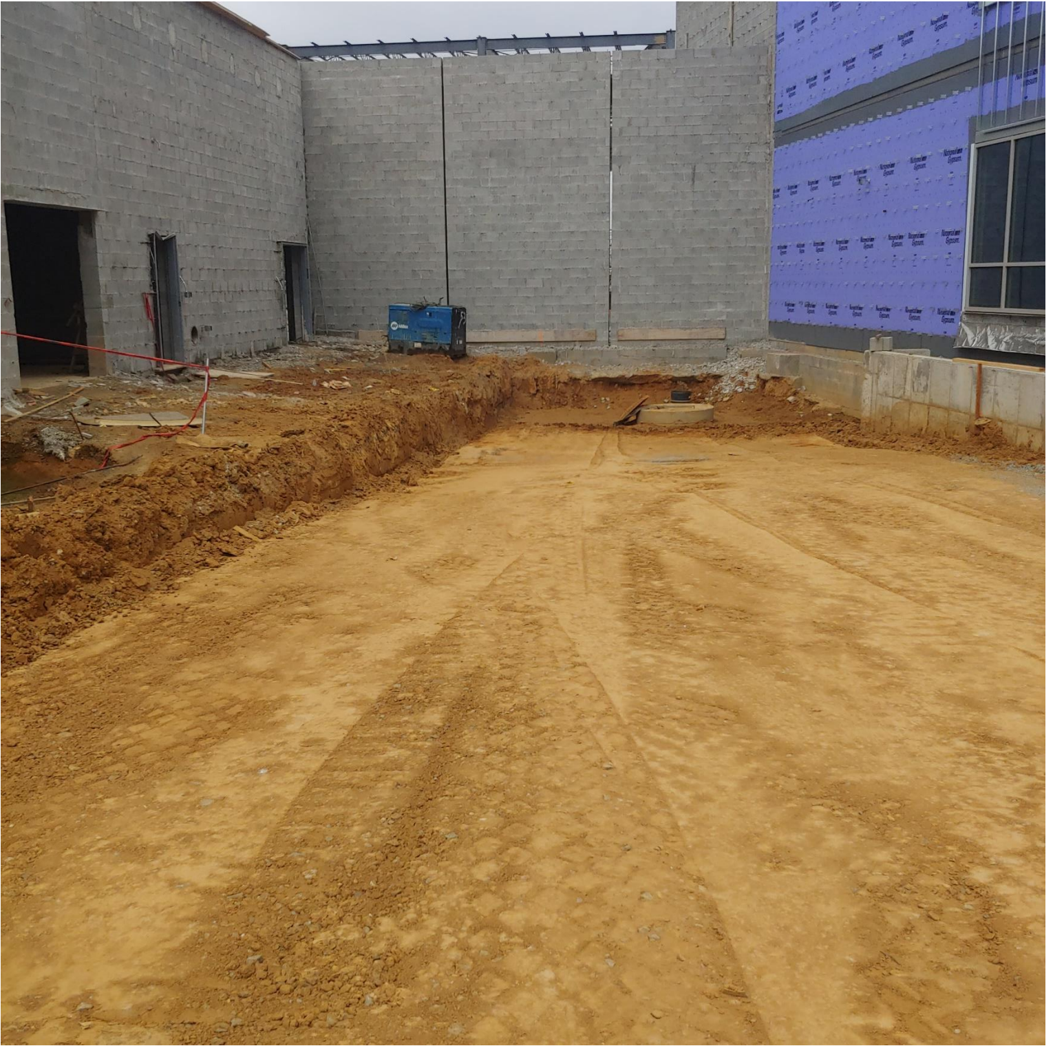
Photo 6 - Loading Dock Ramp has been rough graded
