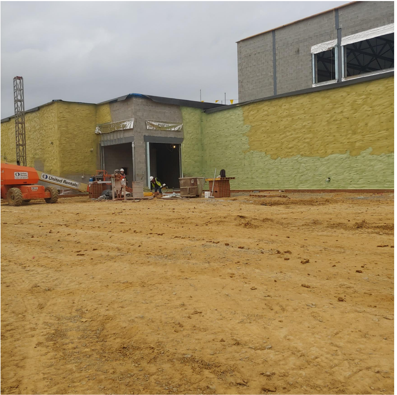
Photo 3 - Metal studs being installed above Door
