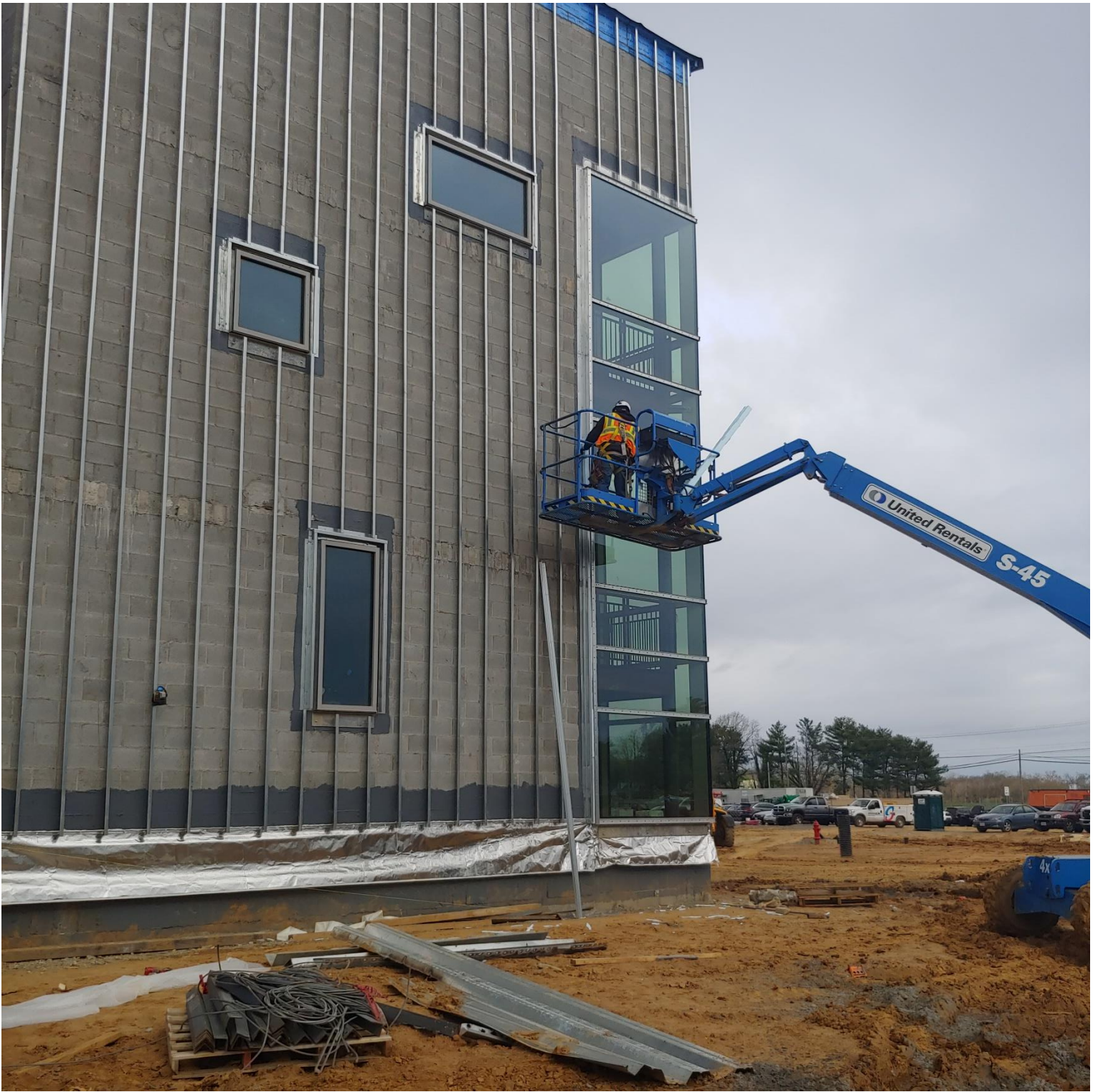
Photo 7 - Foam Board being installed around Storefront
