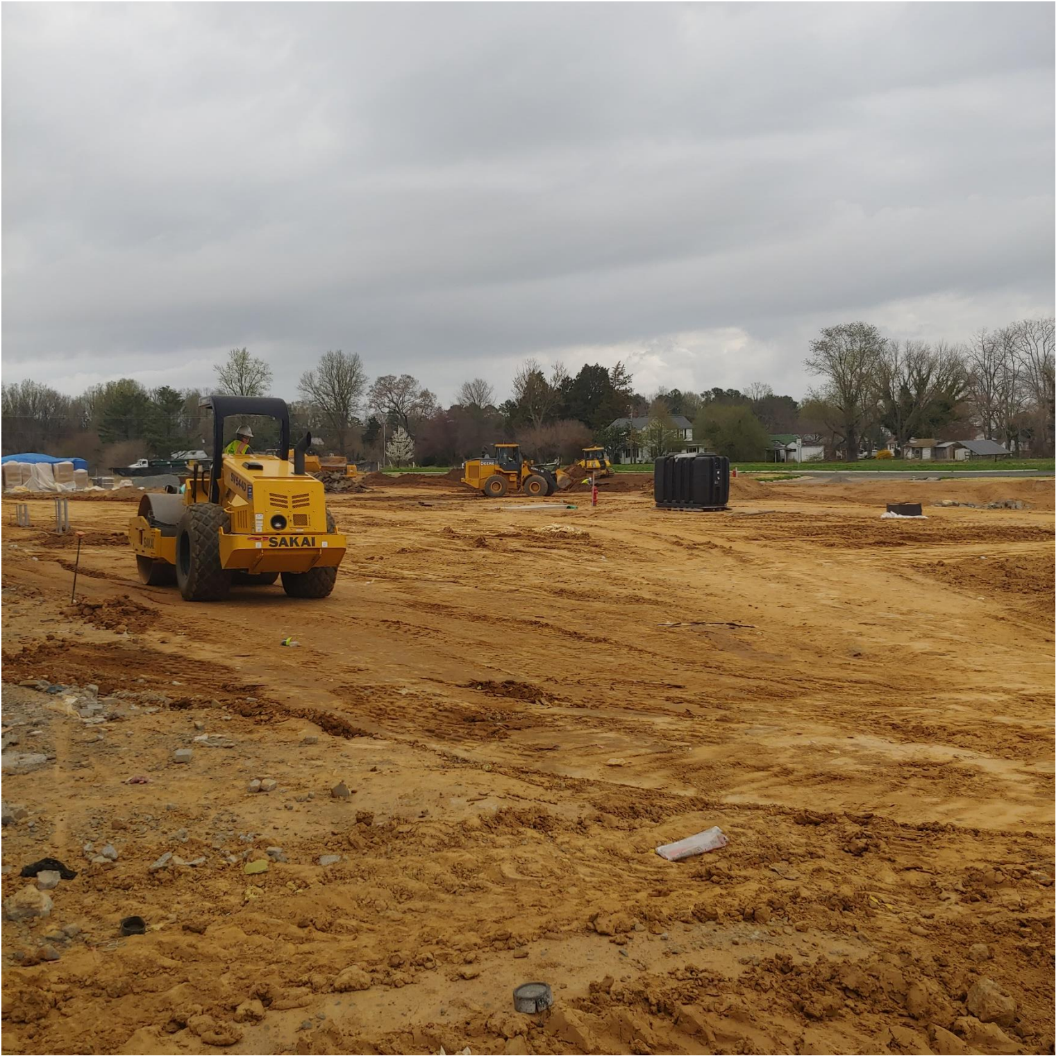
Photo 5 - Beuchert has begun to grade the Eastside of site.
