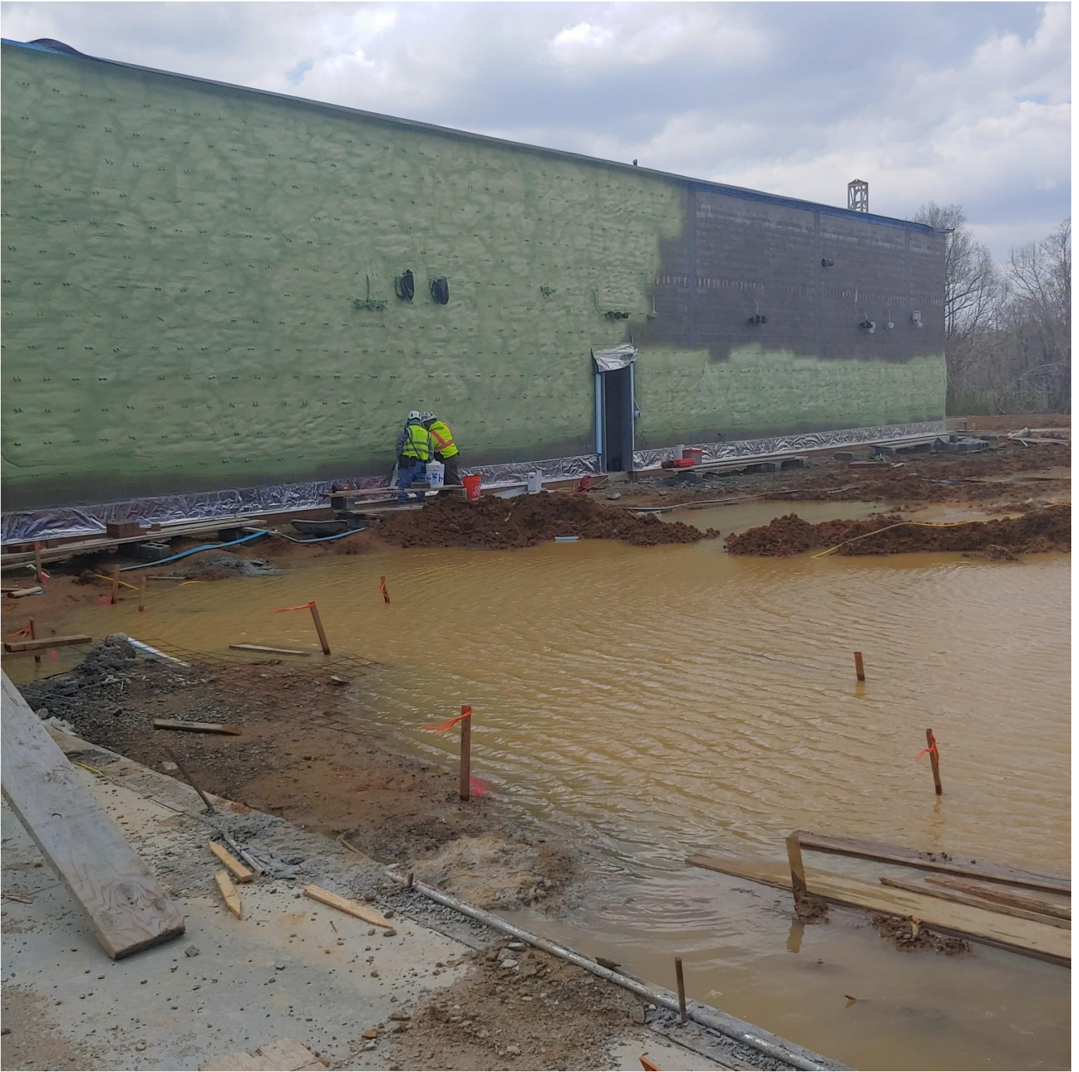
Photo 2 - Brick Flashing being installed on the Northside of Area E
