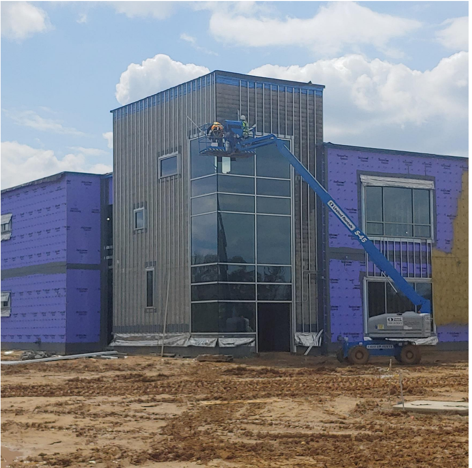
Photo 1 - Metal framing being installed on block of Stairwell #1
