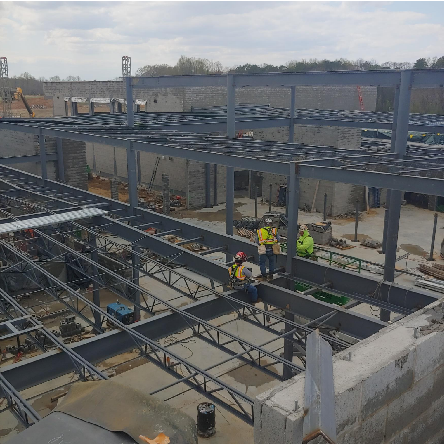
Photo 6 – Weldon Steel welding Steel in Area C
