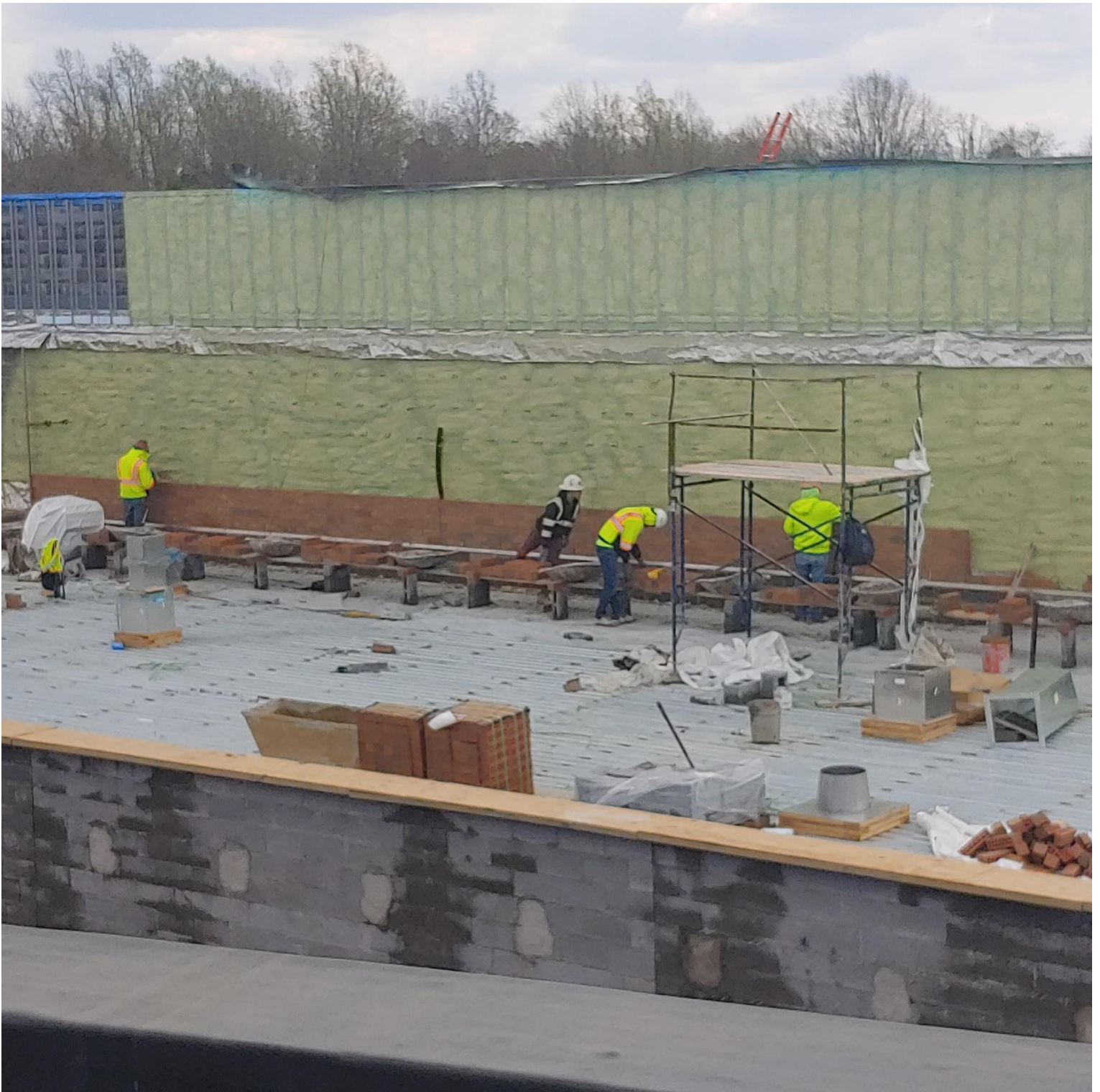
Photo 5 - Masons laying Brick on the Northside of Area D
