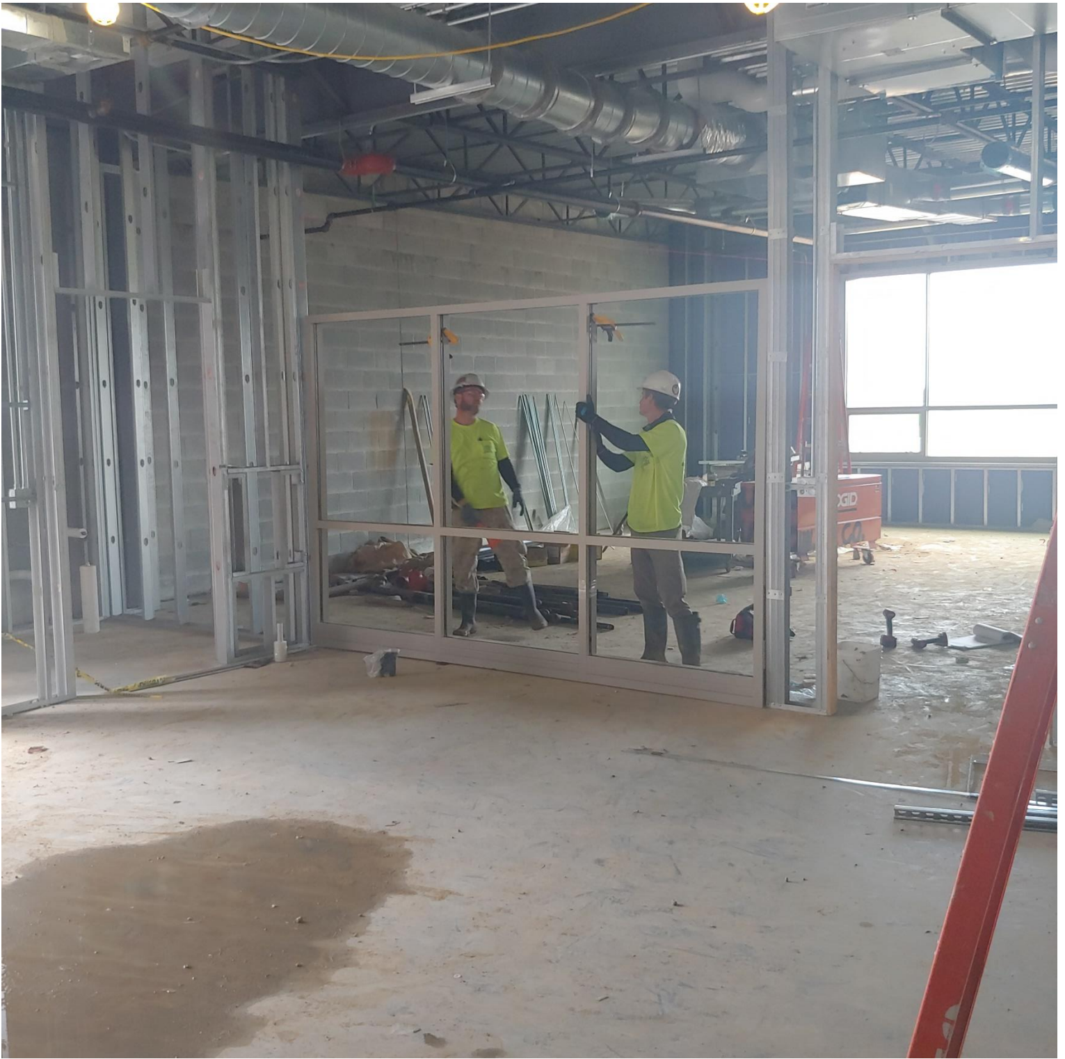
Photo 4 - Storefront being set on the 2nd Floor of Area A
