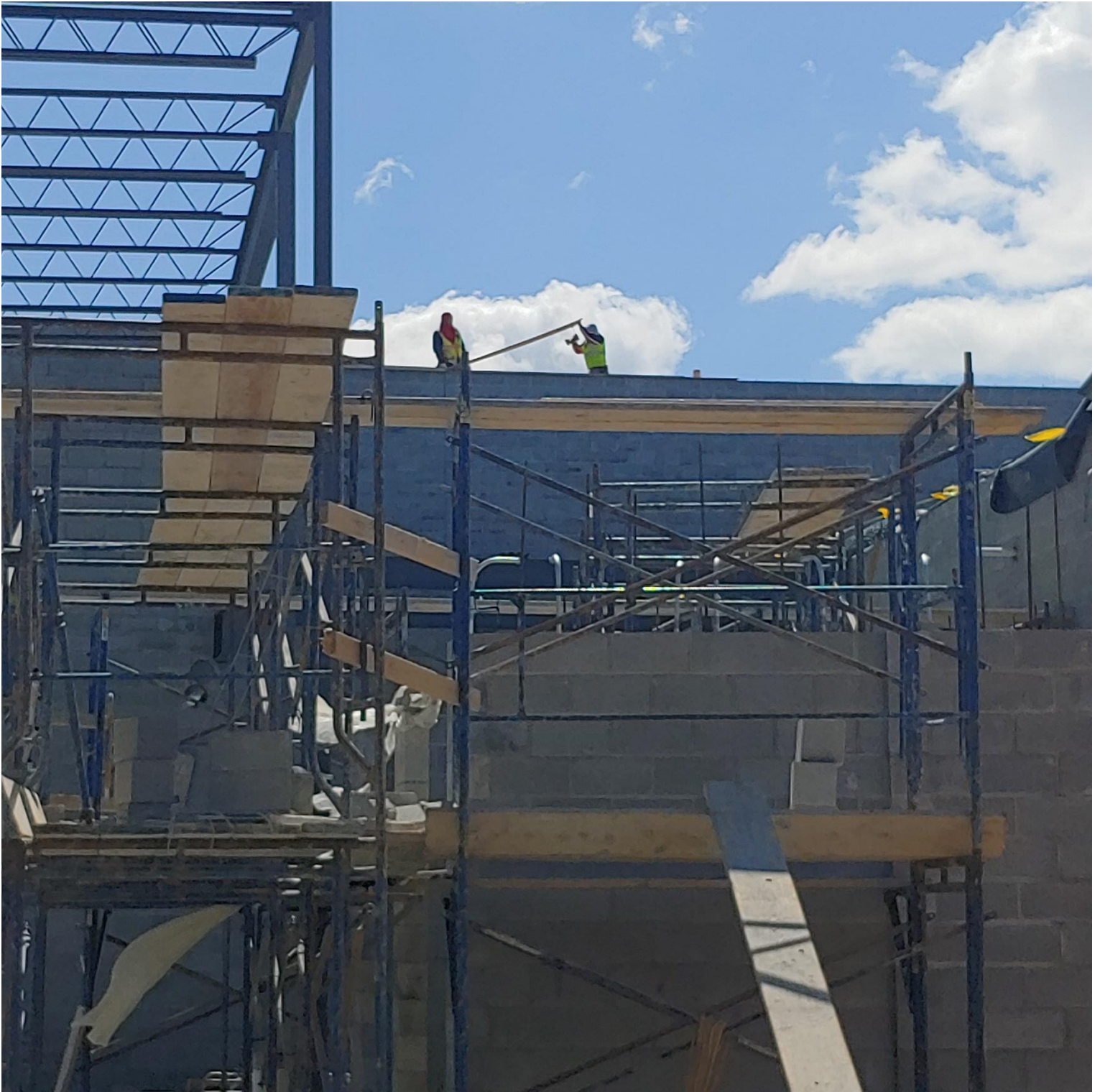
Photo 1 - Parapet wall being constructed on the high roof of Area E
