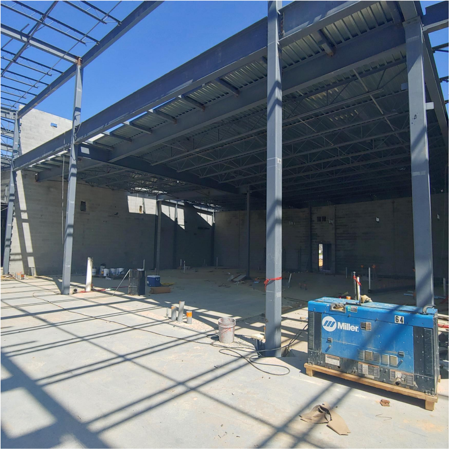
Photo 6 - Metal decking has been laid above the Kitchen in Area C
