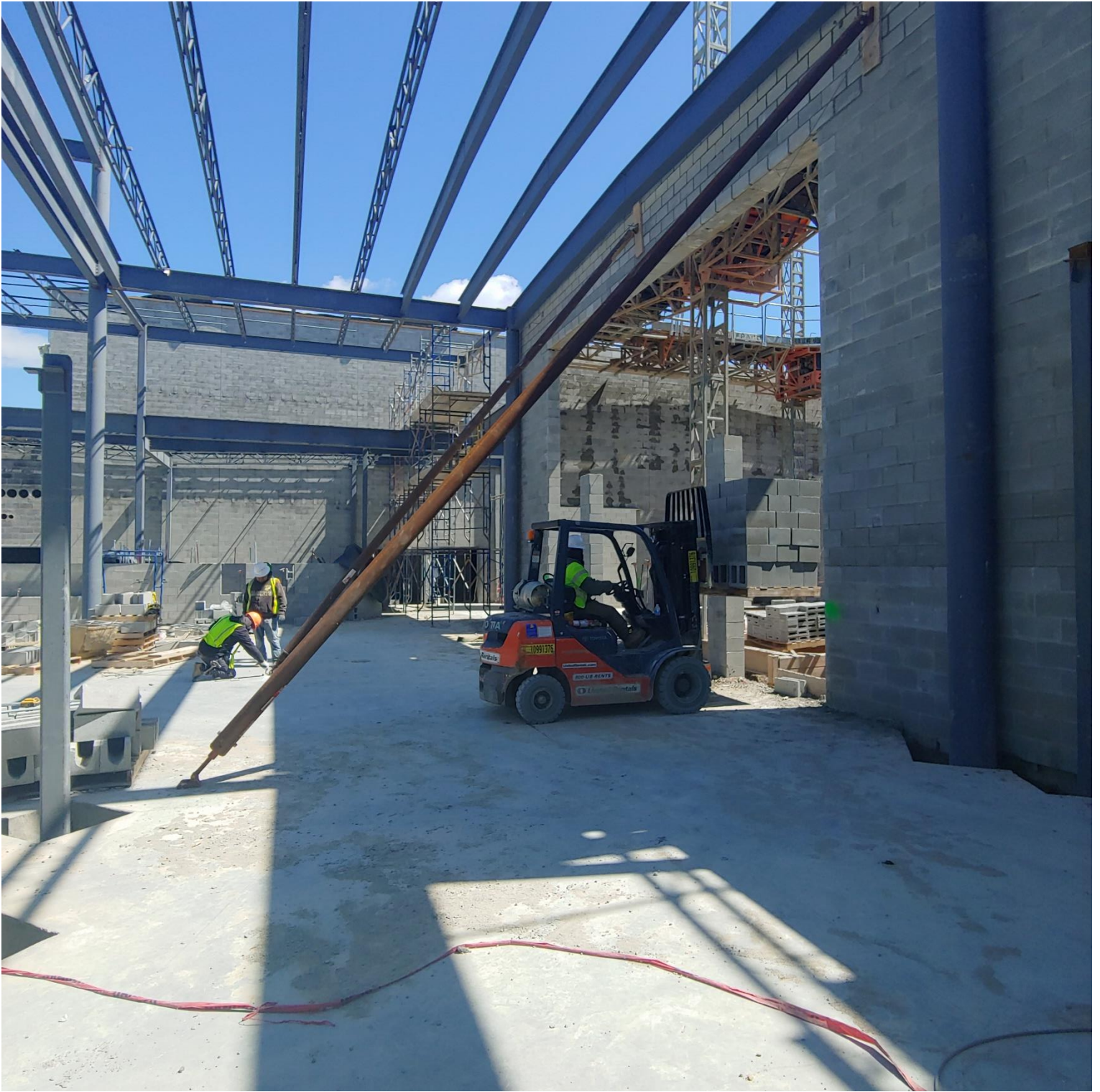
Photo 3 - South wall of Area C being braced
