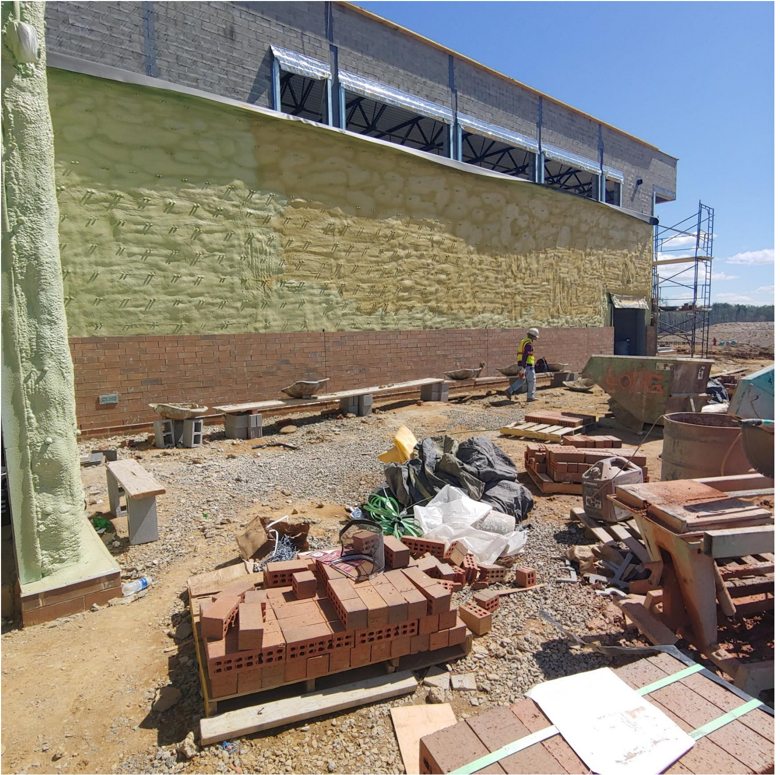
Photo 4 - Brick being laid on the West wall of the Gym
