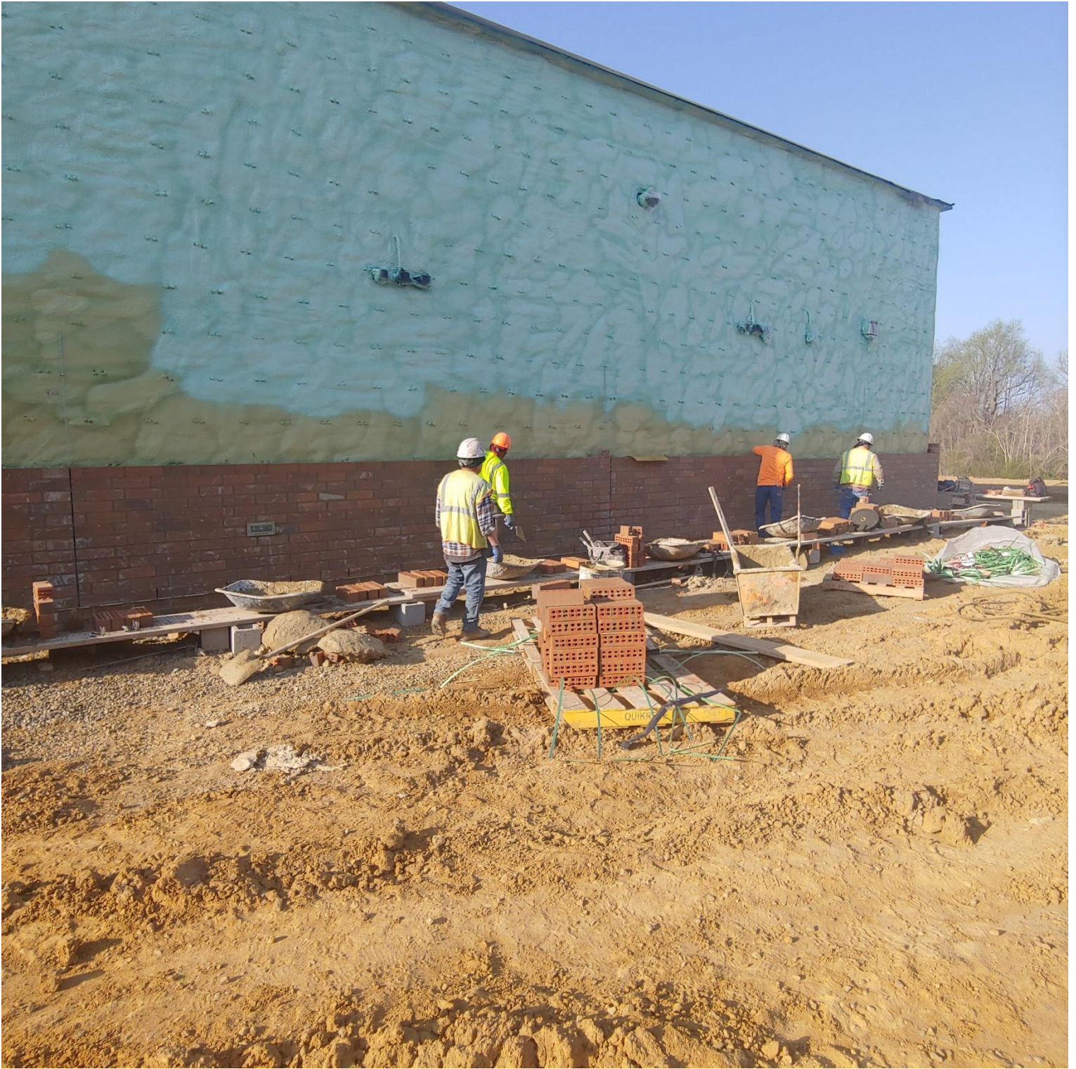
Photo 3 - Brick is being laid on the Northside of Area E
