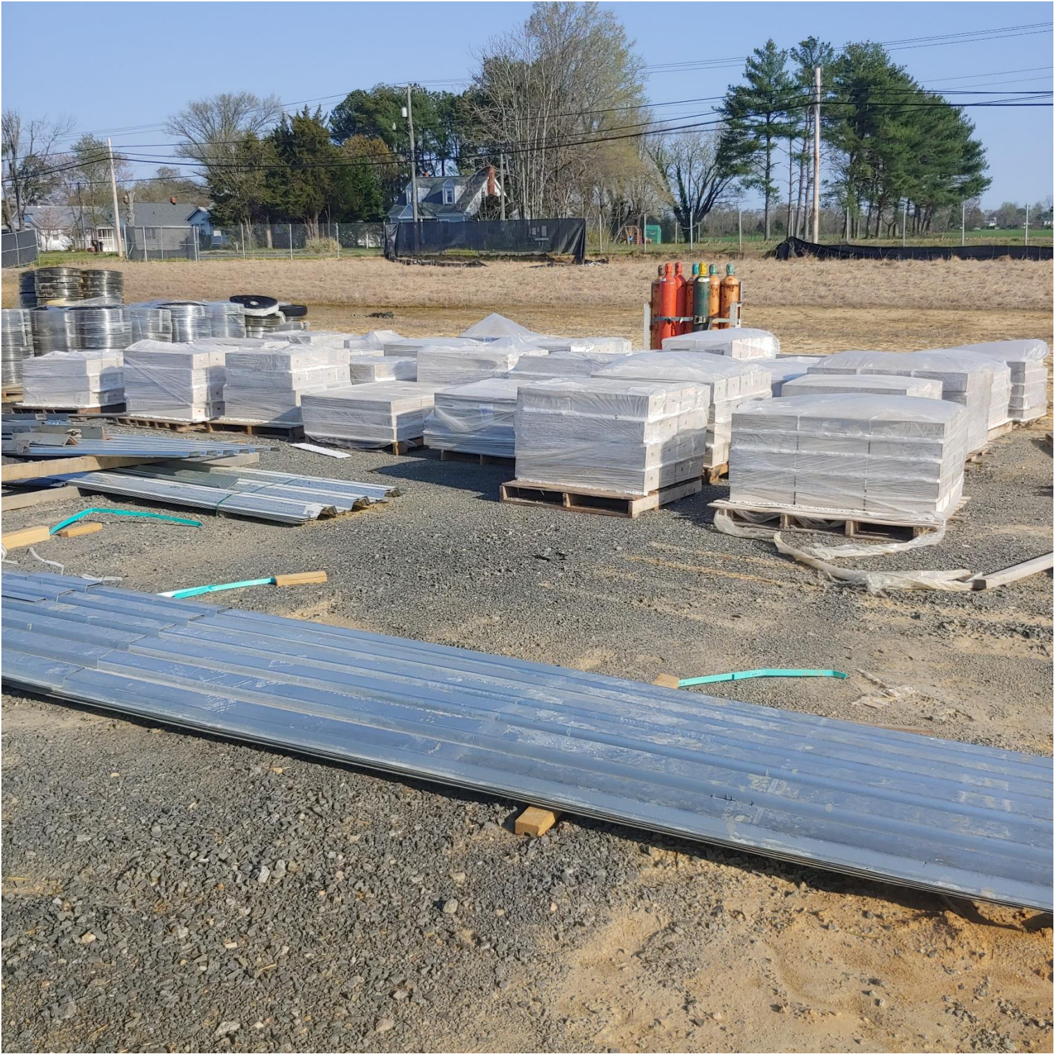
Photo 7 - Pre-cast Package staged on site.
