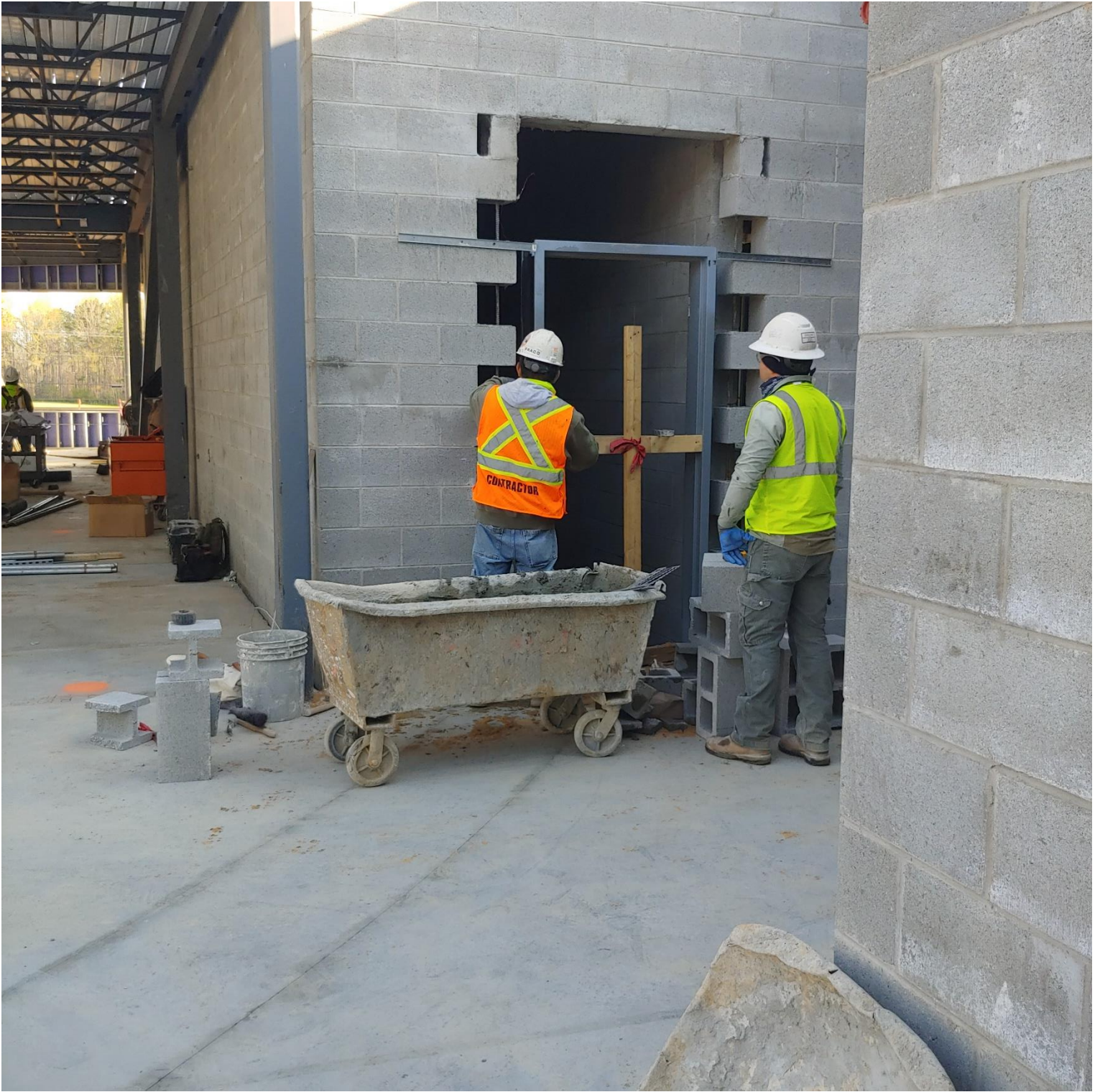
Photo 4 - Block being laid around the door frame of Stair #4, 2nd floor.
