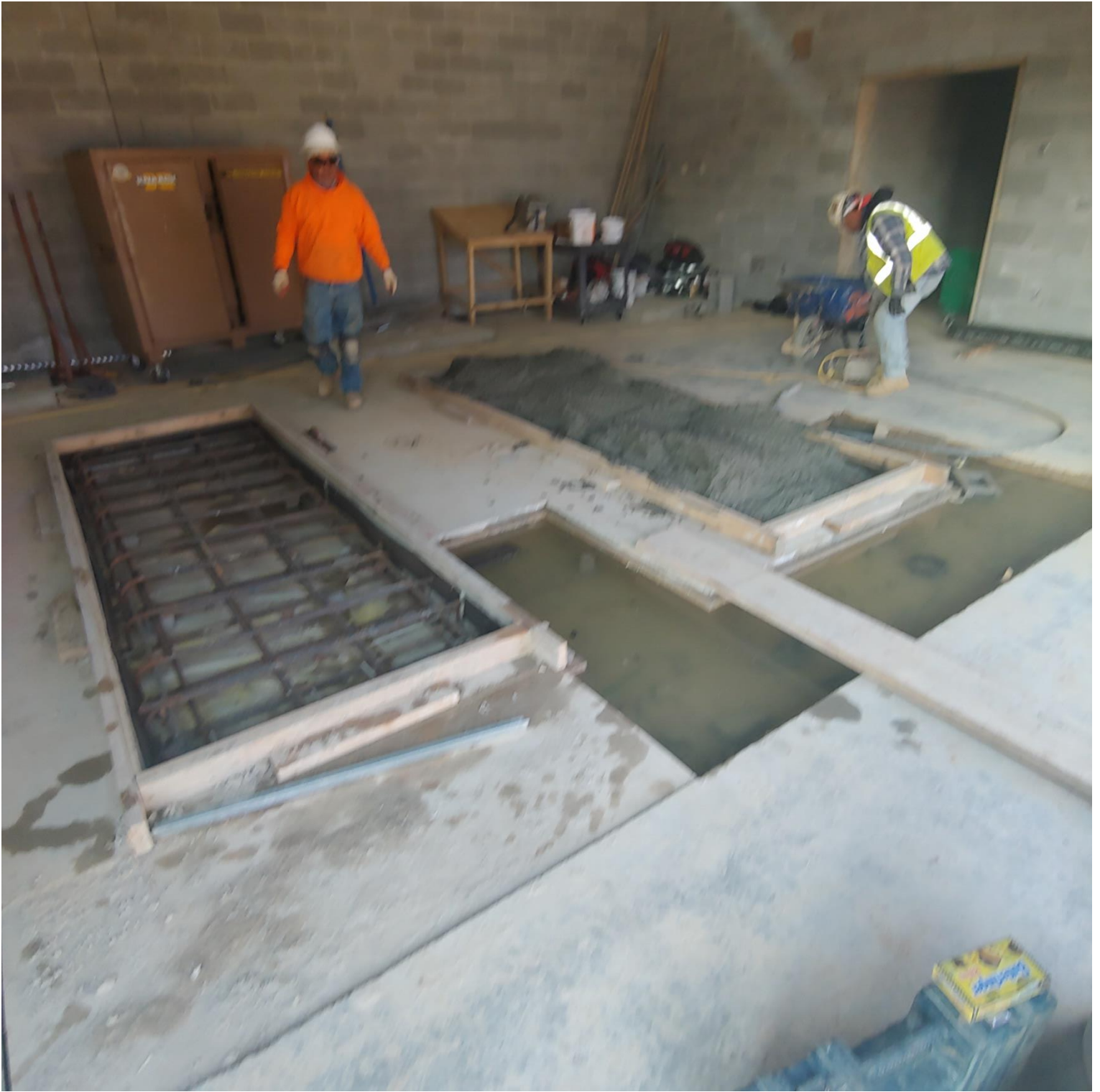
Photo 1 - Raised Mechanical Equipment Slabs are being poured in Area D
