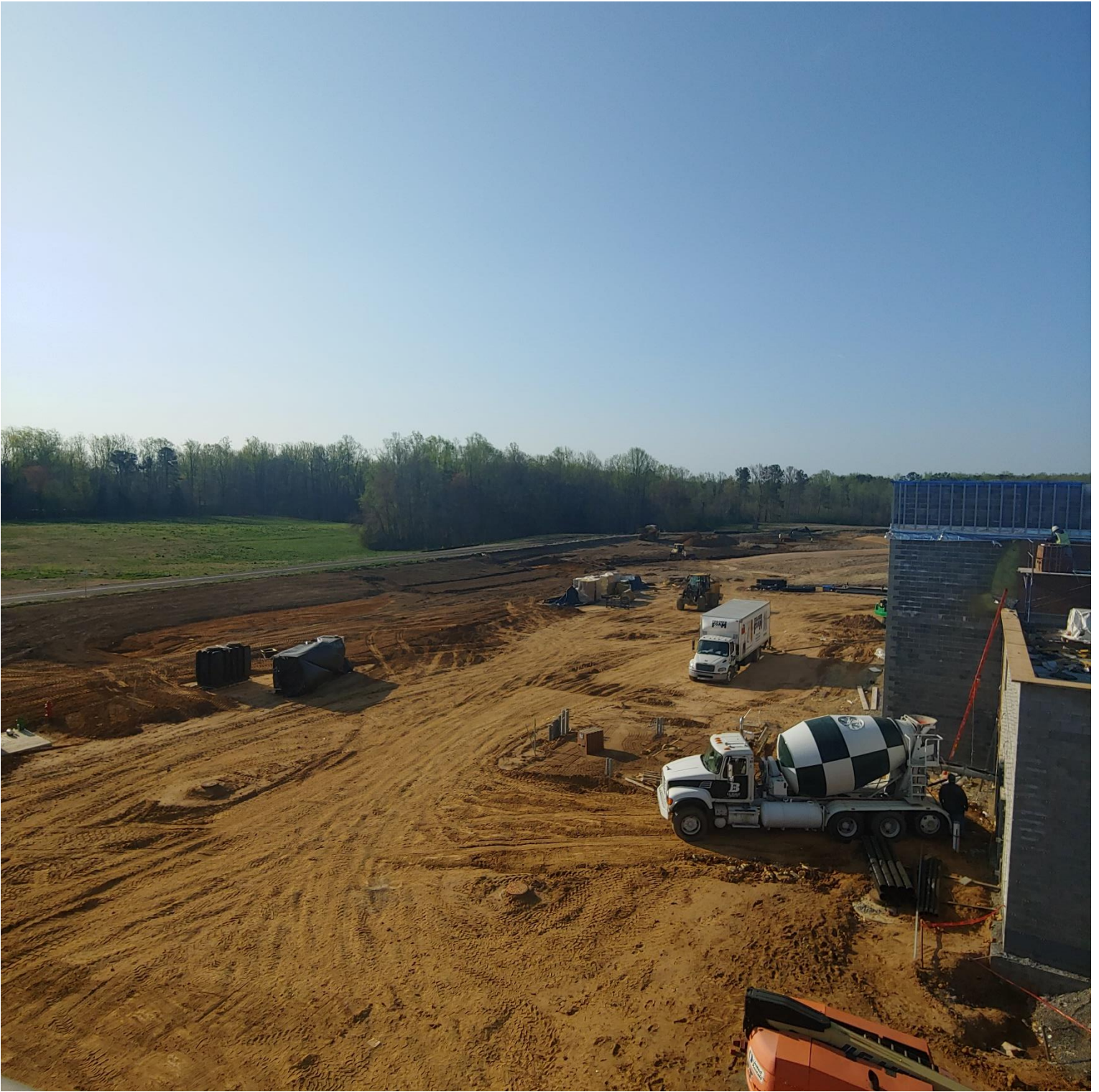
Photo 6 - Beuchert continues to grade and shape the Eastside of the site.
