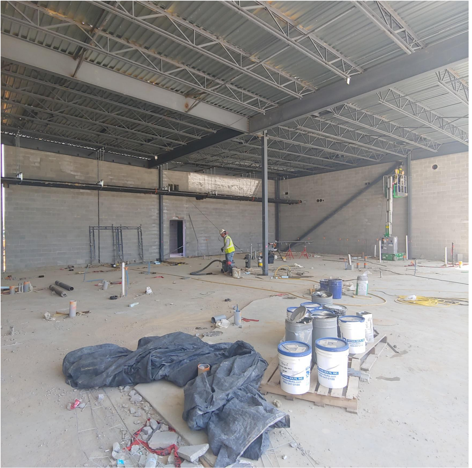
Photo 6 - Steel being welded in the Kitchen Area
