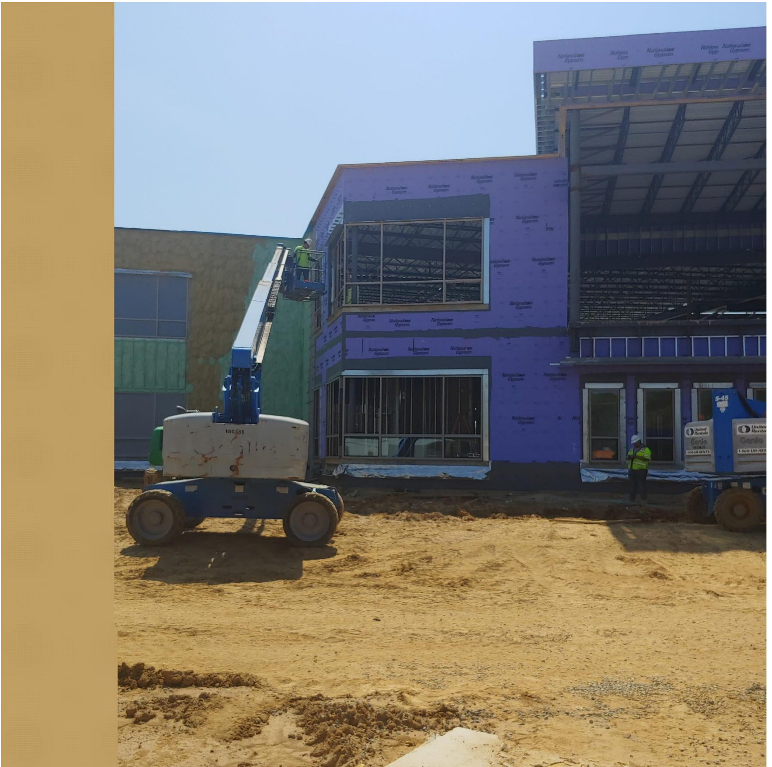
Photo 1 Storefronts being set on the 2nd floor of Area A
