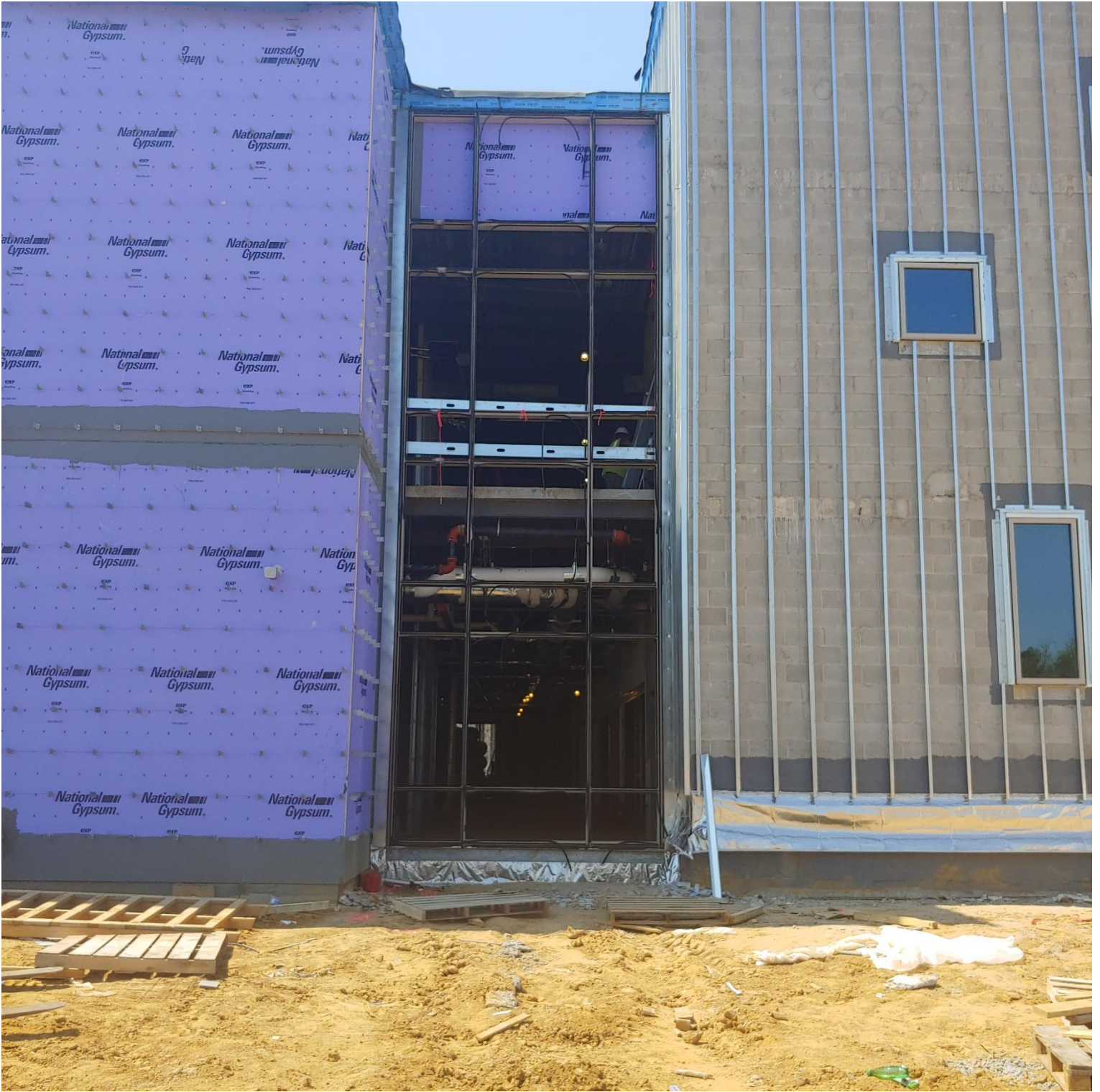
Photo 3 - Large Storefront on the Eastside of Area A has been set
