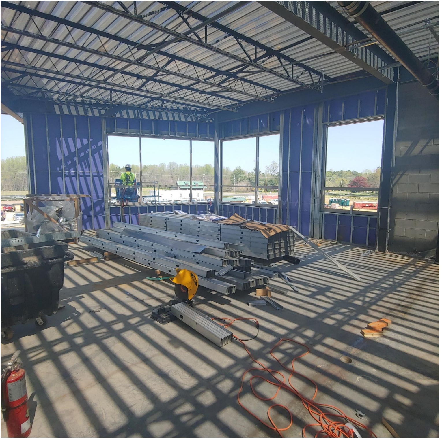
Photo 8 - Storefronts being set on the 2nd floor of Area A
