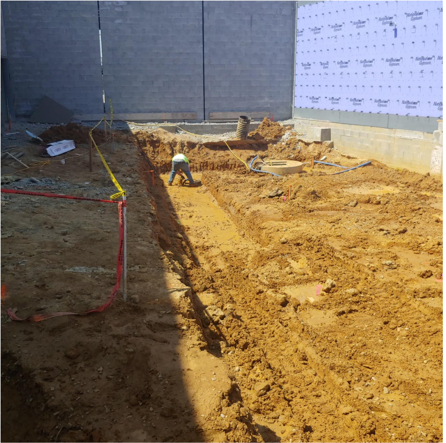
Photo 4 - Work continues on the Loading Ramp
