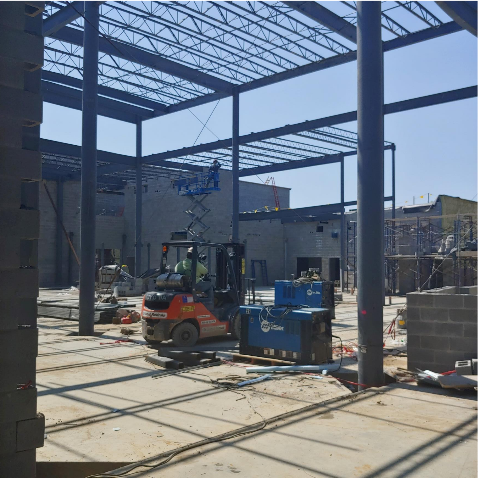
Photo 5 - Trusses set and being welded in Area C
