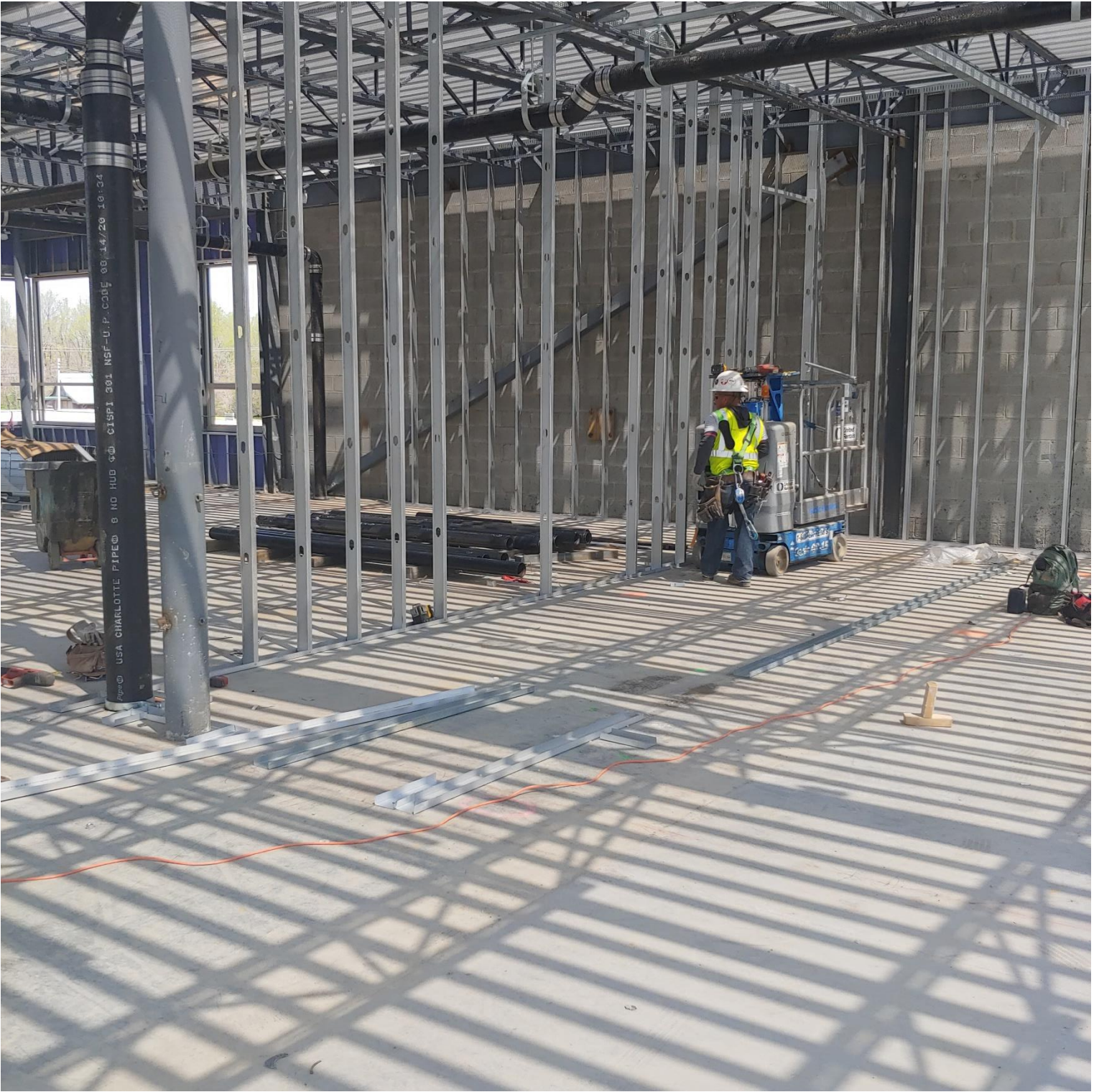
Photo 7 - Interior walls are being framed in Area A
