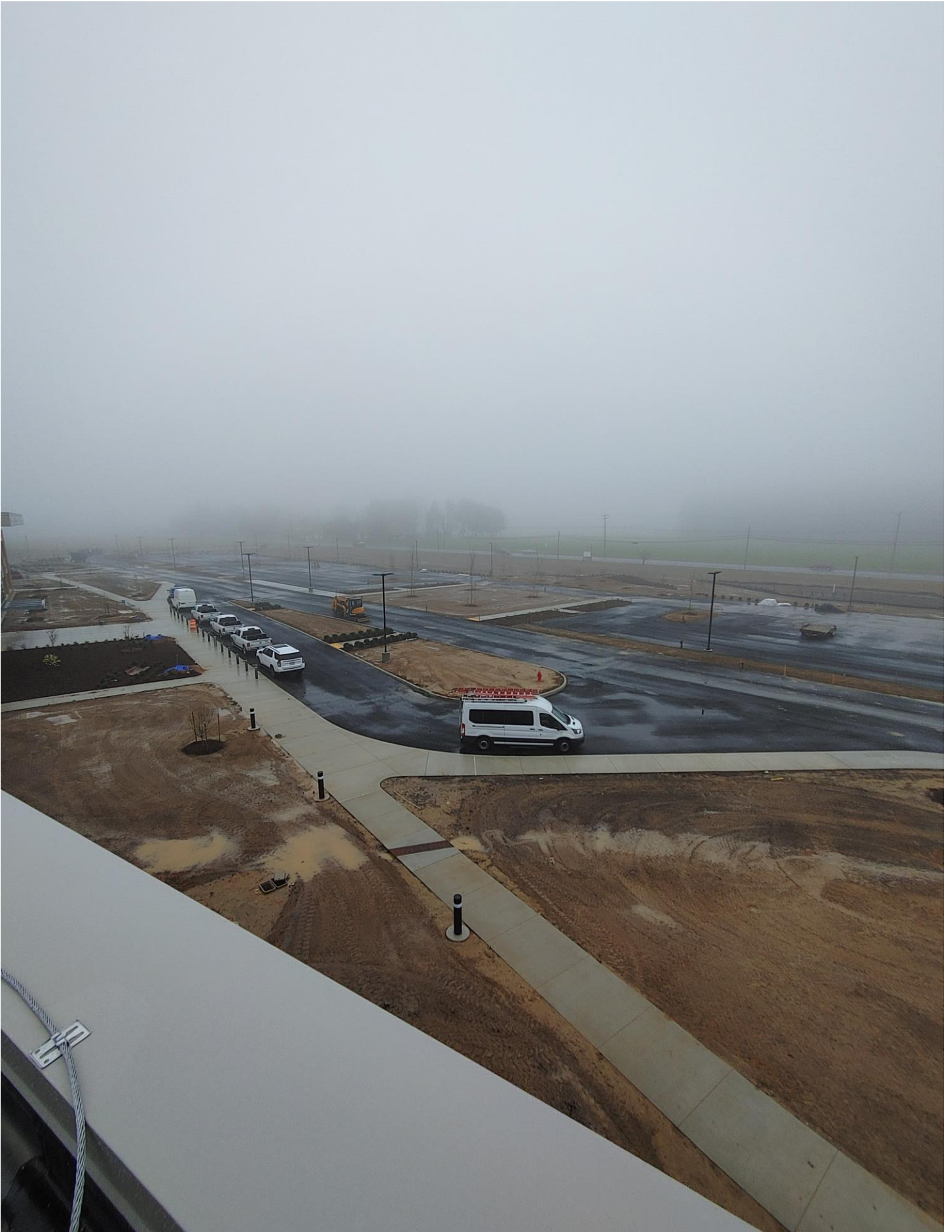
Photo 14 - Front of site
