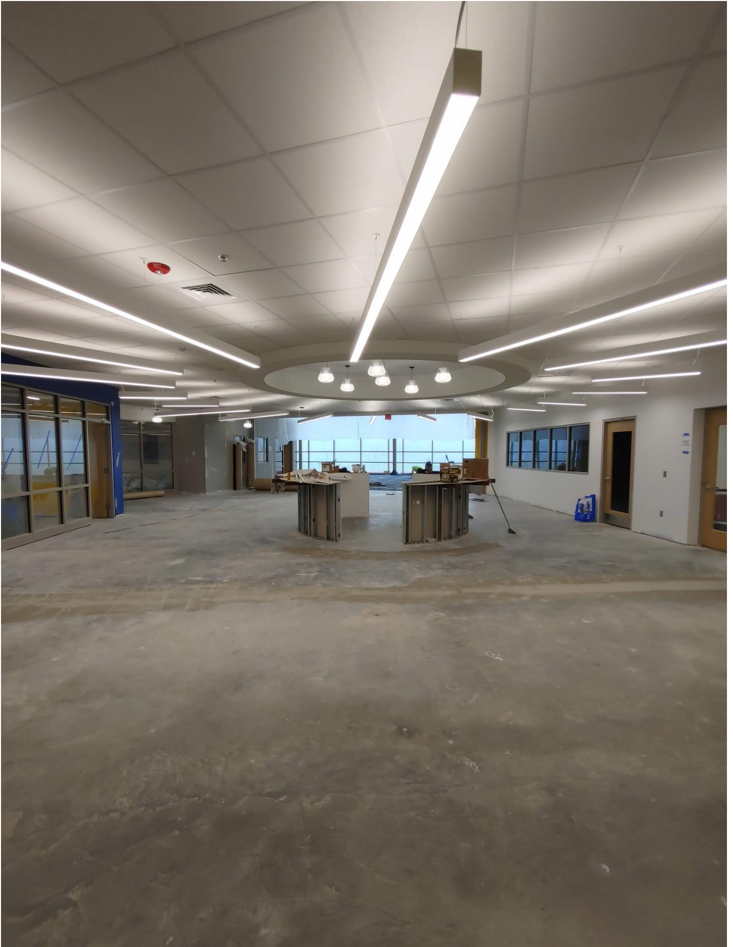
Photo 11 - Area A - 2nd Floor
