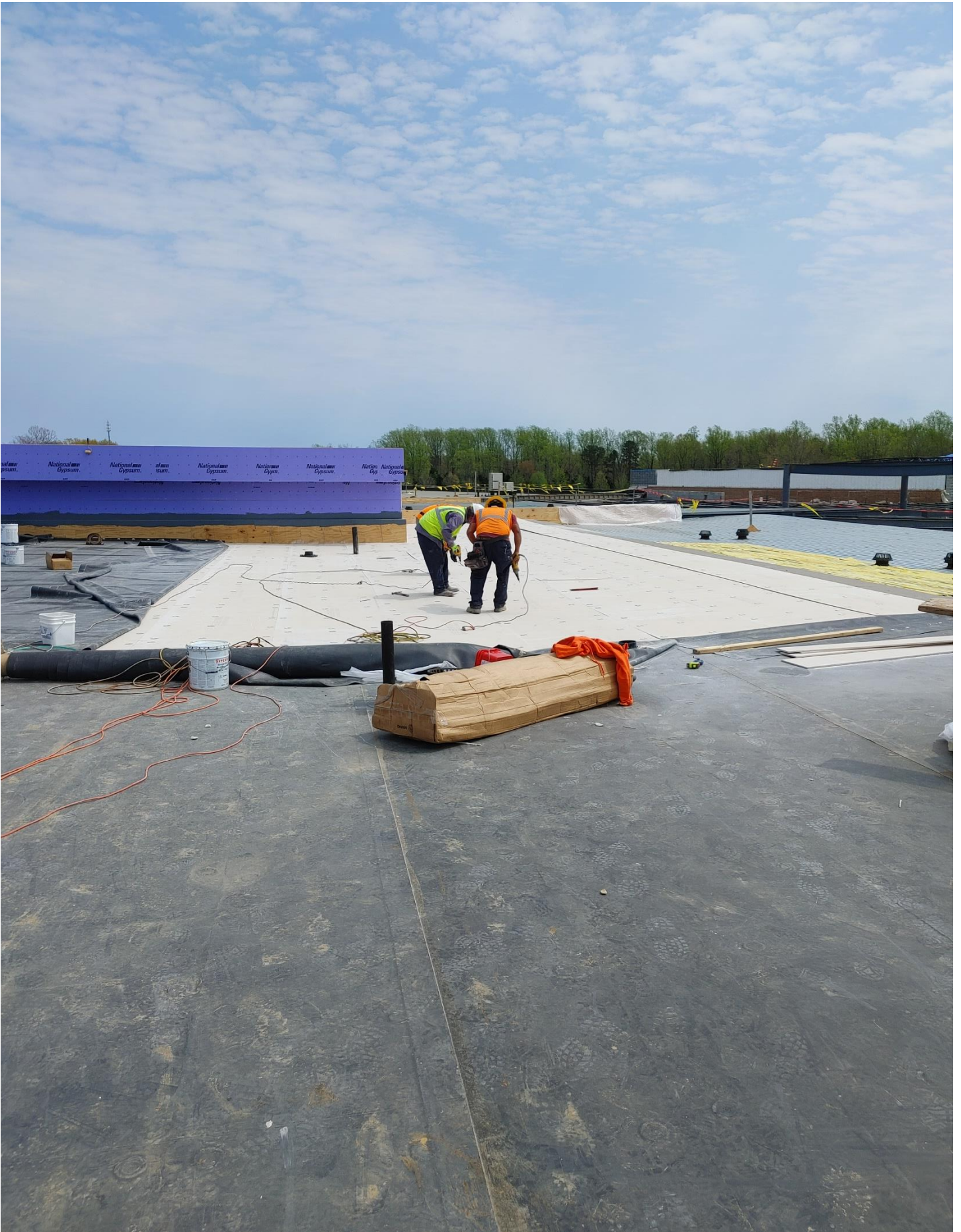
Photo 11 - Roofers working on Area B Roof
