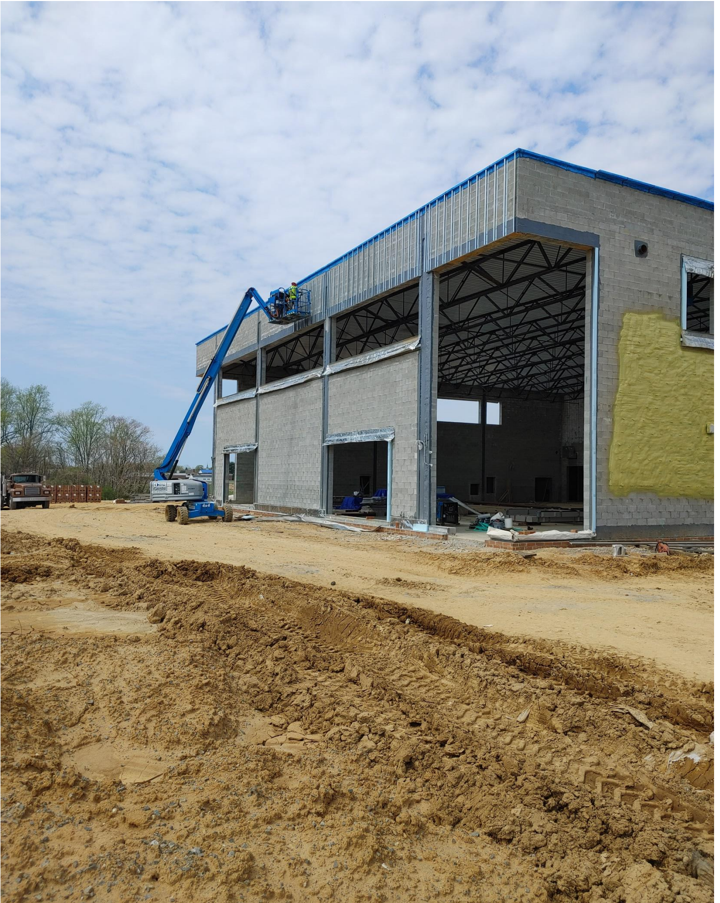
Photo 6 - Metal framing being installed on the Southside of Area E
