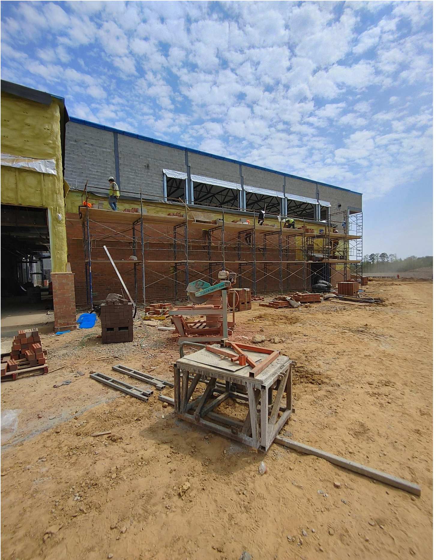
Photo 9 - Brick continues to be laid on the Westside of Area E
