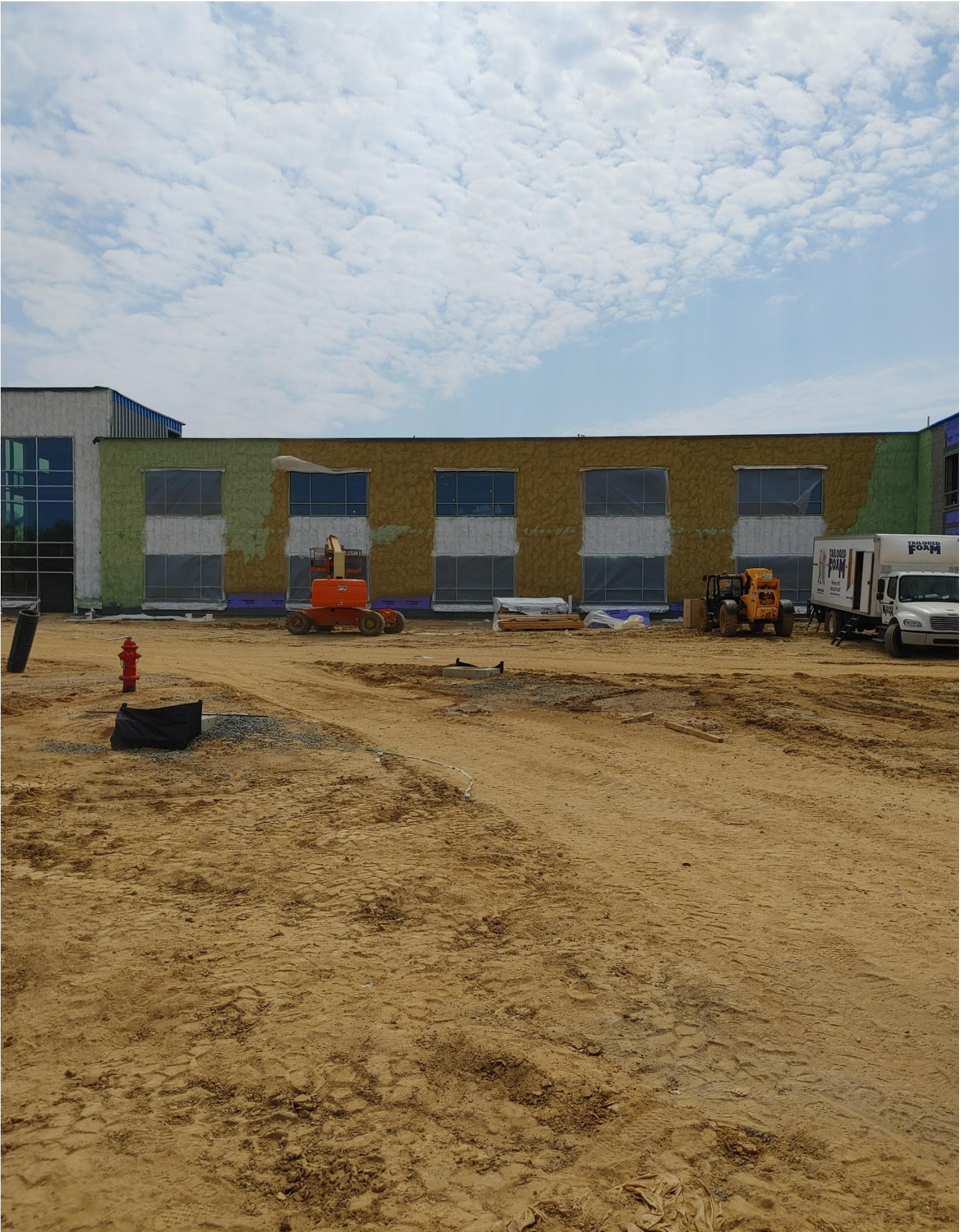
Photo 1 - Taylor Foam applying fire proofing coat under storefronts
