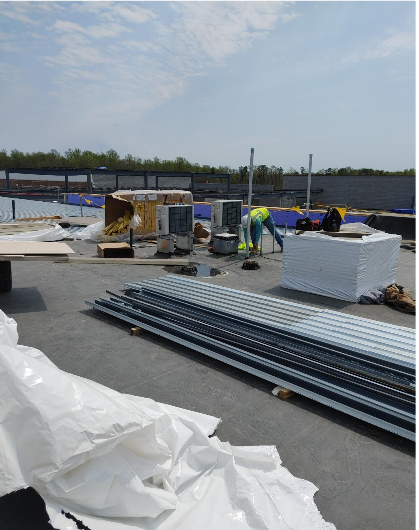
Photo 12 - Mini Splits being set on the roof of Area B
