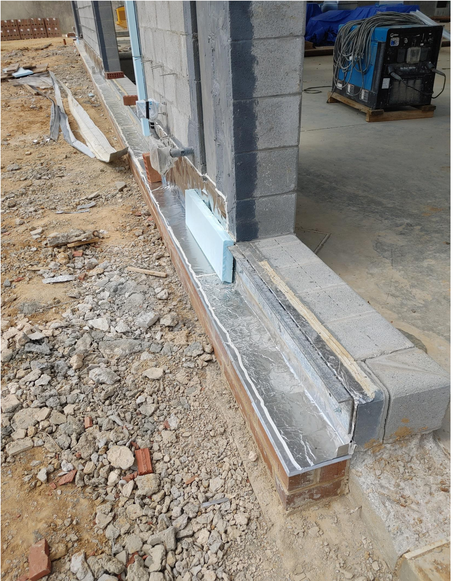
Photo 8 - Flashing installed and sealed on the Southside of Area E
