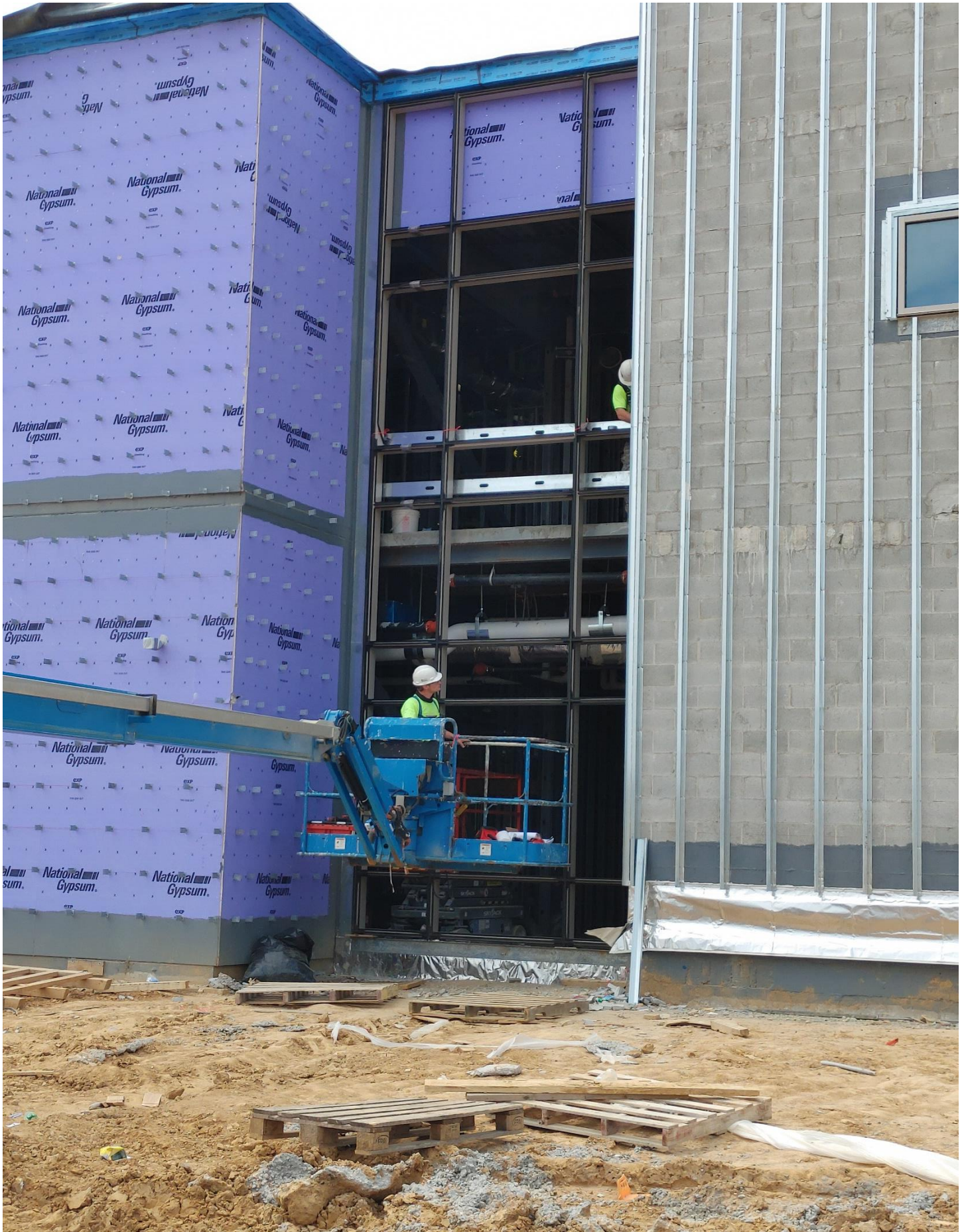
Photo 2 - FM&G working on large storefront on Eastside of Area A
