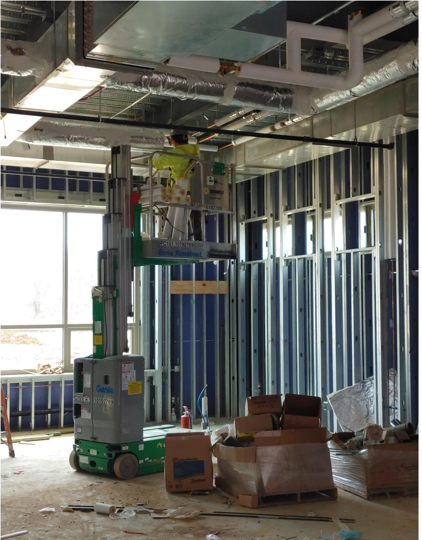
Photo 10 - Waterlines being insulated on the 1st floor of Area B
