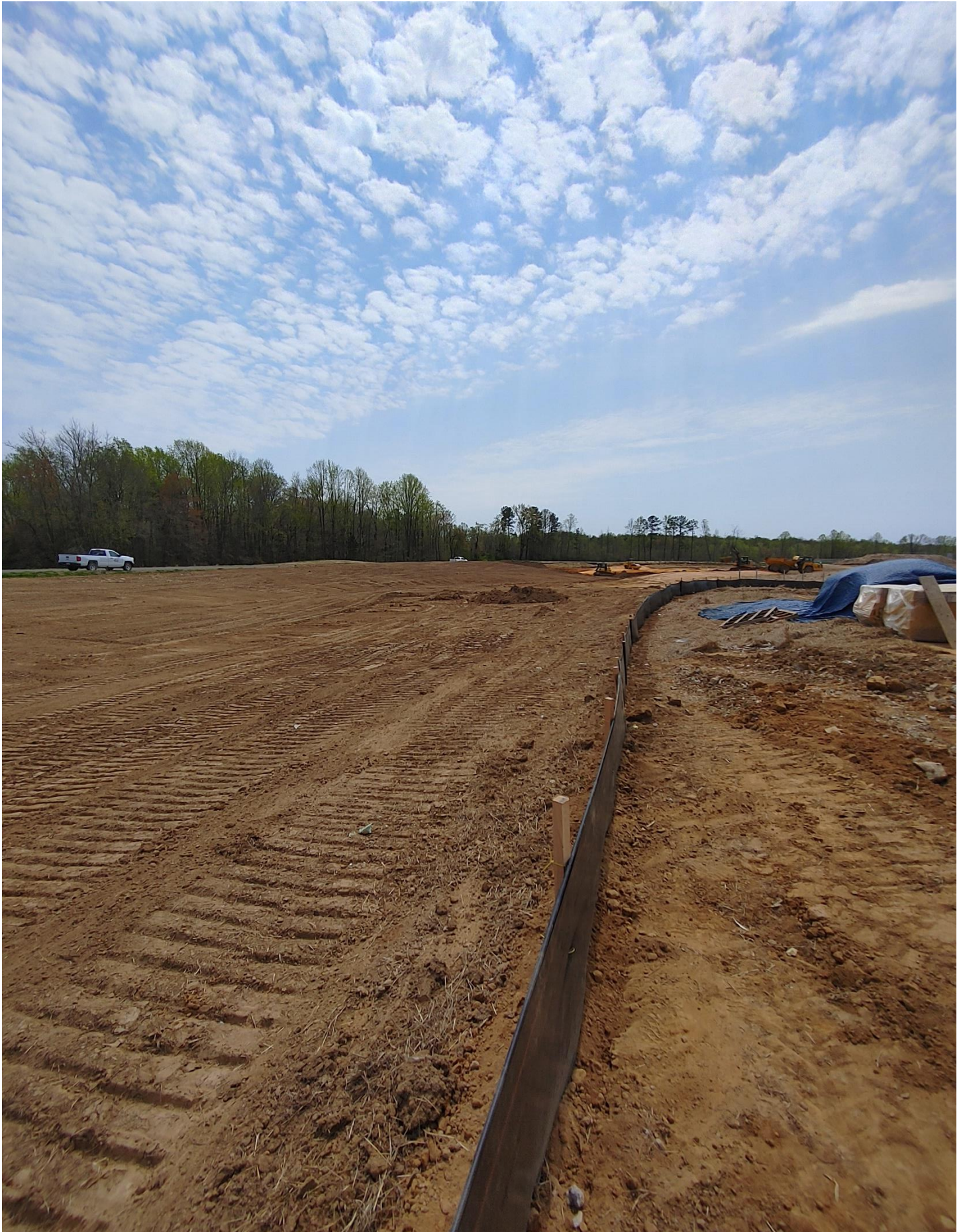
Photo 5 - Beuchert continues to work on the Eastside of the site.
