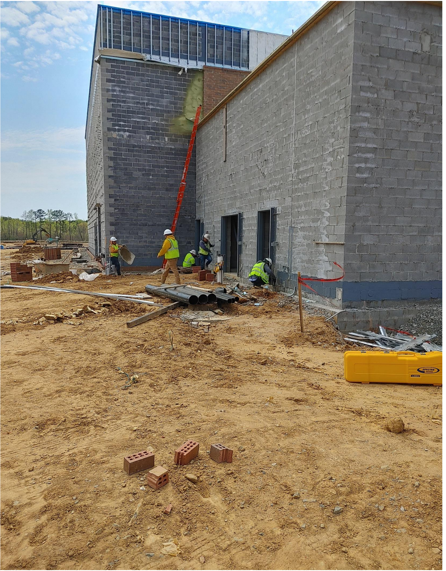
Photo 3 - Masons laying brick on the Eastside of Area D
