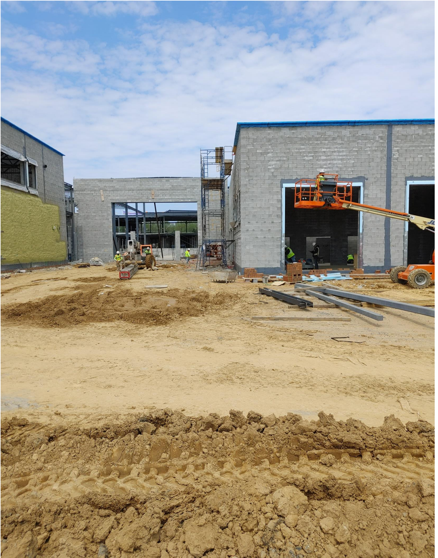
Photo 7 - Fraco Scaffolding being broken down on the Southside of Area C
