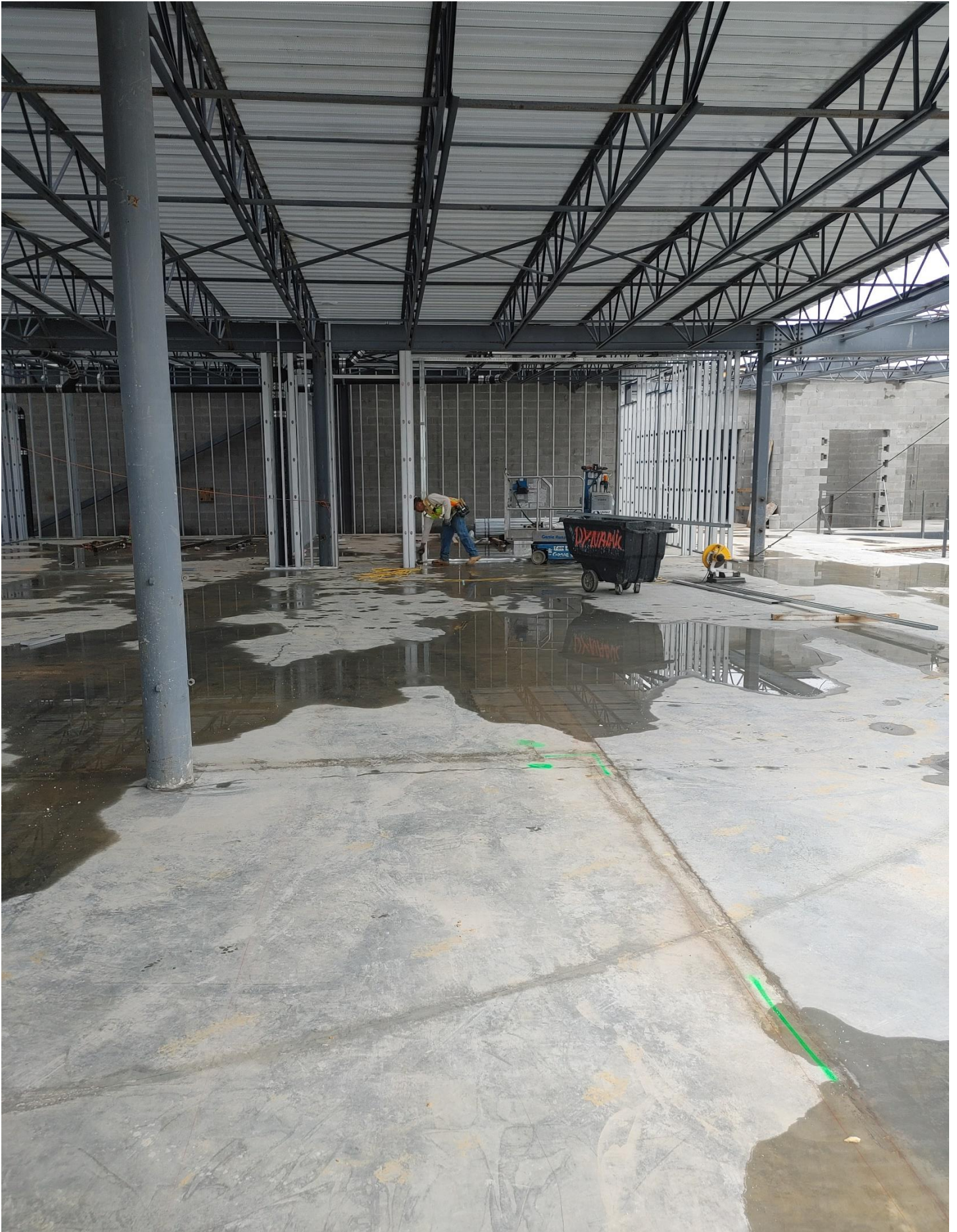
Photo 8 - Walls are being framed on the 2nd floor of Area A
