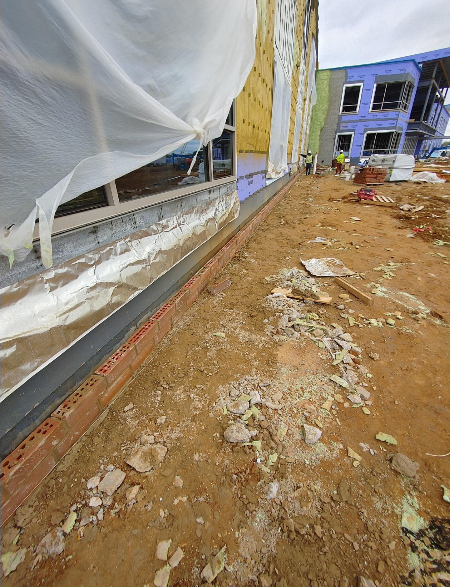
Photo 1 - Brick being laid on the Northside of Area A
