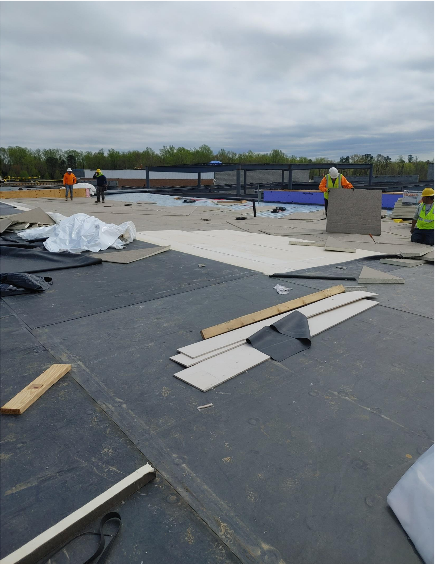
Photo 10 - Roofers continue to work on the Rook of Area B
