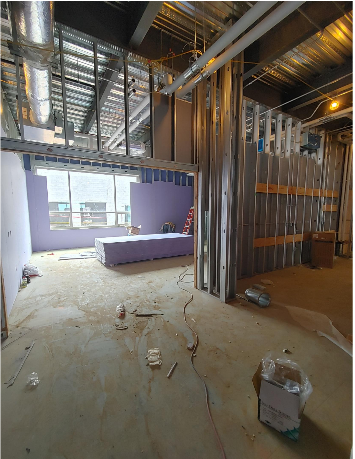
Photo 4 - Sheetrock being hung in Area A
