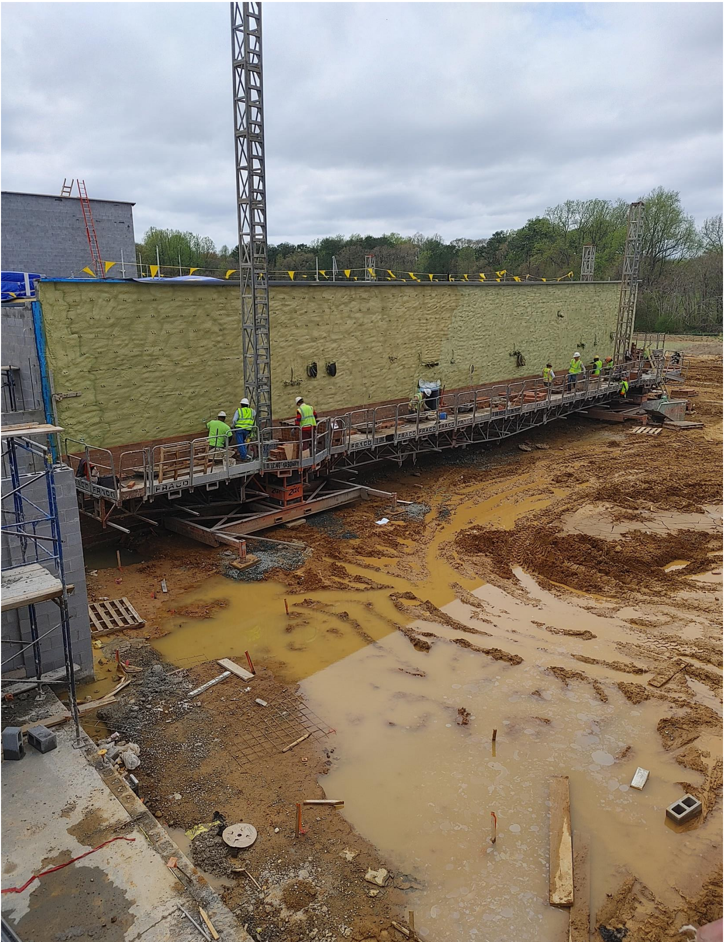
Photo 9 - Masons are laying Brick on the Northside of Area E
