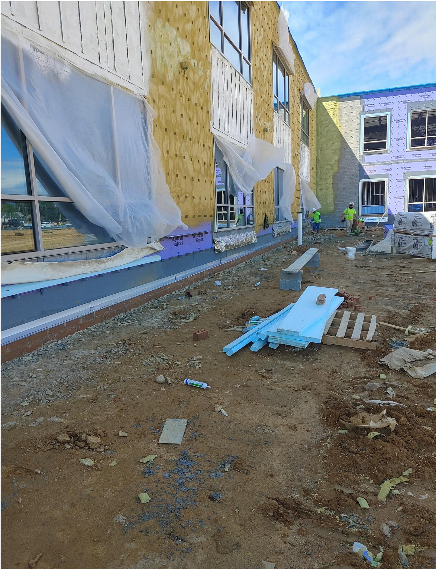
Photo 1 – Flashing being installed on the Northside of Area A
