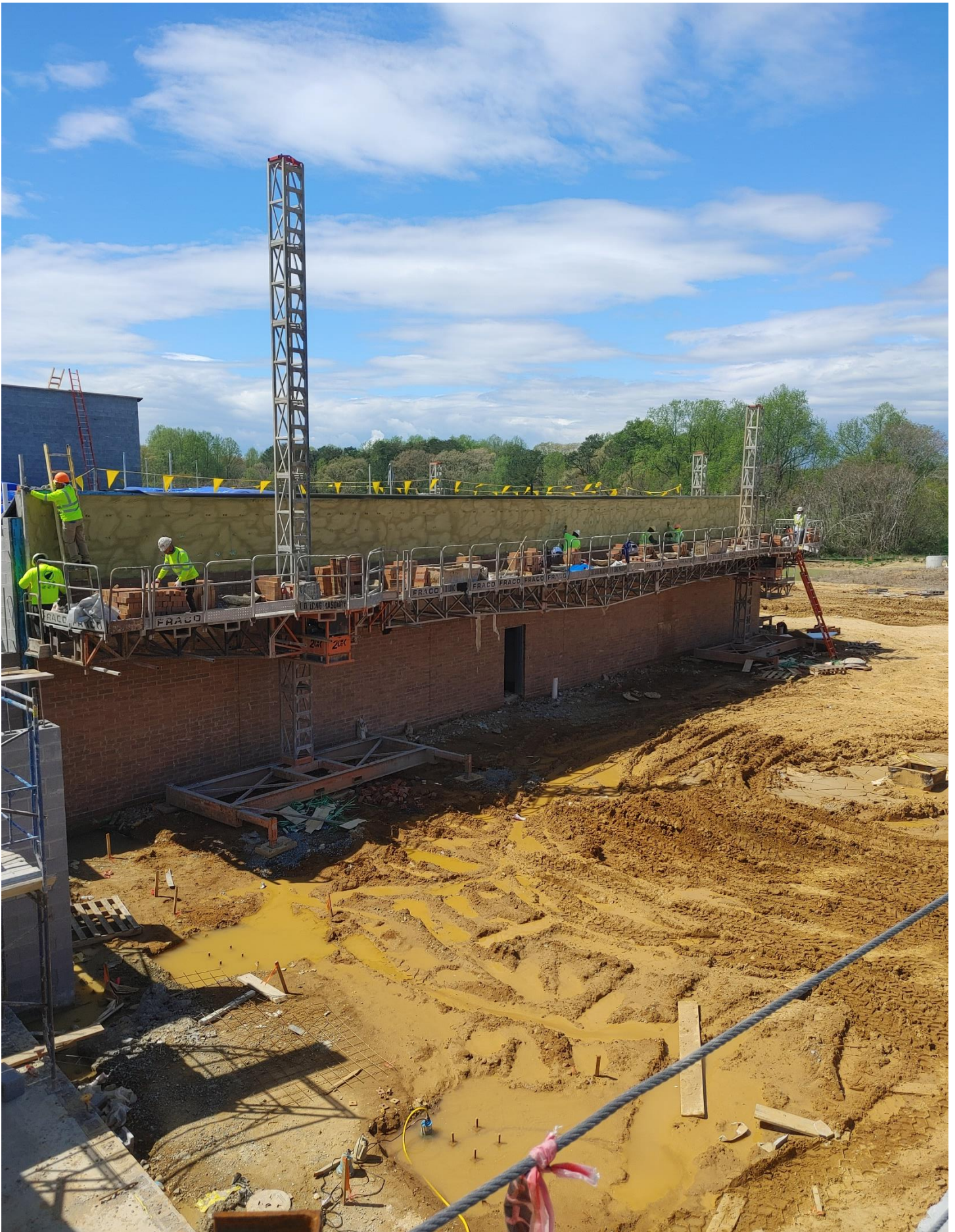
Photo 10 - Brick continues to be laid on the Northside of Area E
