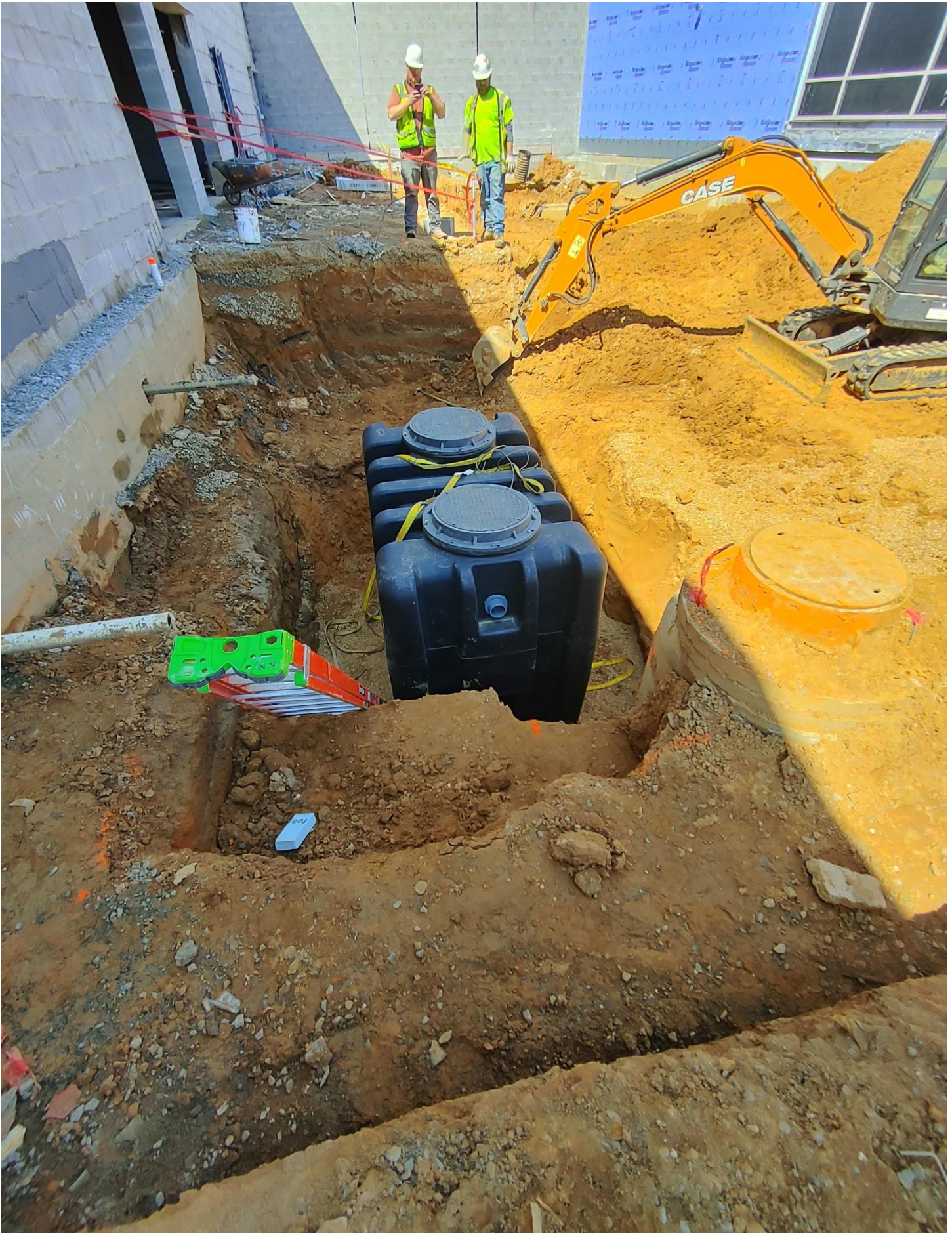
Photo 5 - Grease Trap has been set
