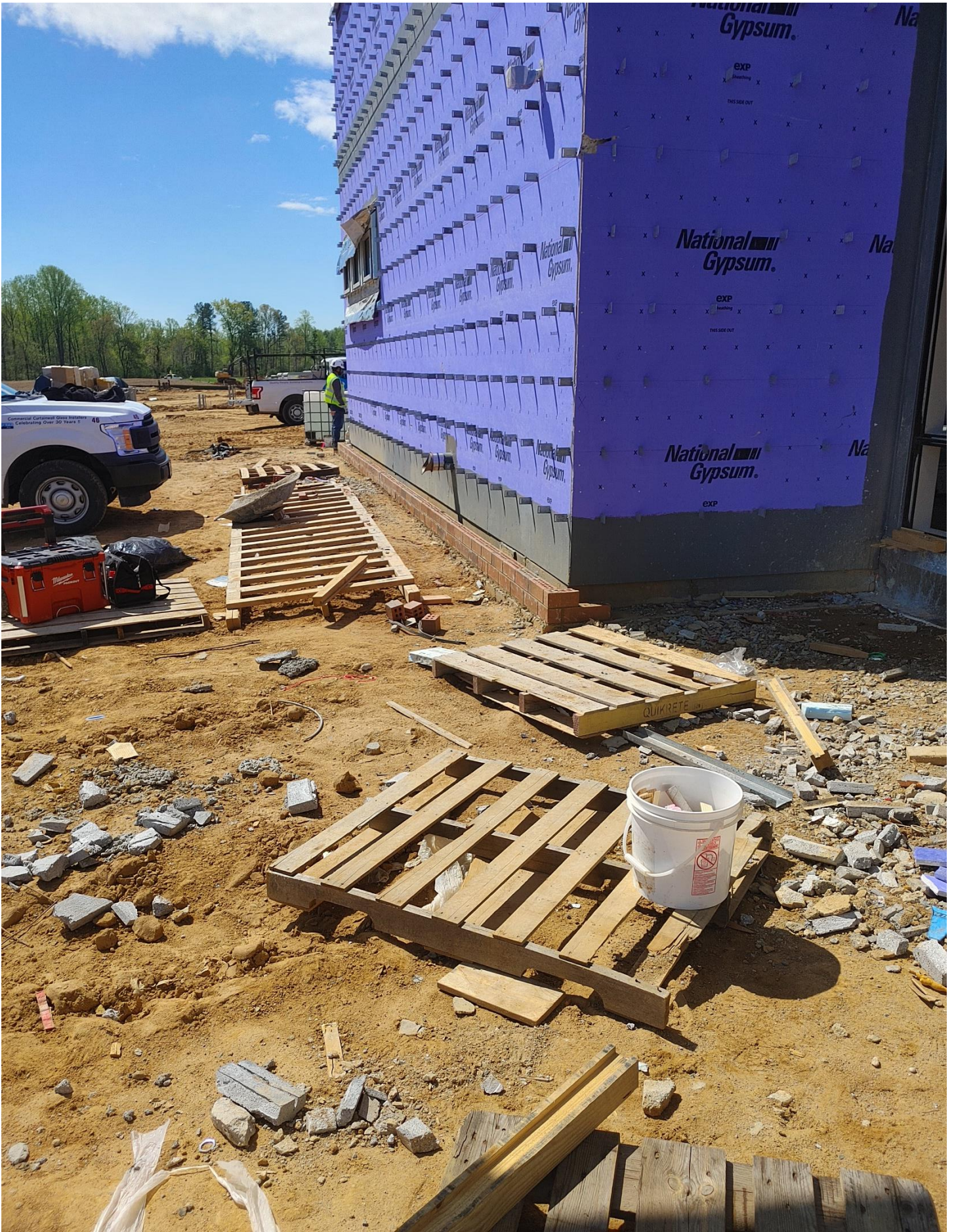
Photo 4 - Brick continues to be laid on the Eastside of Area A
