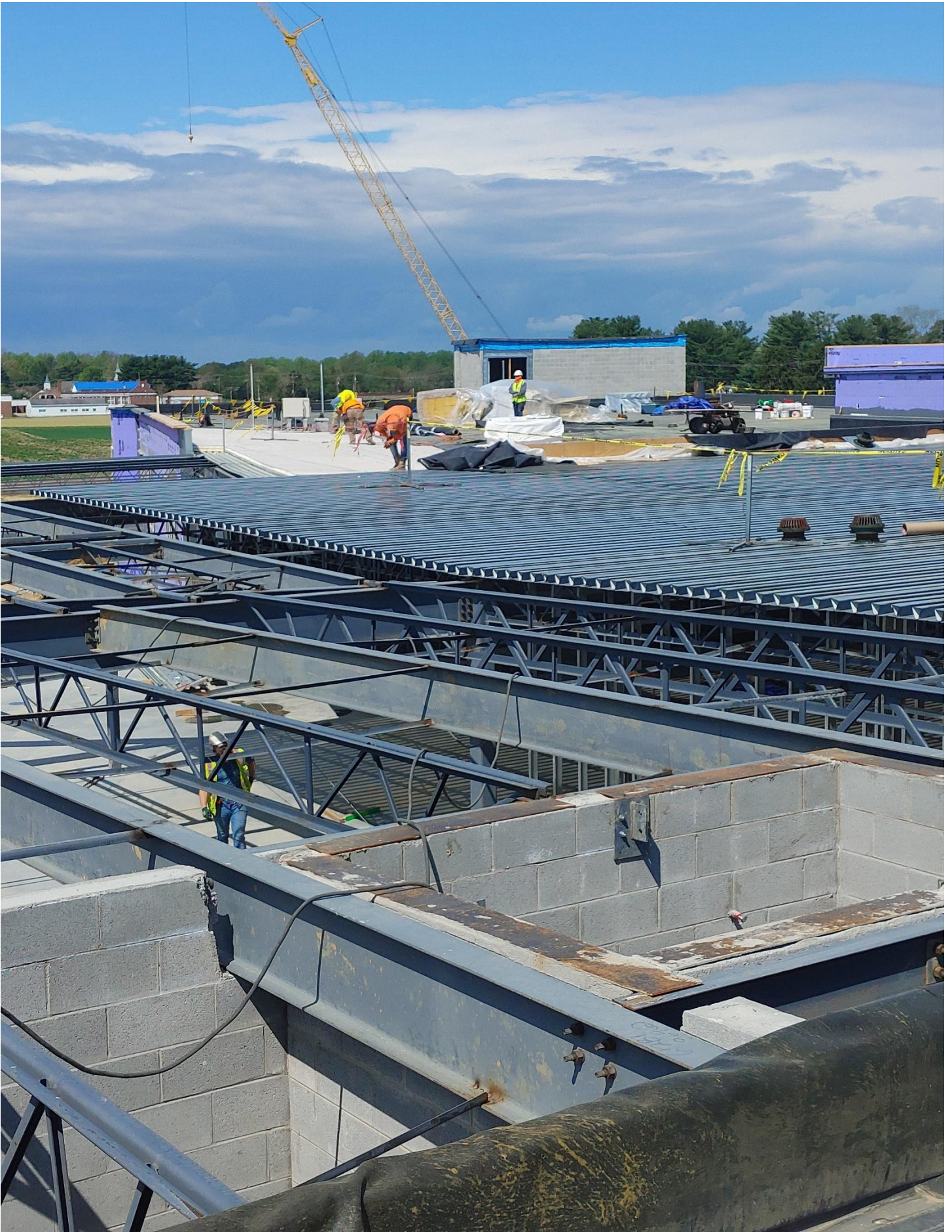
Photo 7 - Roofer continue to work on the roof of Area A
