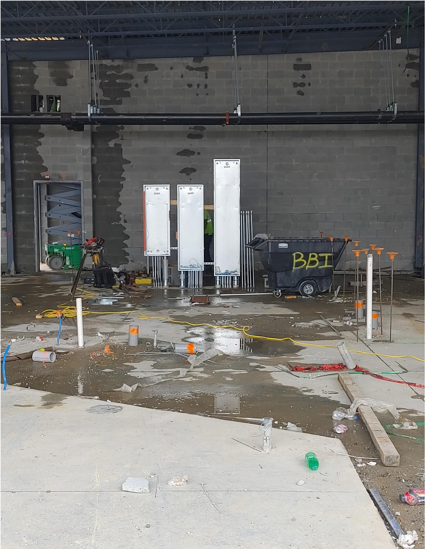
Photo 5 - Hazzard Electric setting Panel Boxes in the Kitchen Area
