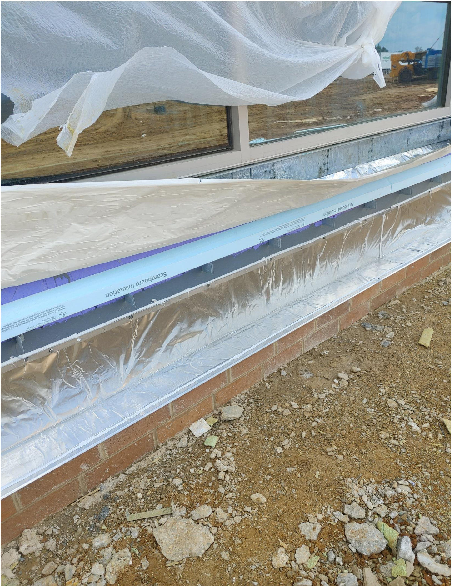
Photo 14 - Completed Brick Flashing on the Northside of Area A
