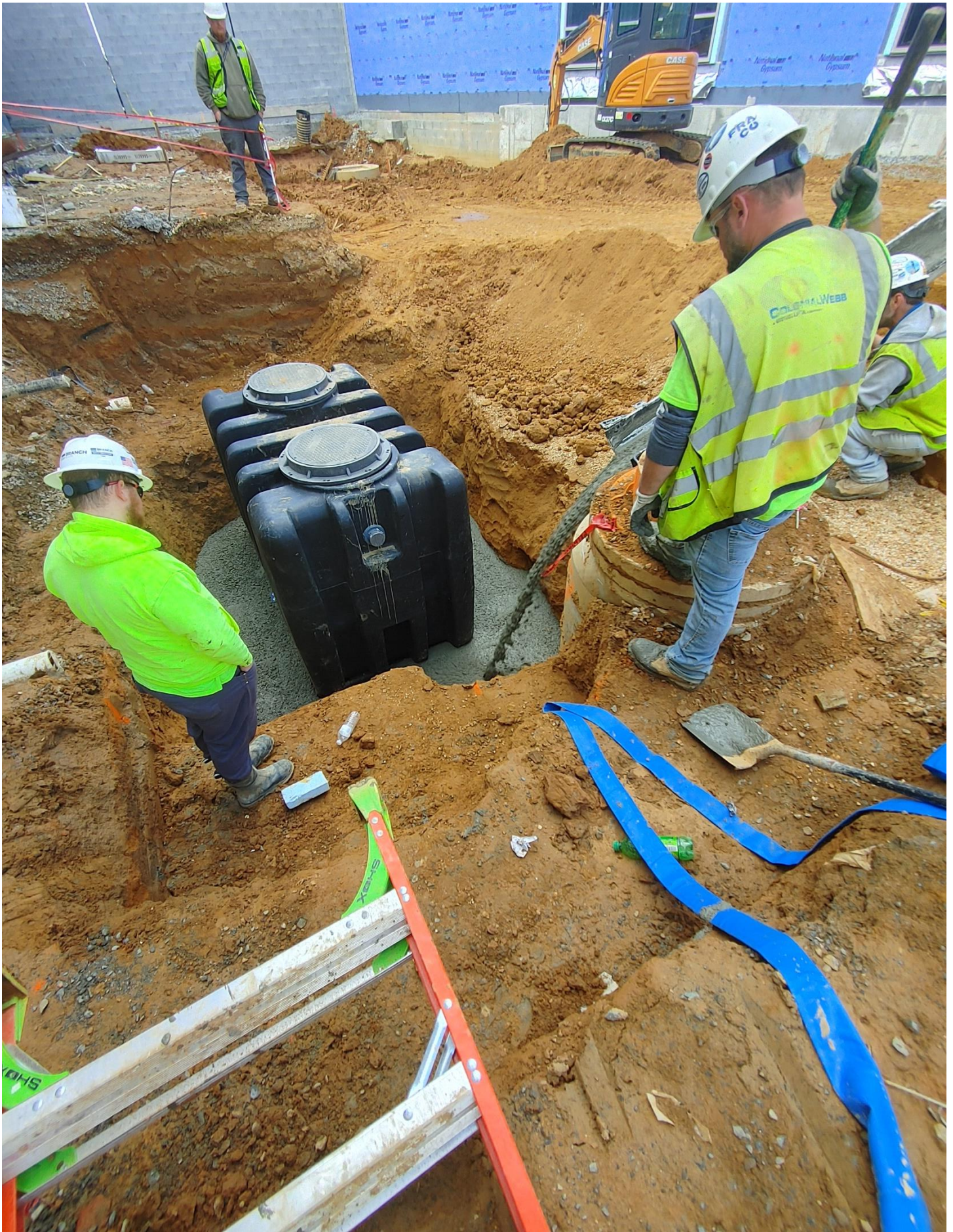
Photo 2 - Concrete being poured around Grease Trap
