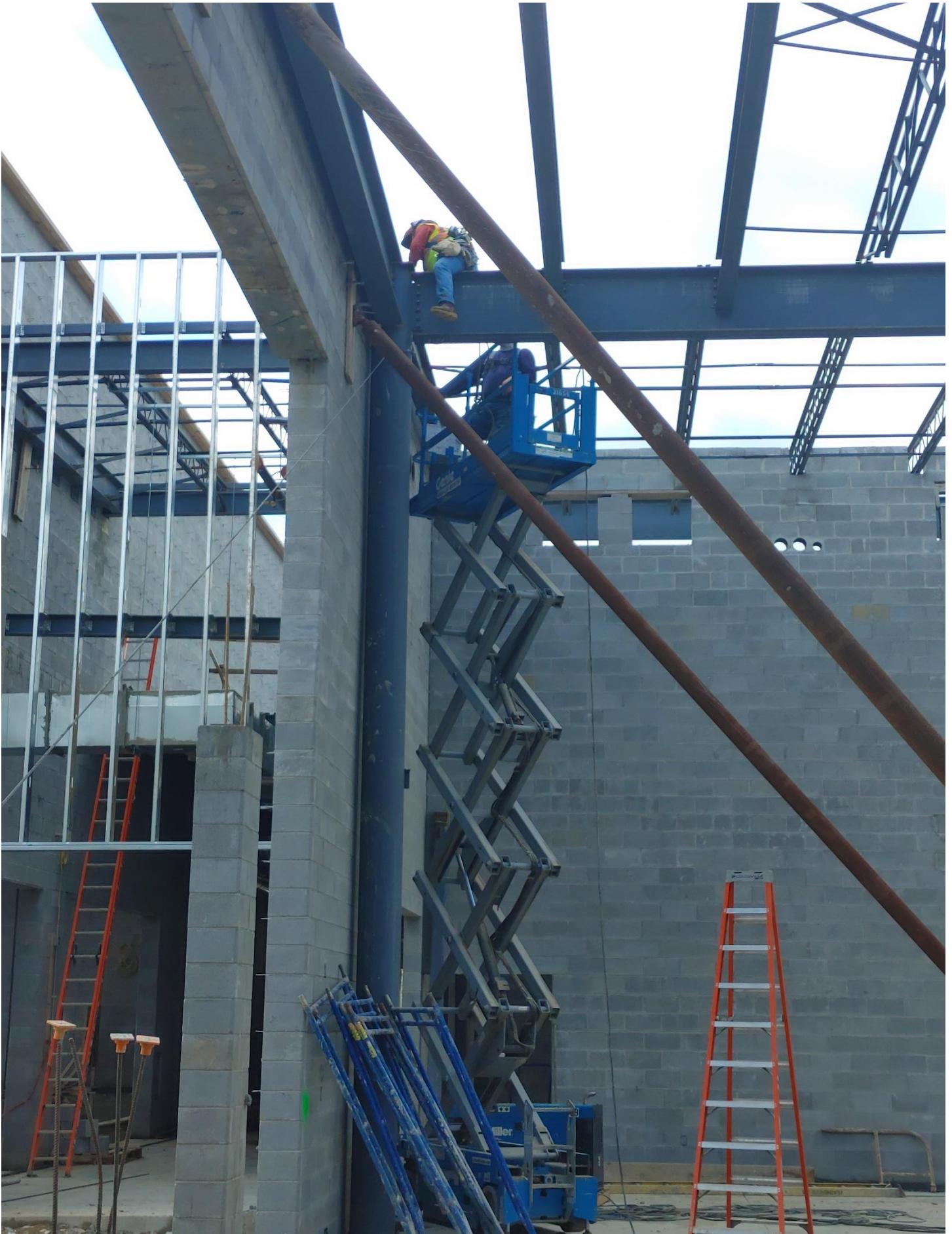
Photo 3 - Steel being welded in Area C
