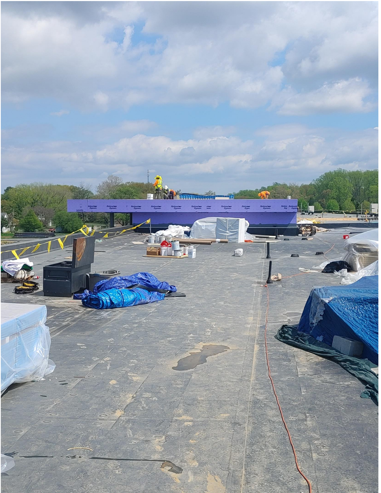
Photo 11 - Roofers working on the high roof of Area A
