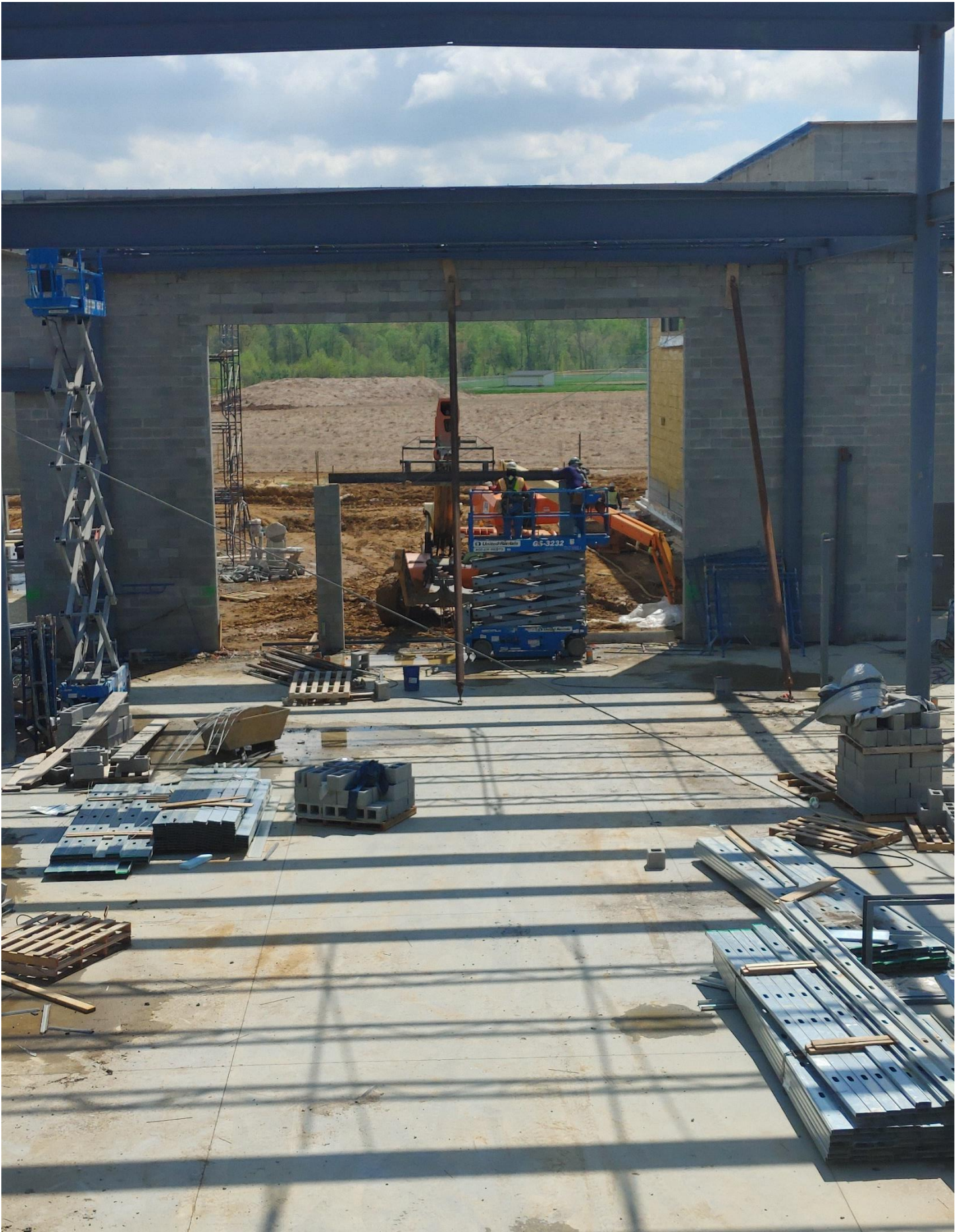
Photo 12 - Weldon Steel setting steel I-Beam in Area C
