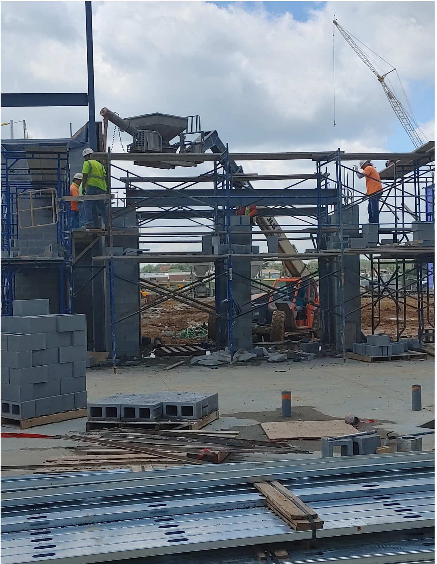
Photo 6 - Block being laid and Grouted in Vestibule C10
