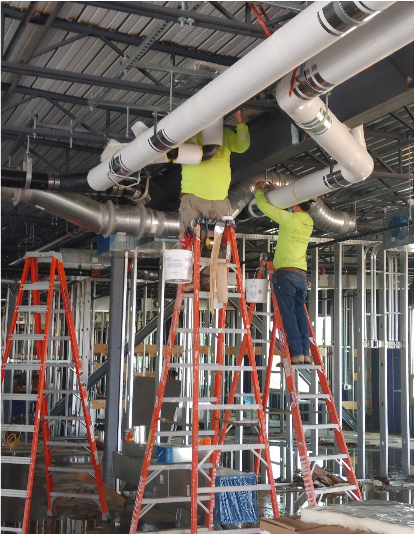
Photo 10 - Pipe being insulated in Area B
