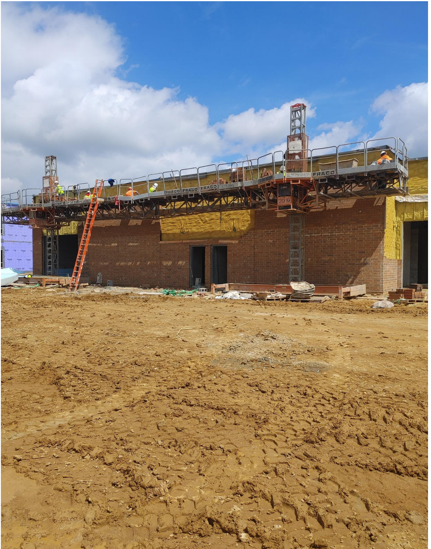
Photo 7 - Masons laying Brick on the Westside of Area E
