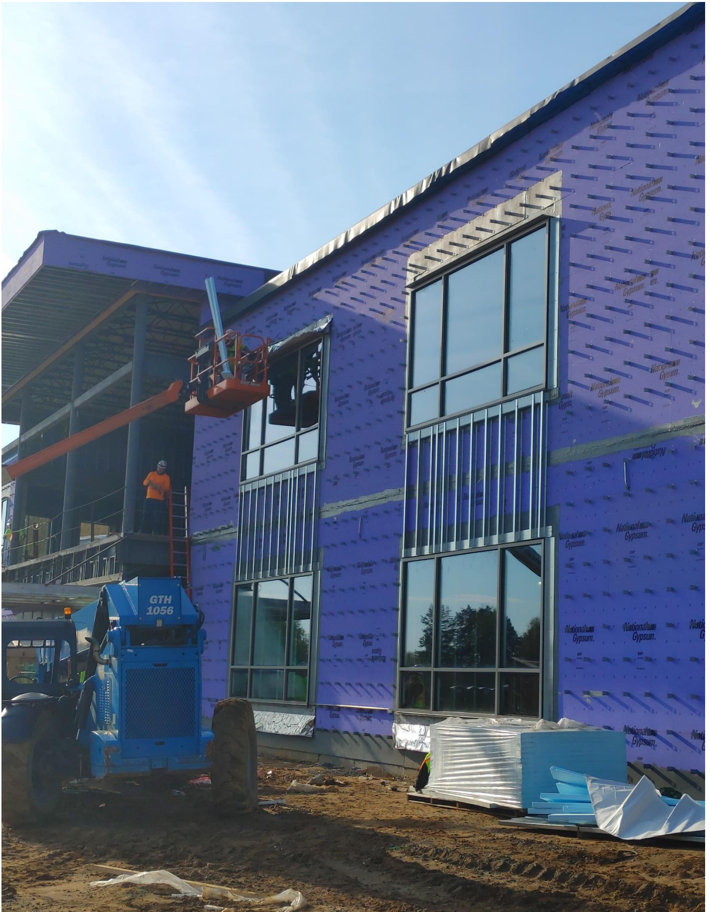
Photo 5 - Windows are being flashed on the Northside of Area B
