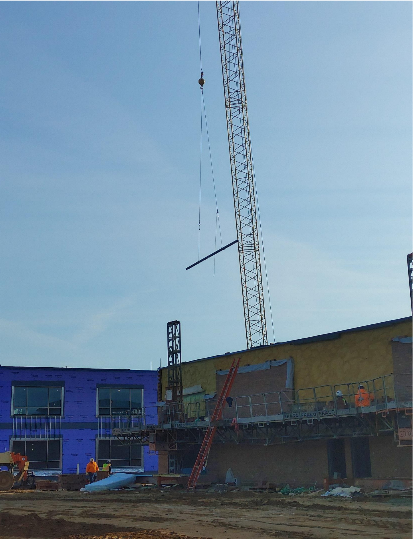
Photo 3 - Weldon Steel setting steel in Area C
