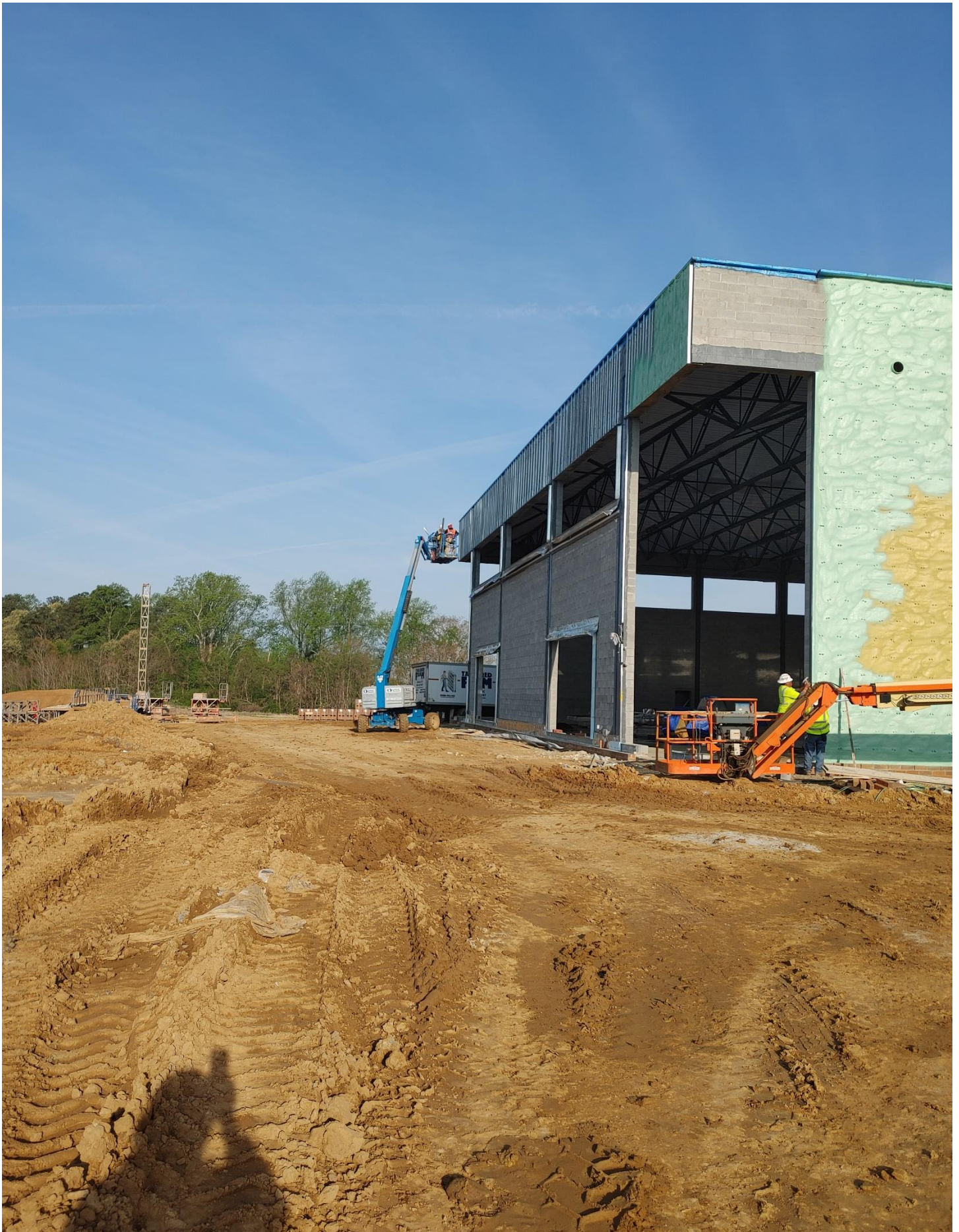
Photo 1 - JP installing metal framing on the Southside of Area E
