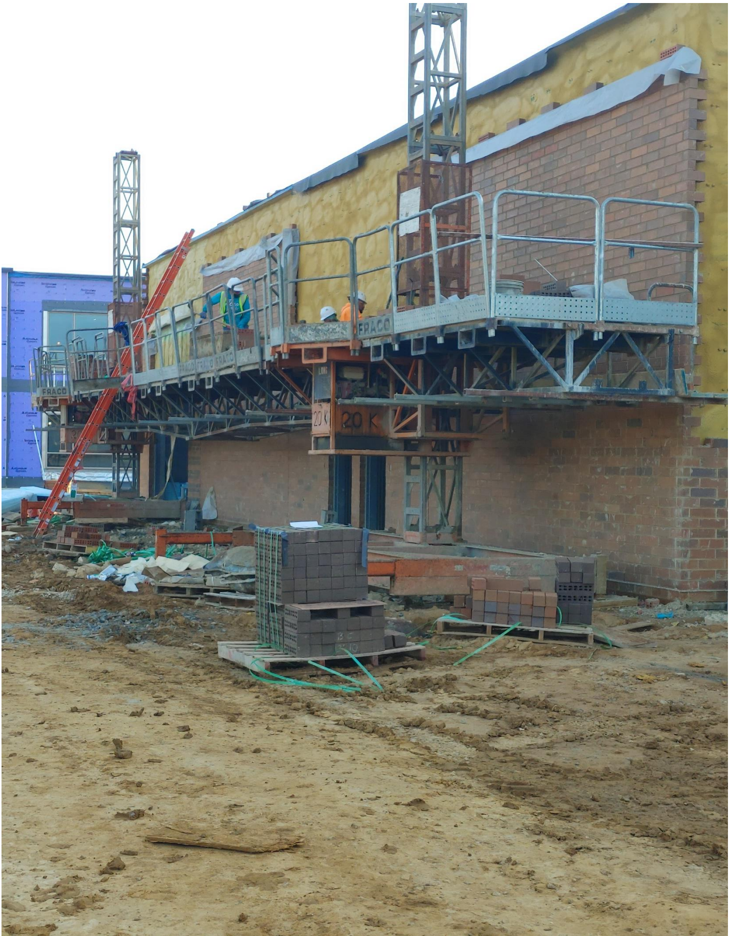
Photo 4 - Masons laying brick on the Westside of Area E
