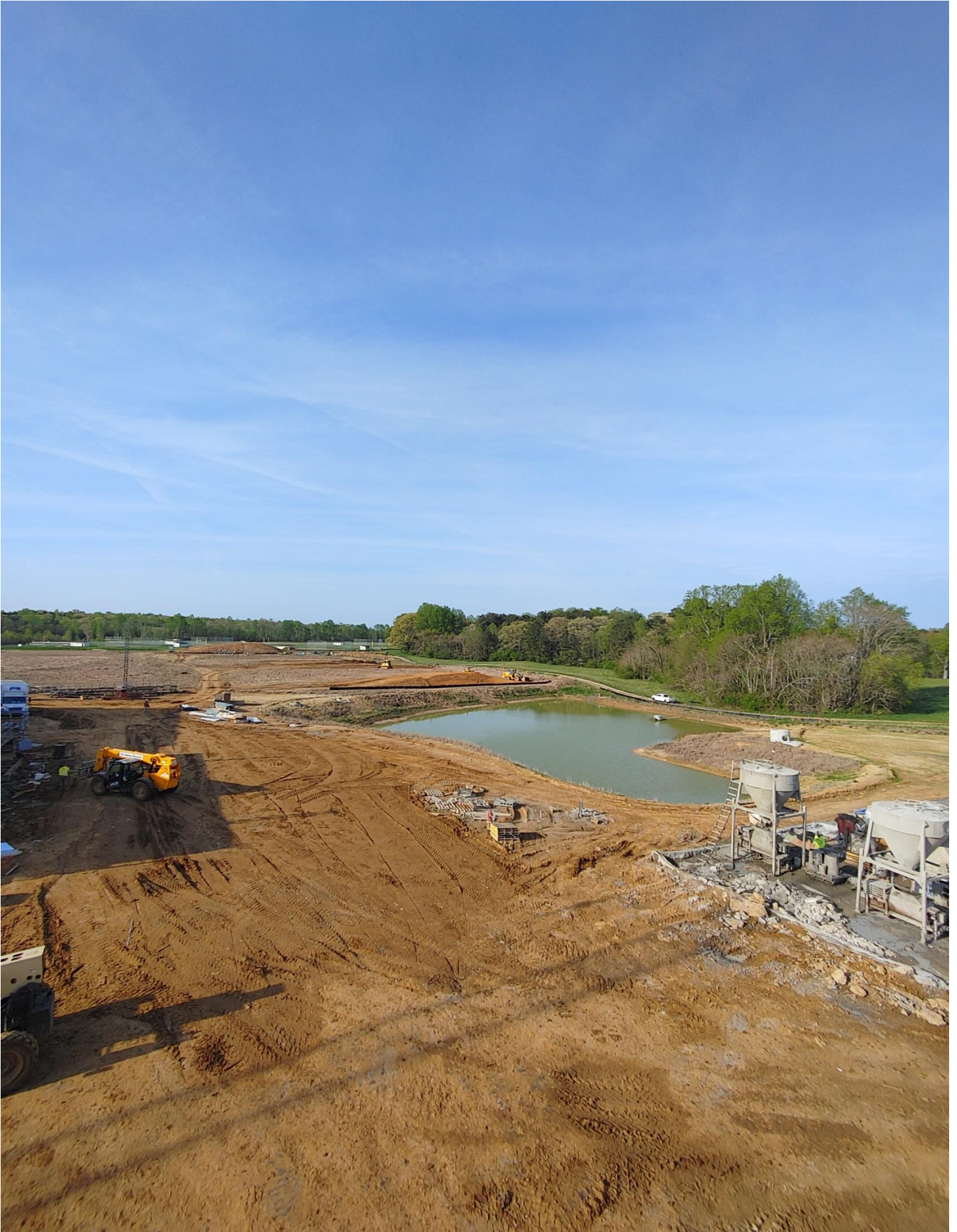
Photo 9 - Beuchert continues to work on the Westside of the Site.
