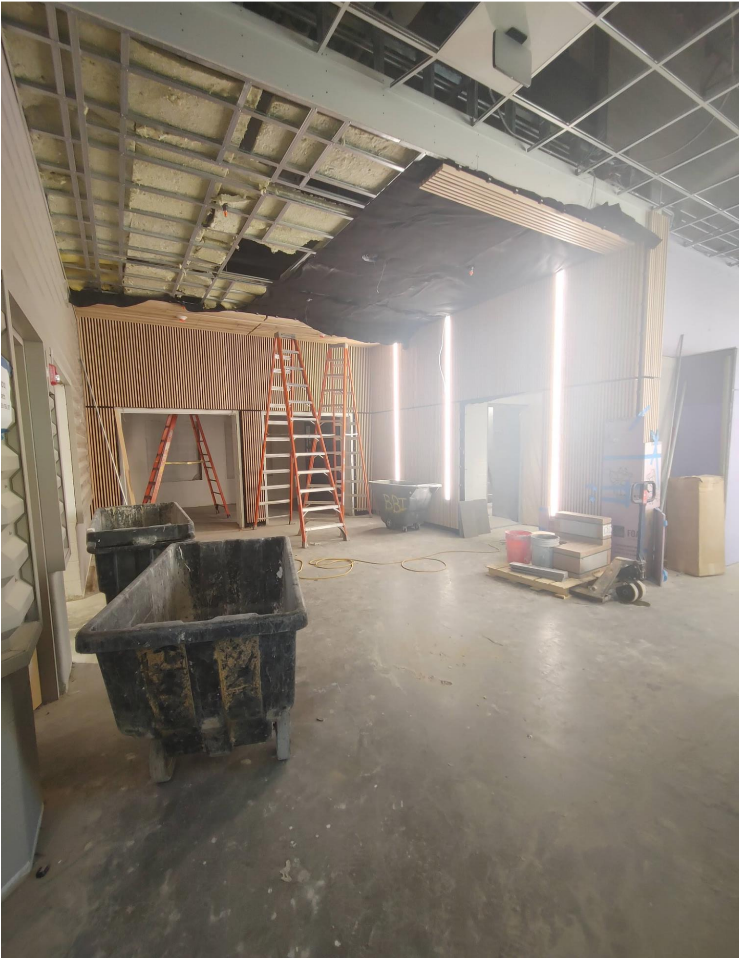
Photo 3 - Wood Wall is being installed outside of Auditorium
