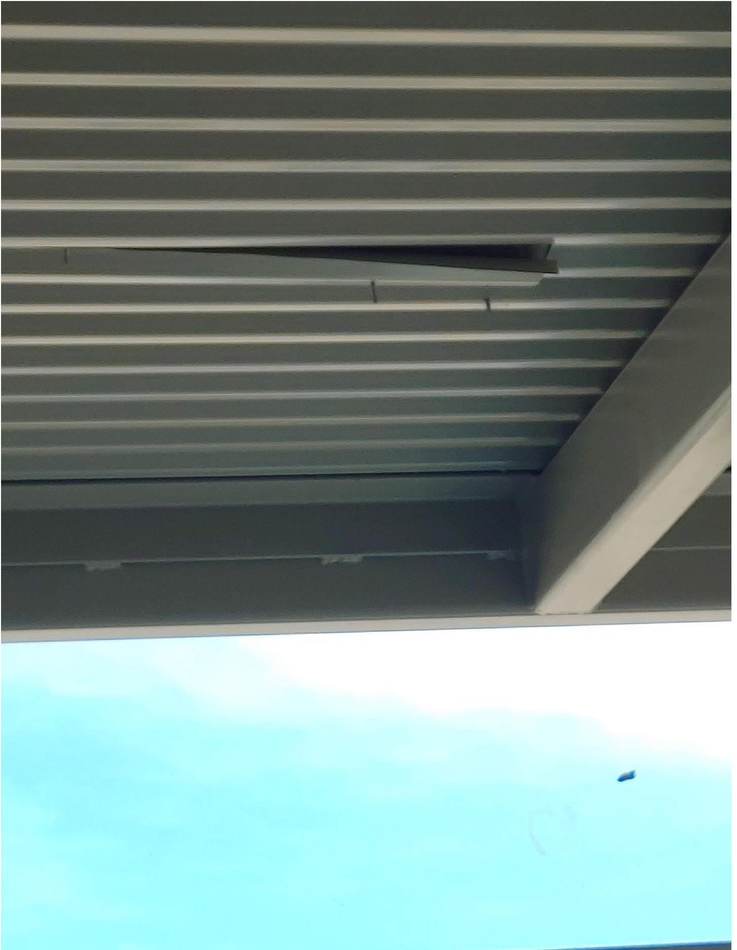
Photo 14 - Metal Pan of second landing in Stairwell #1
