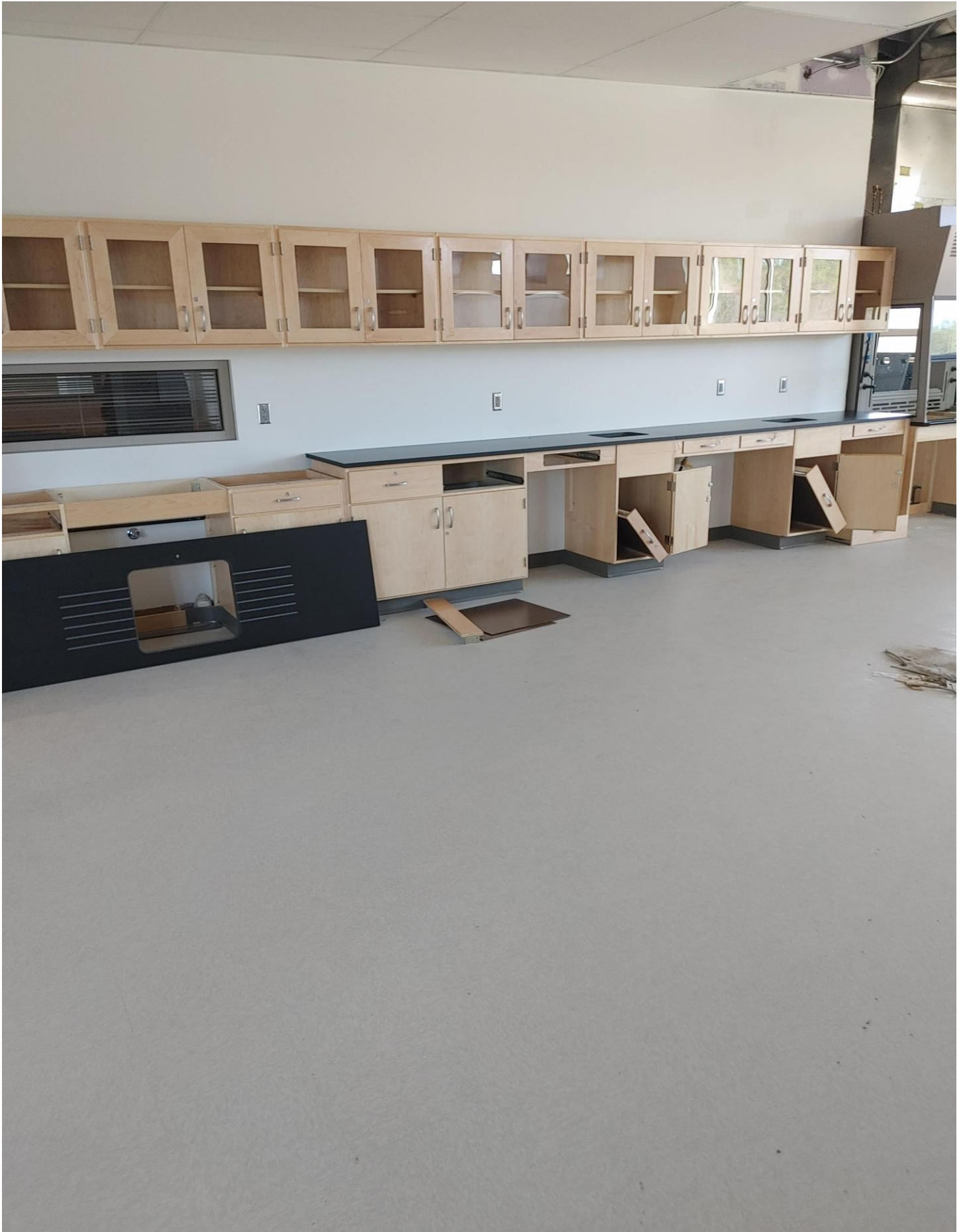
Photo 18 - Counter tops are being installed in Area B, 2nd floor
