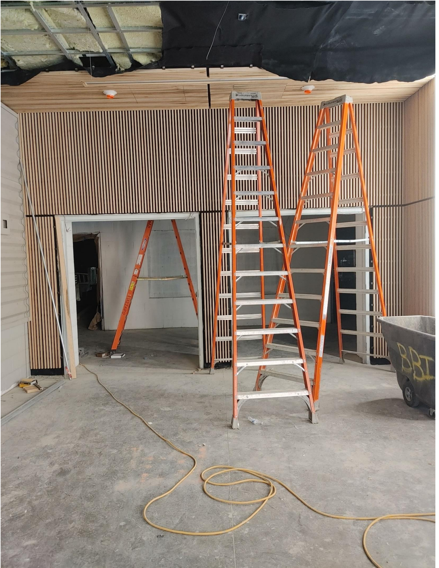
Photo 4 - Wood Wall at Auditorium Entrance
