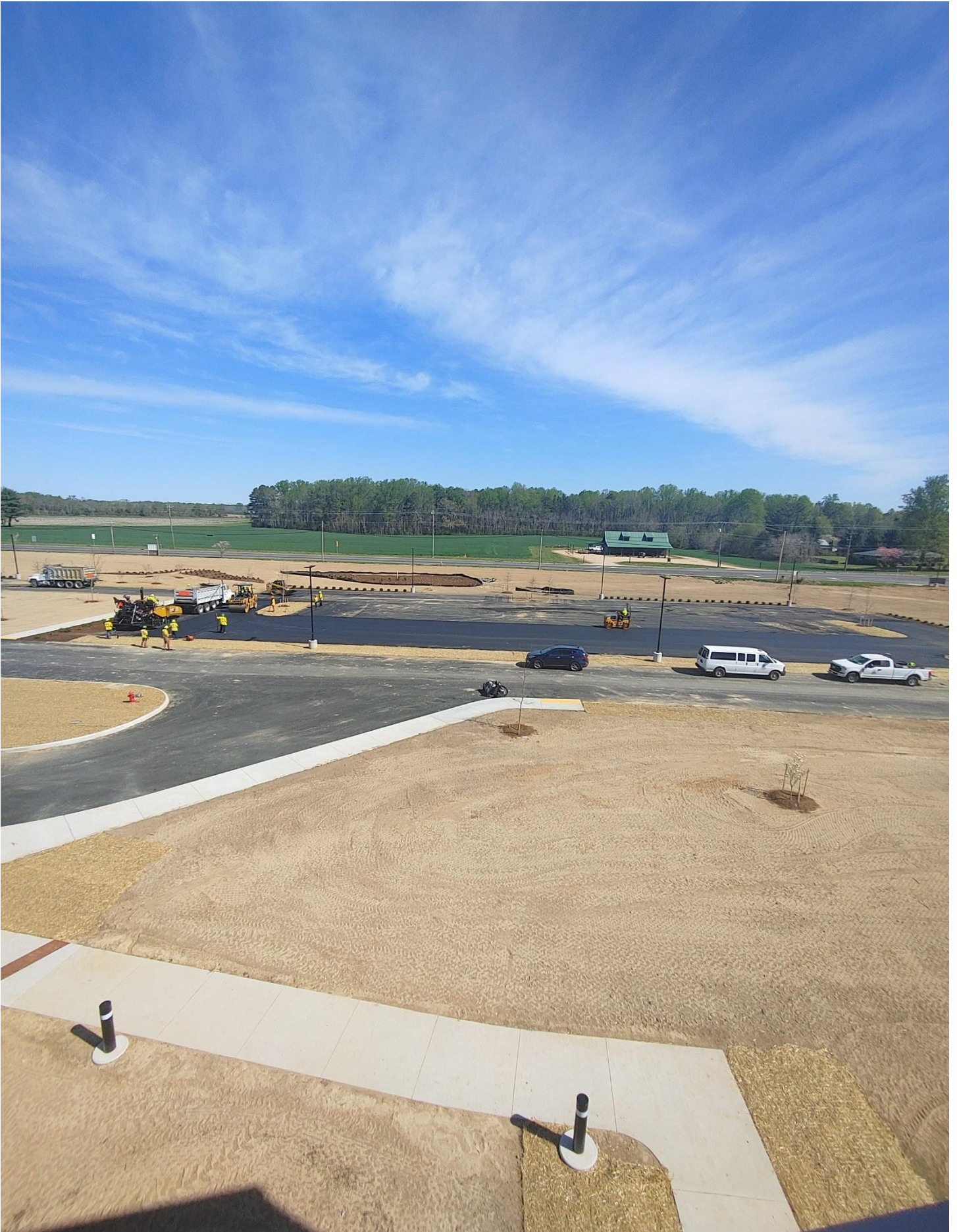
Photo 15 - Topping Layer of Asphalt being laid in the front Parking lot.
