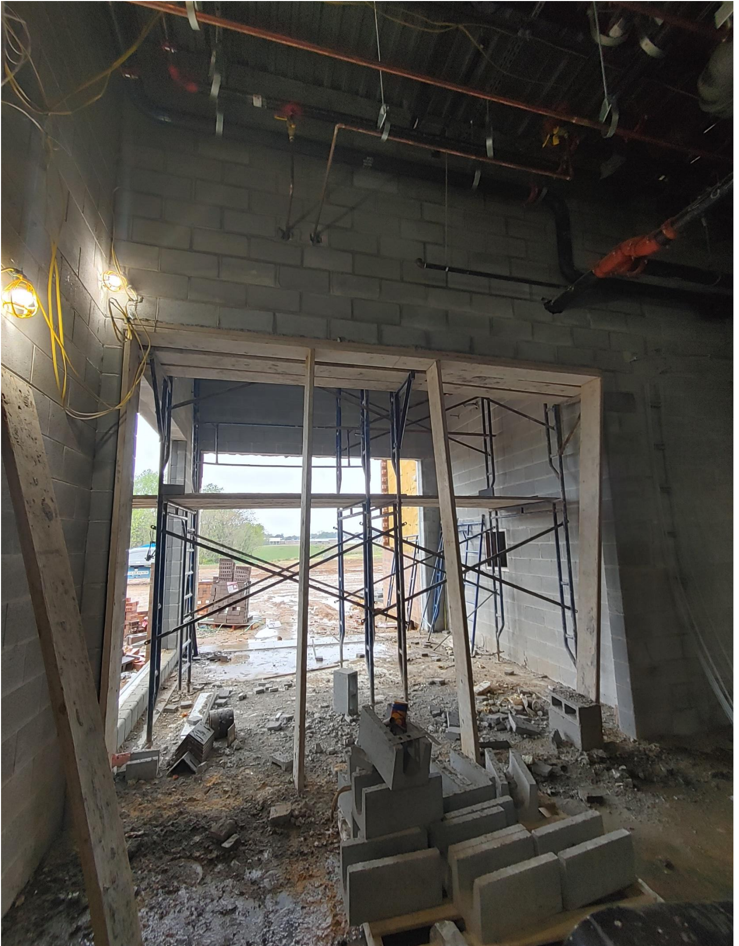
Photo 7 - Masons laid block above E10A & 10B, Area E
