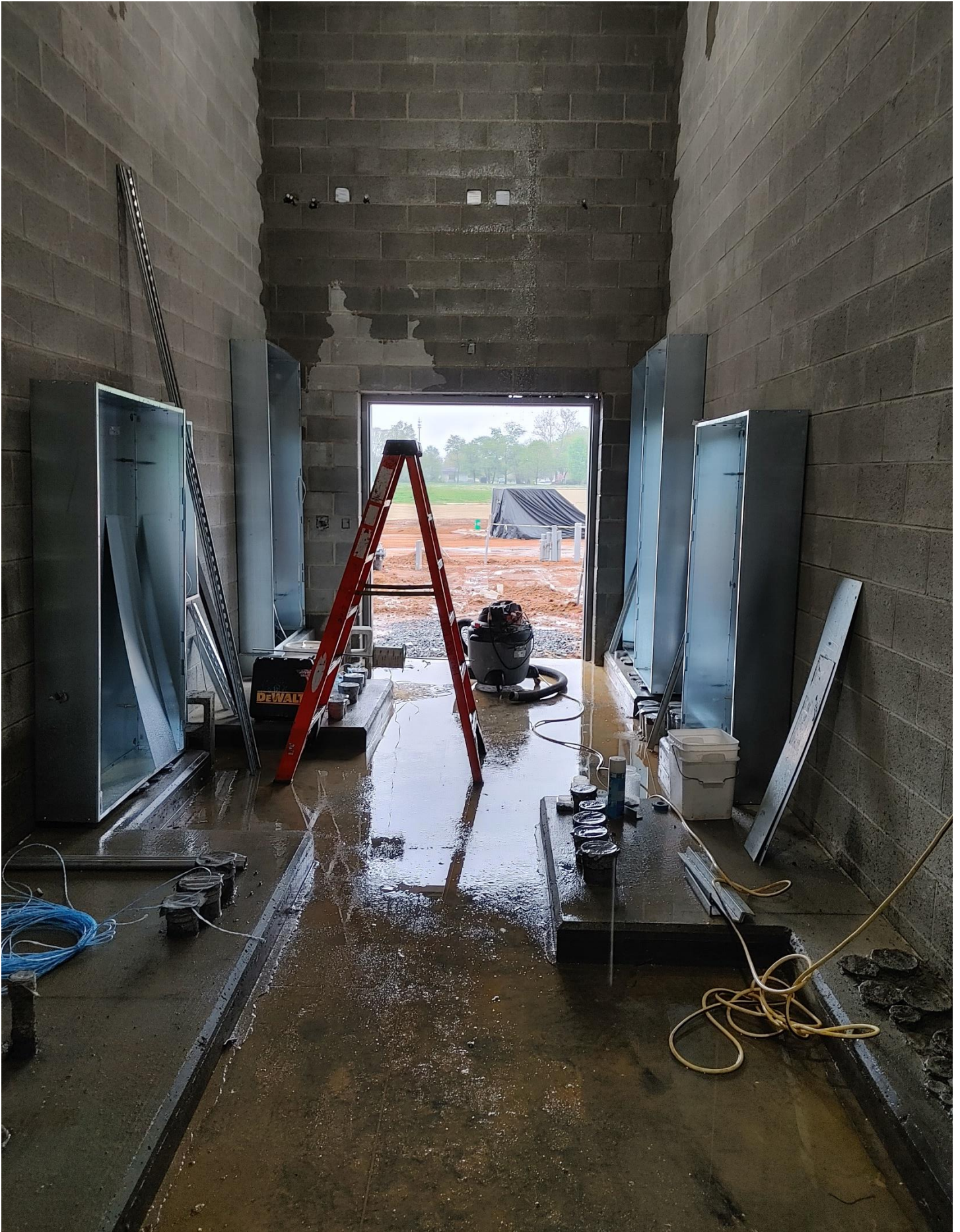
Photo 6 - Electricians are setting their boxes in Electrical Room D158, Area D
