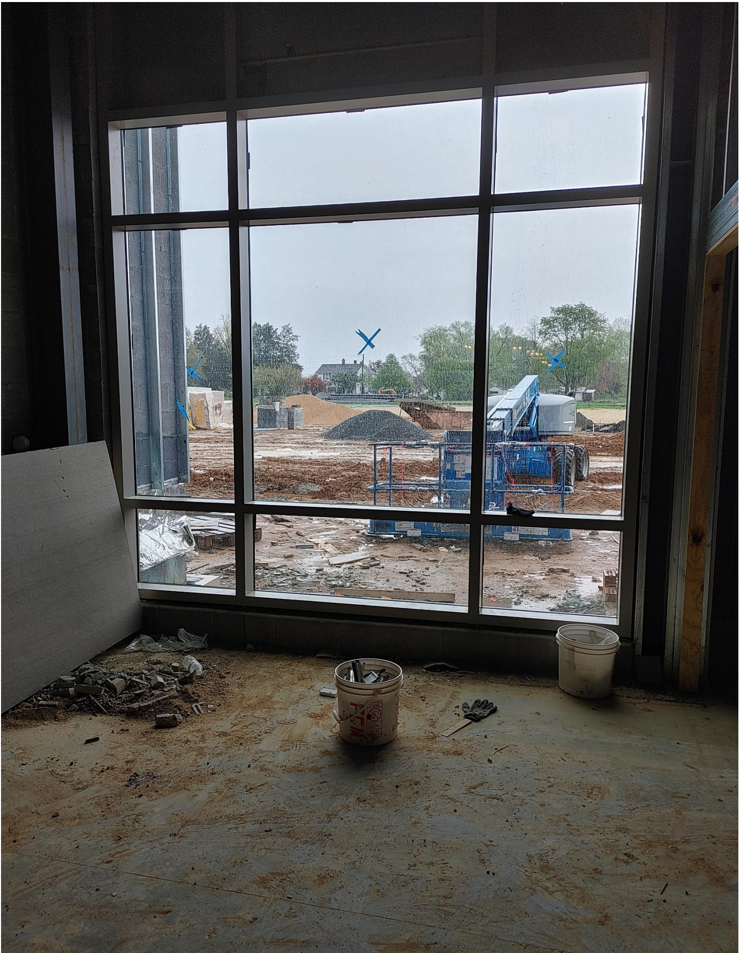
Photo 3 - Glass installed on the Eastside of Area A
