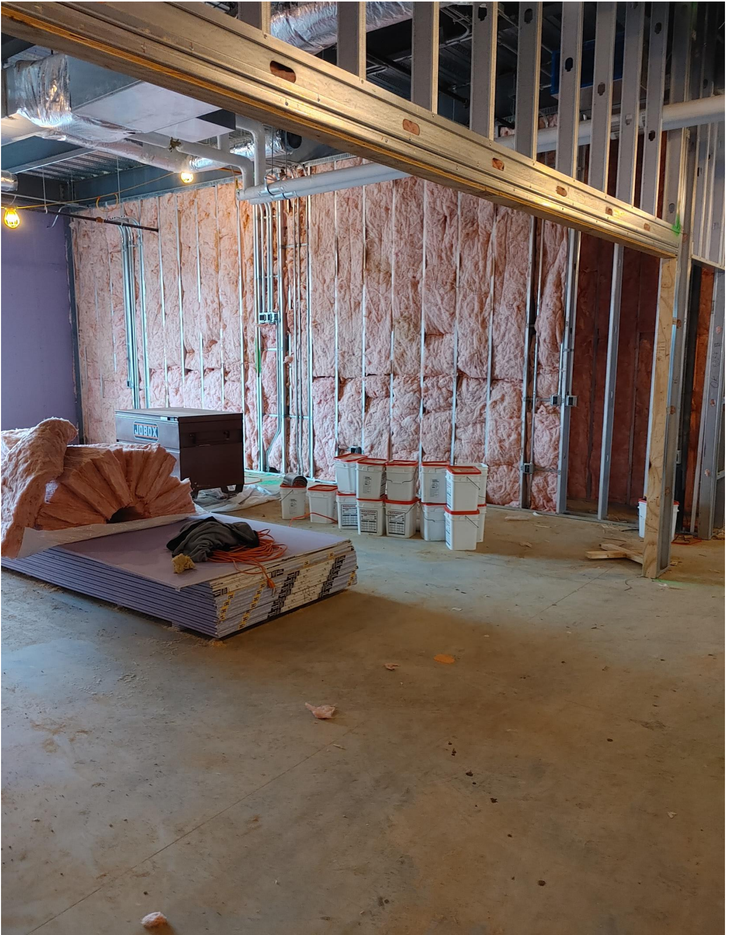
Photo 1 - Batt Insulation is being installed in Area A
