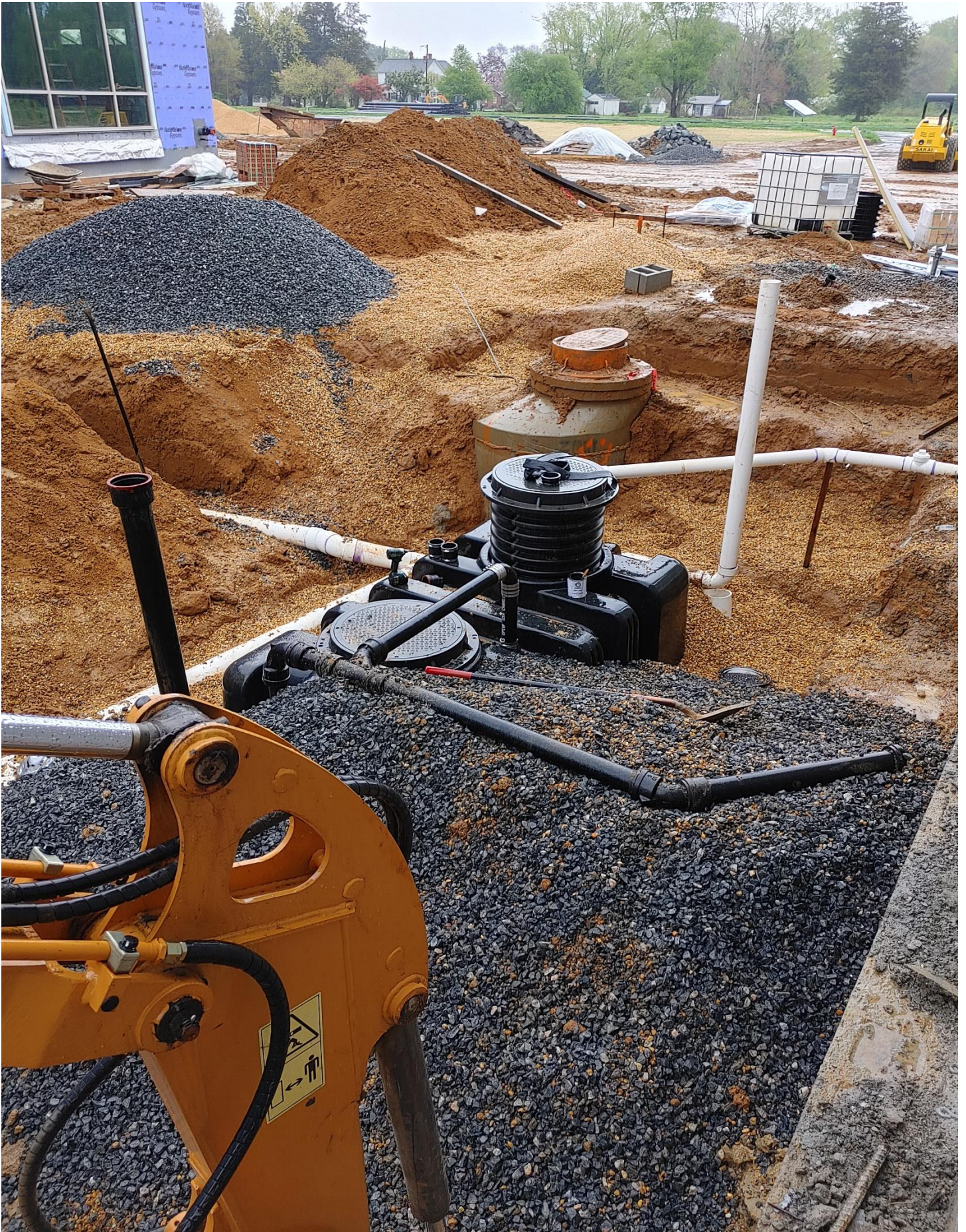
Photo 5 - Progress is being made on the Grease Trap
