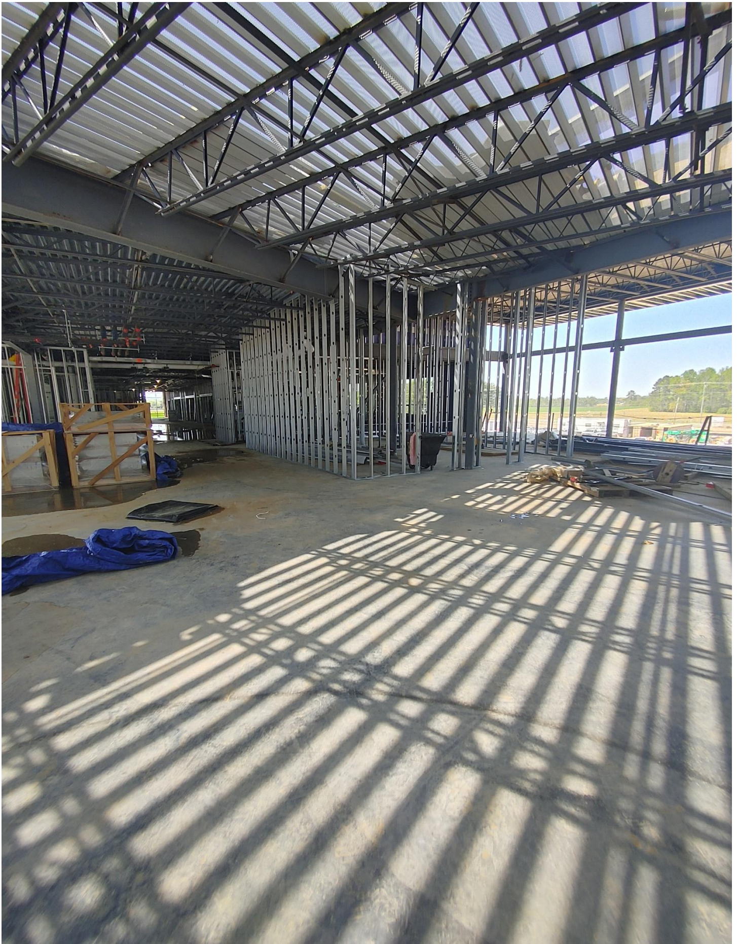
Photo 7 - Interior walls being framed on the 2nd Floor or Area A
