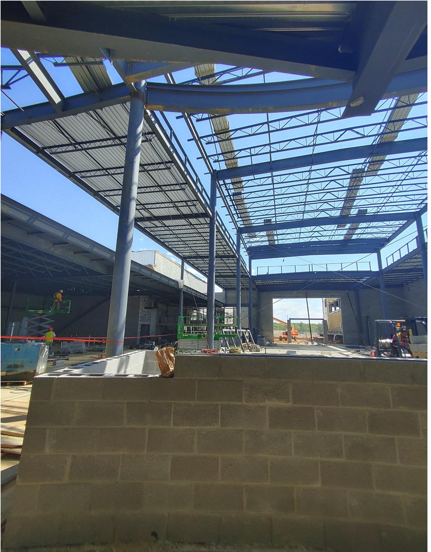
Photo 5 - Metal Decking is being laid in Area C
