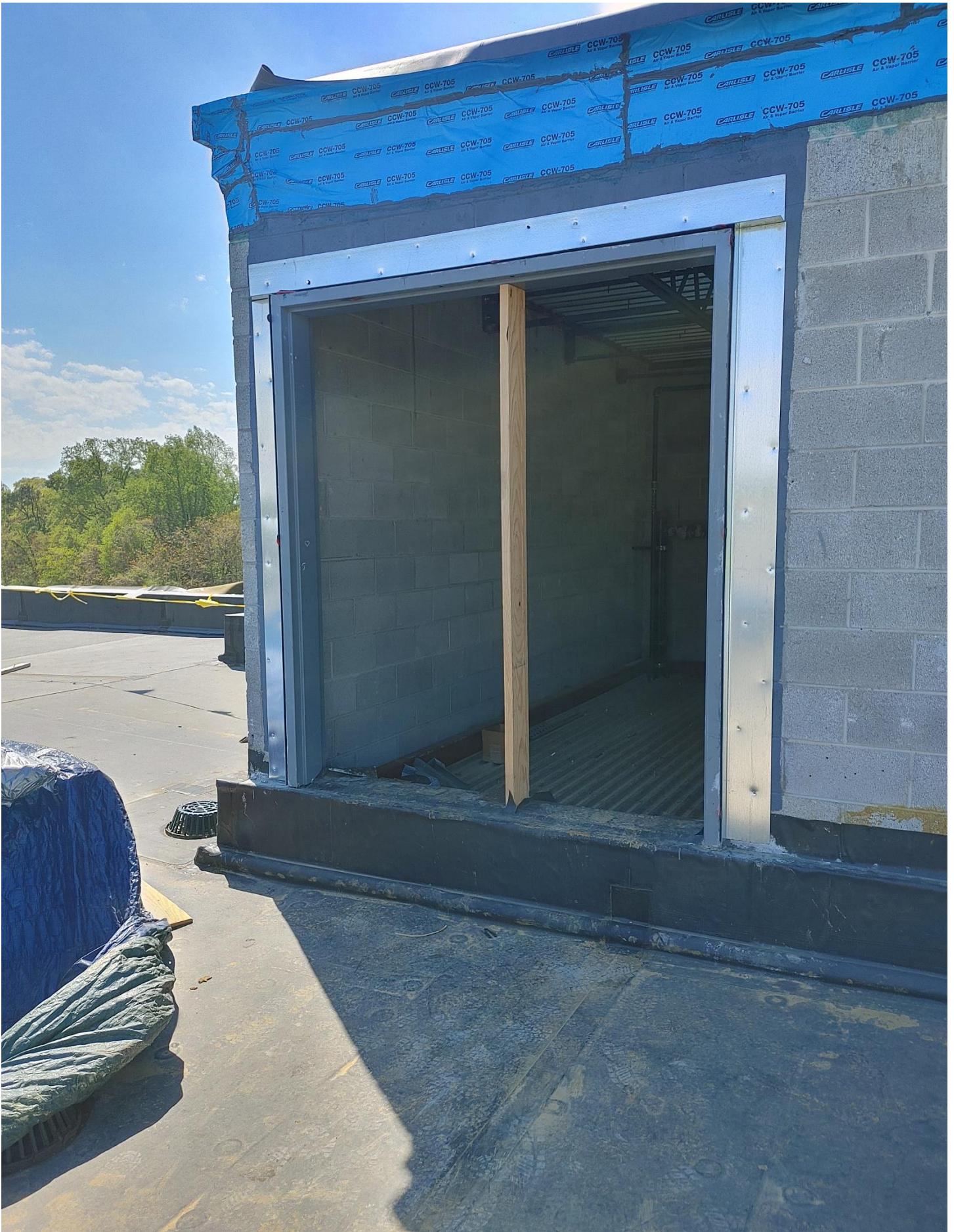
Photo 10 - Door Frame has been set at the top of Stairwell #2.
