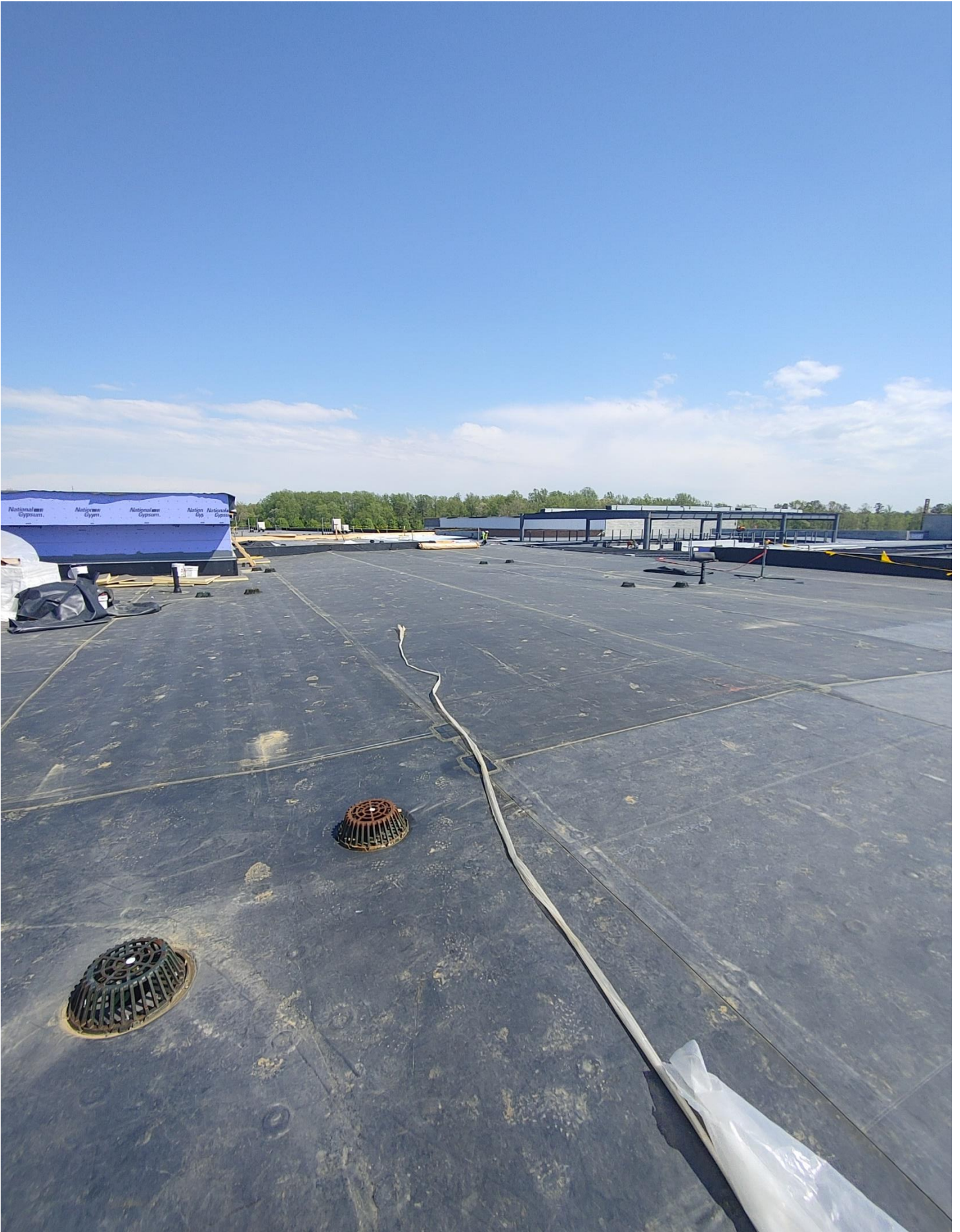
Photo 8 - Roofers are making progress on the Roof of Area A
