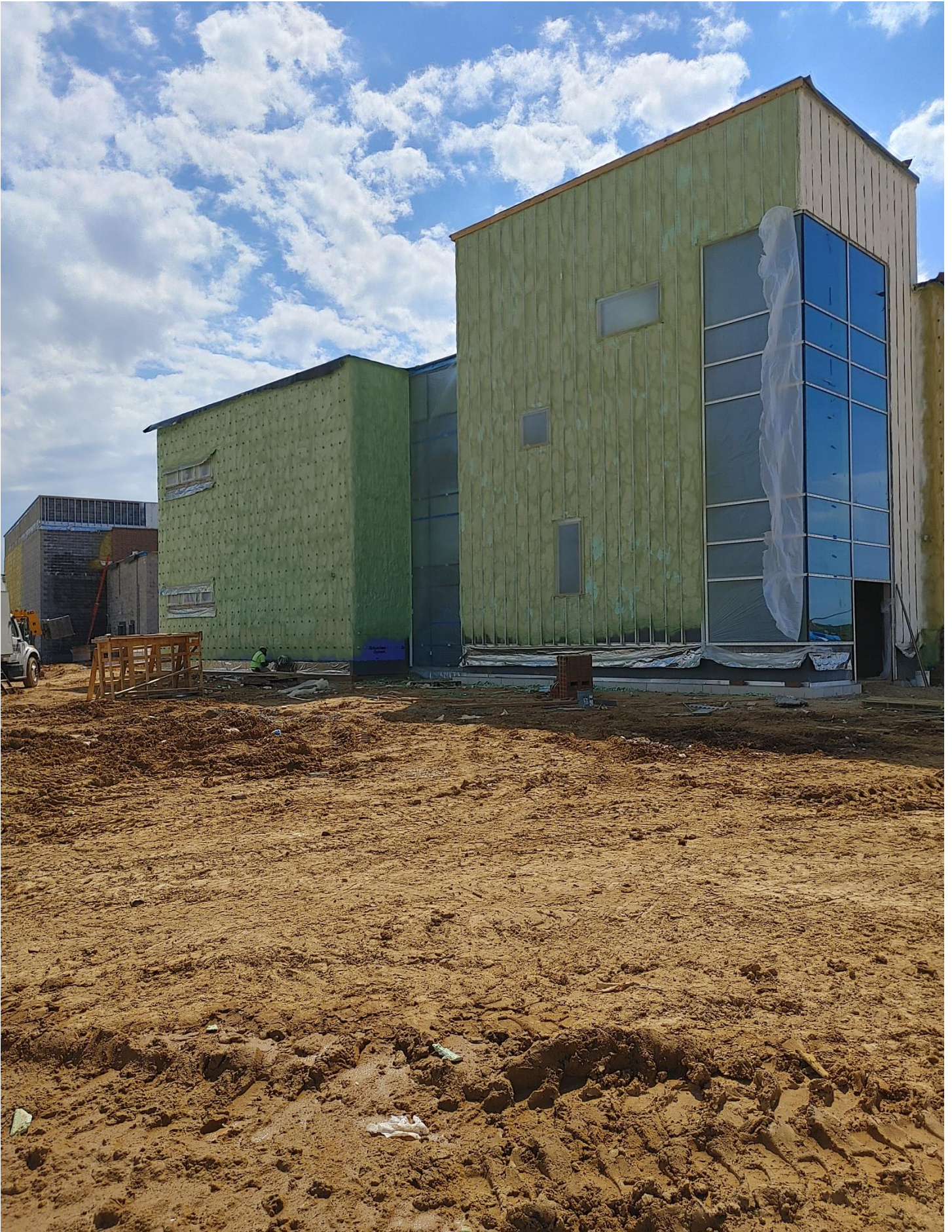
Photo 2 - The East side of Area A has been foamed.
