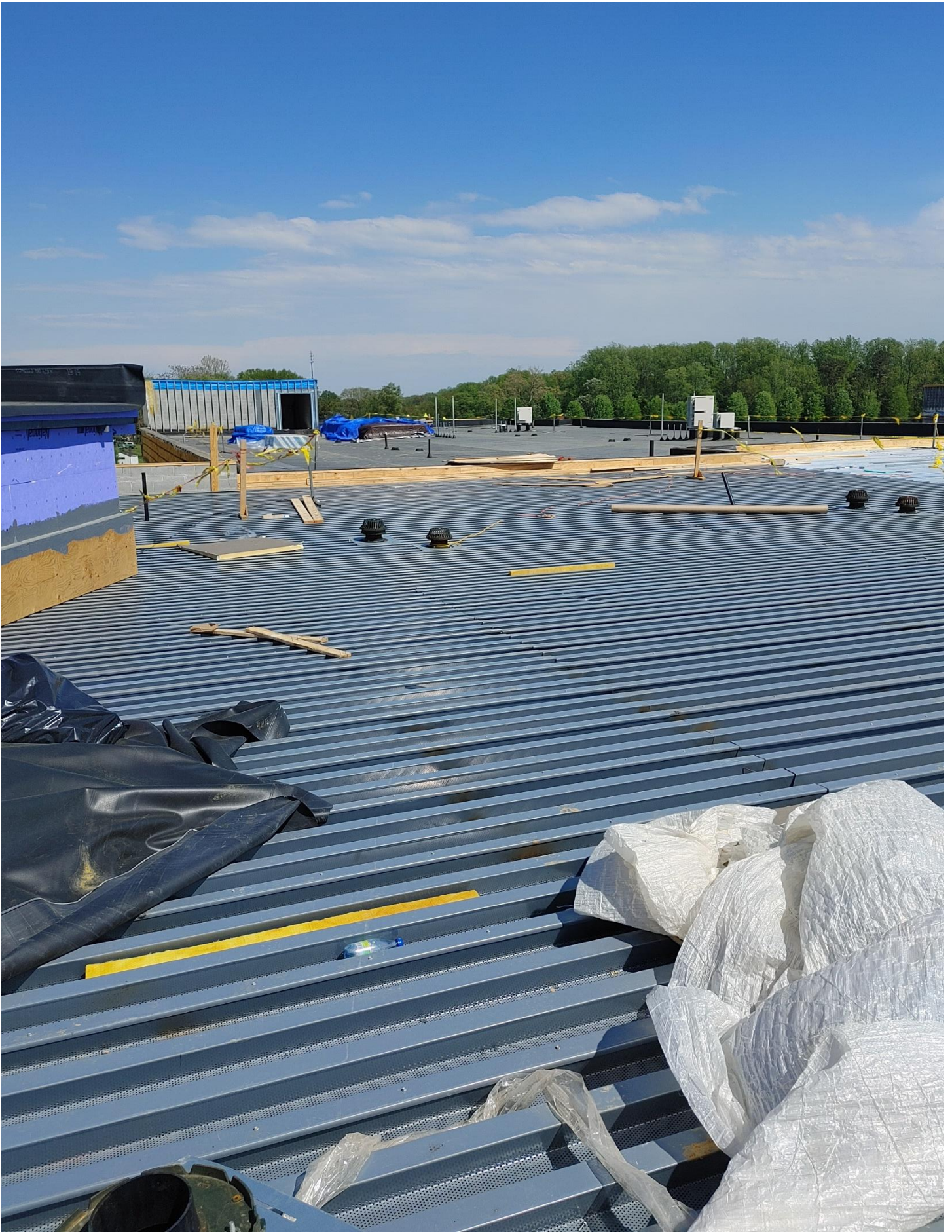
Photo 9 - Parapet Wall being framed in Area A
