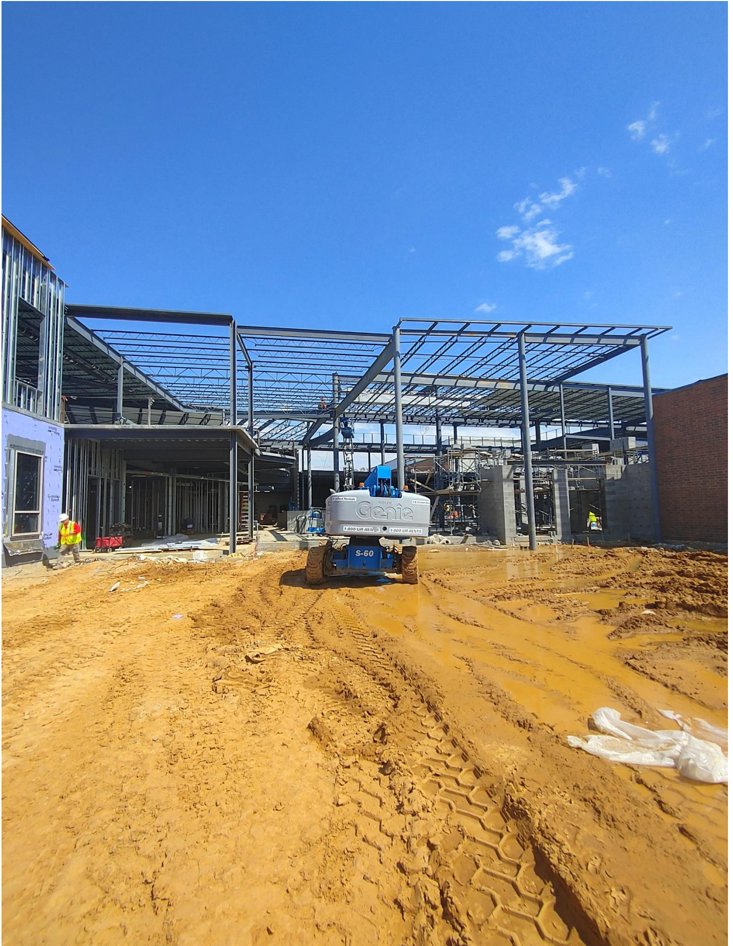
Photo 4 - Steel continues to be set in Area C
