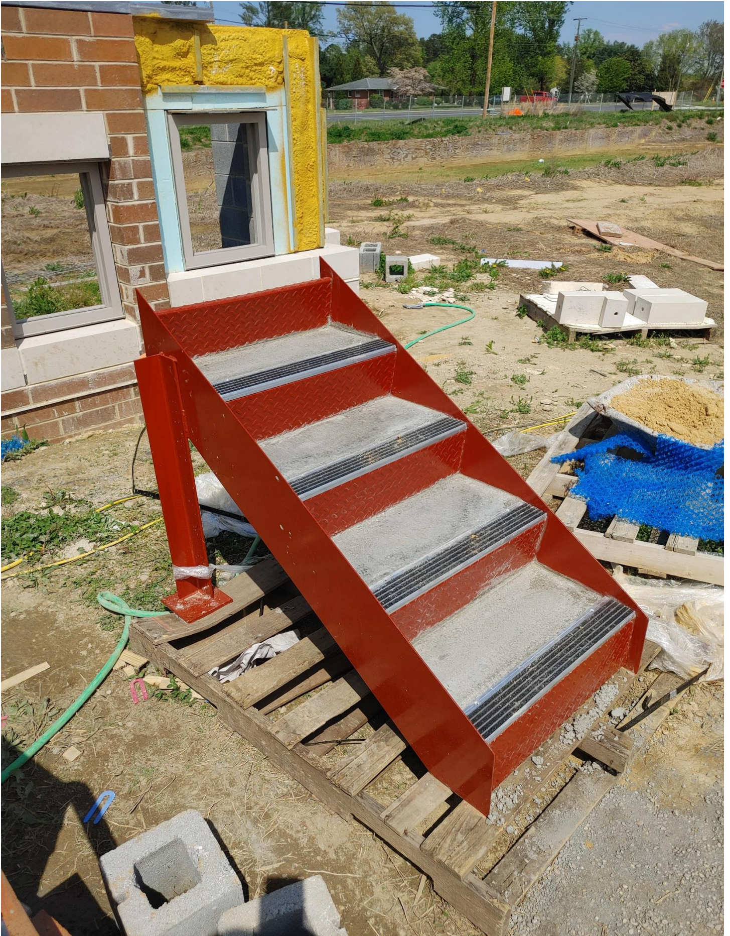
Photo 1 – Stair tread Mockup has been completed.
