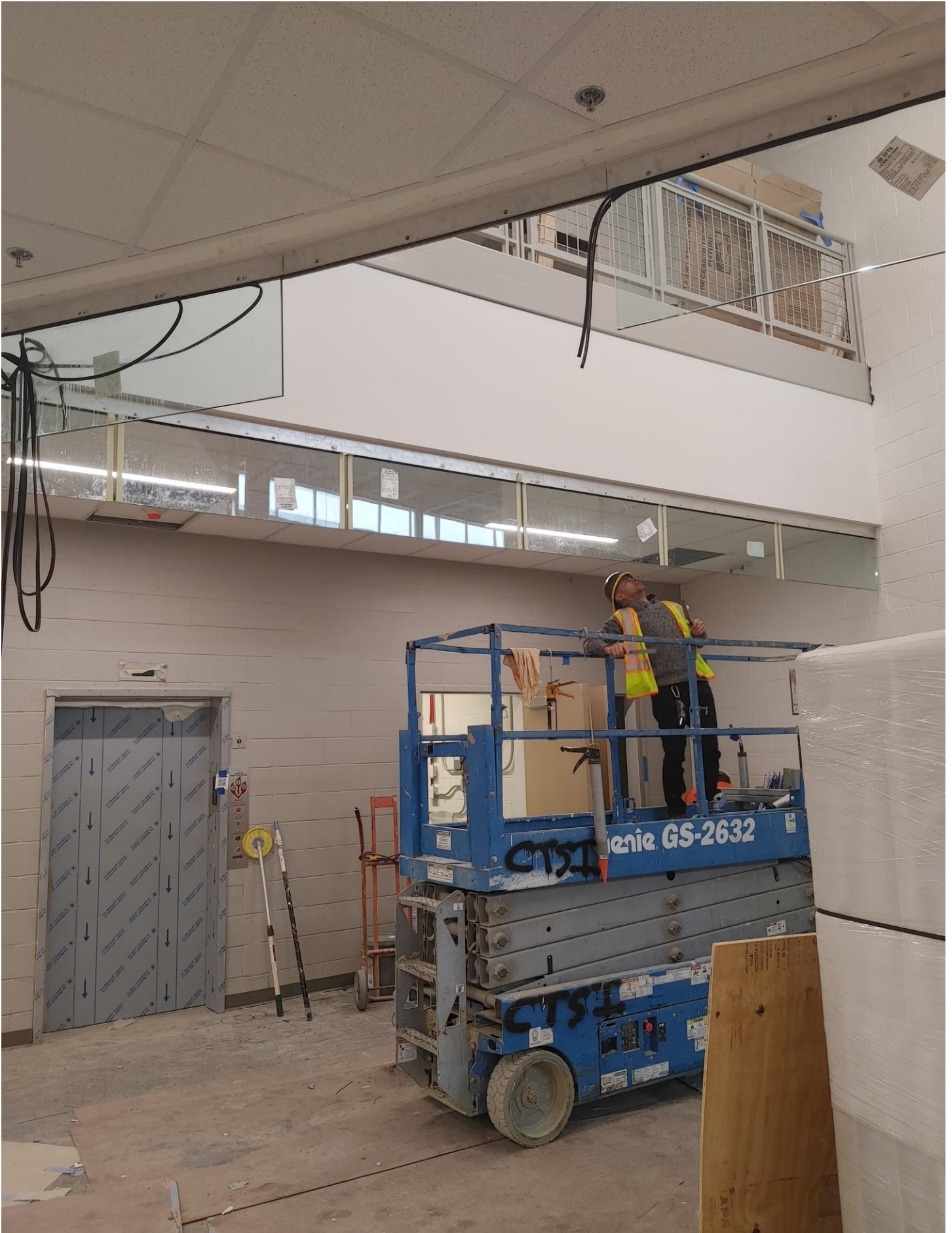
Photo 7 - Curtain Wall Glass is being installed in Area C
