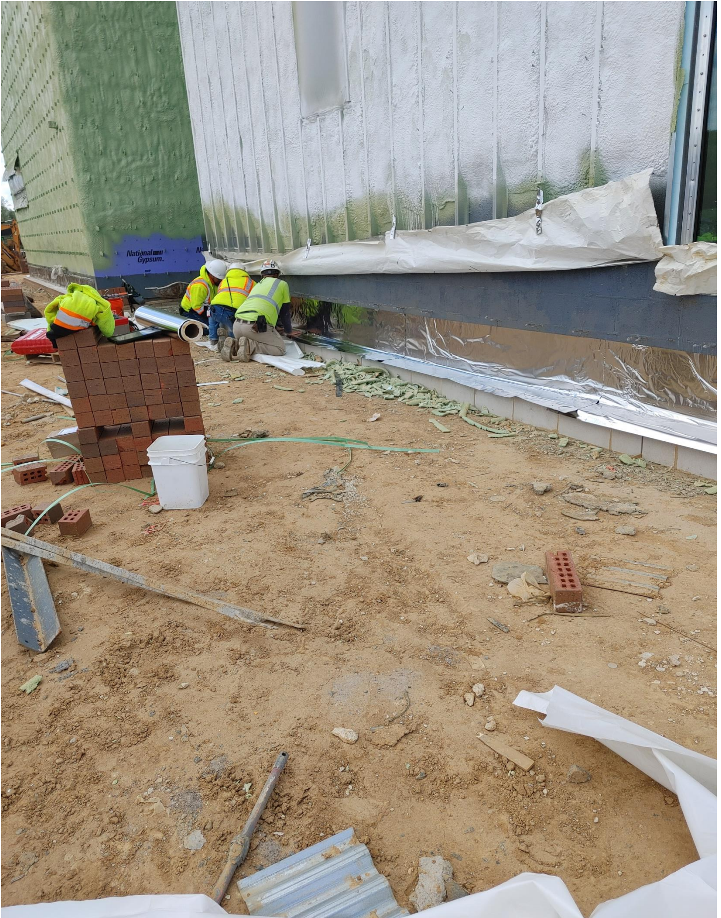
Photo 3 - Flashing being installed on the East side of Area A
