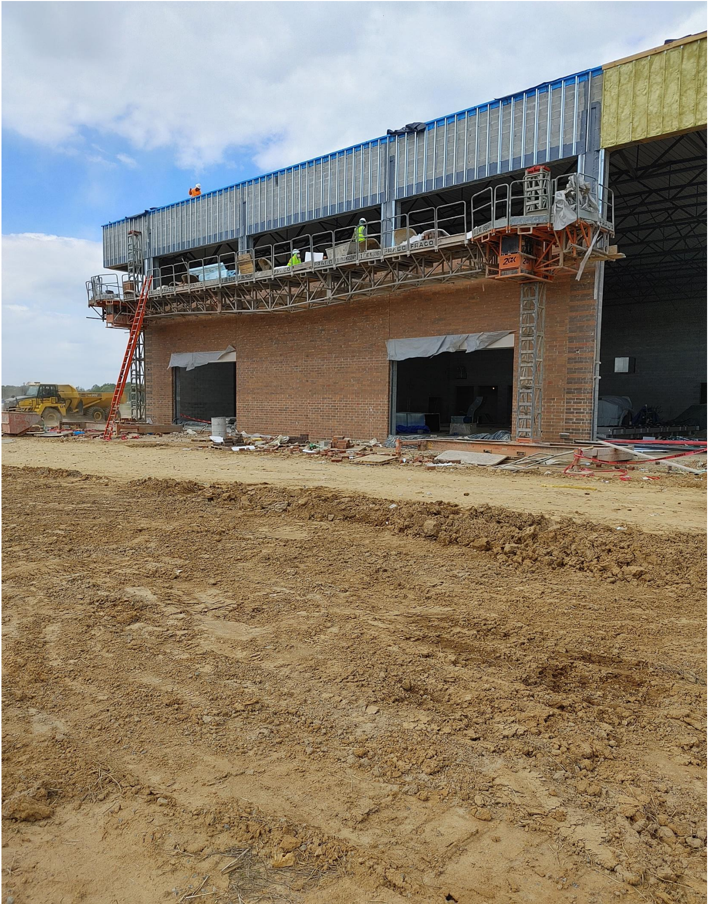
Photo 11 - Brick is being laid on the South side of the Gym
