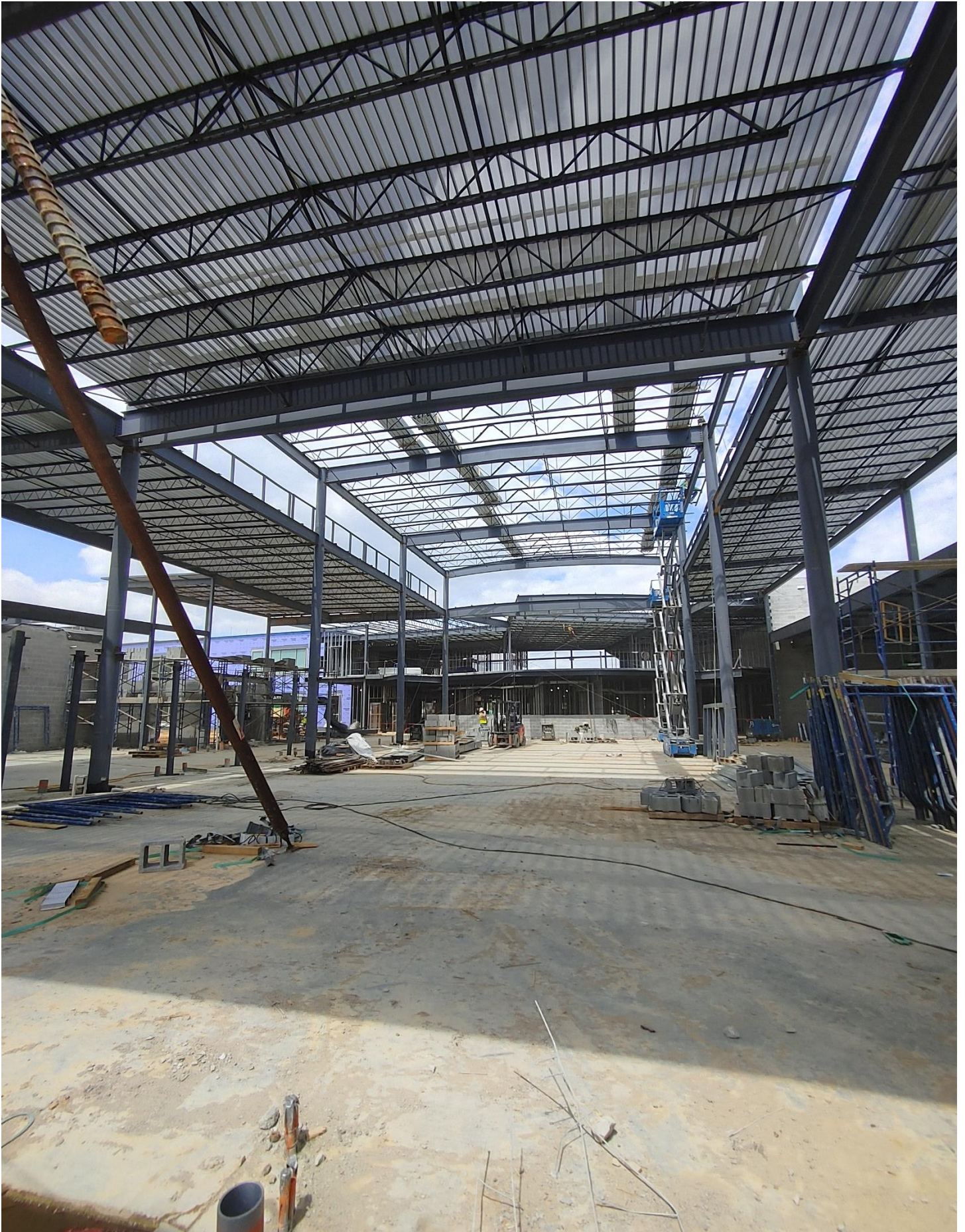
Photo 9 - Metal Decking continues to be laid in Area C.
