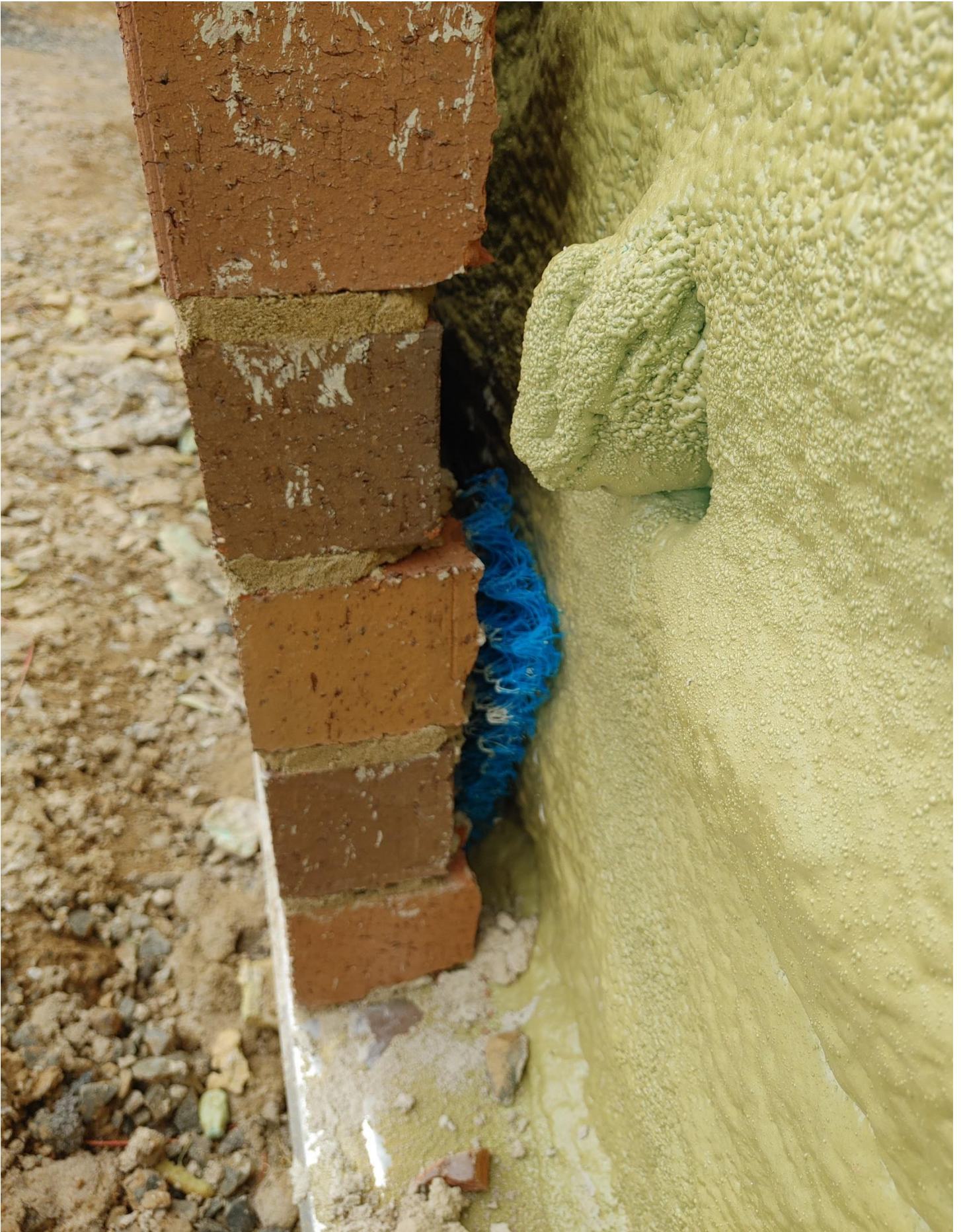
Photo 1 - Verification that Mortar Screen is being used on the Northside of Area A
