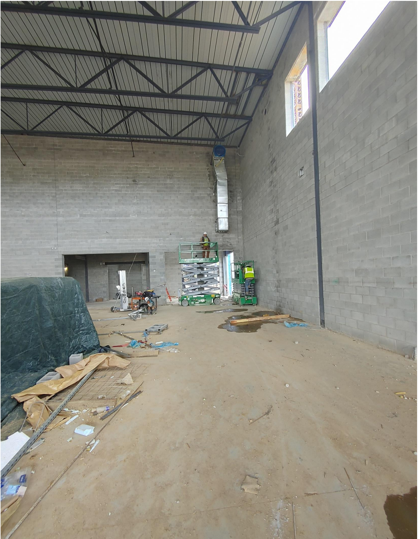
Photo 10 - Colonial Webb has begun to run HVAC Duct in the Gym
