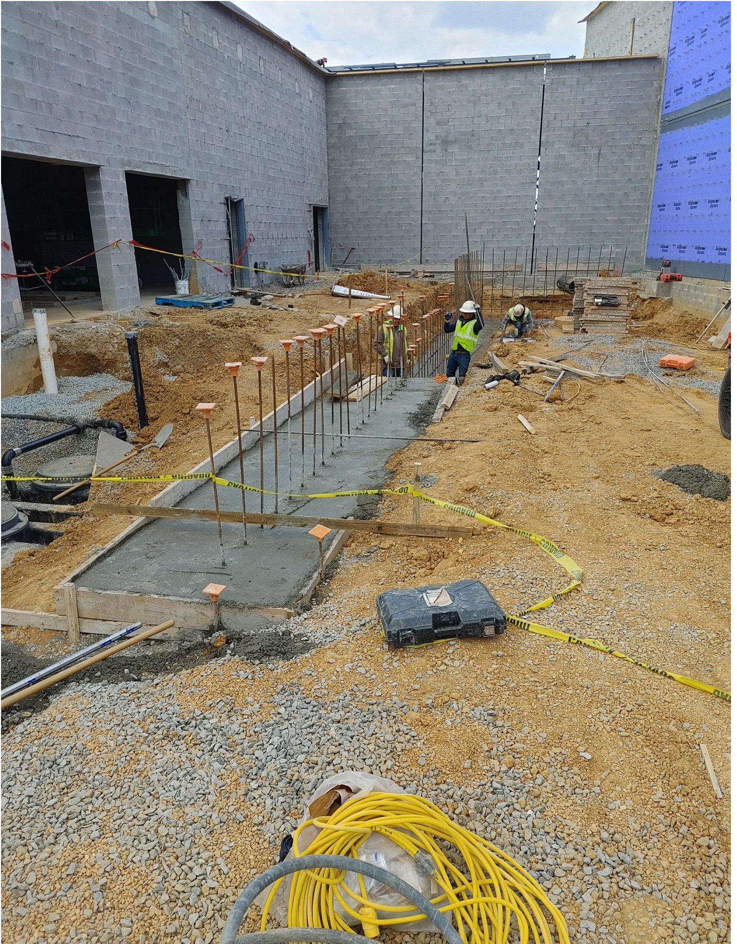
Photo 4 - Concrete Footer poured for Loading Dock Wall
