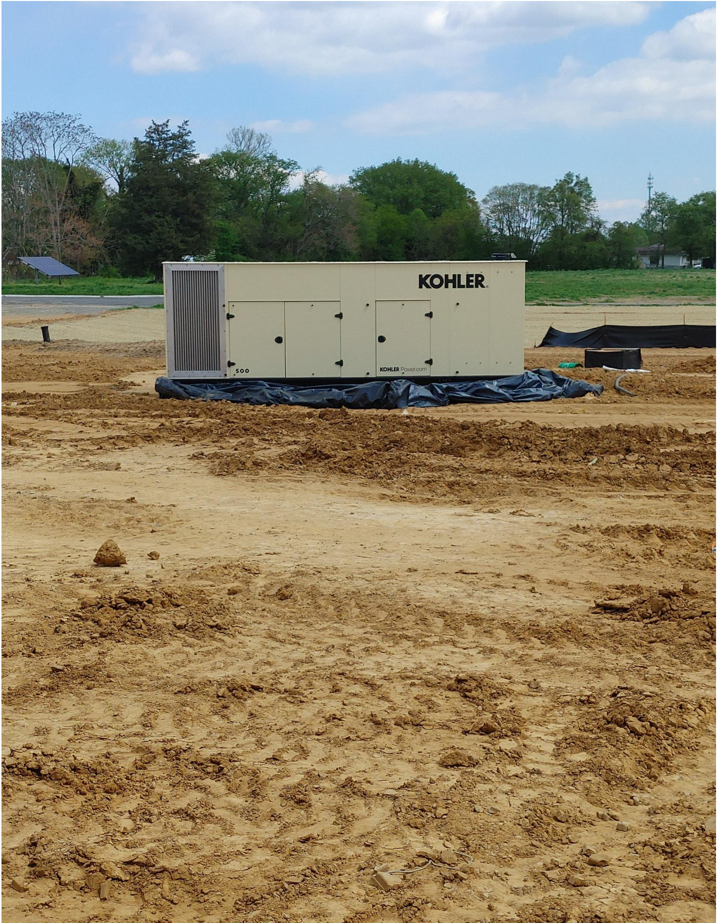
Photo 6 - Generator has been delivered.
