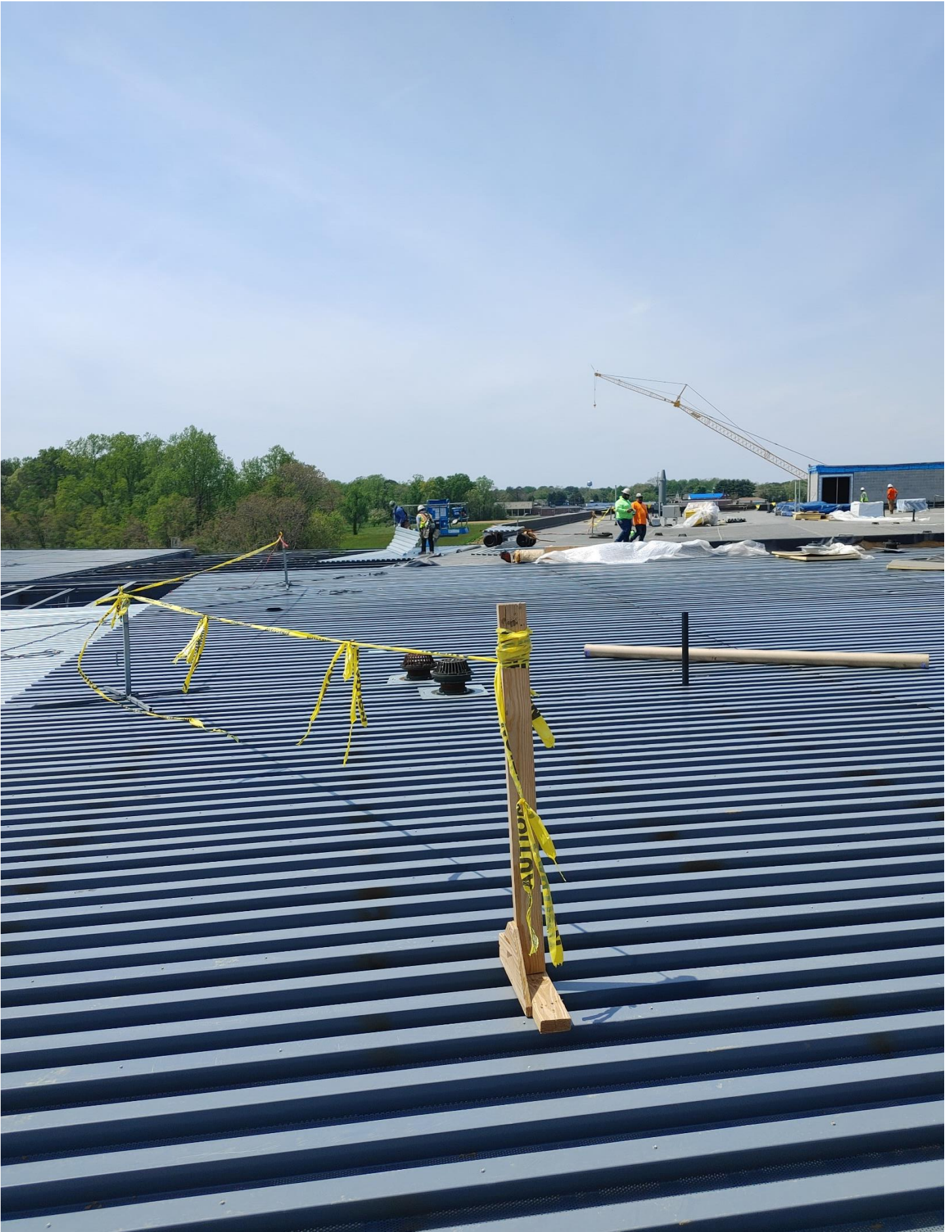
Photo 12 - Metal Decking is being laid between Areas A & C.
