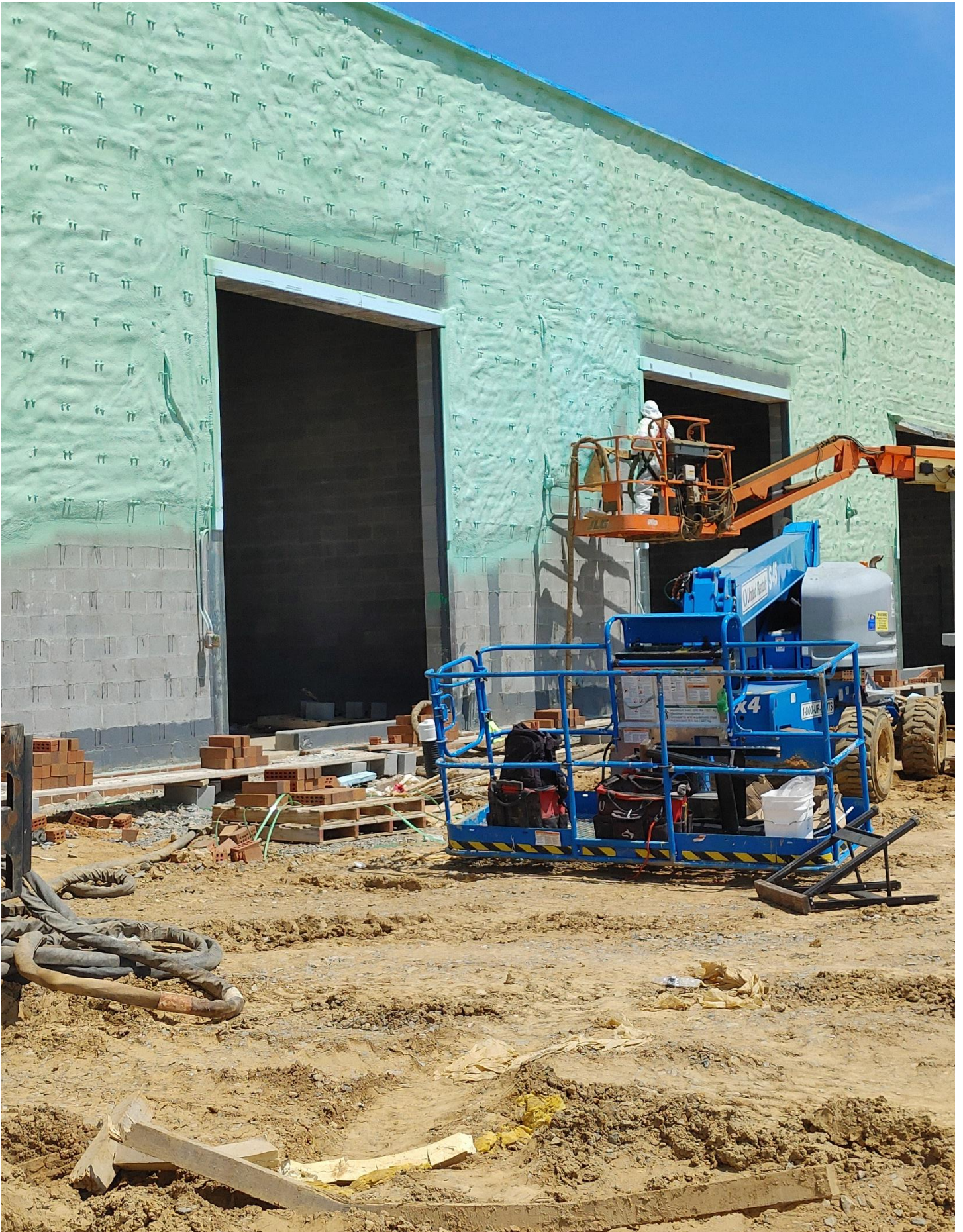
Photo 2 - South side of Area D is being Spray Foamed
