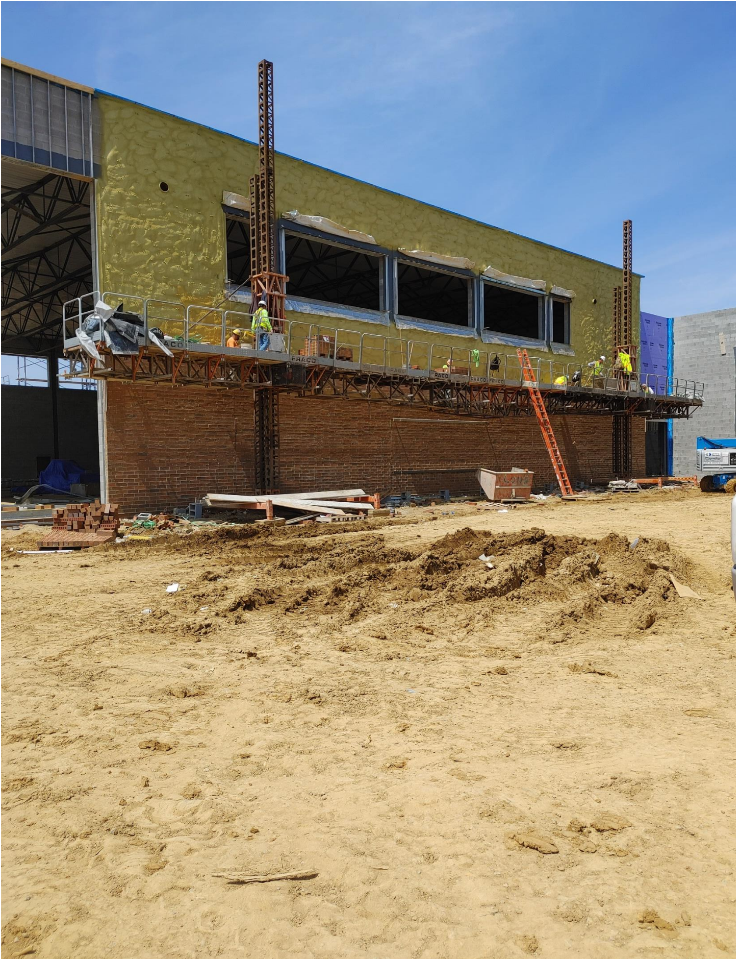
Photo 3 - The Masons continue to lay Brick on the East side of Gym.
