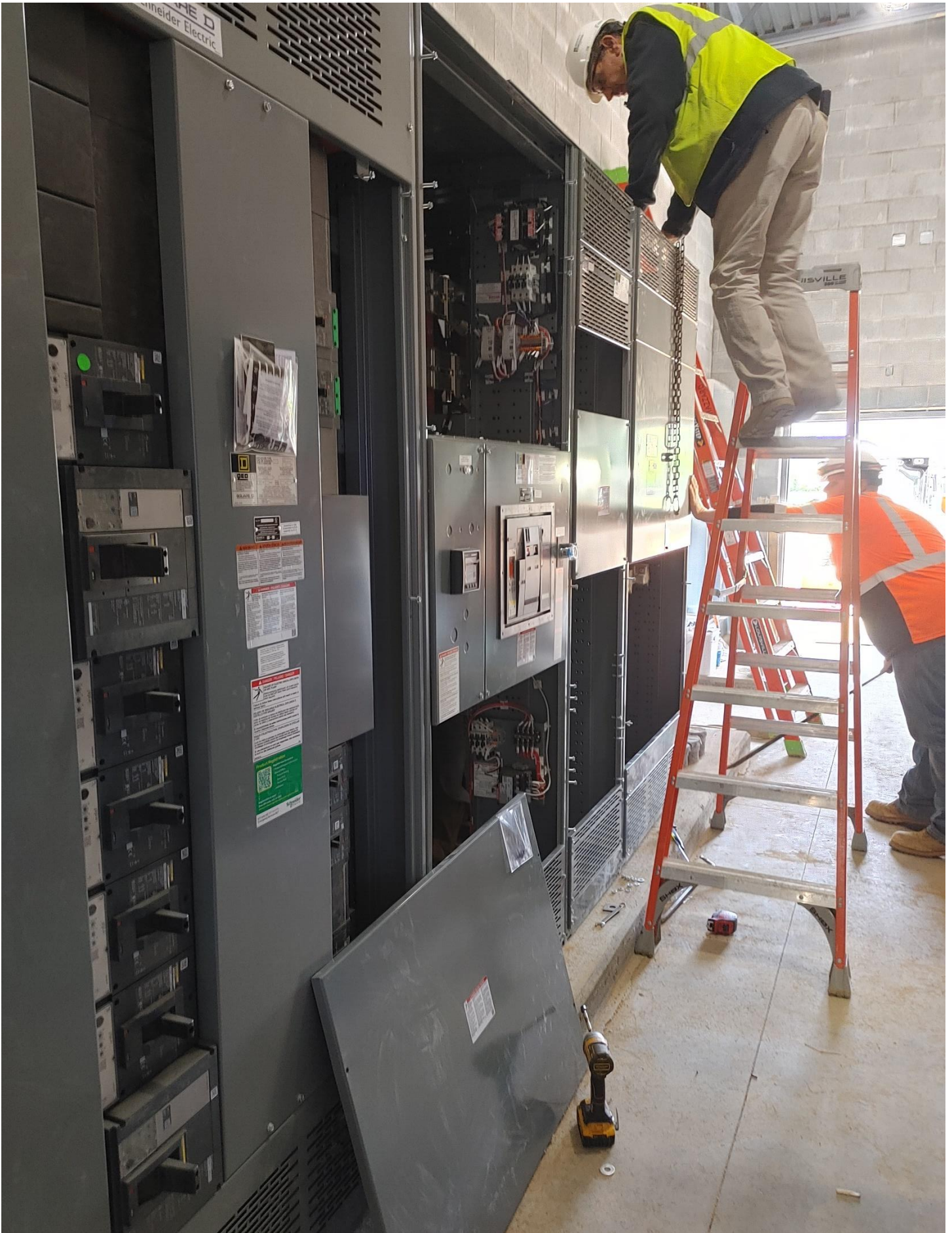
Photo 5 - The Electricians have set several more Switch Gears since yesterday.
