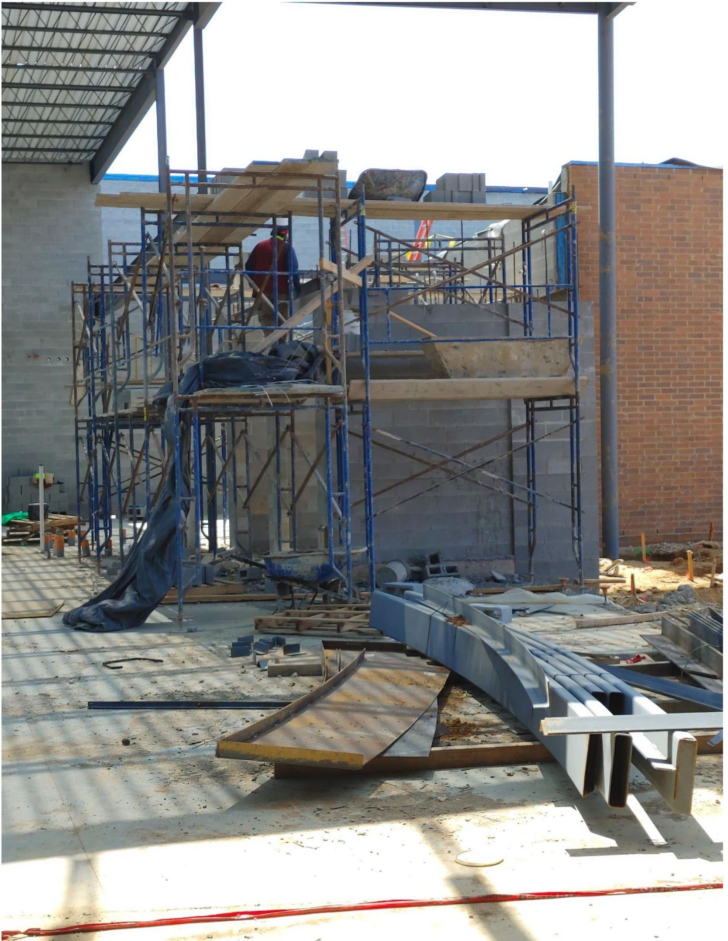
Photo 10 - Masons are laying block in Vestibule C10
