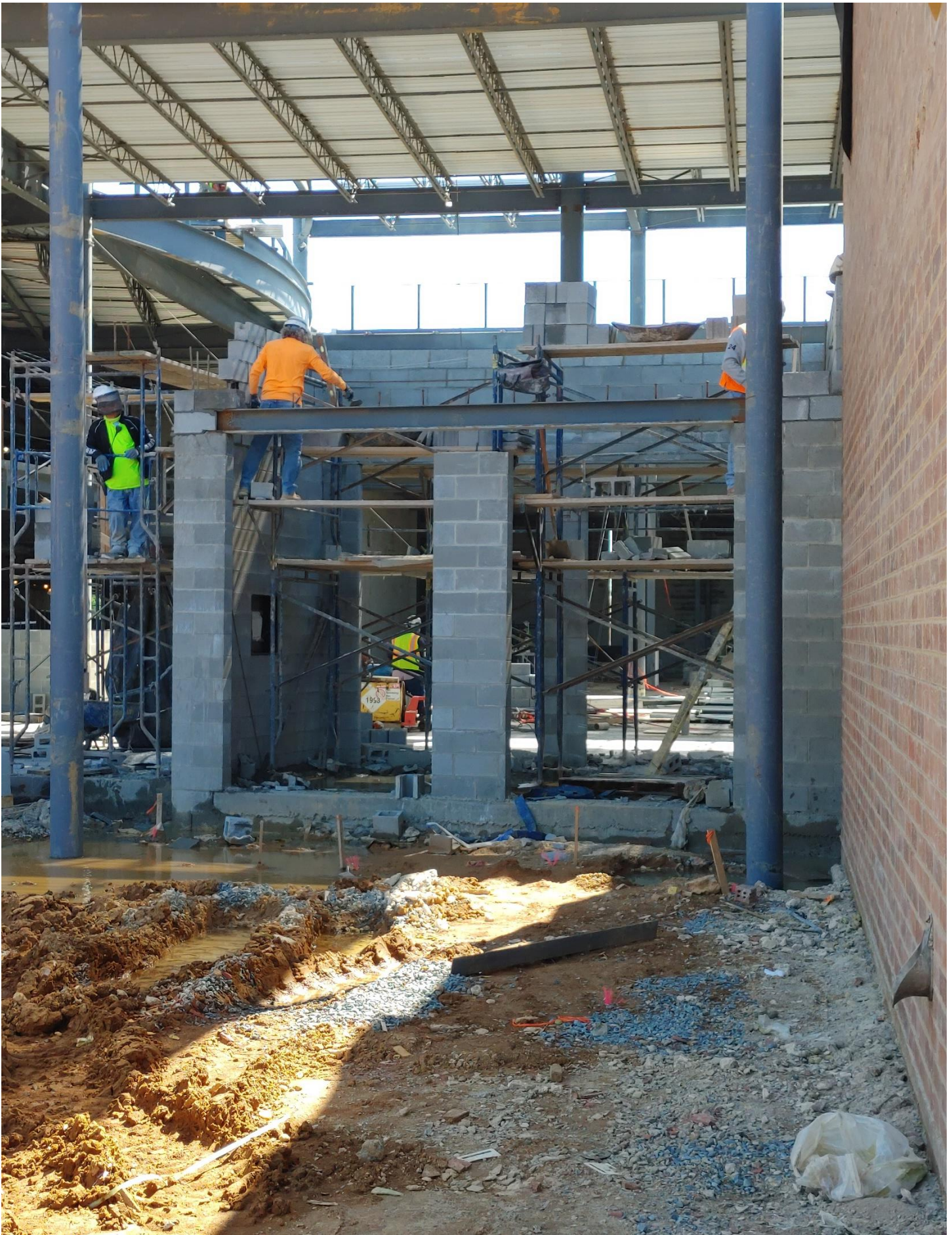
Photo 6 - J. D. Long laying block in Vestibule c10, Area C.
