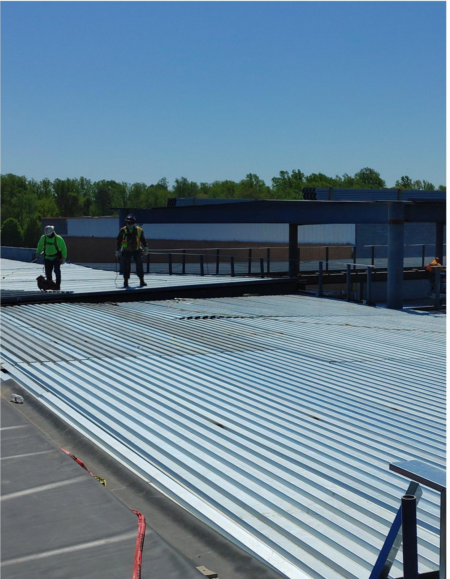
Photo 8 - Weldon Steel installing metal decking , Area A
