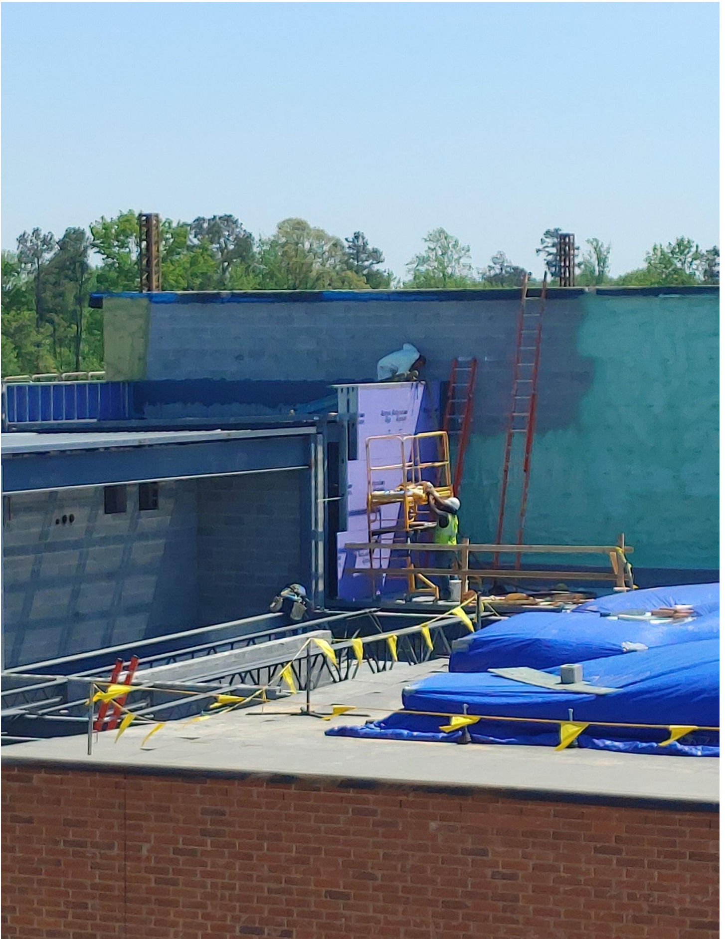
Photo 10 - Area E high wall on the North side being foamed.
