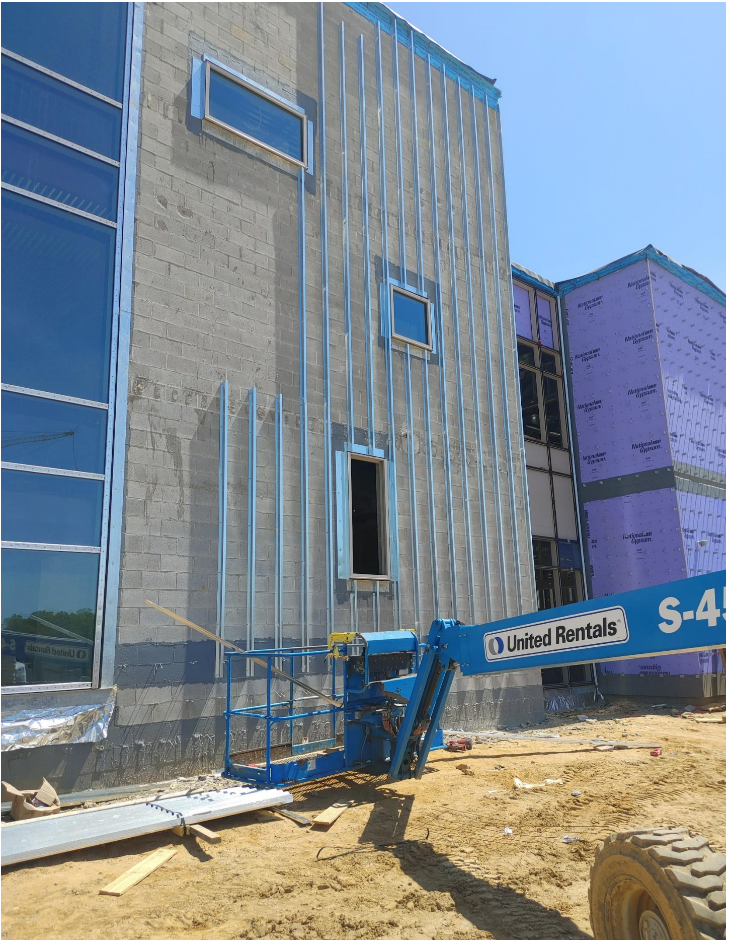
Photo 7 - Stairwell #2 being framed for panels.
