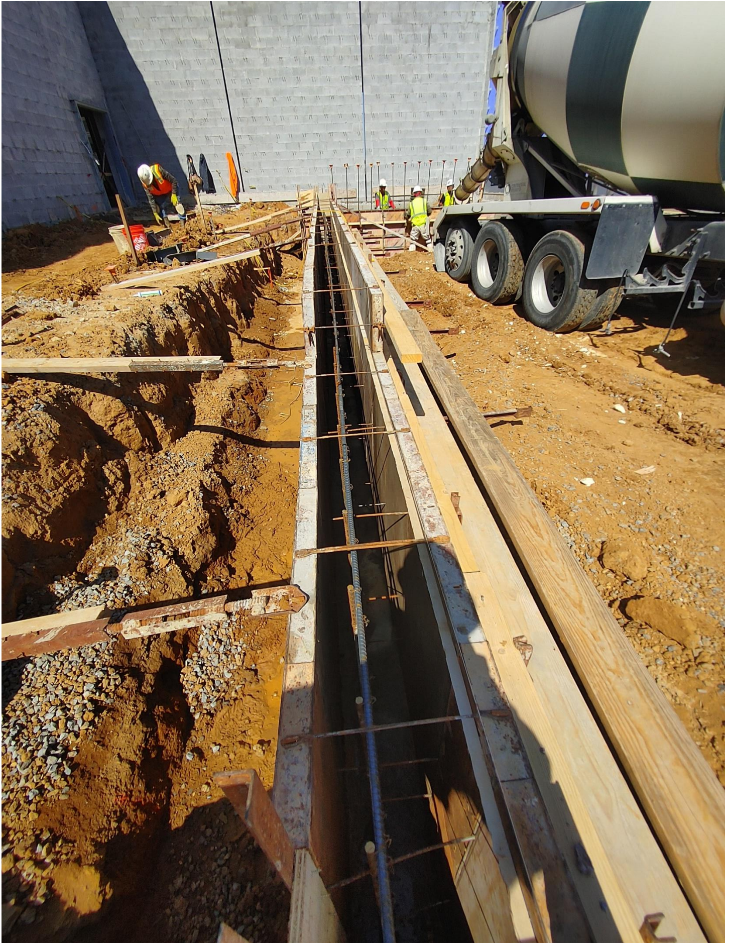
Photo 4 - Verification of Rebar in Loading Dock Wall
