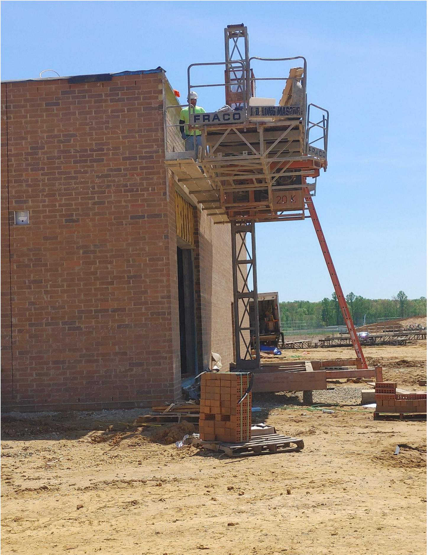
Photo 8 - Lintel and Precast set above Storefront SF6
