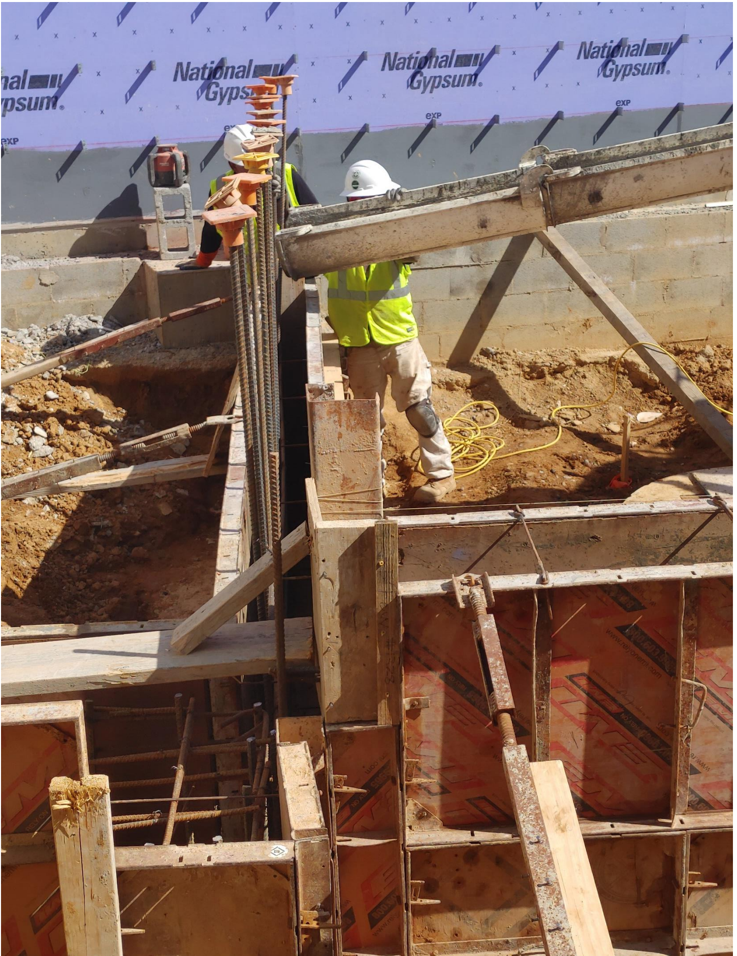
Photo 1 - Preparing to pour the Concrete for the Loading Dock Wall
