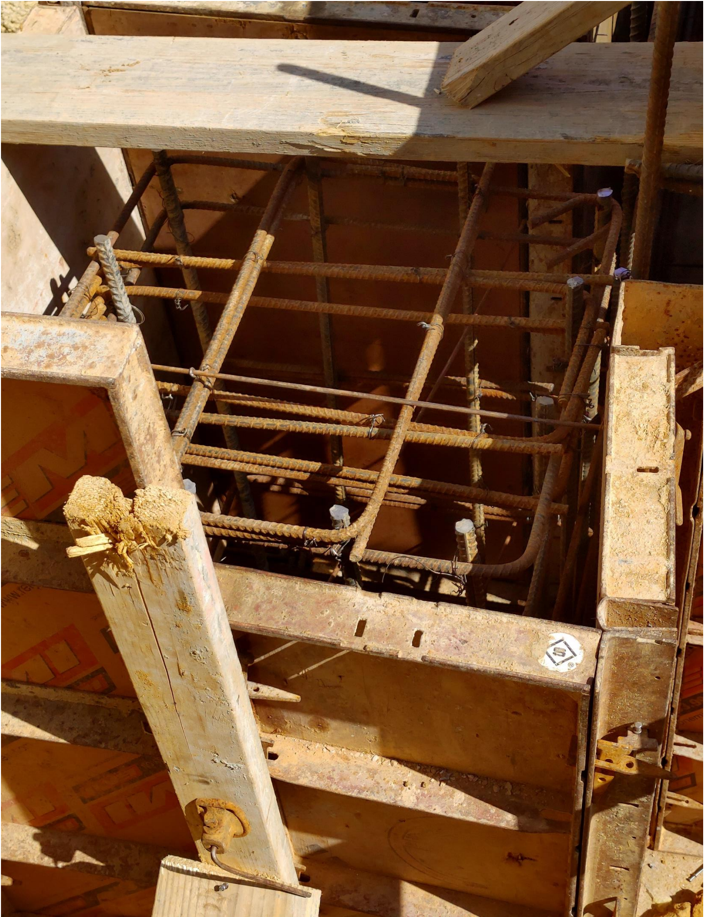
Photo 3 - Rebar cage in corner of Loading Dock Wall
