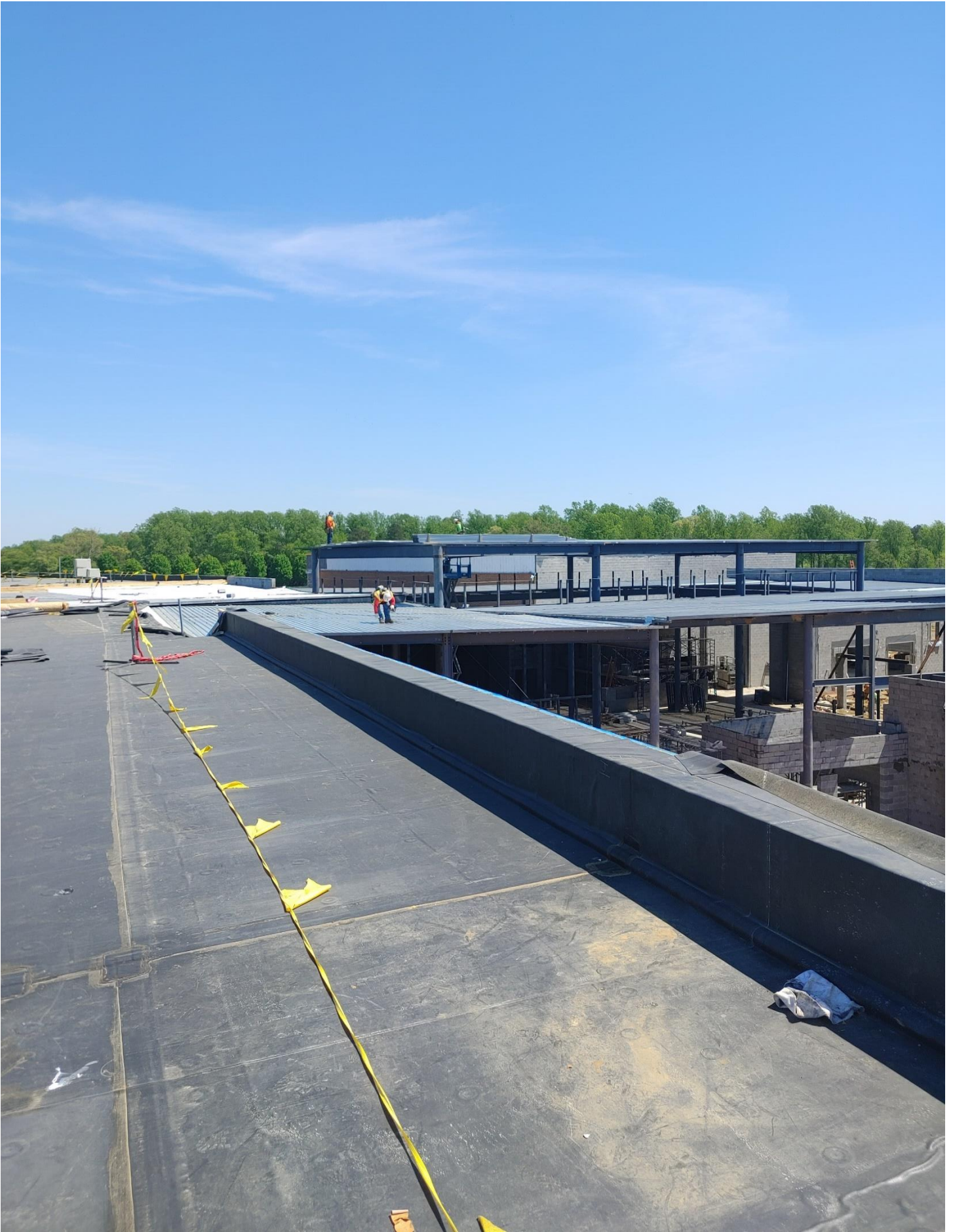
Photo 11 - Metal Decking continues to be laid in Area C
