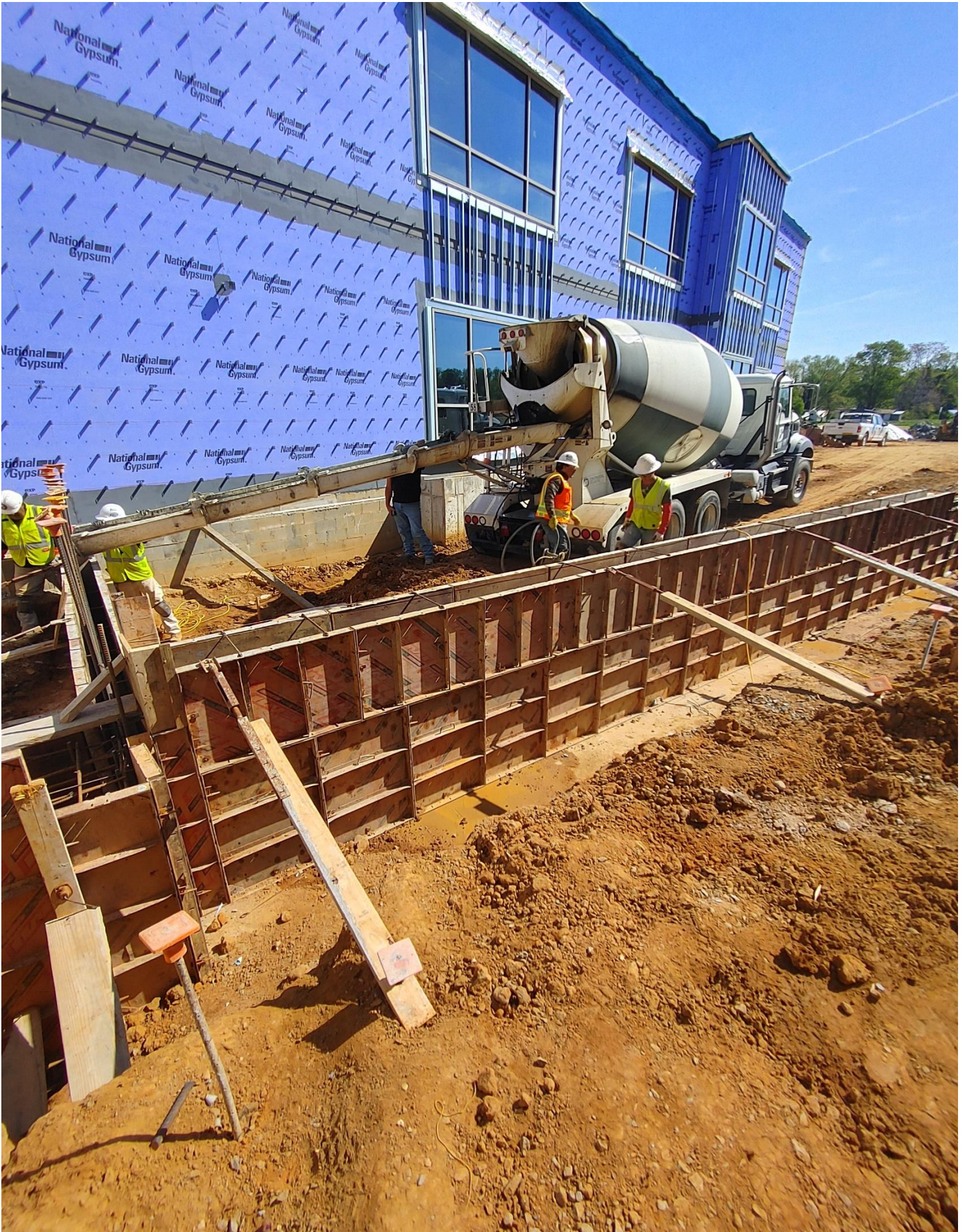
Photo 2 - Loading Dock wall being poured
