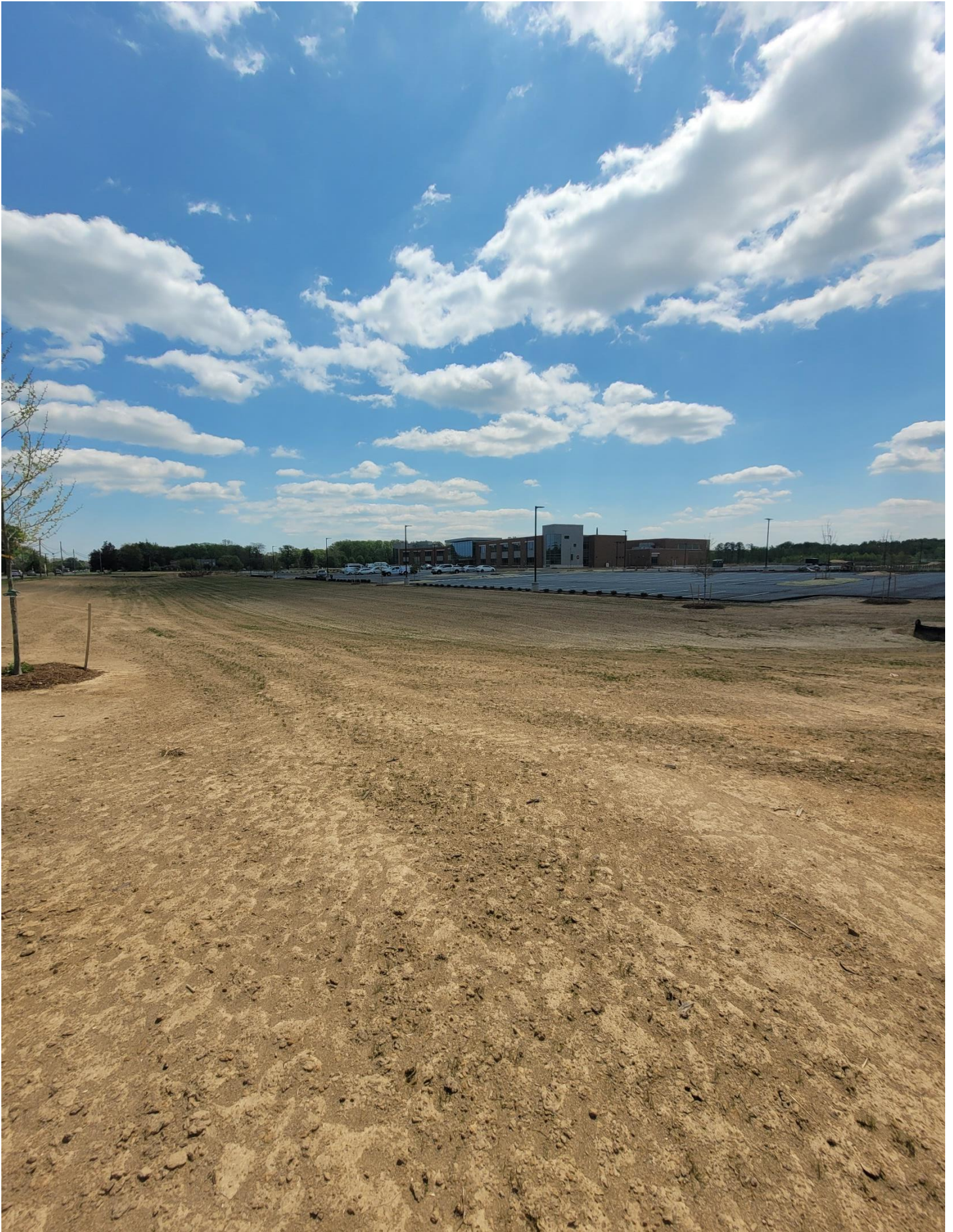
Photo 11 - Grass is starting to come up in Various areas
