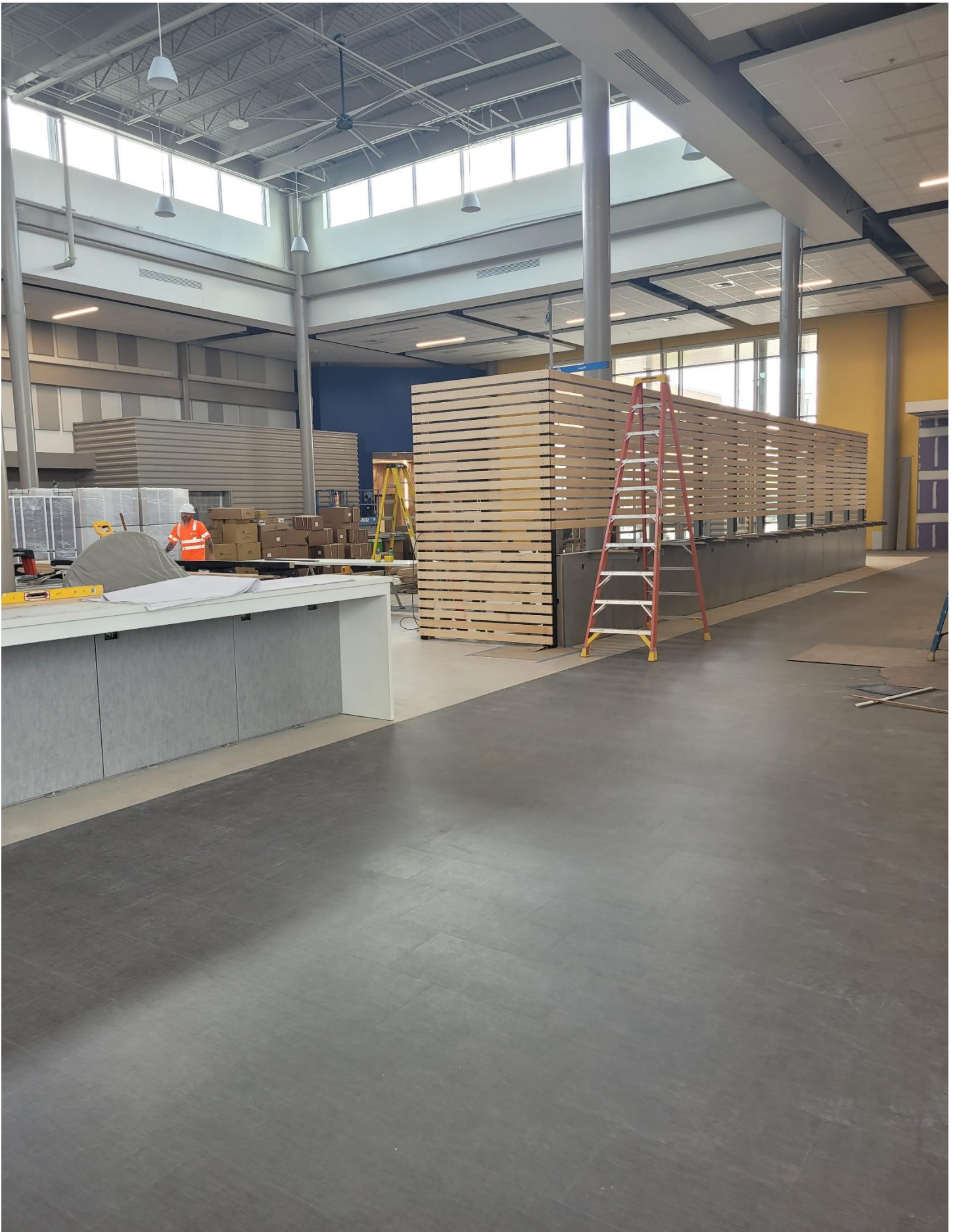
Photo 1 - Decorative Wood wall is being constructed in Area C
