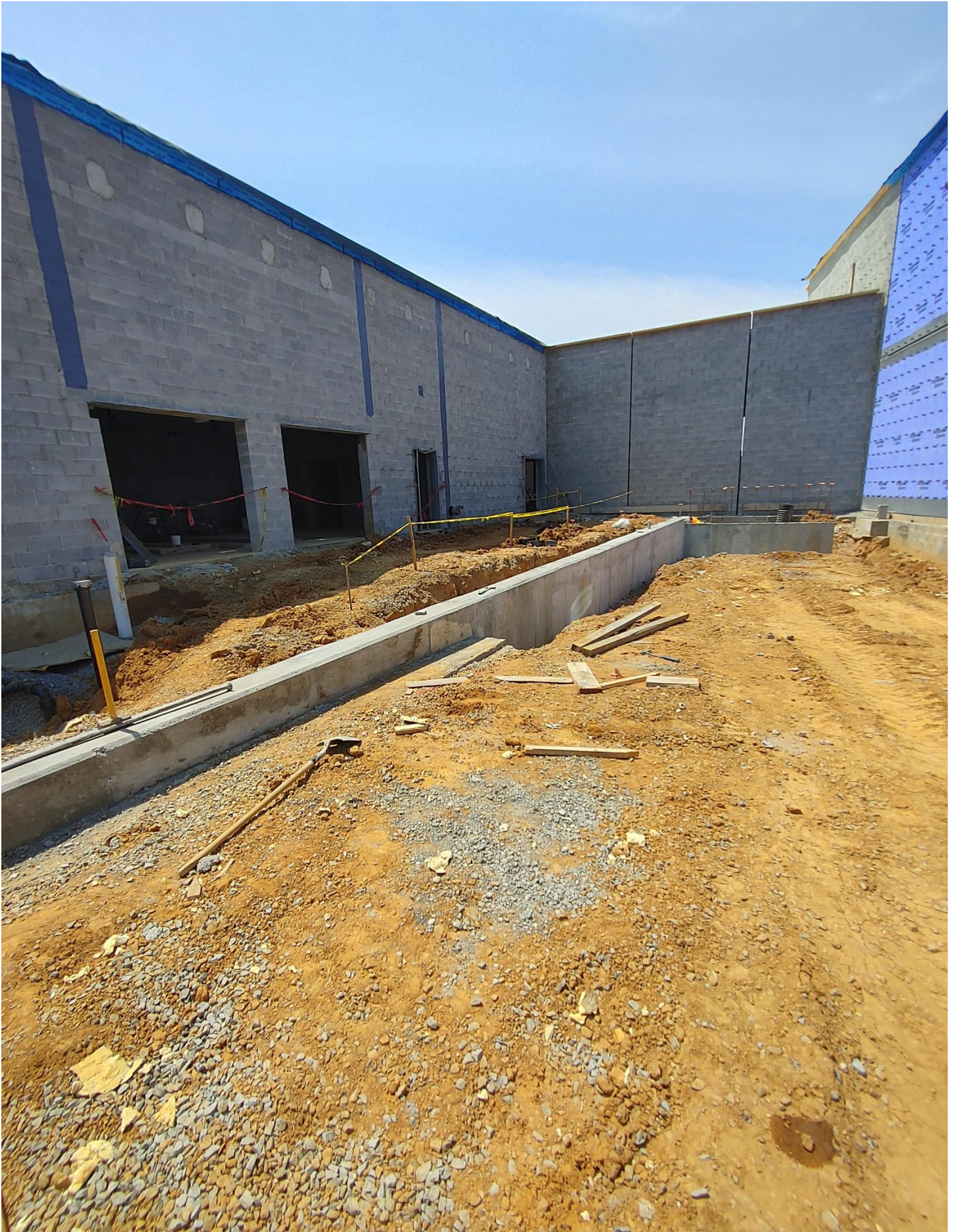
Photo 1 - Forms being stripped from Loading Dock Wall.
