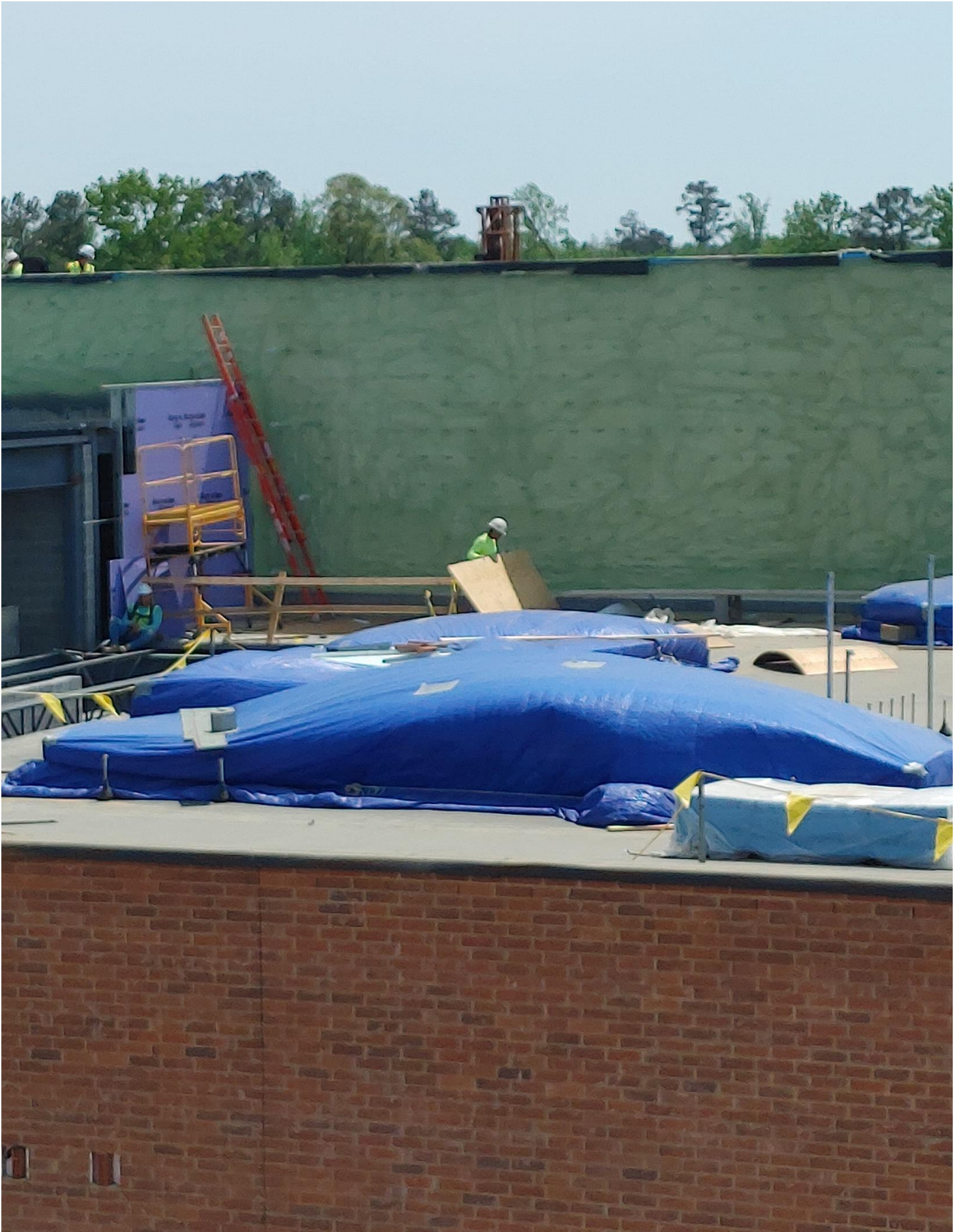
Photo 7 - Roof being protected with Poly and Plywood prior to Mason starting.
