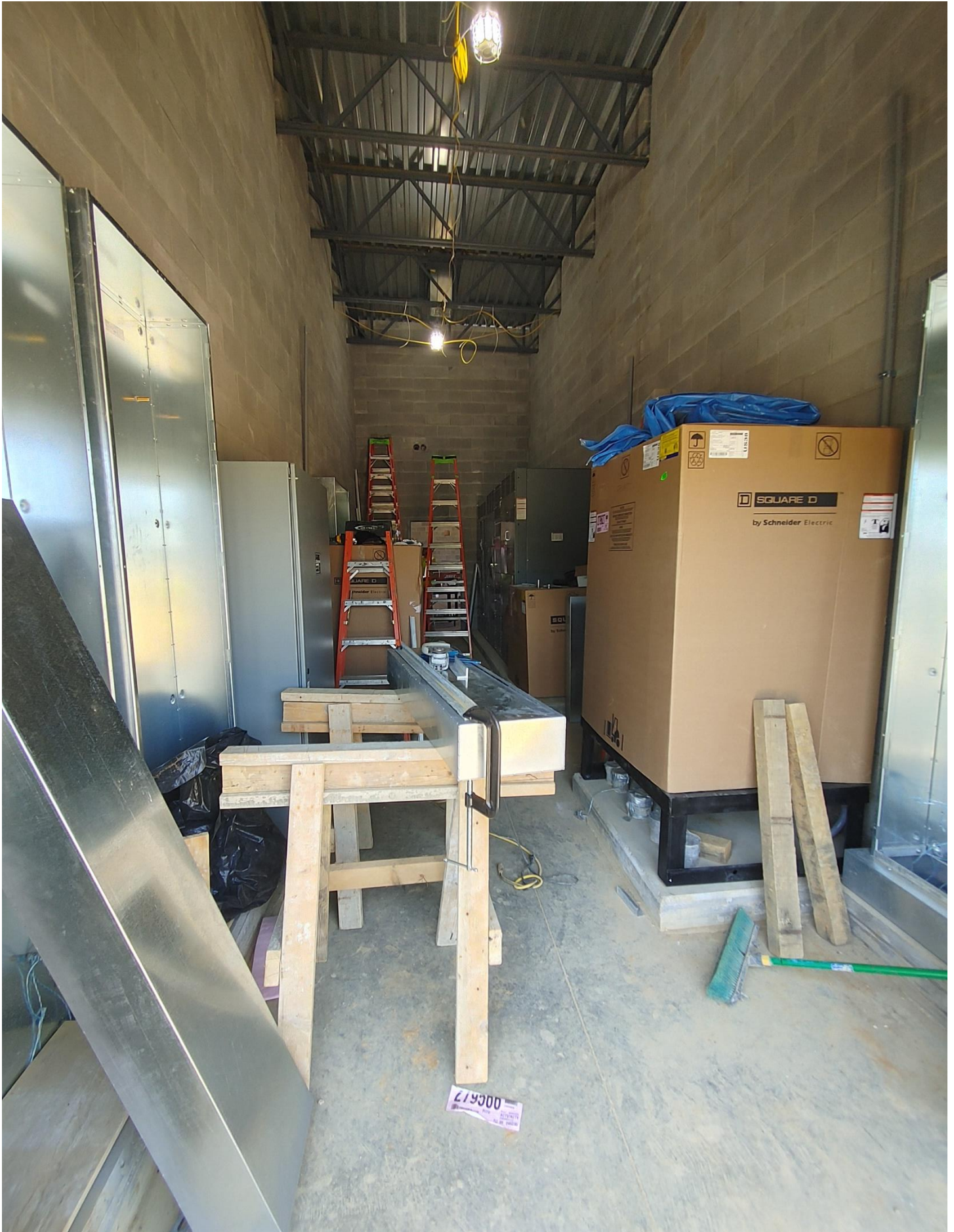
Photo 2 - More equipment being installed in Electrical Room D158
