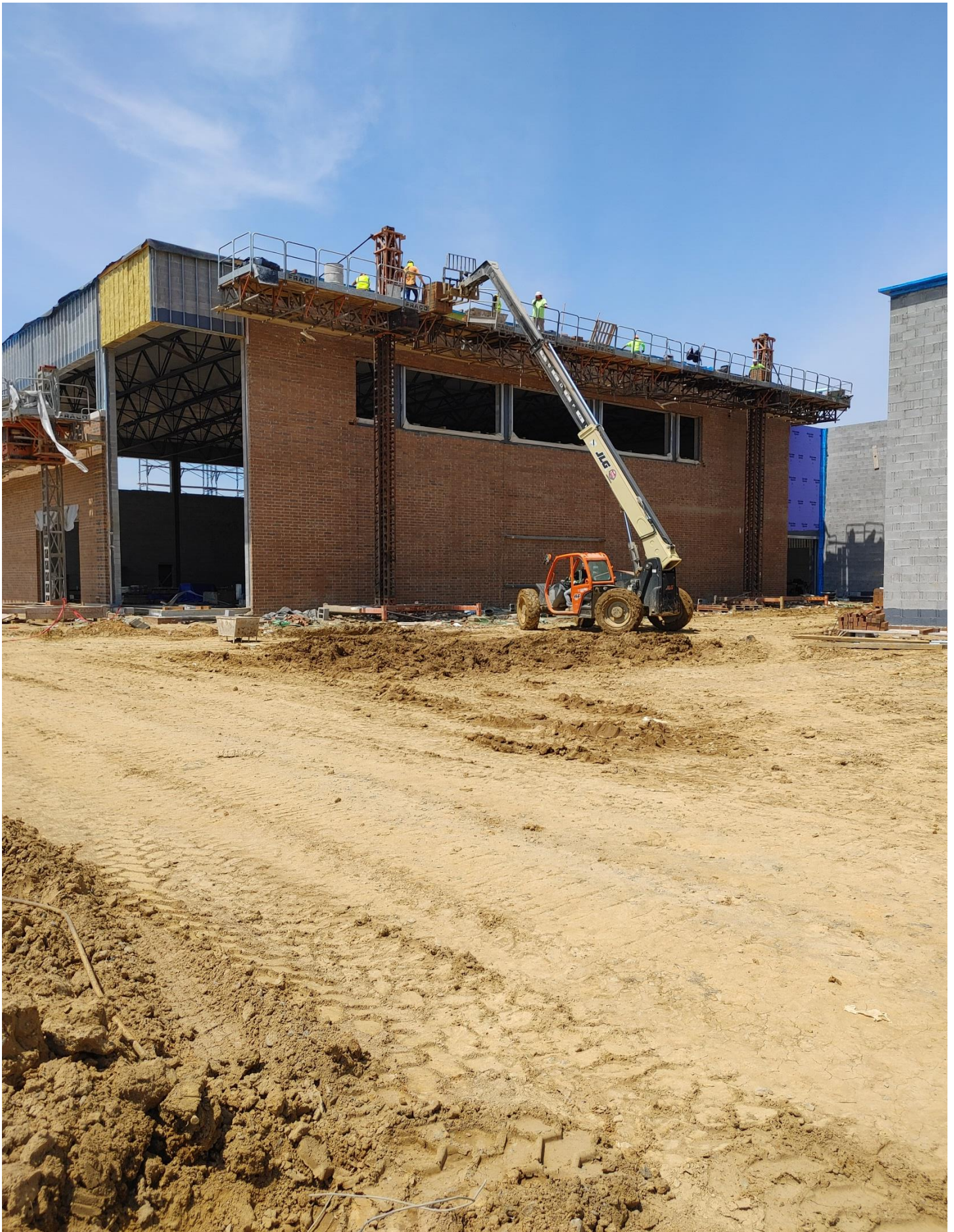
Photo 3 - Masons are laying Brick on the East side of Area E
