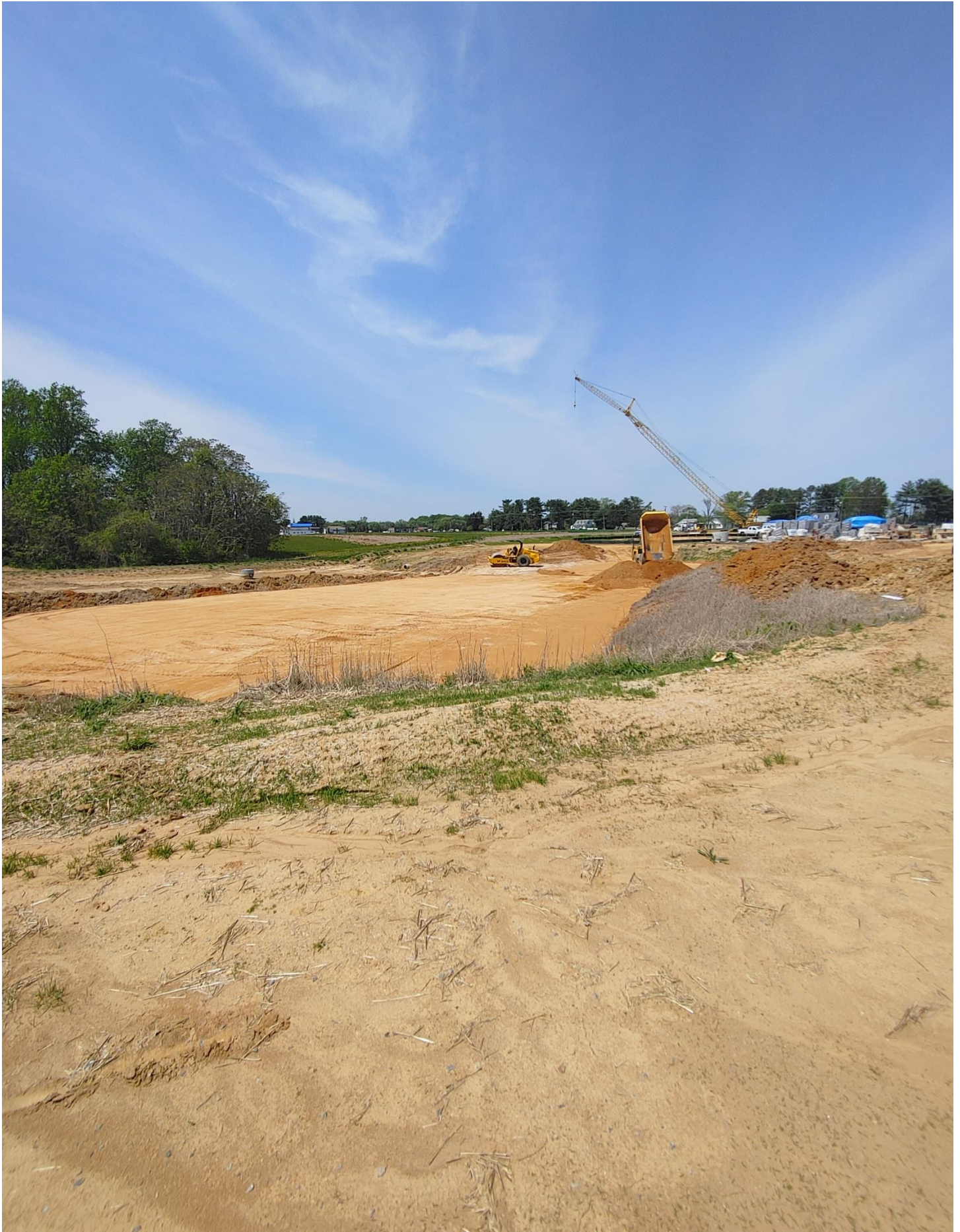
Photo 4 - Rework of Retention Pond #1 continues.
