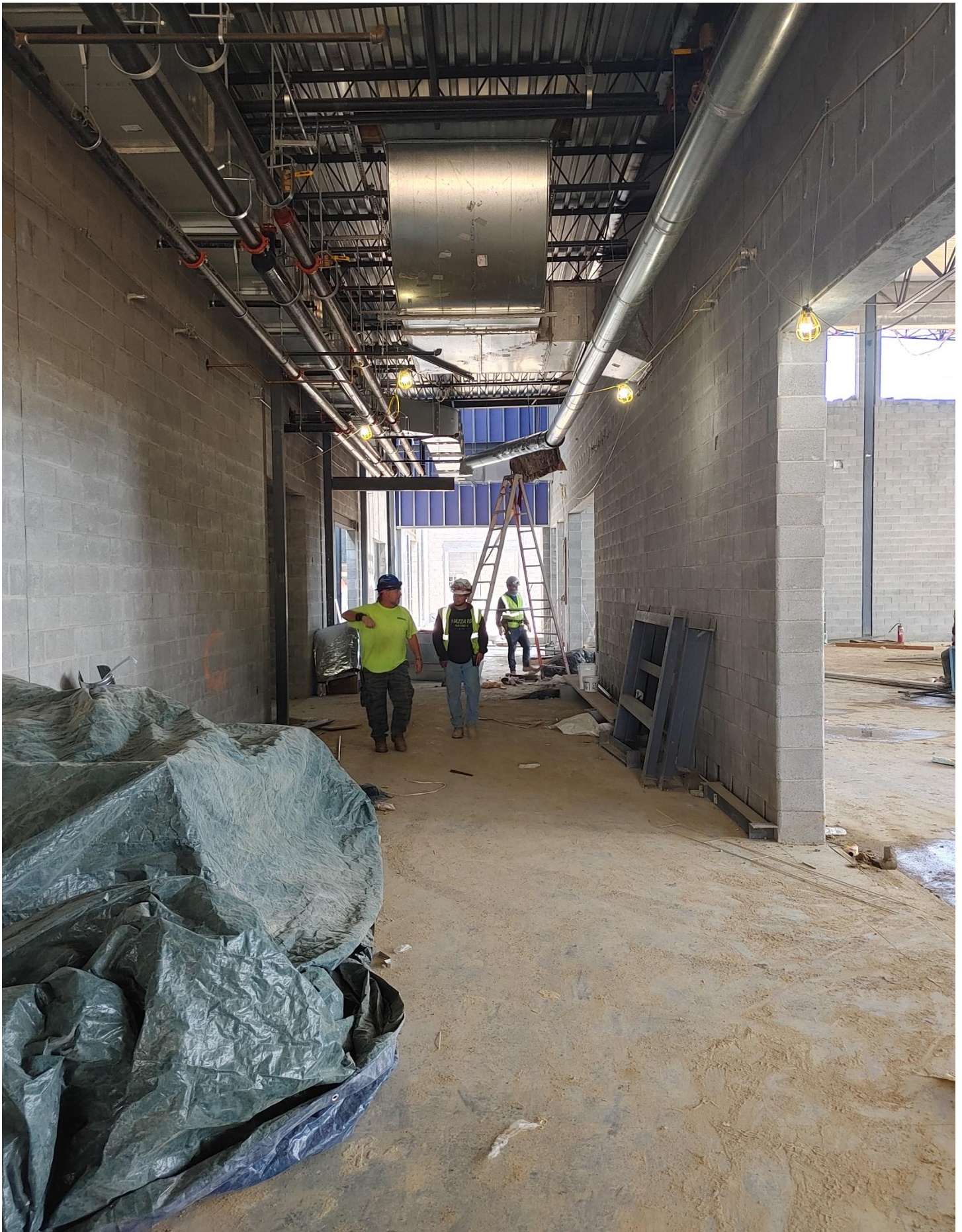
Photo 5 - HVAC Duct being insulated in Area E
