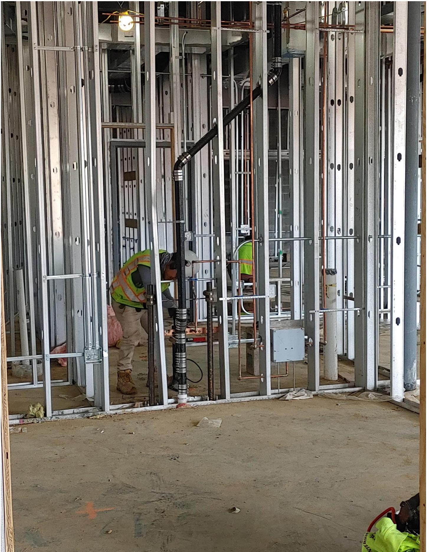
Photo 6 - Colonial Webb pressurizing lines in Area A.
