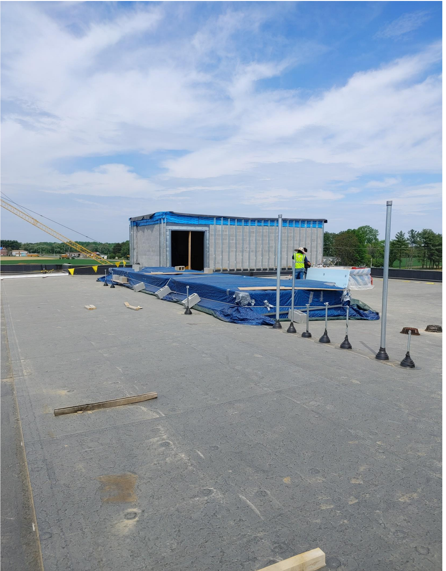
Photo 6 - Z-Channel Framing continues on Stairwell #2
