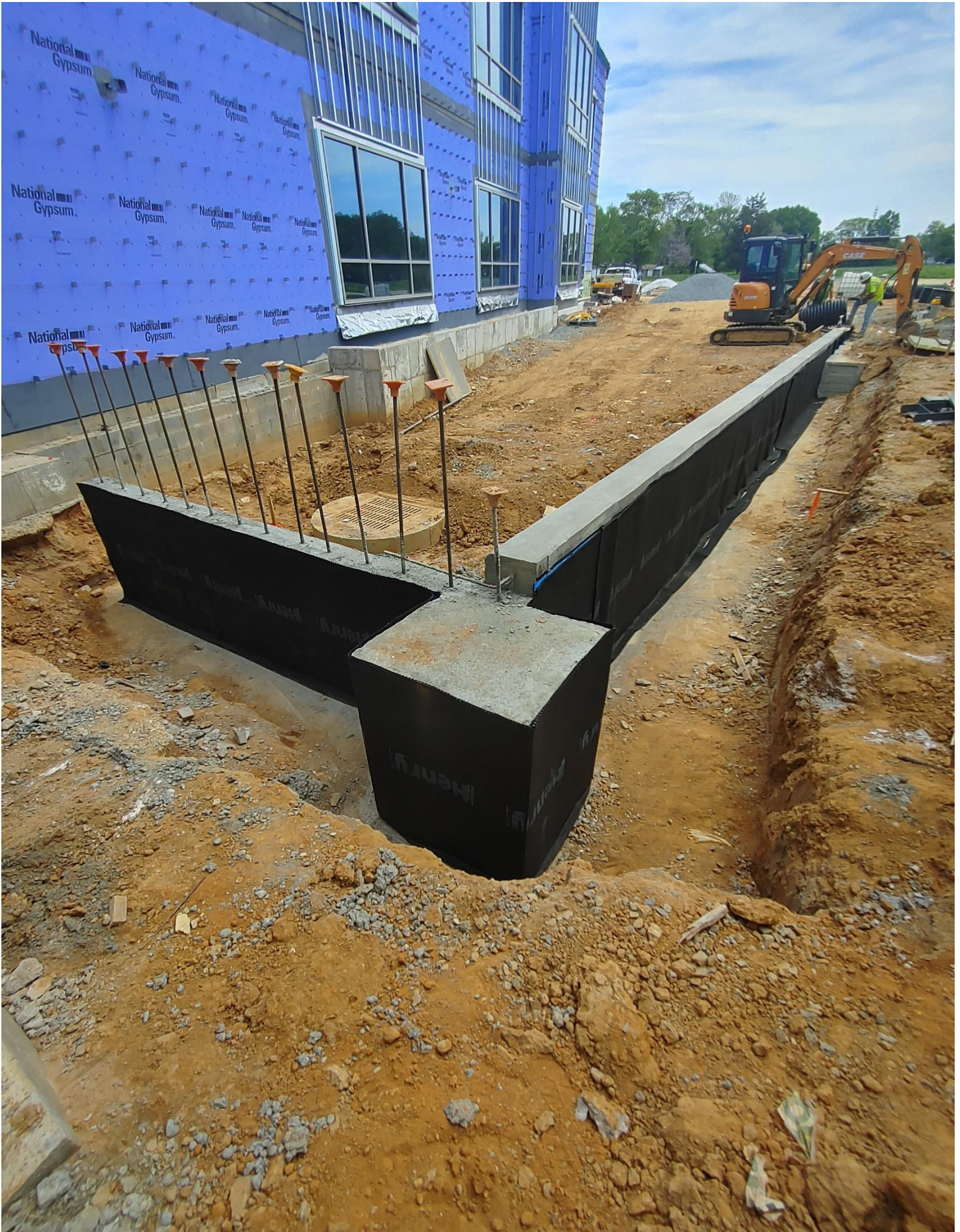
Photo 3 - Loading Dock Wall has waterproof Membrane installed.
