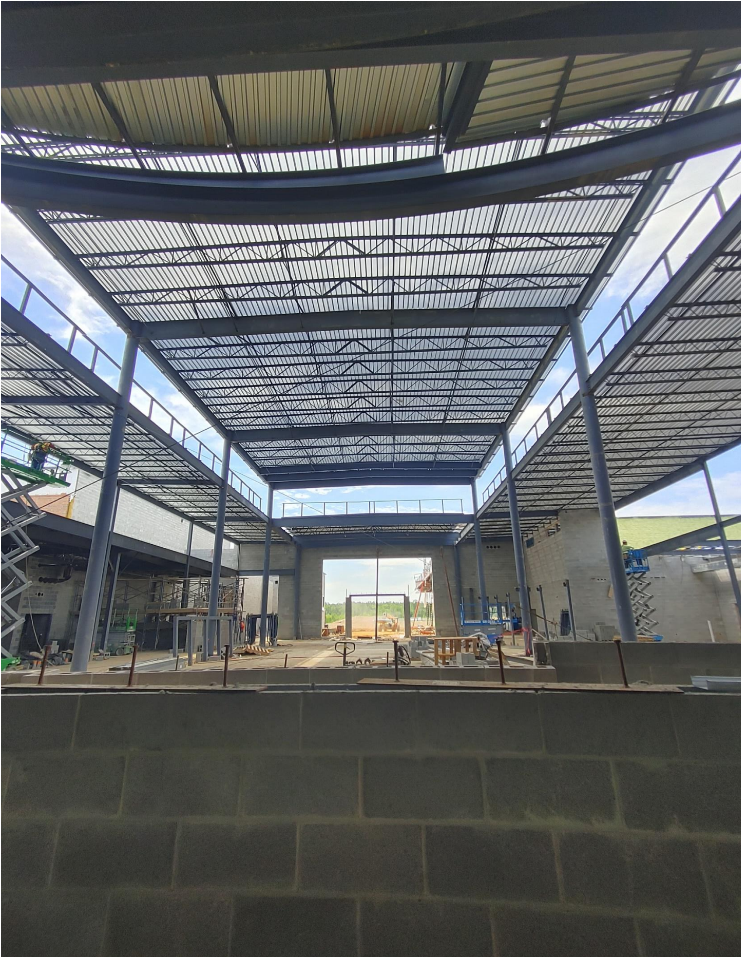
Photo 1- Roof Decking almost completed in Area C
