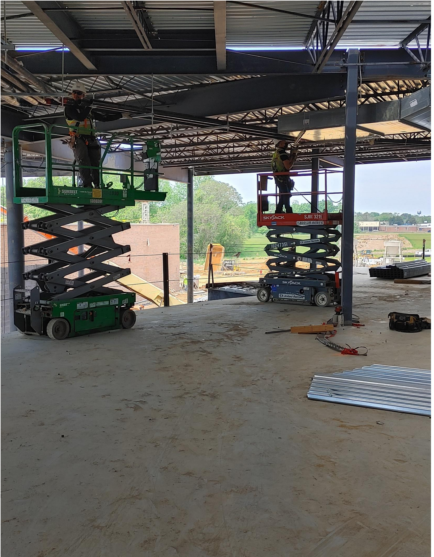
Photo 4 - Colonial Webb continues to run pipe in Area A
