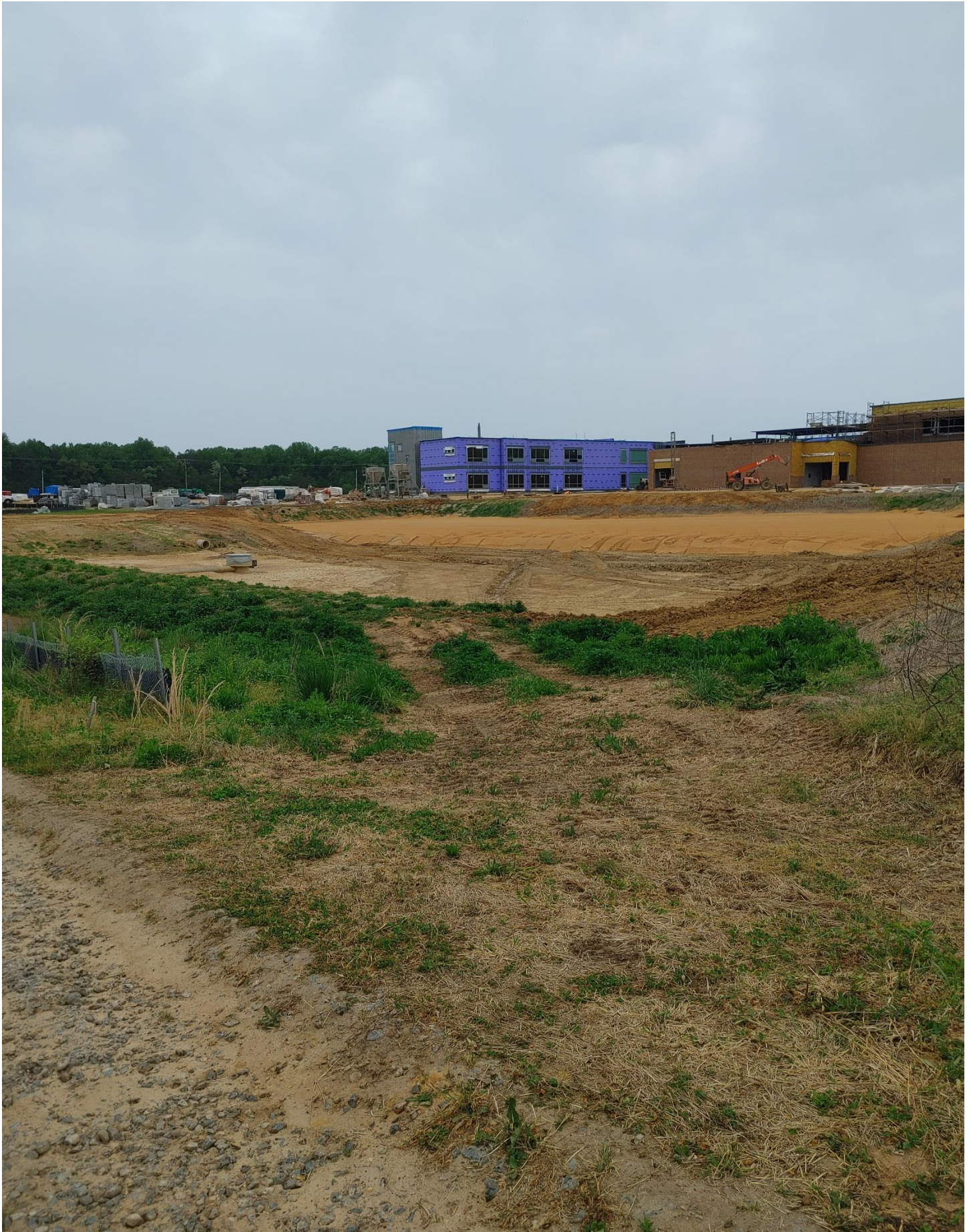
Photo 2 - Retention Pond #1 being reworked.
