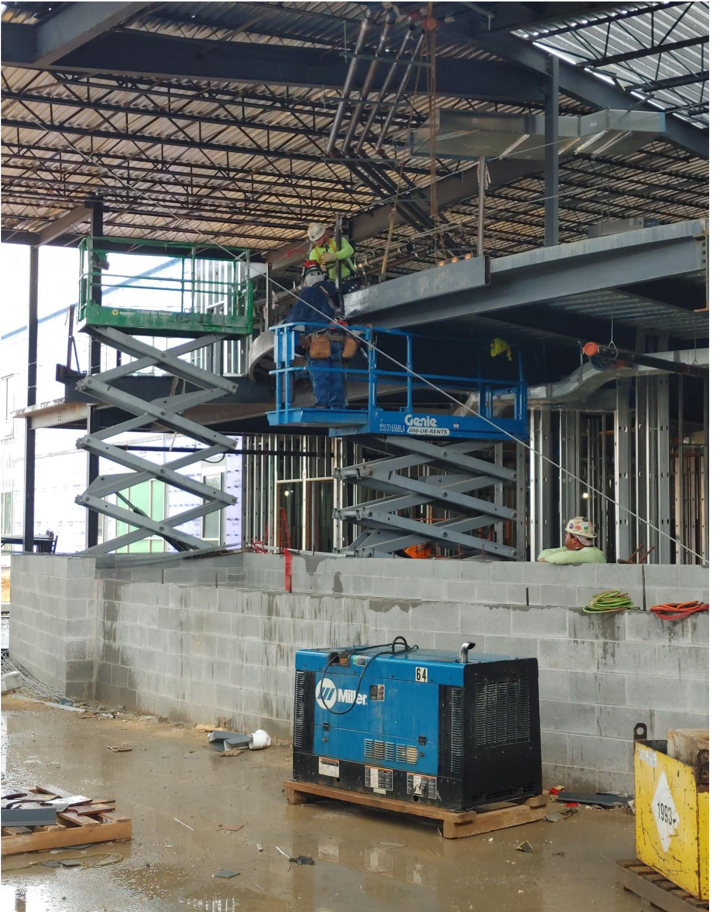
Photo 3 - Weldon Steel working of Stair #3
