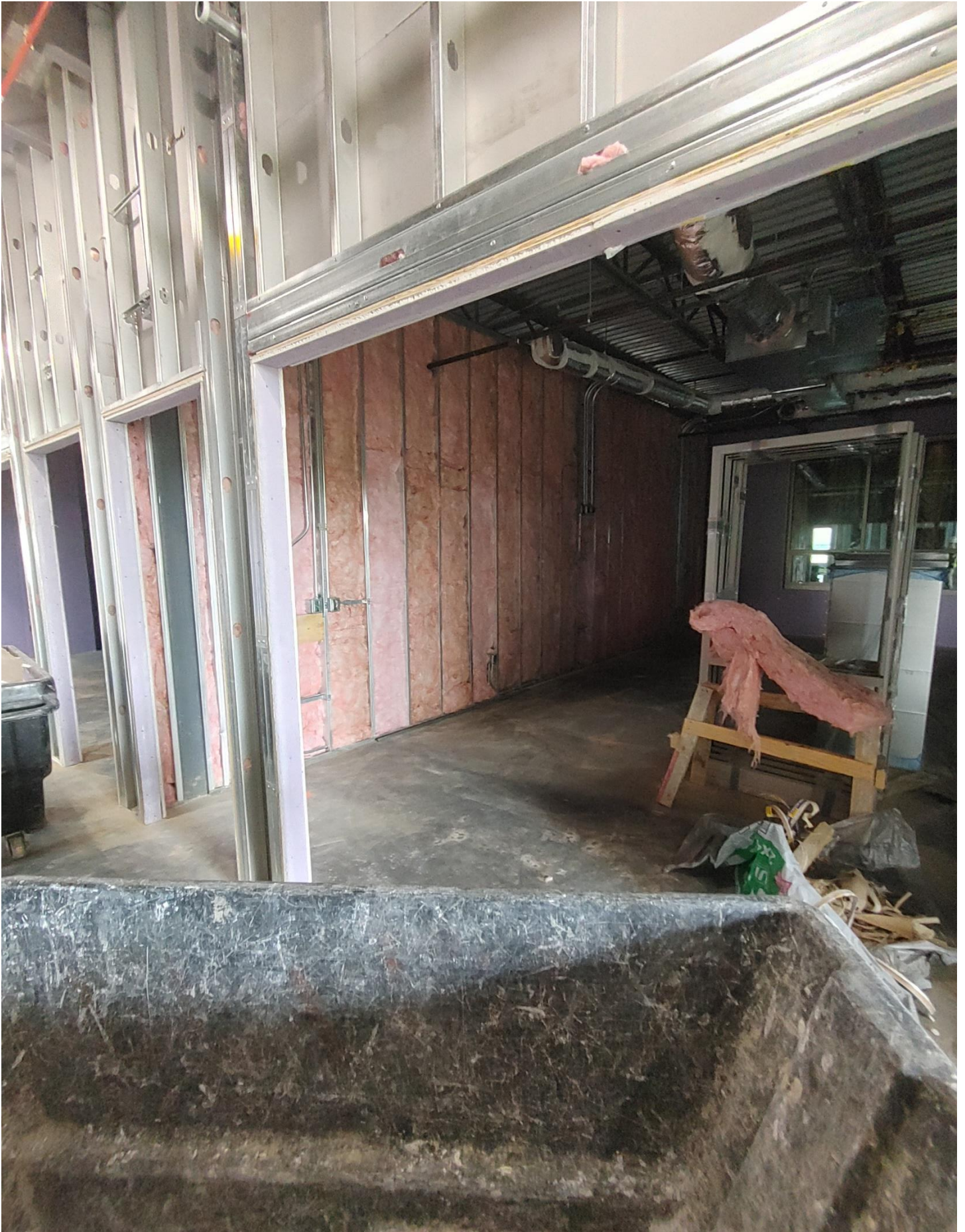
Photo 5 - Walls being insulated in Area A
