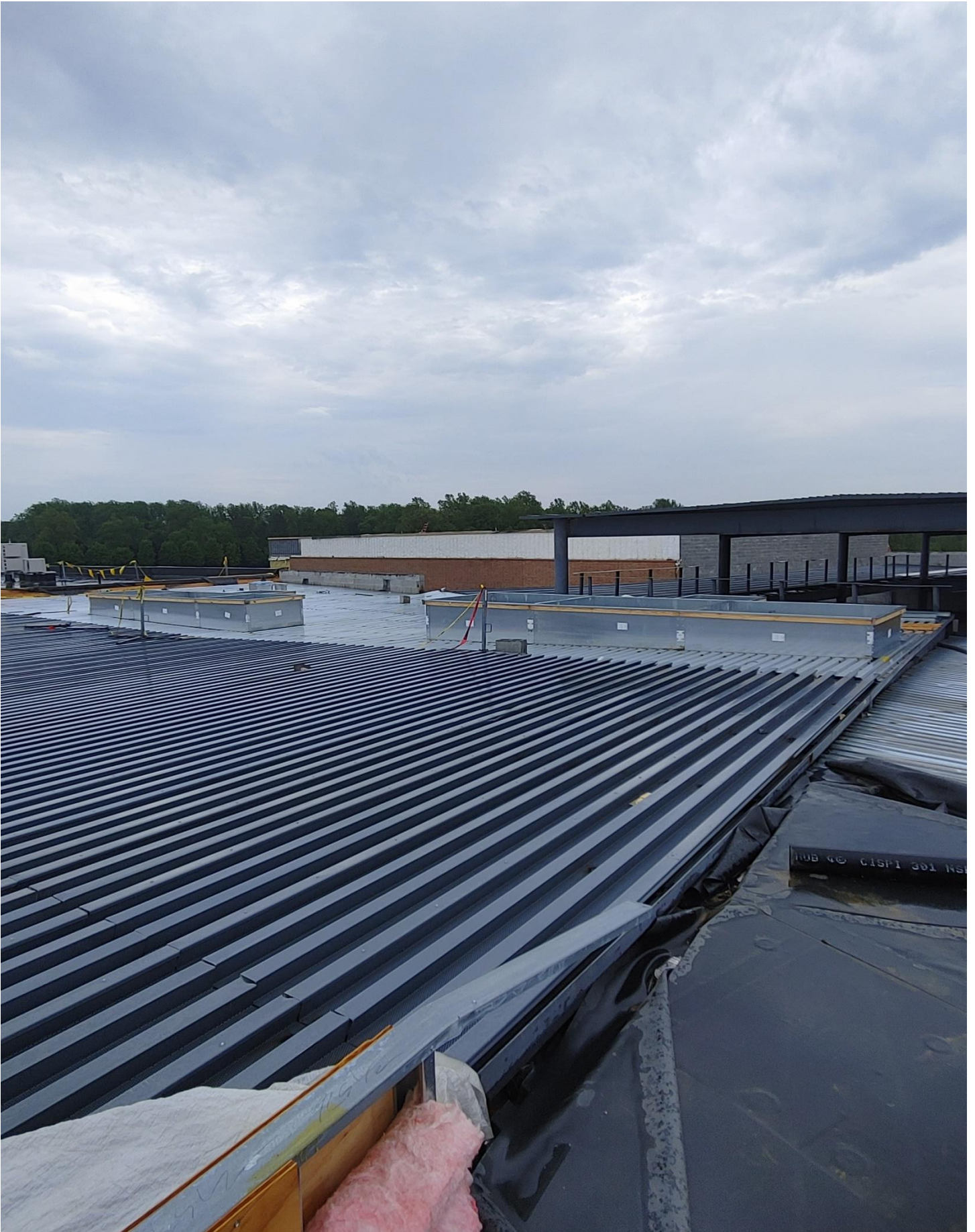
Photo 7 - HVAC equipment curbs being constructed above Area A.
