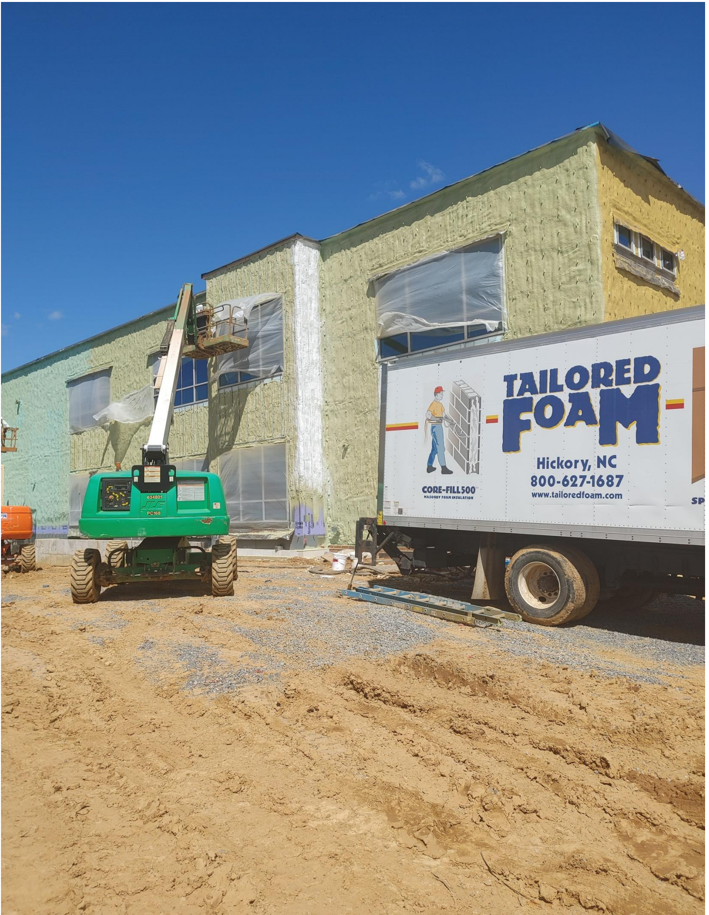
Photo 1 – Spray foam being applied to the South Side of Area A
