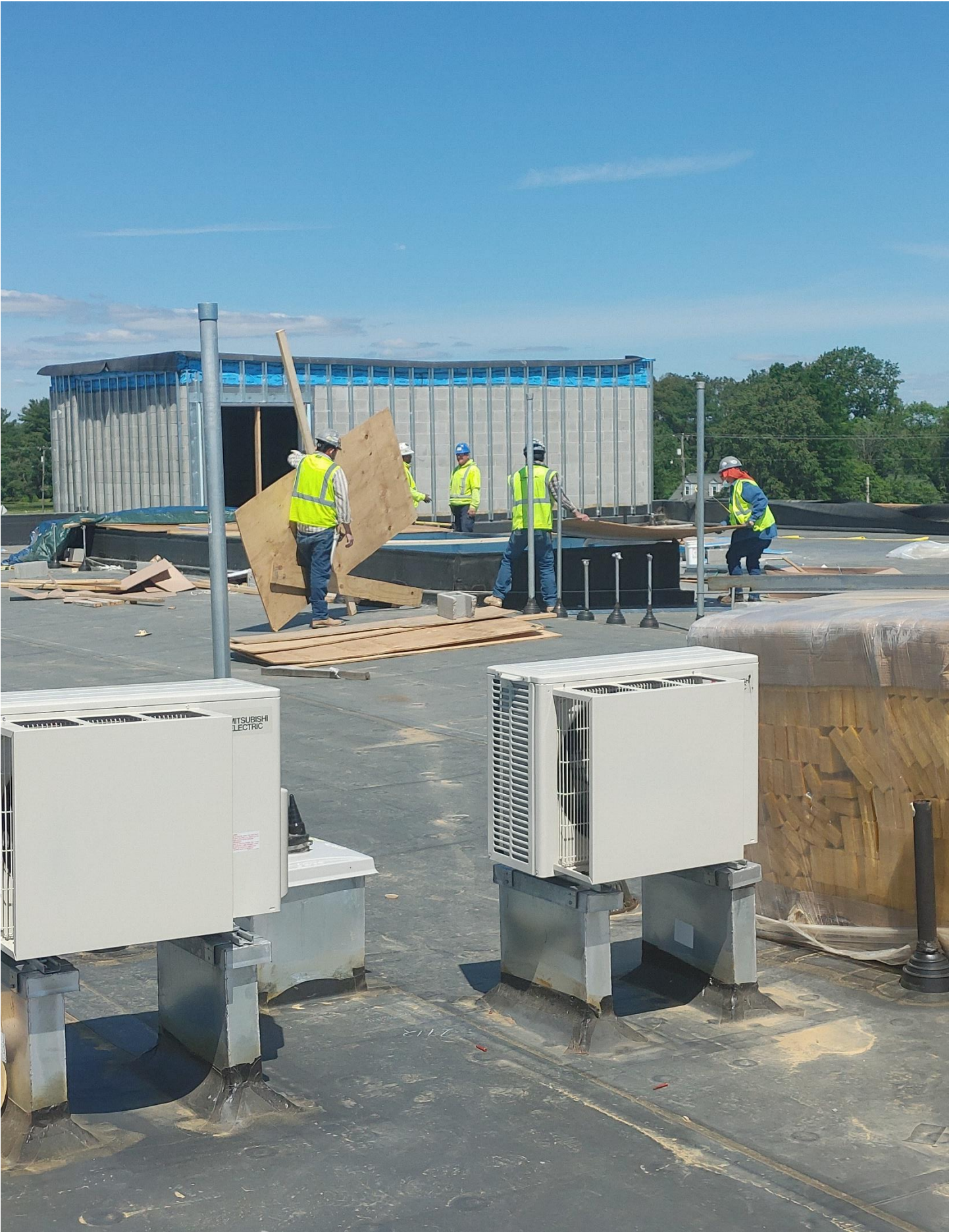
Photo 14 - Colonial Webb working on Curbs on the Roof of Area B
