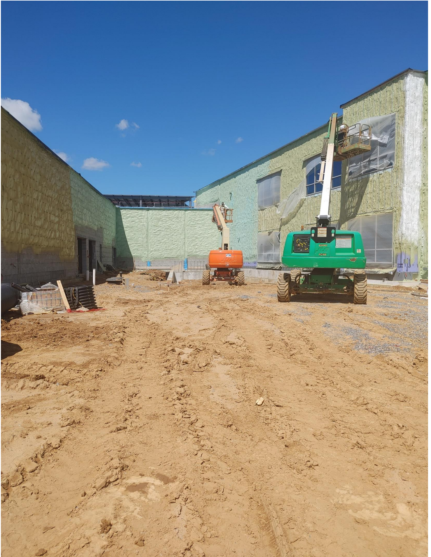
Photo 2 - Spray foam being applied to the East side of Area C
