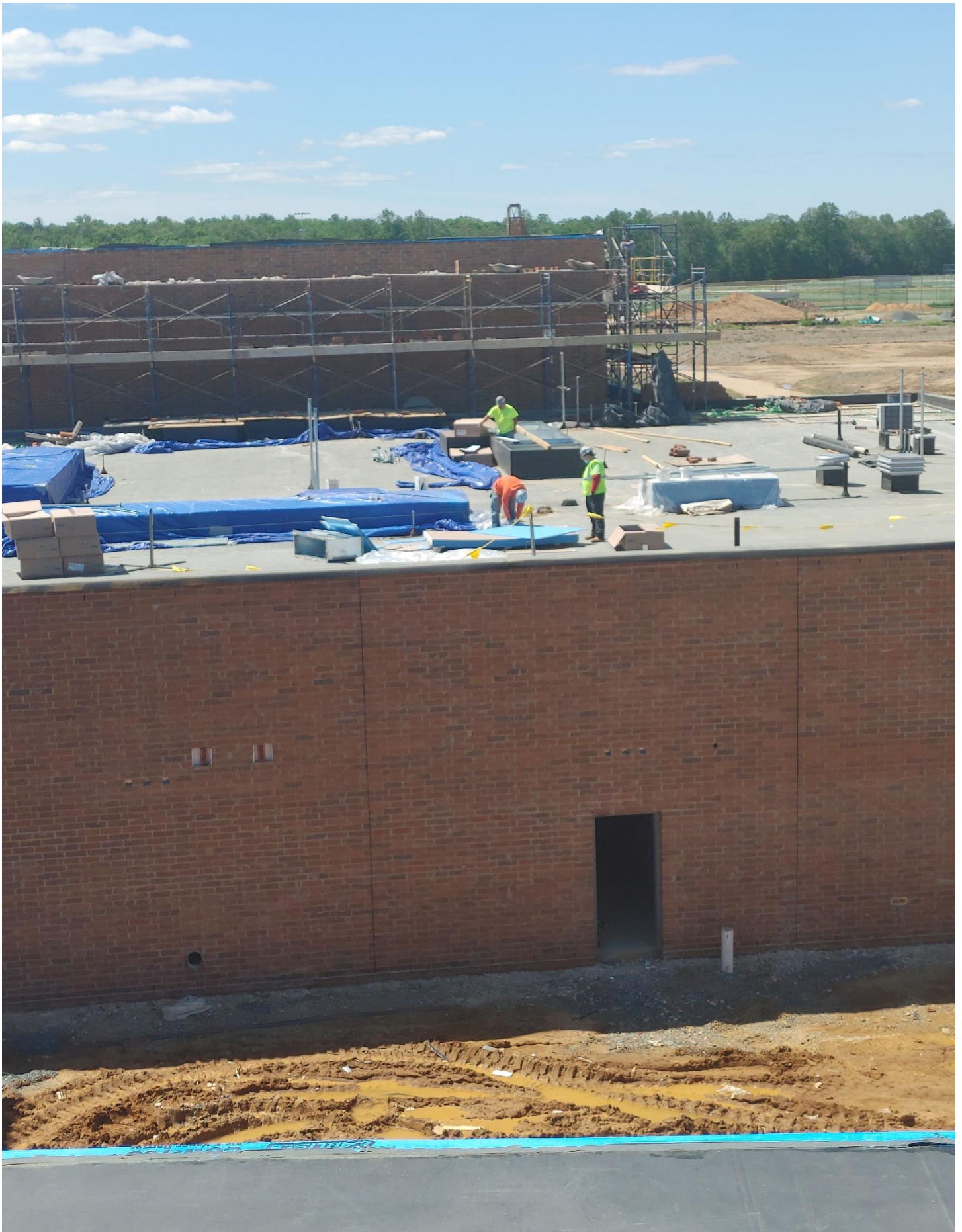
Photo 13 - Colonial Webb working on Curbs on the Roof of Area E
