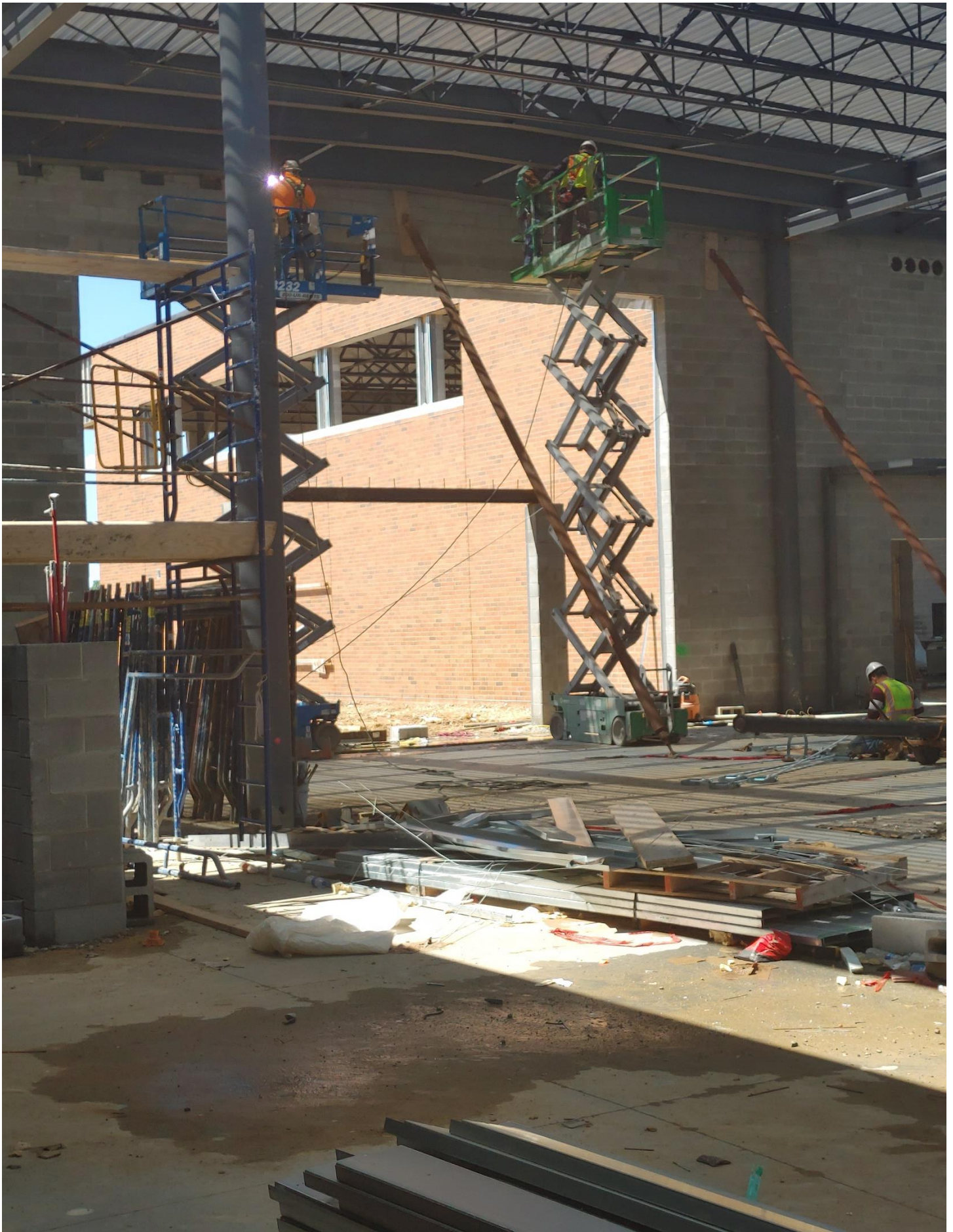
Photo 6 - Steel being welded in Area C
