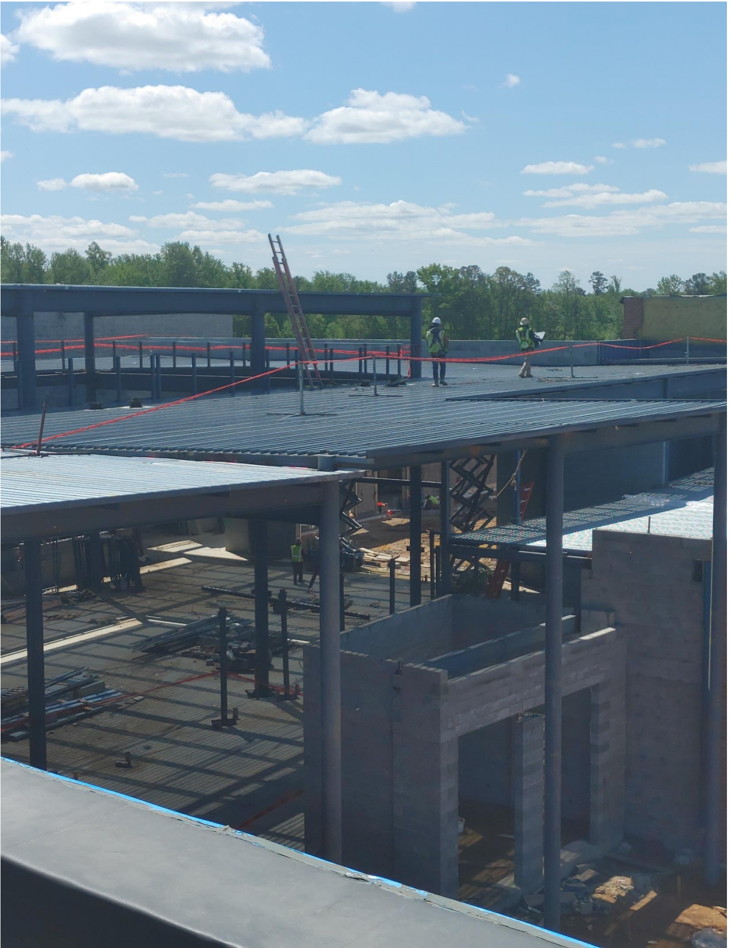
Photo 12 - Roof Drains being set in Area C
