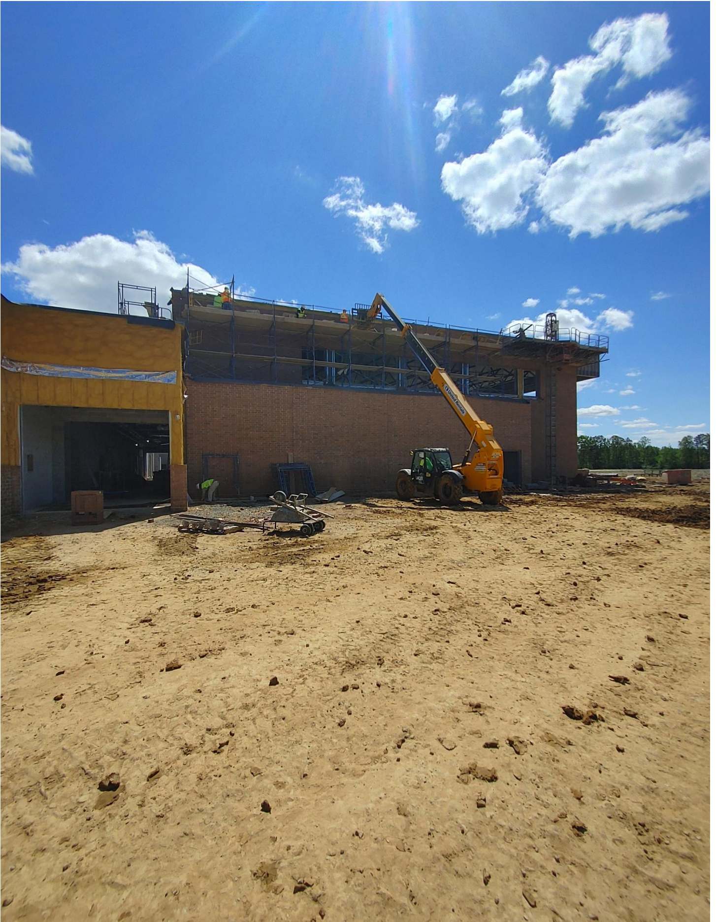
Photo 9 - Masons are laying Brick on the West side of Area E
