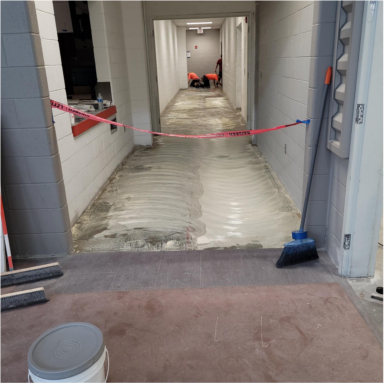
Photo 5 - Tile is being laid in Corridor D#14 & #15
