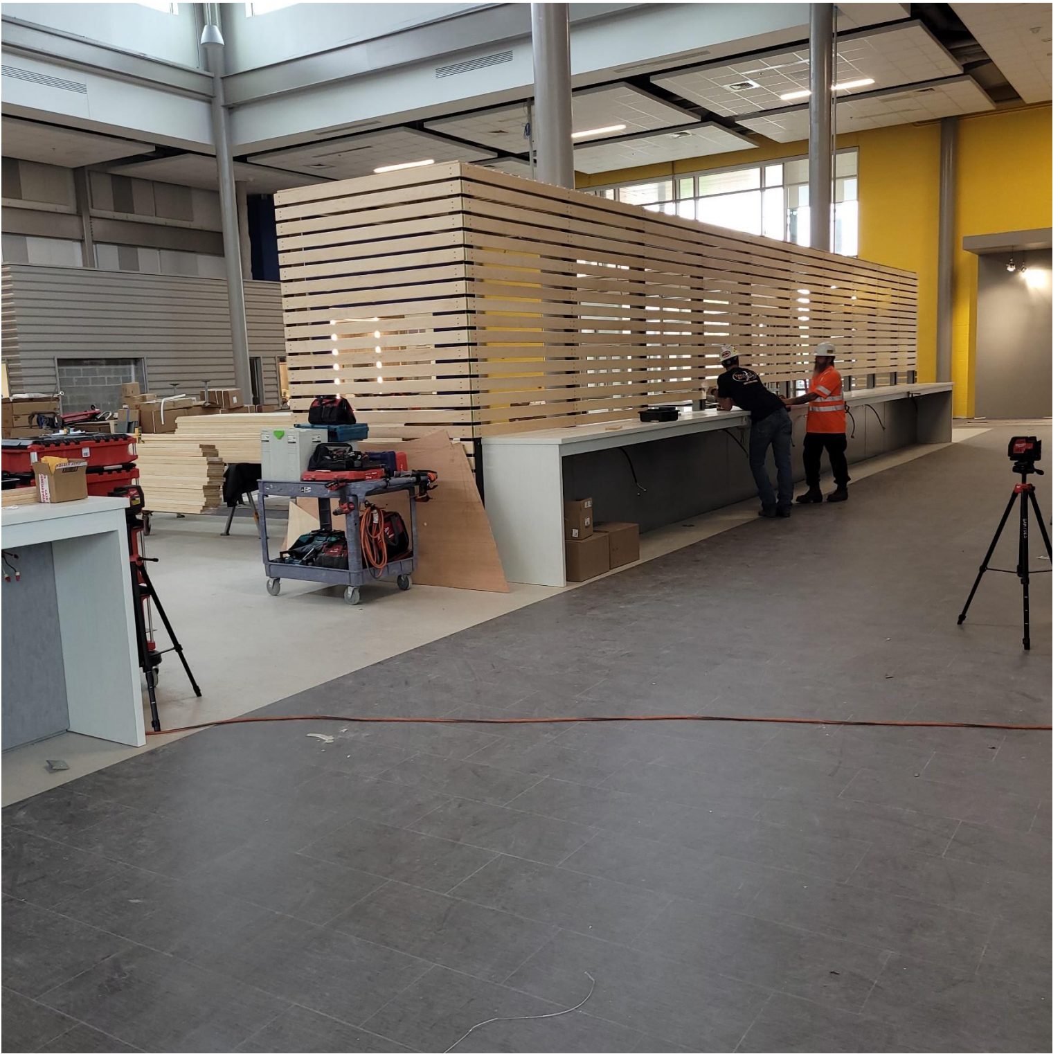
Photo 4 - Work continues in Area C - Commons Area - Wood Slats
