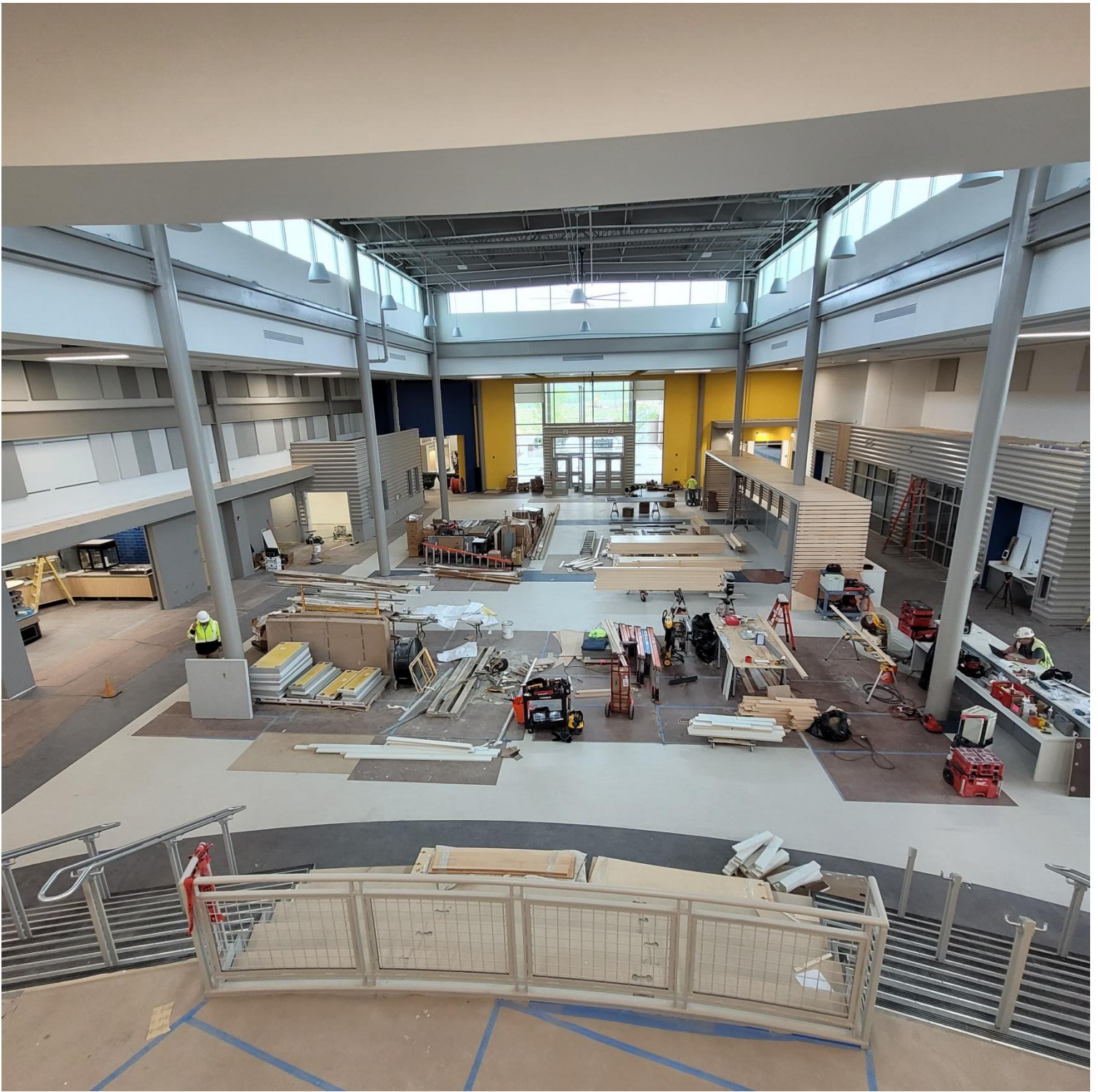
Photo 14 - Area C Mezzanine view
