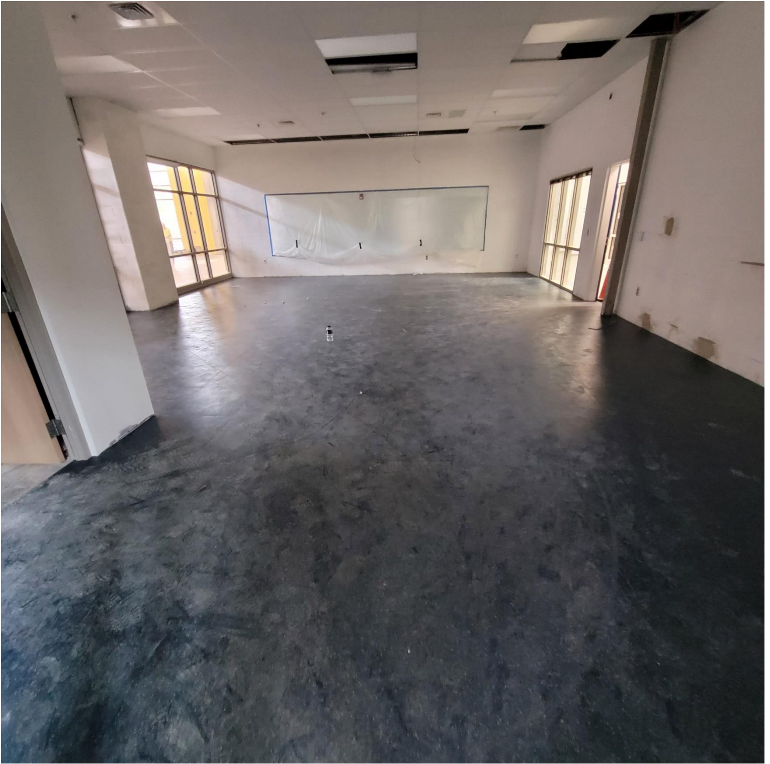
Photo 12 - Fitness E122 Floor has been installed
