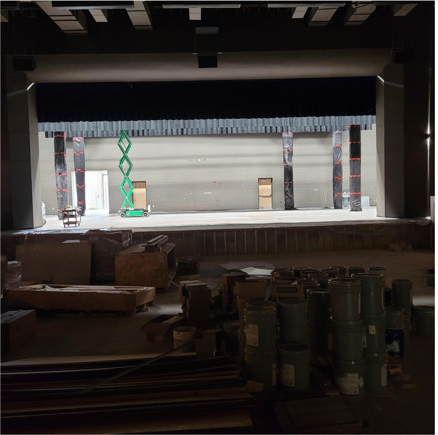
Photo 7 - Stage Curtains have been installed
