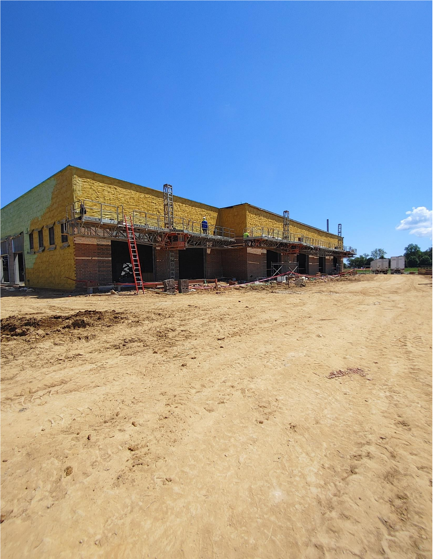
Photo 4 - Brick is being laid on the South side of Area D
