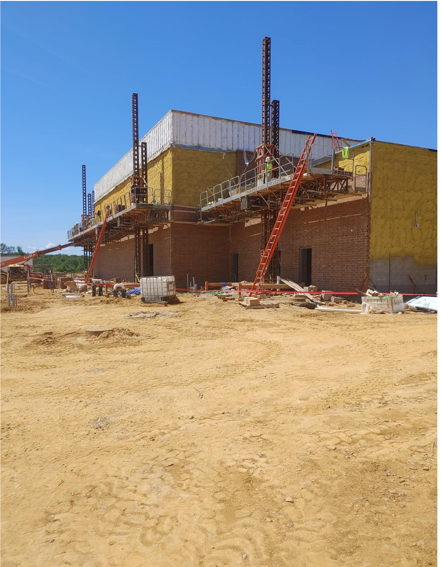
Photo 3 - Masons are laying brick on the East side of Area D
