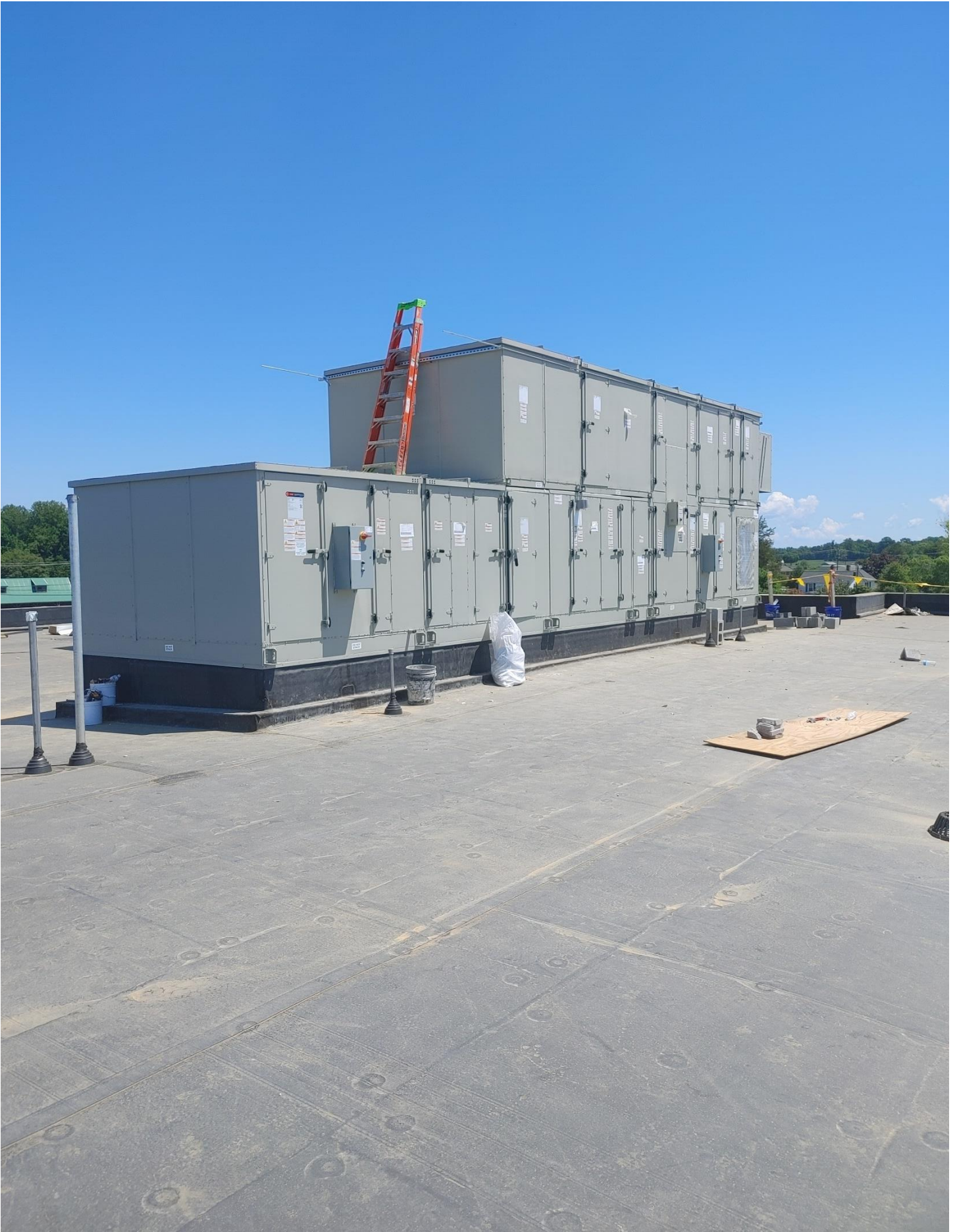
Photo 14 - Roof Top Unit has been set in Area A
