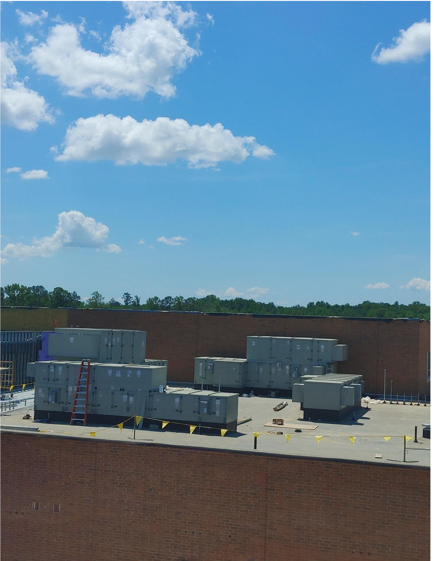
Photo 13 - Roof Top units have been set in Area E
