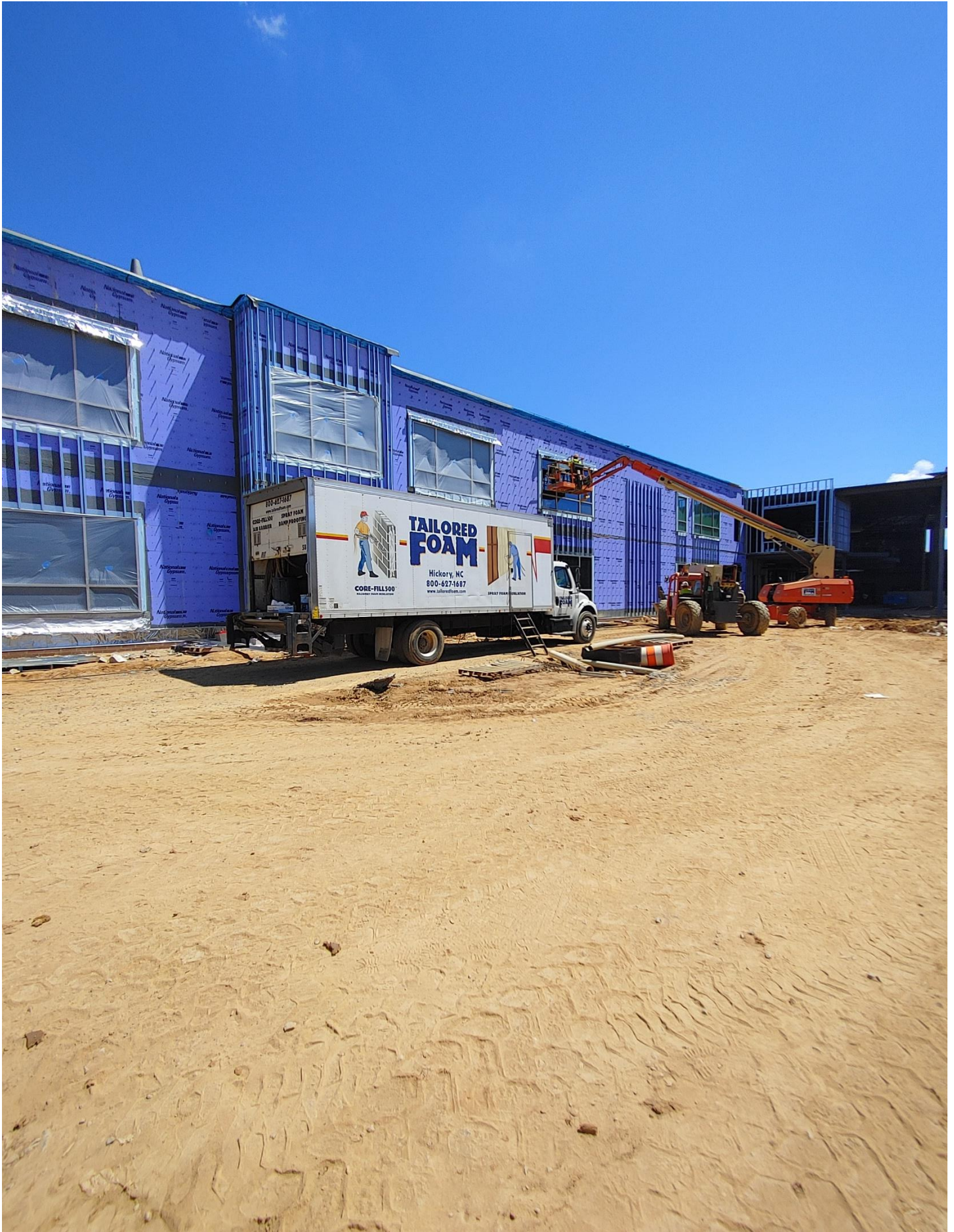
Photo 8 - Tailored Foam setting up on the South side of Area B
