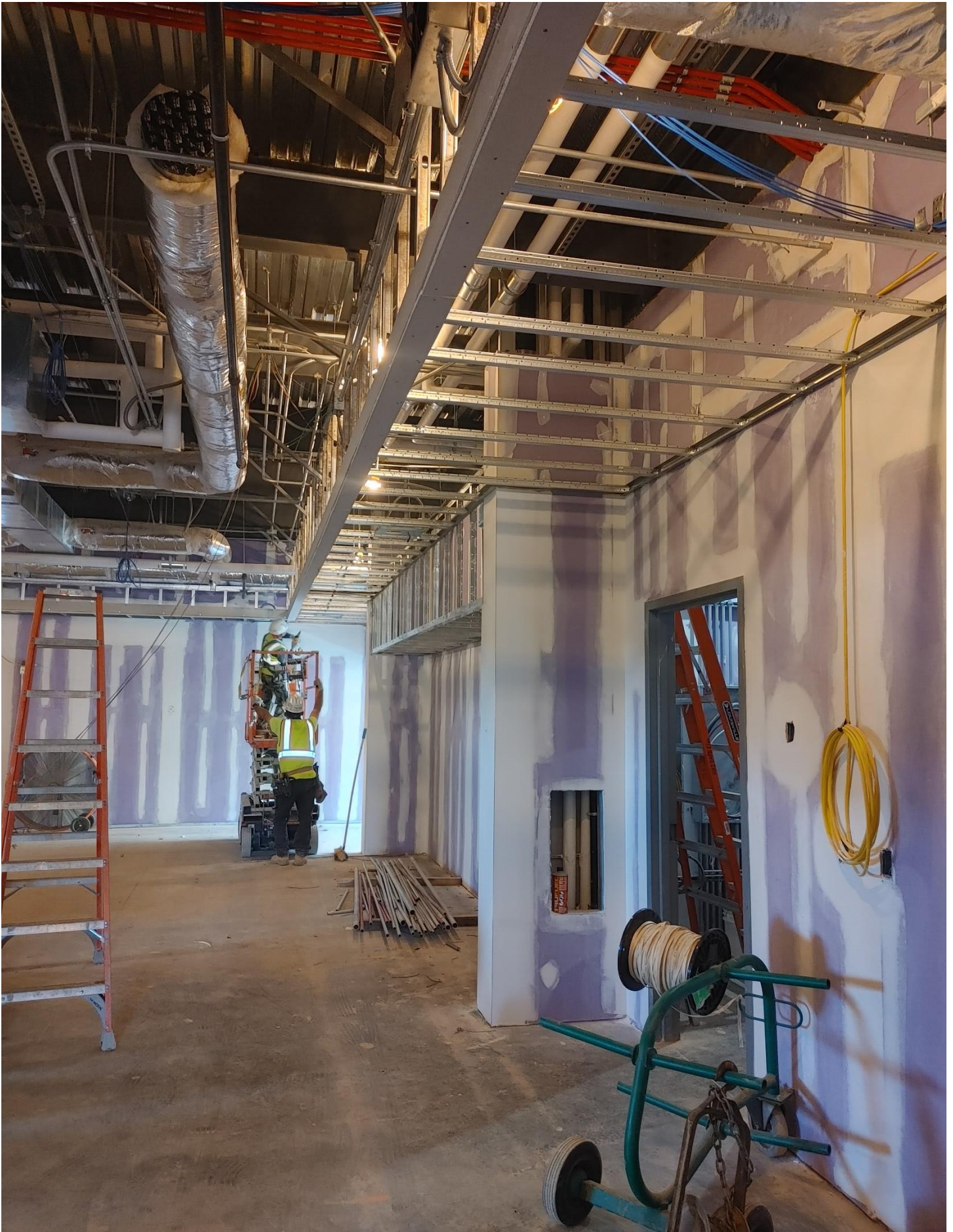
Photo 2 - Bulk Heads being constructed in Area A
