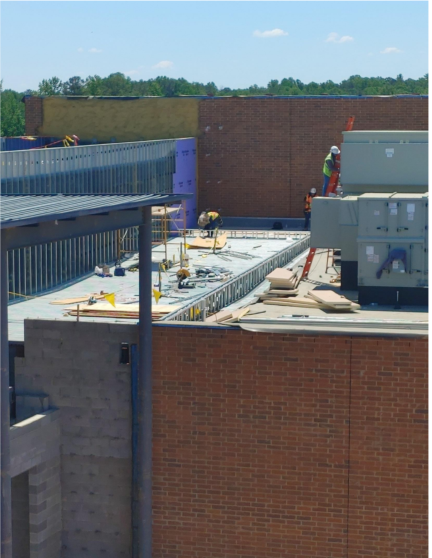
Photo 7 - Parapet walls being constructed on the roof of Area E
