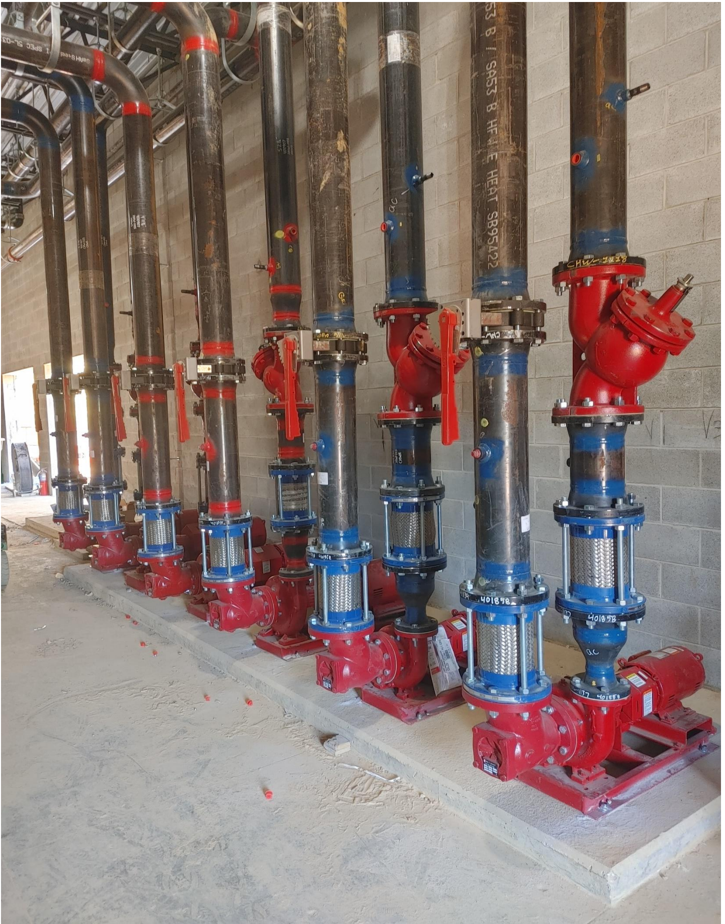
Photo 1 - Work continues in Area D Mechanical Room
