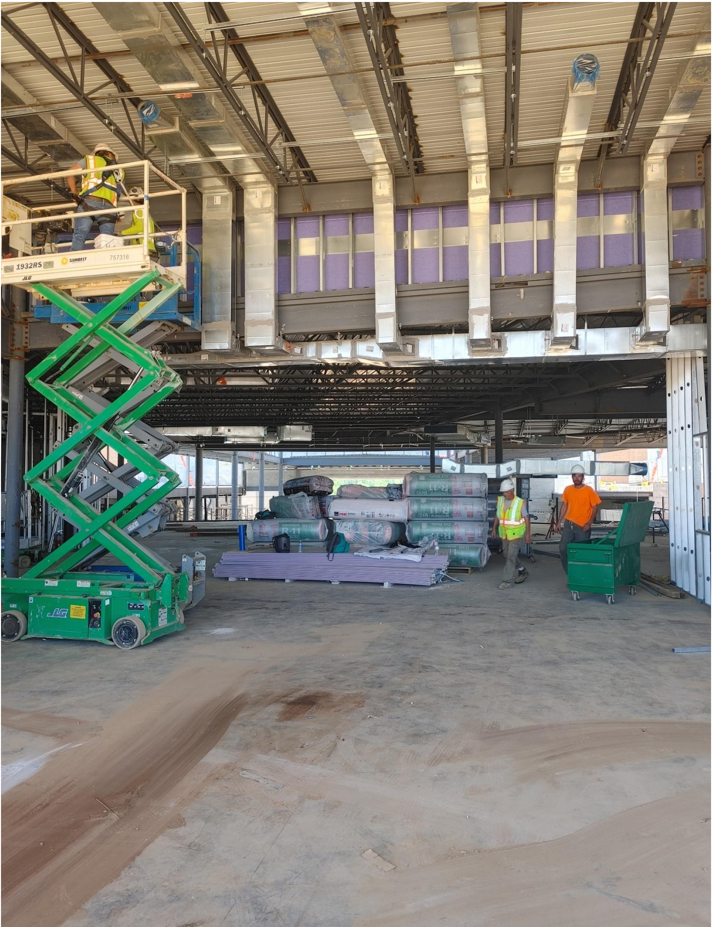
Photo 4 - Duct Banks being run in Area A
