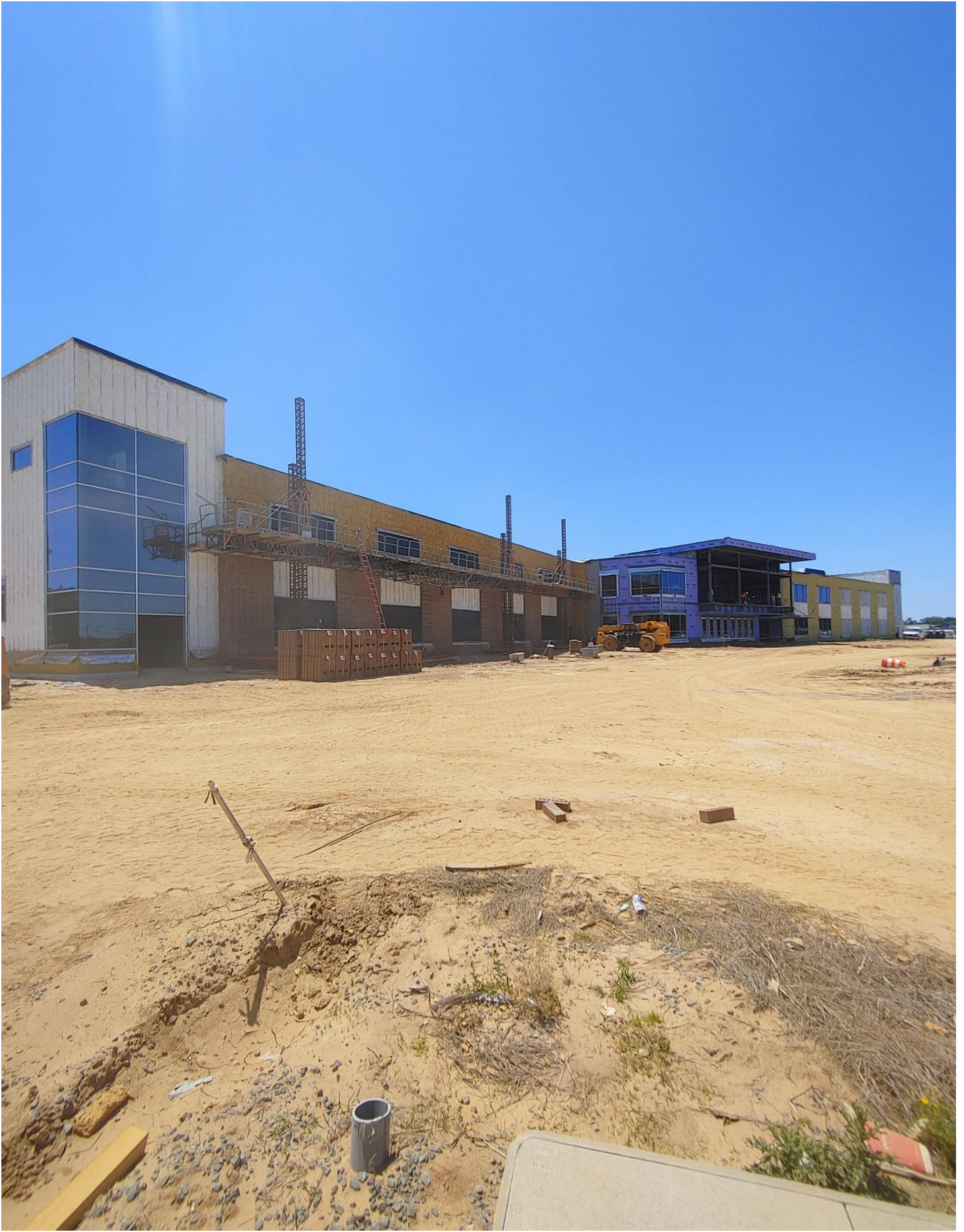
Photo 8 - Front elevation coming along
