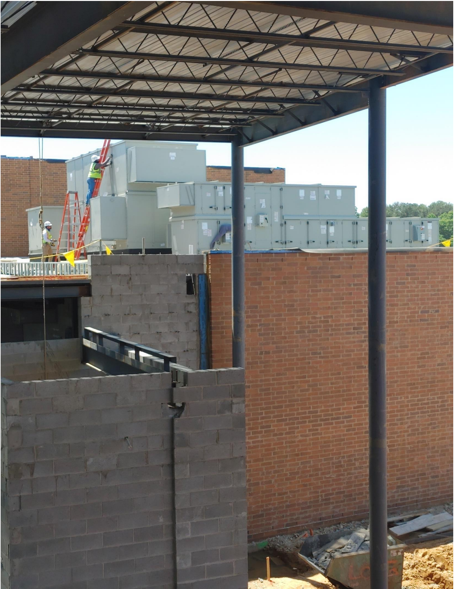
Photo 5 - Work continues on the roof top units in Area E
