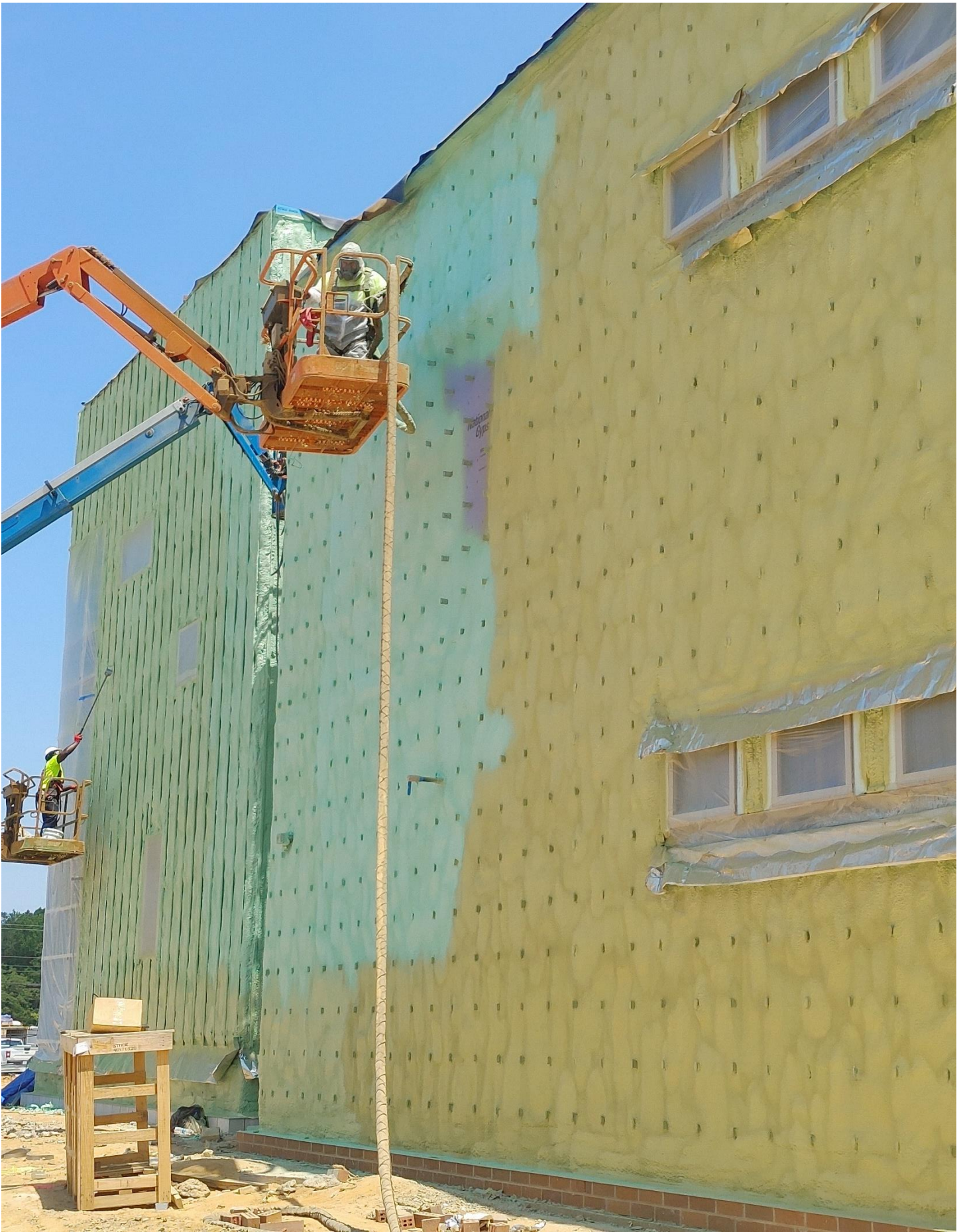
Photo 9 - West side of Area B receiving Spray Foam
