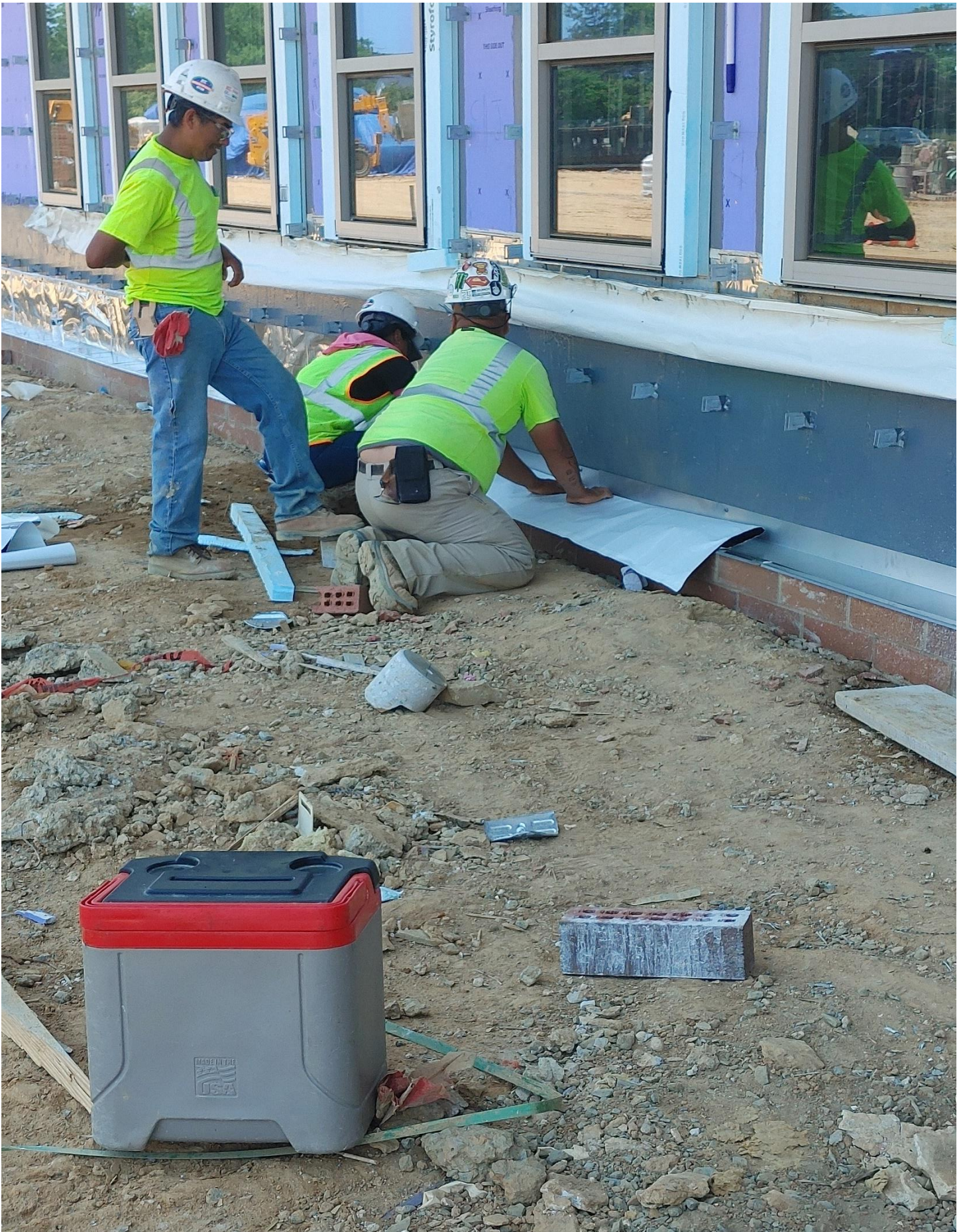
Photo 10 - Brick being flashed on the North side of Area A
