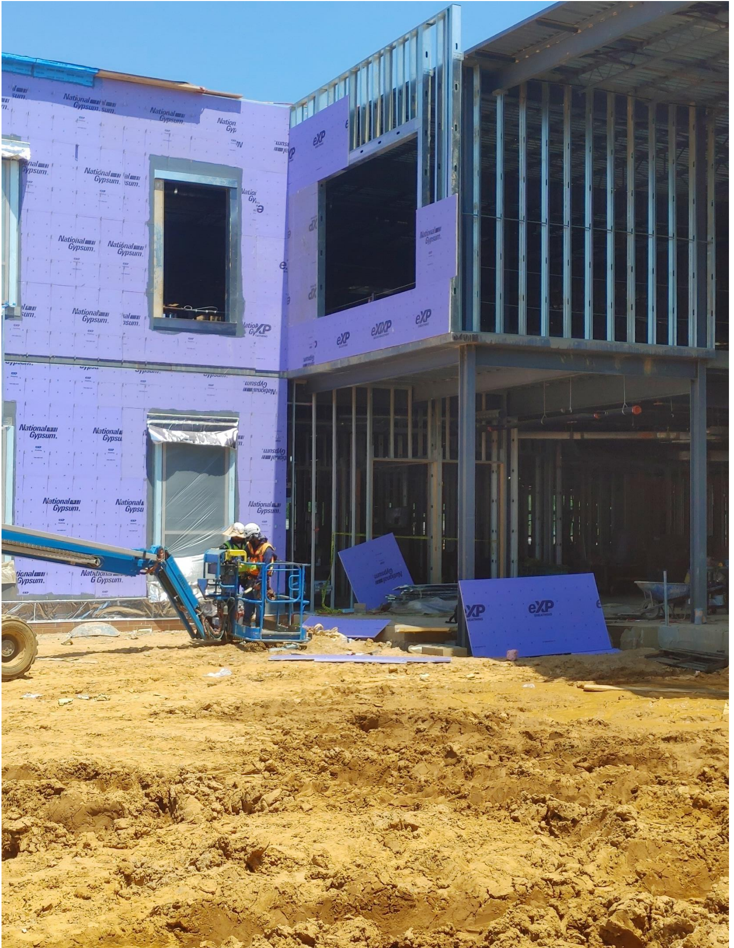
Photo 8 - Gyp Board being hung on the West side of Area C
