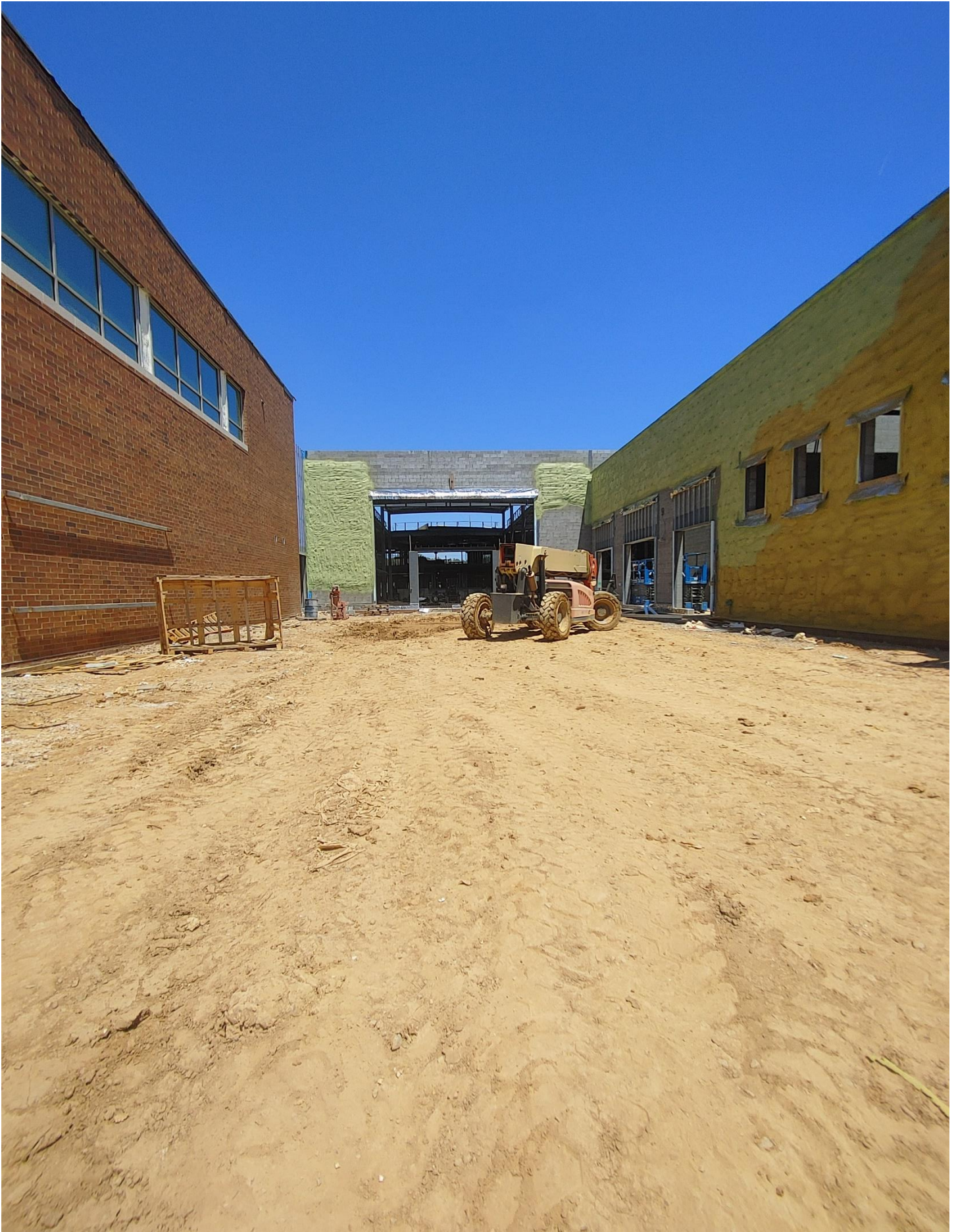
Photo 3 - The South side of Area C has begun to receive foam.
