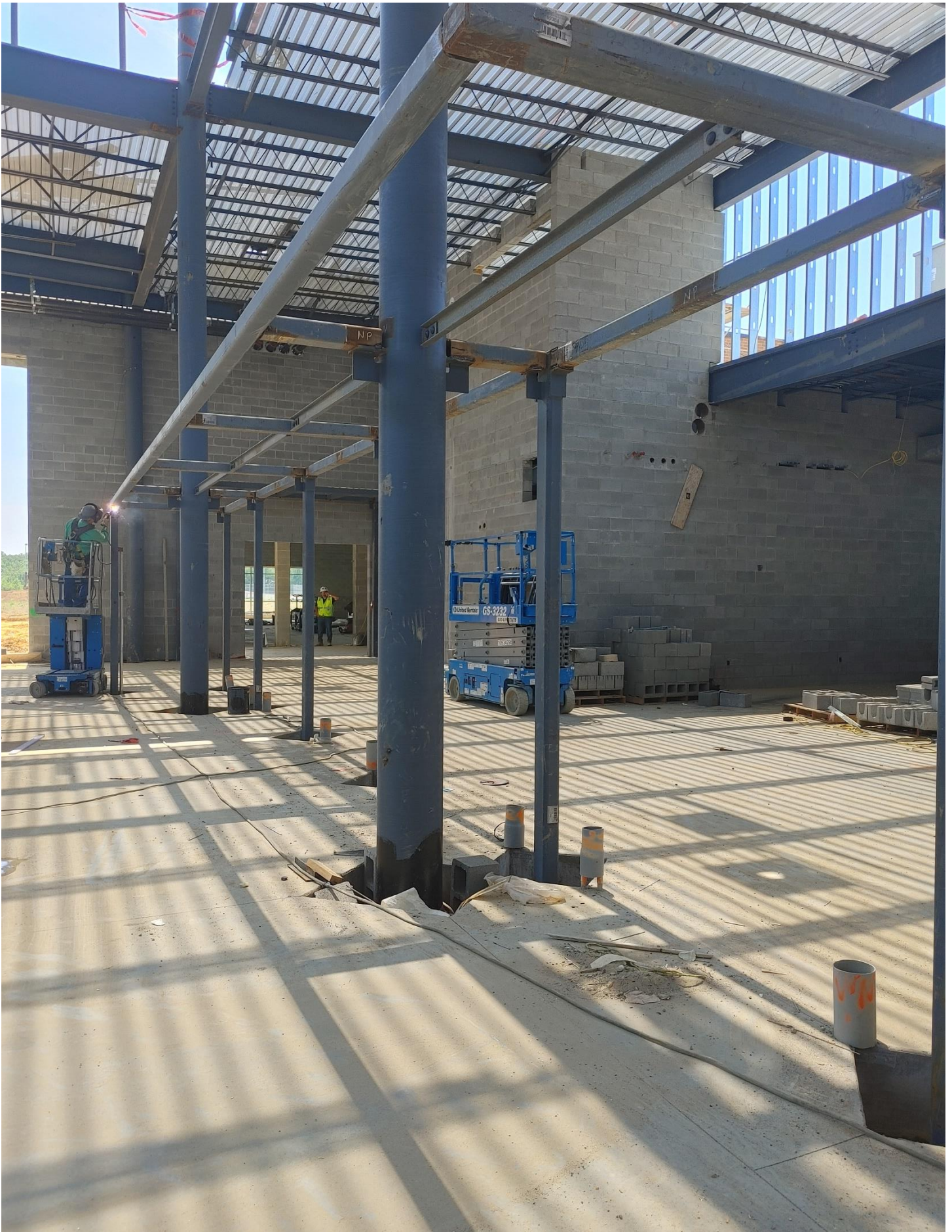
Photo 7 - Steel being welded in Area C.
