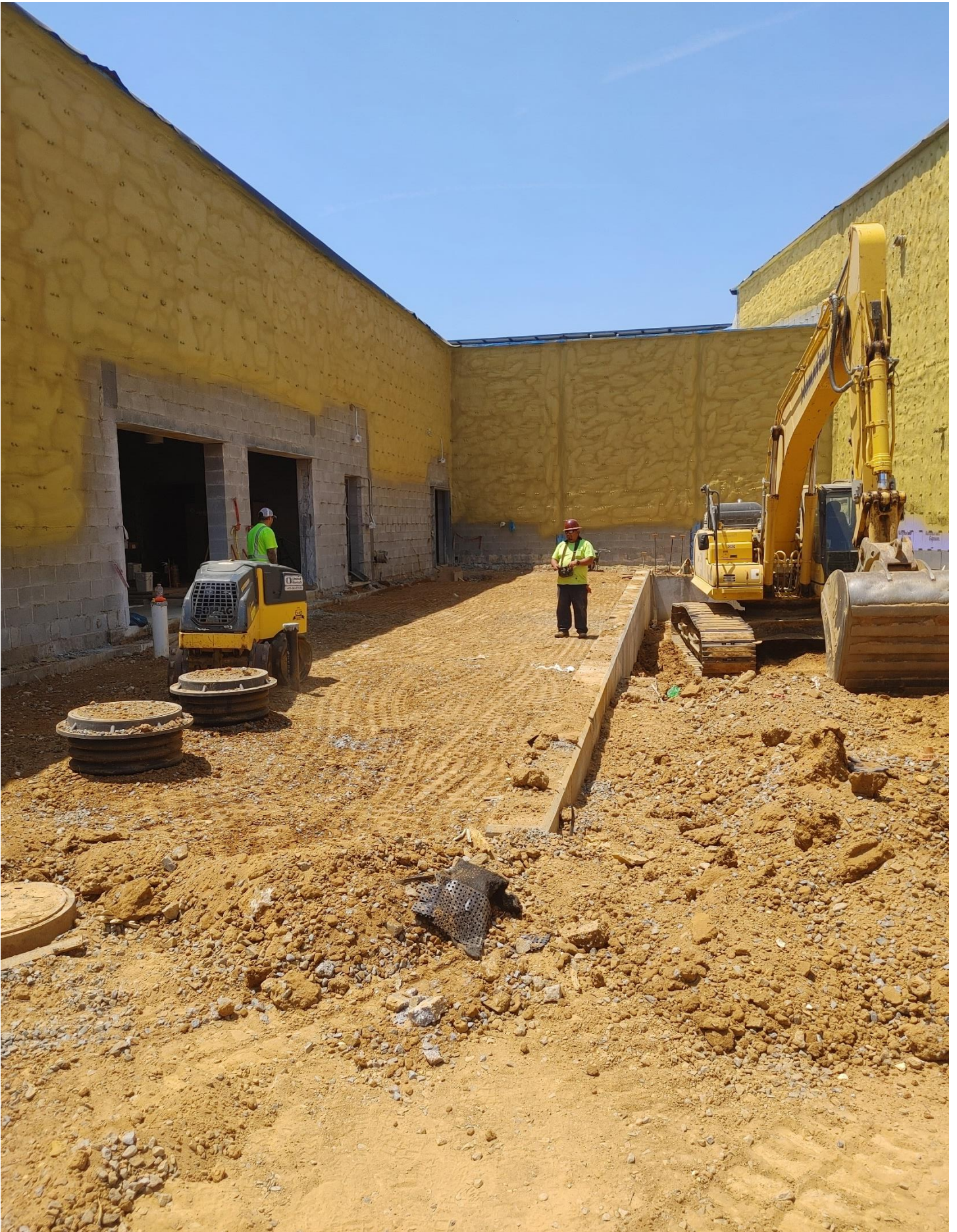
Photo 4 - Beuchert is compacting soils in the Loading Dock Area.
