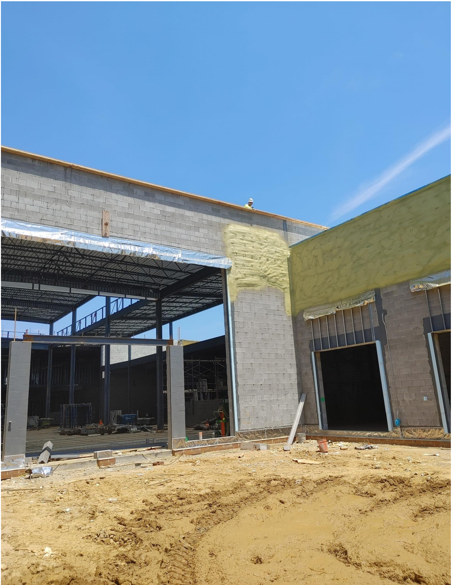
Photo 5 - the Cap of the Parapet wall is being constructed.
