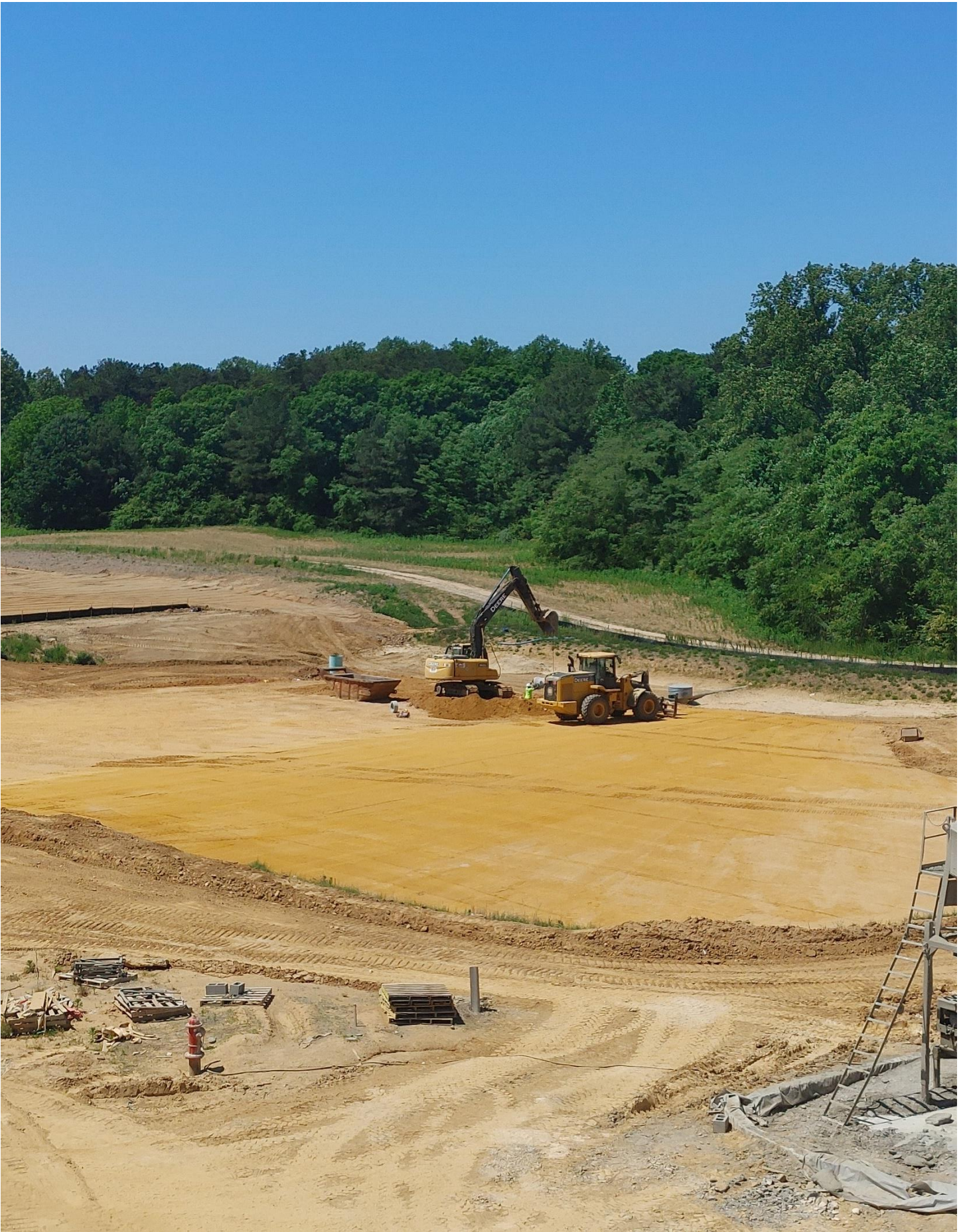
Photo 4 - Storm sewer pipe being laid on the West side of the site.
