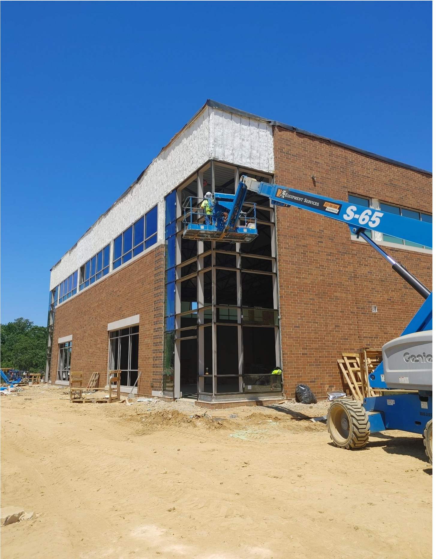
Photo 5 - Work continues on the Curtain walls of Area E
