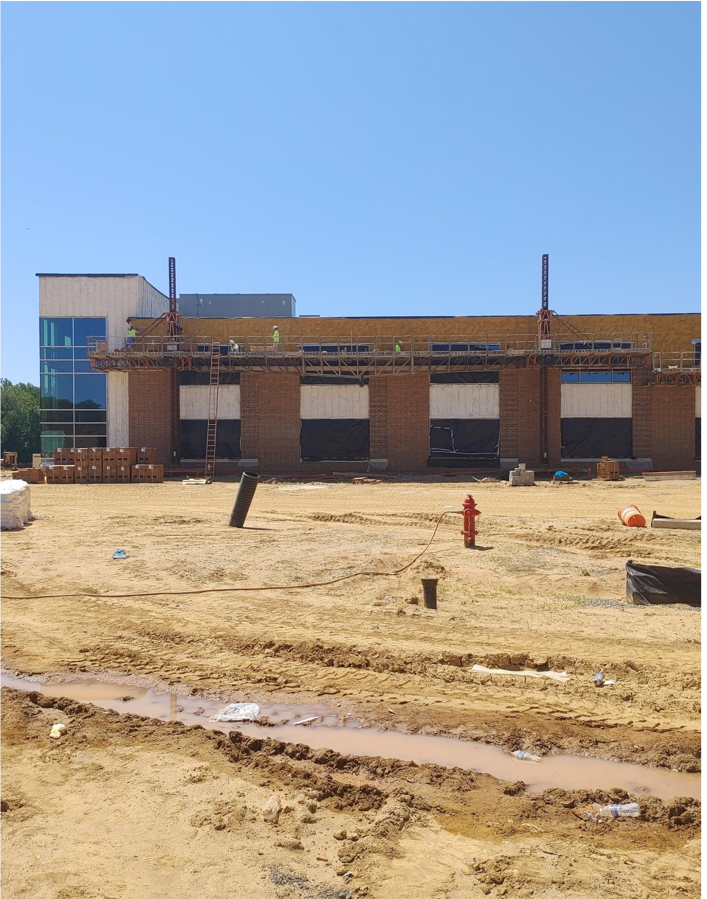
Photo 1 - Masons are laying brick on the North side of Area A
