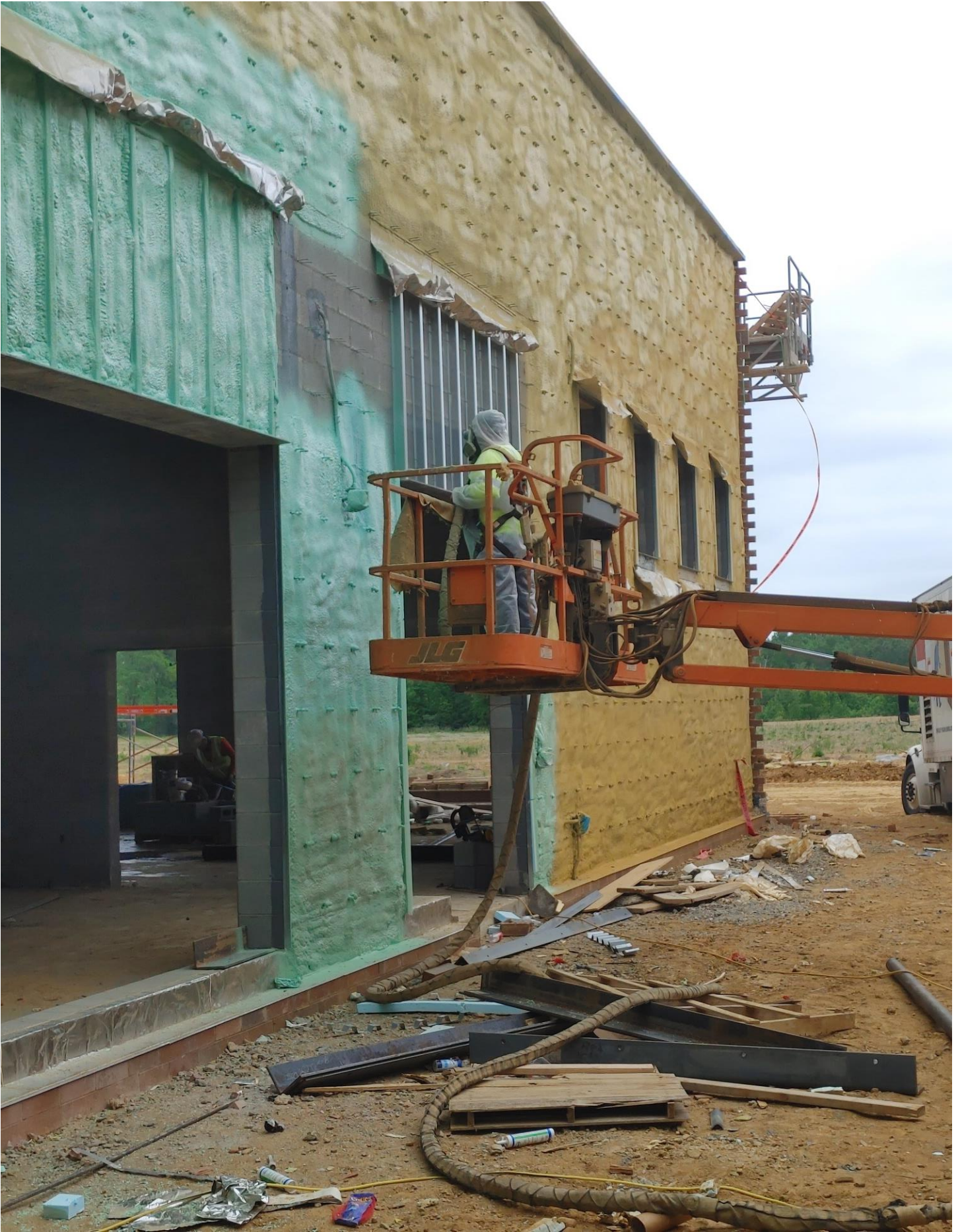
Photo 5 - Spray Foam being applied to the West wall of Area D
