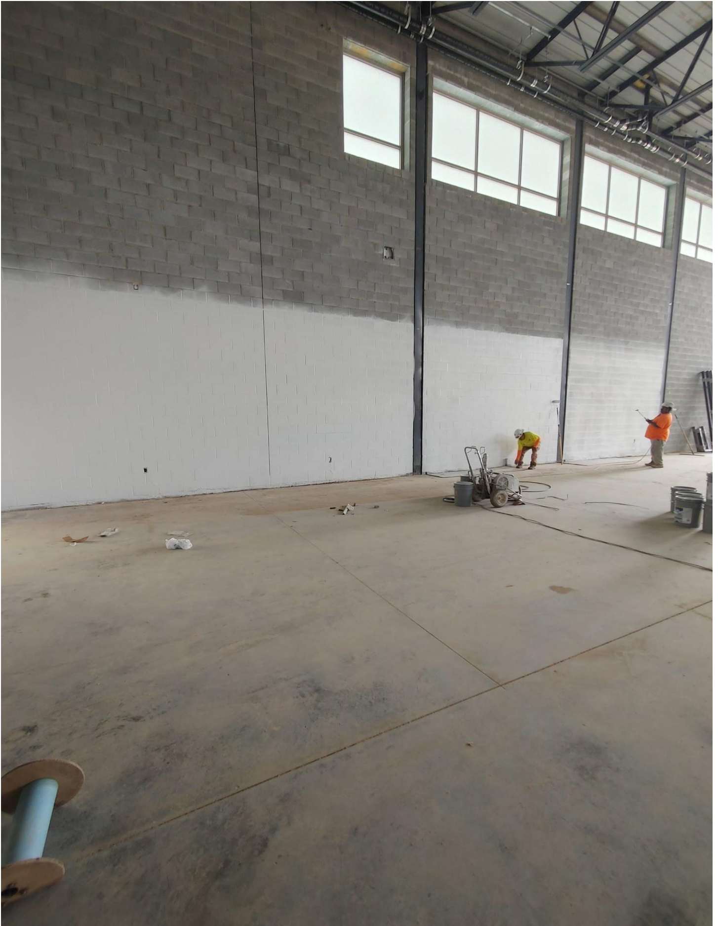
Photo 6 - Block filler & Sealer being sprayed and rolled in the Gym.
