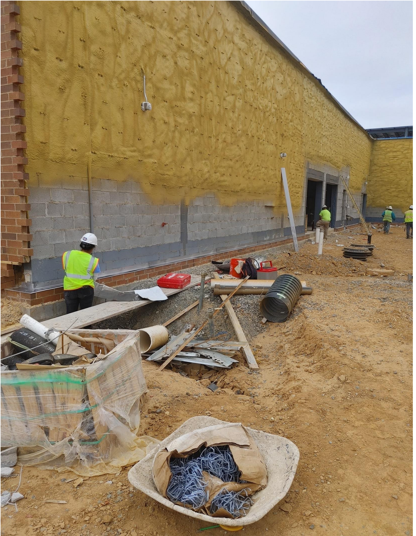
Photo 3 - Flashing being installed on the North side of Area D
