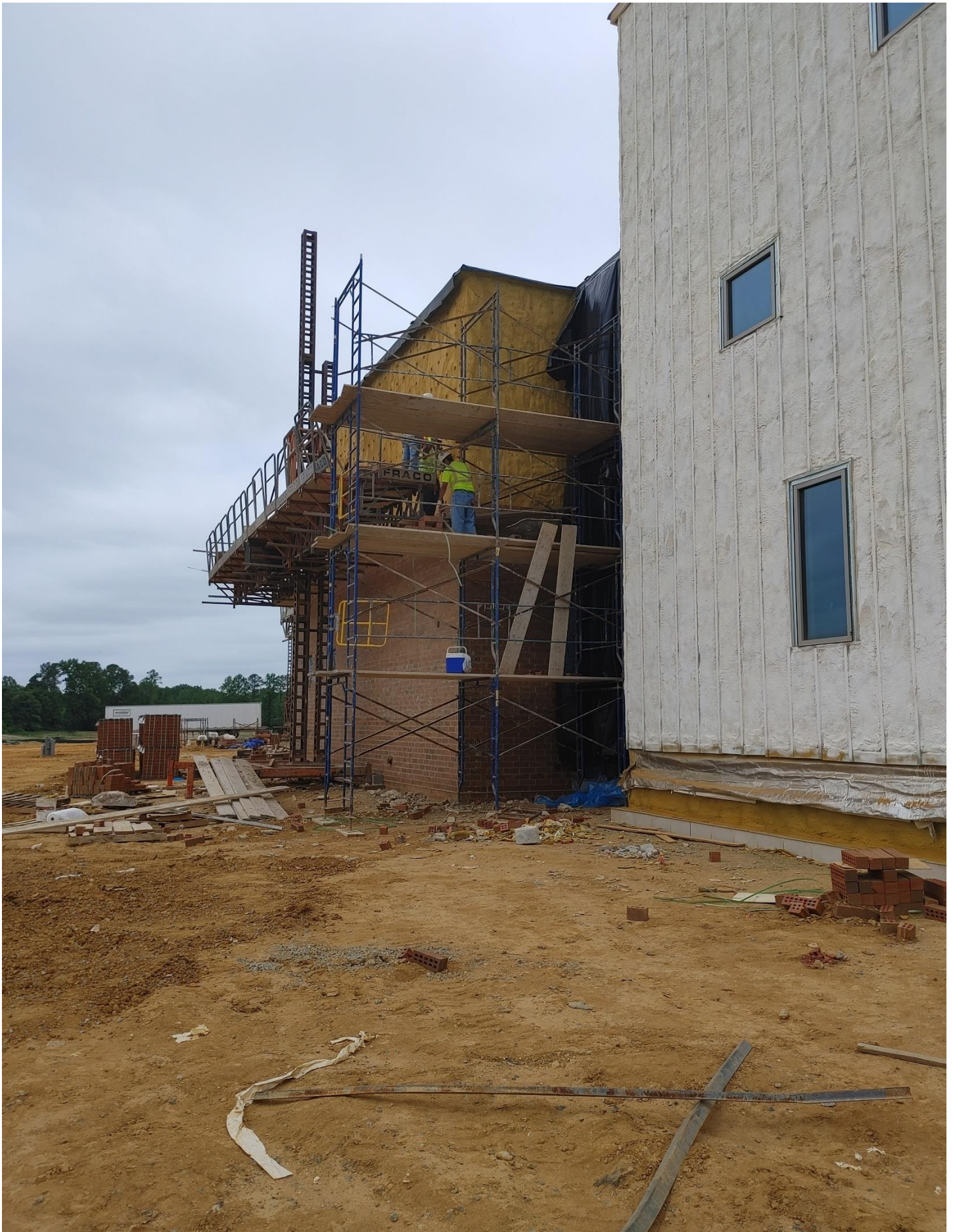
Photo 2 - Brick being laid on the East side of Area A
