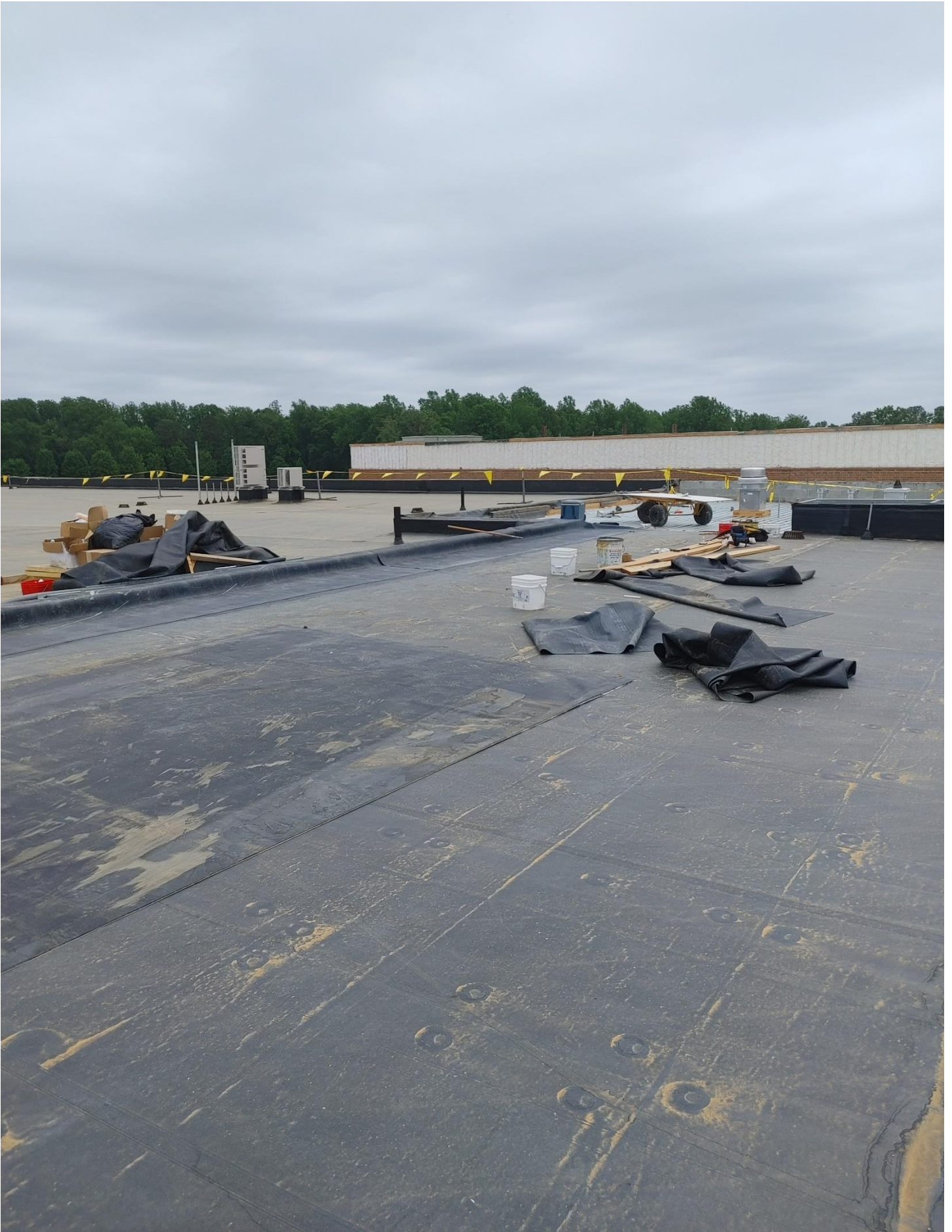
Photo 10 - Roofer working on Parapet wall on the roof of Area A
