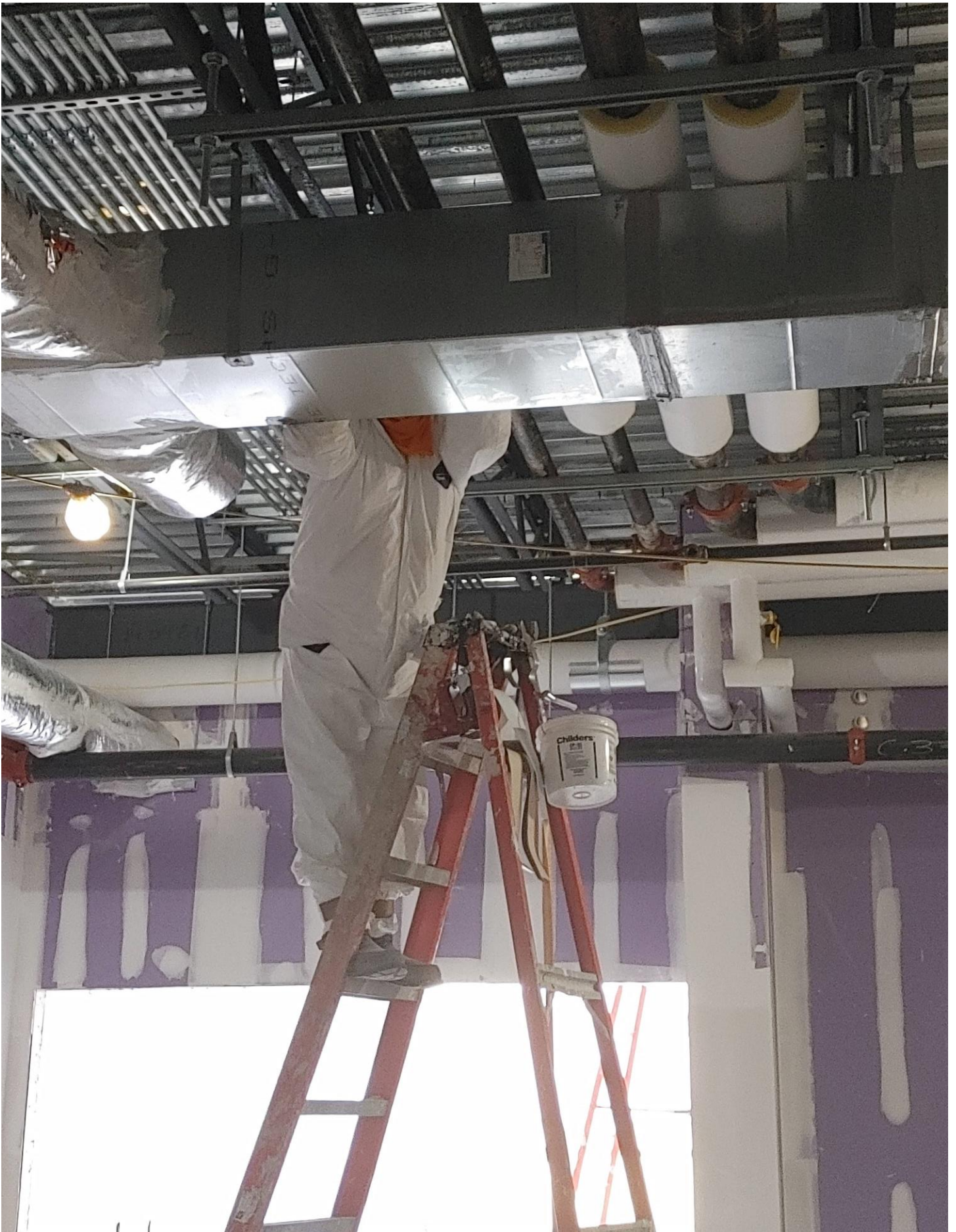
Photo 9 - HVAC Duct being insulated in Area A
