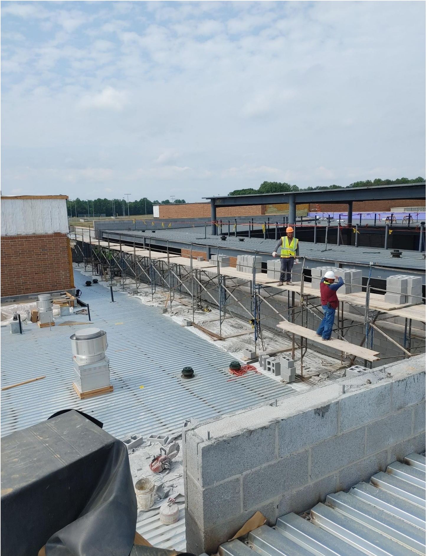
Photo 7 - Block being laid on the Parapet wall in Area C.
