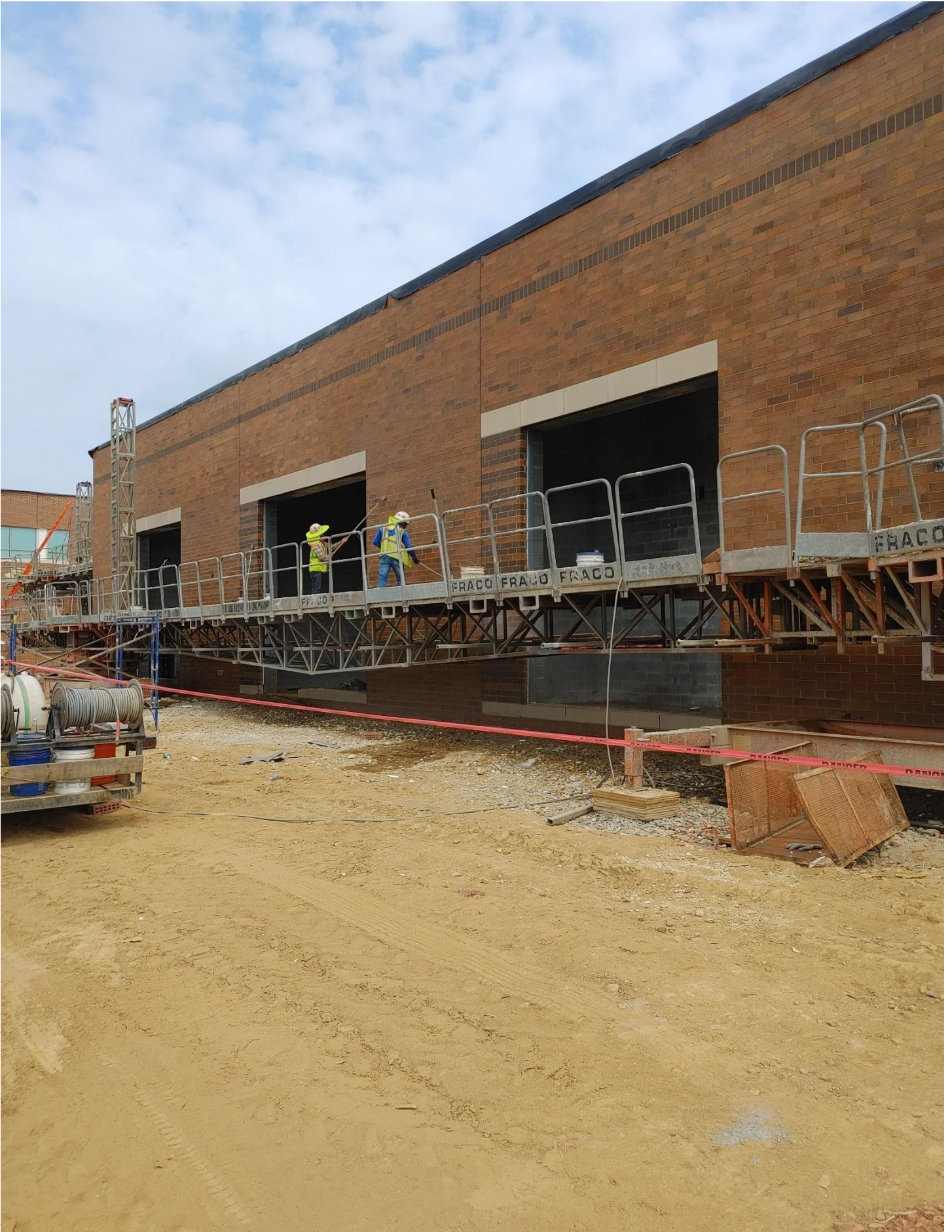
Photo 8 - Brick is being washed on the South side of Area D.
