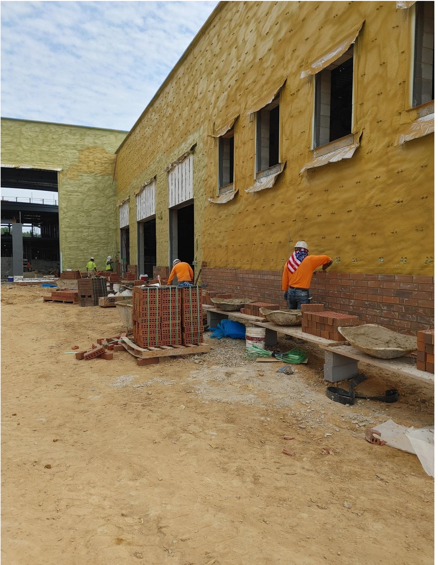
Photo 9 - Brick is being laid on the West side of Area D.
