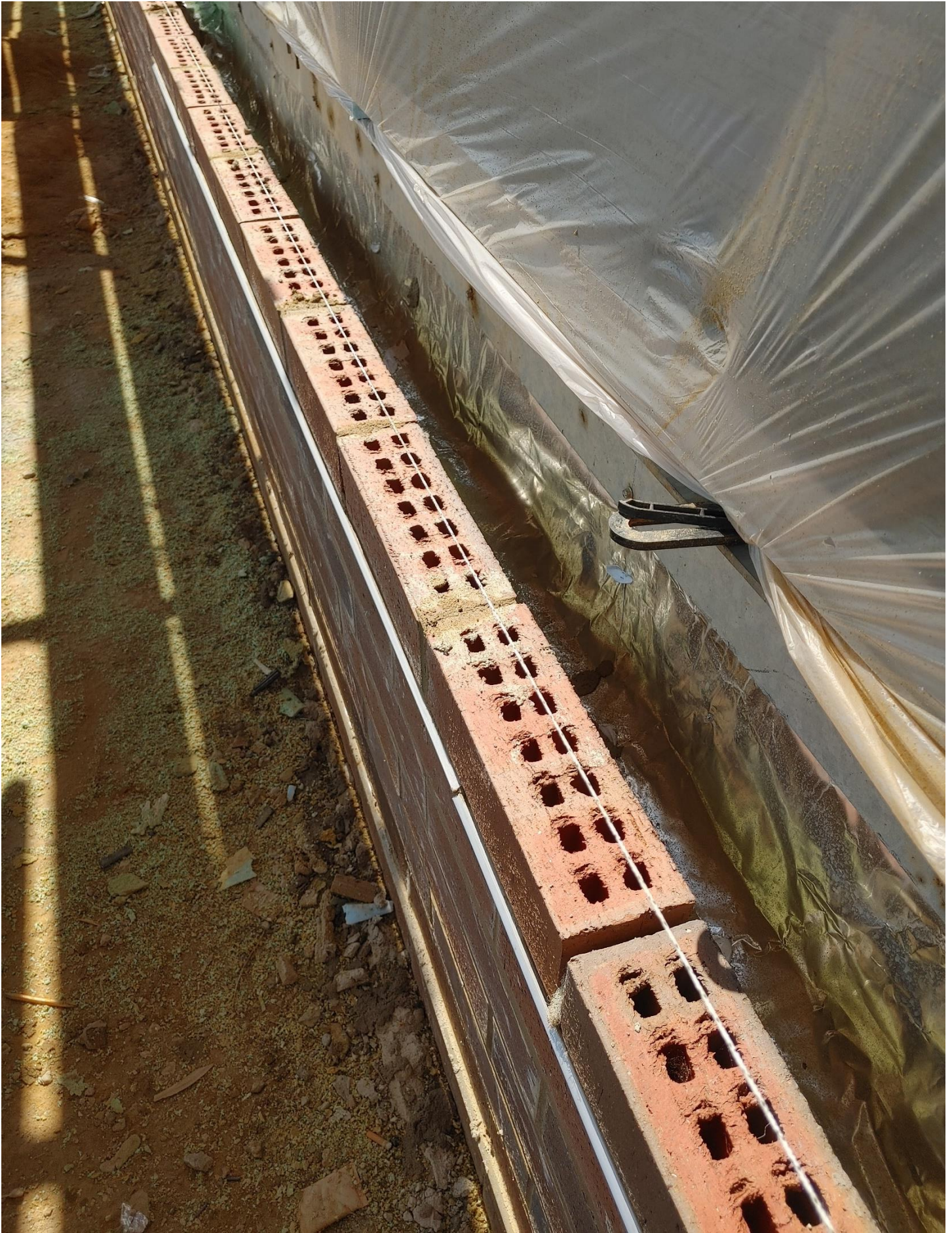
Photo 3 - Flashing installed on the North side of Area B.
