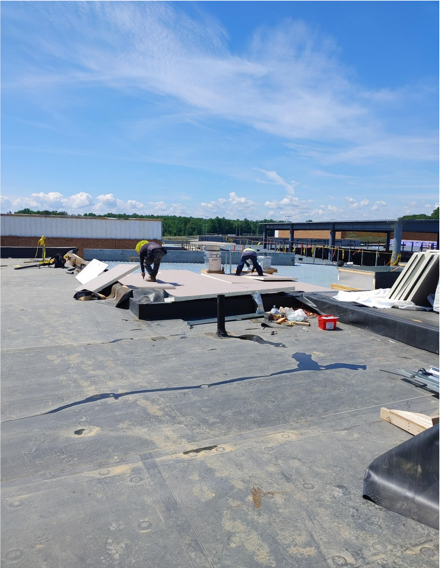
Photo 3 - Roofers are working on a section of Area A.
