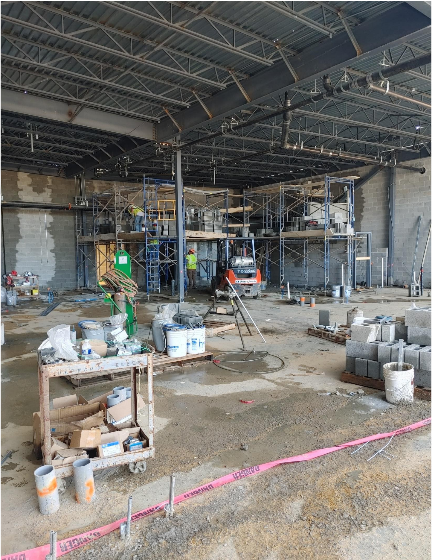
Photo 2 - Block is being laid in the Kitchen Area.
