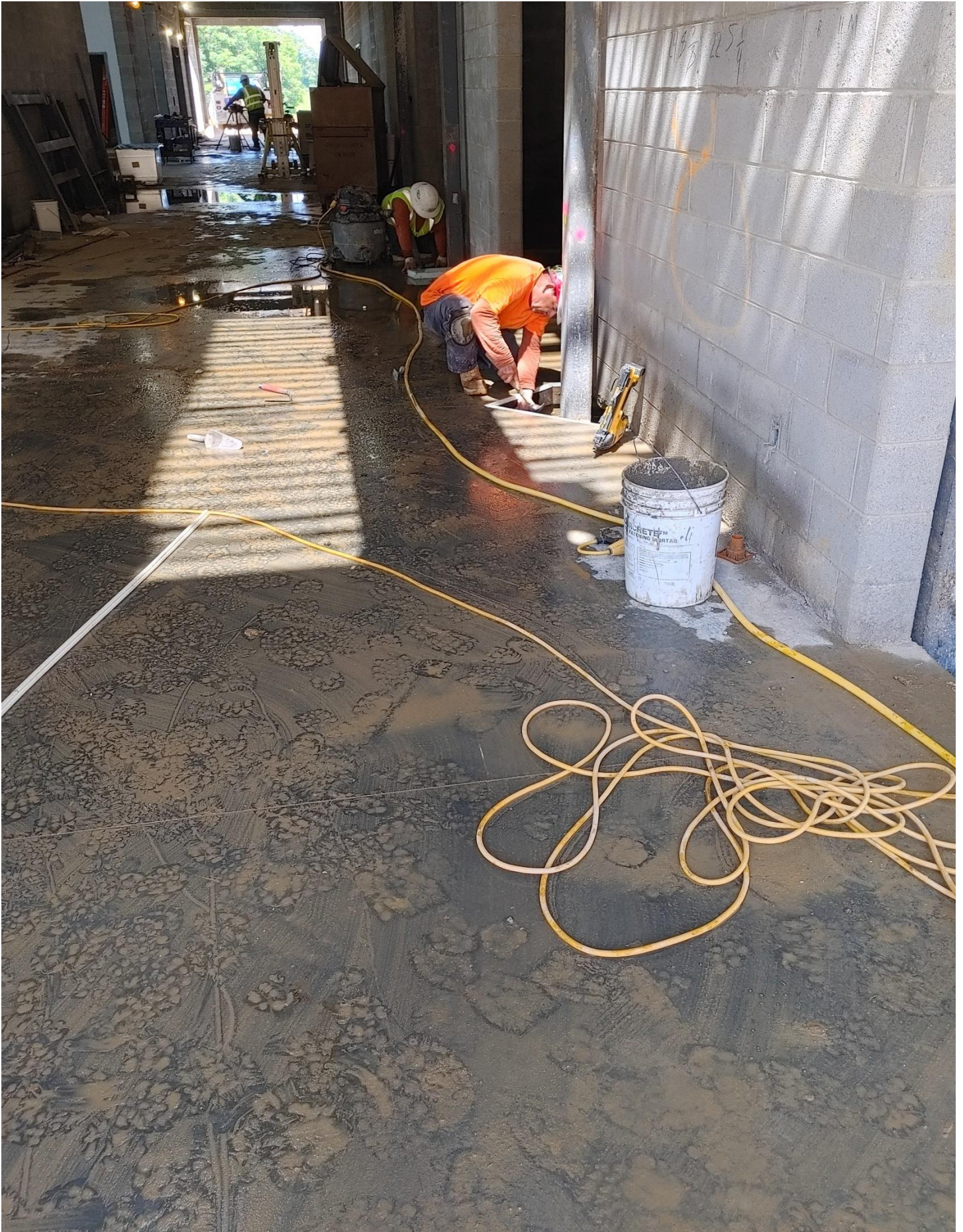
Photo 7 - Diamonds are be prepped for concrete.
