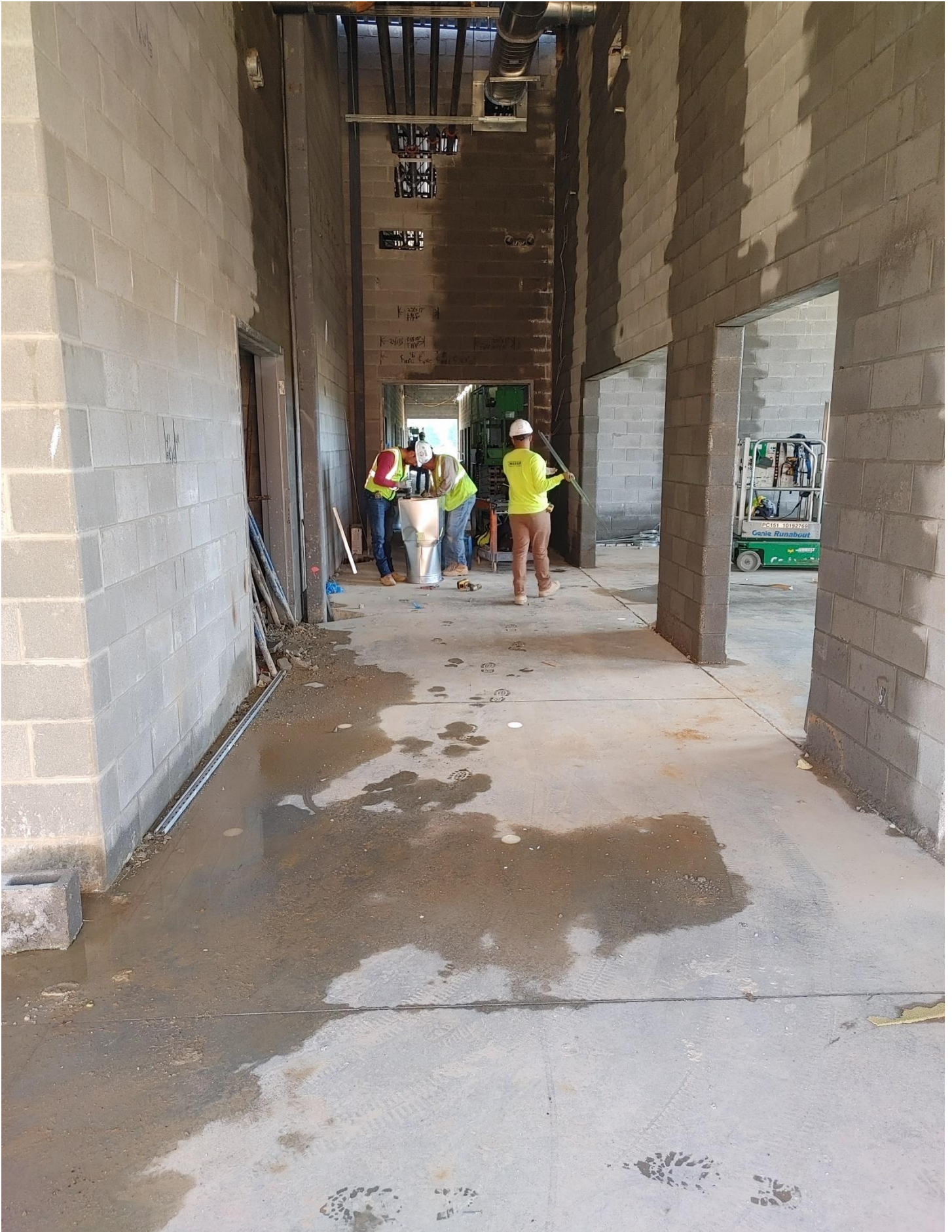
Photo 8 - HVAC duct is being run in Corridor D12
