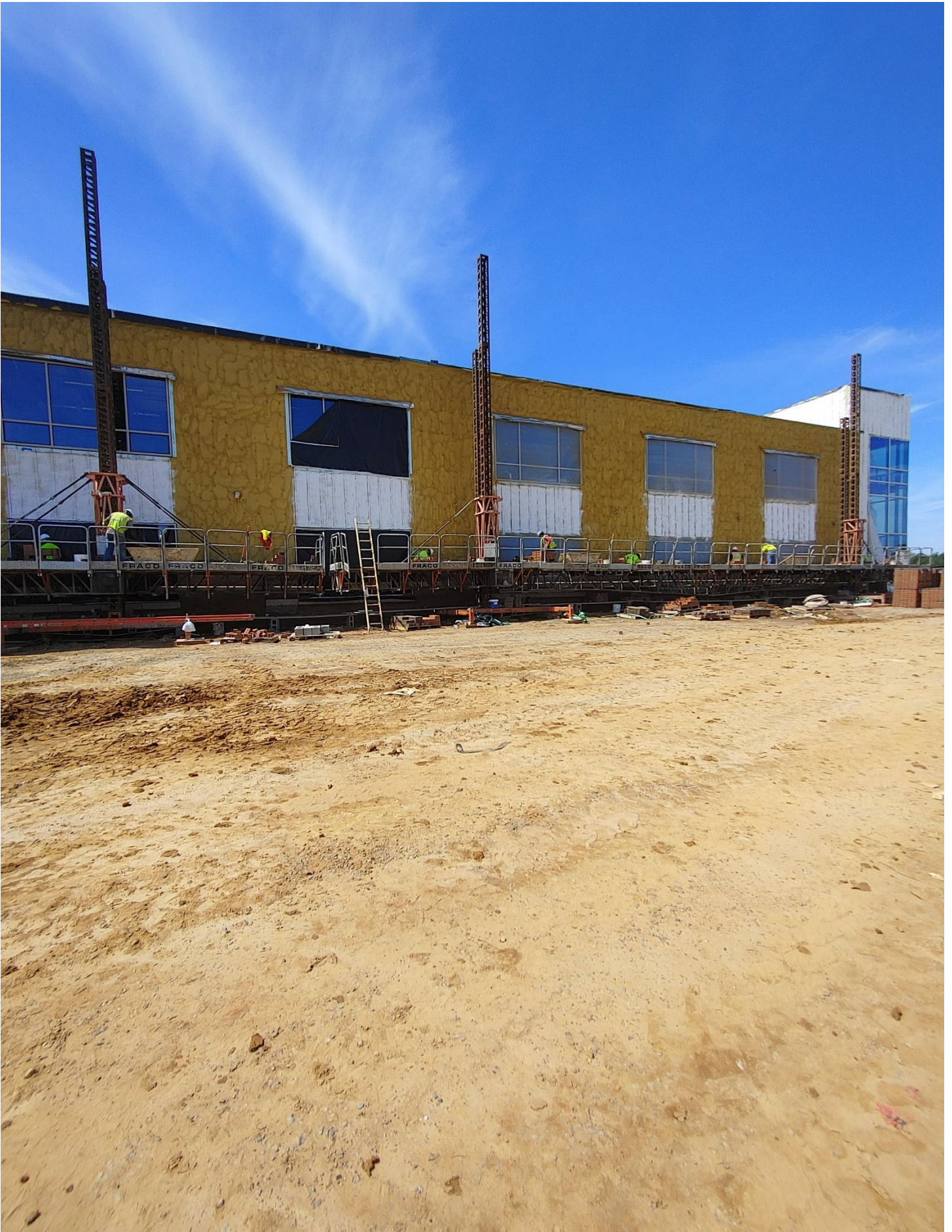
Photo 1 - Brick is being laid on the North side of Area B.
