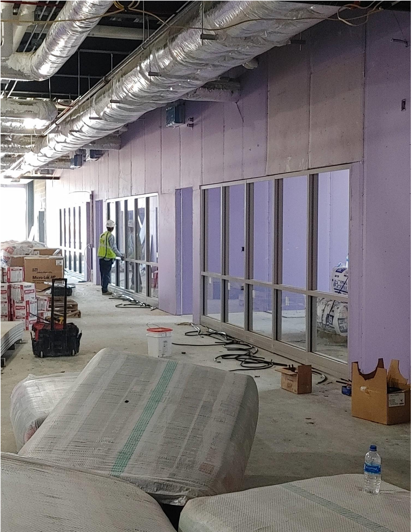
Photo 6 - Glass and backer rod is being installed in Area B.
