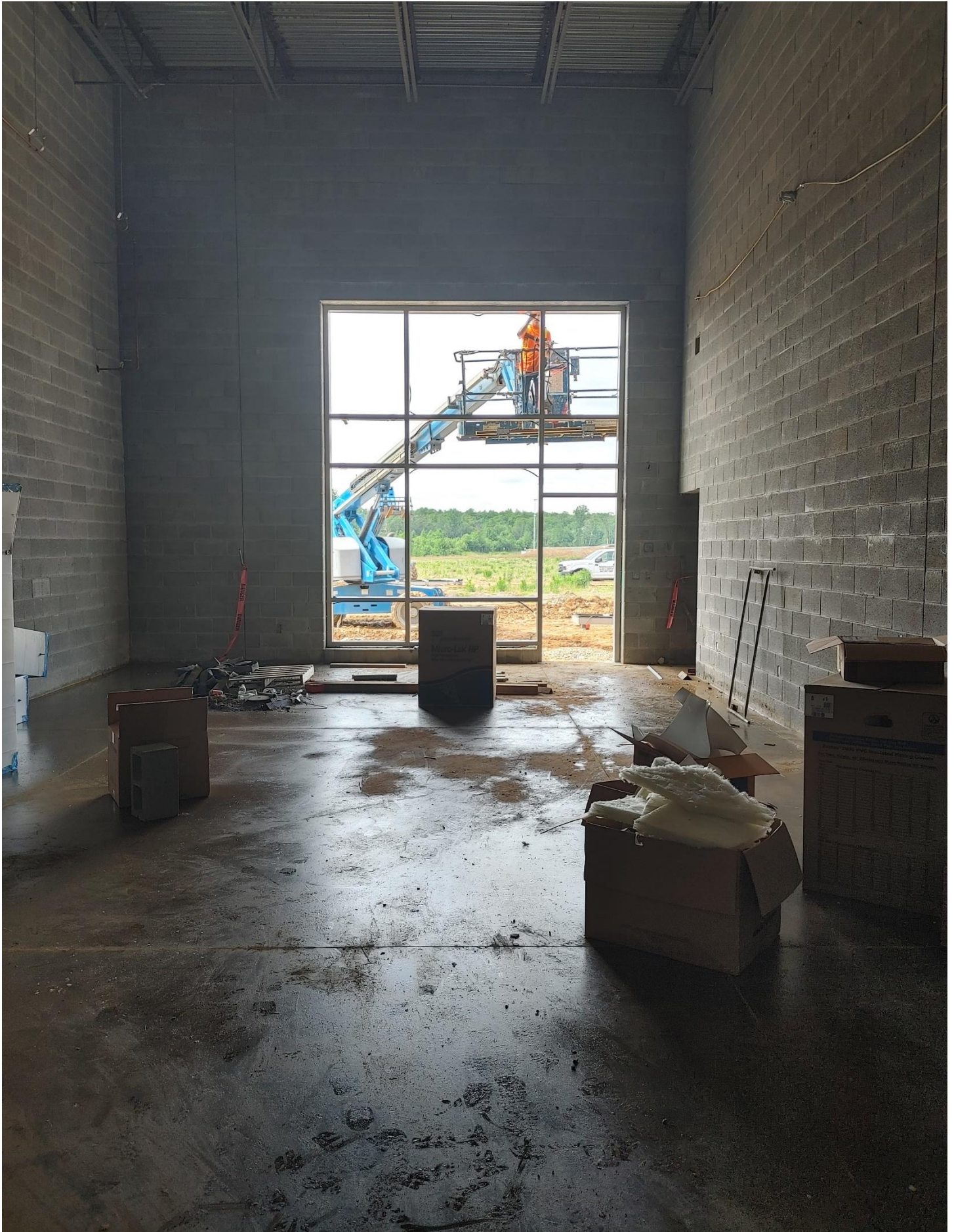
Photo 9 - Storefront frames being installed in Area D.
