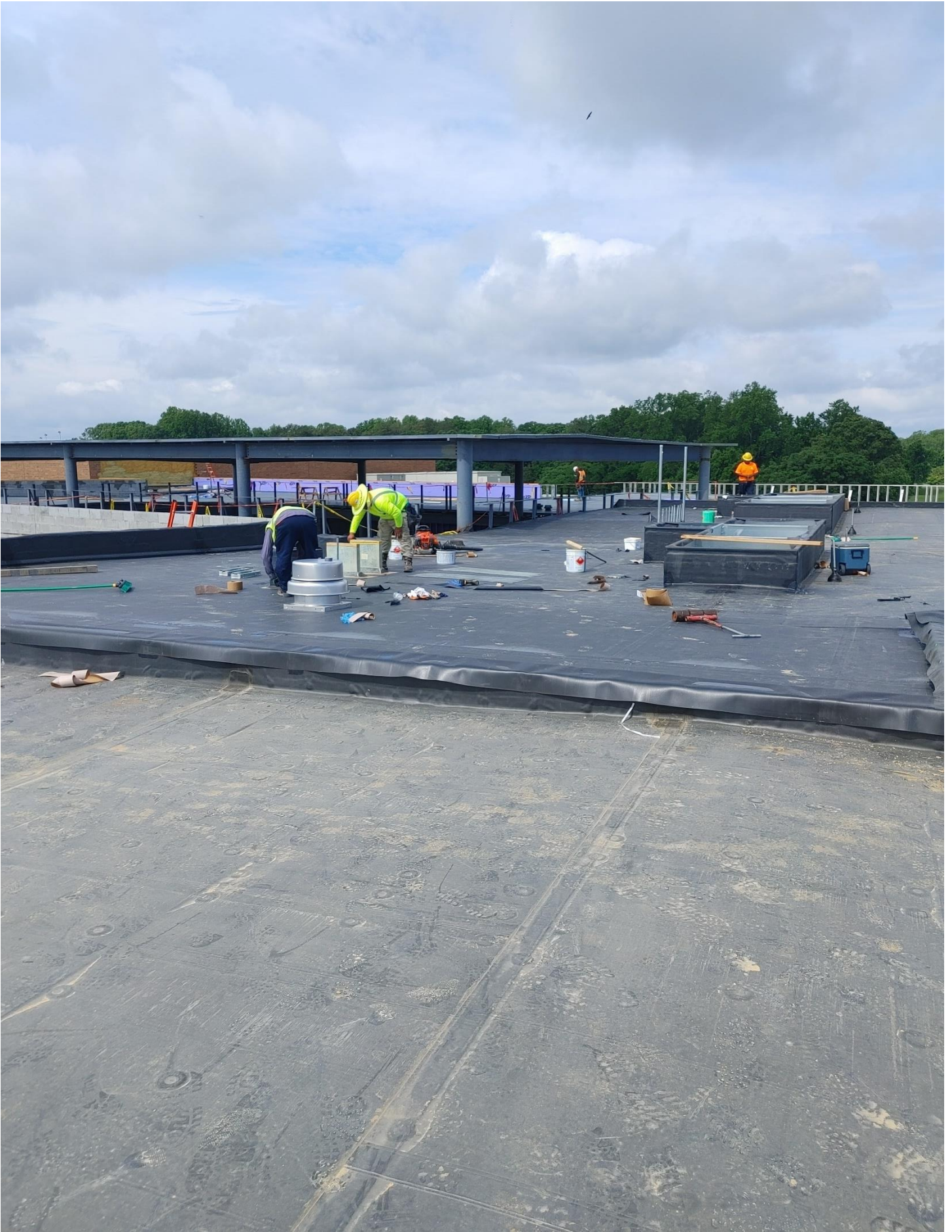
Photo 1 – Roofers are working on Area A's roof.
