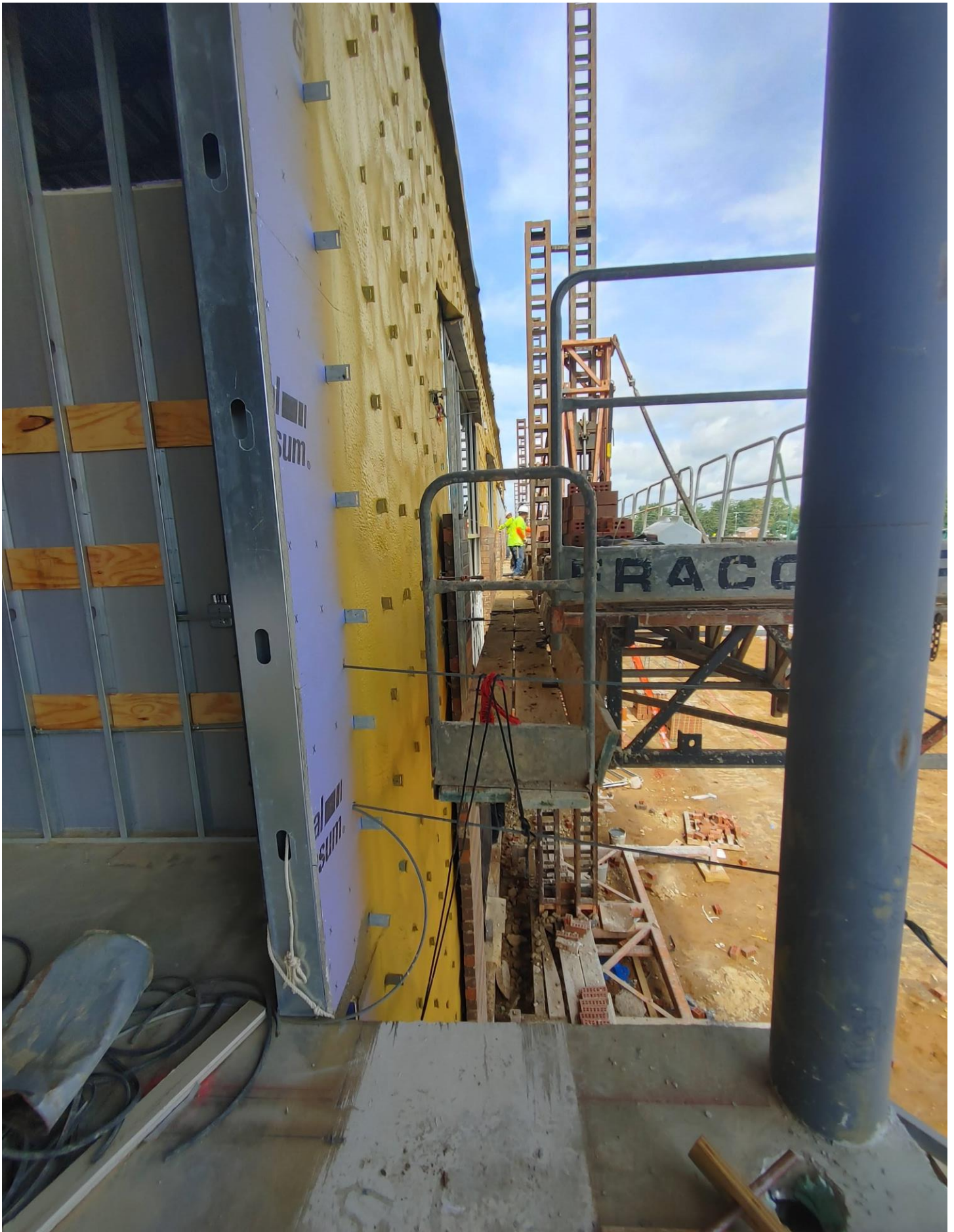
Photo 4 - Masons are laying Brick on the North side of Area B.
