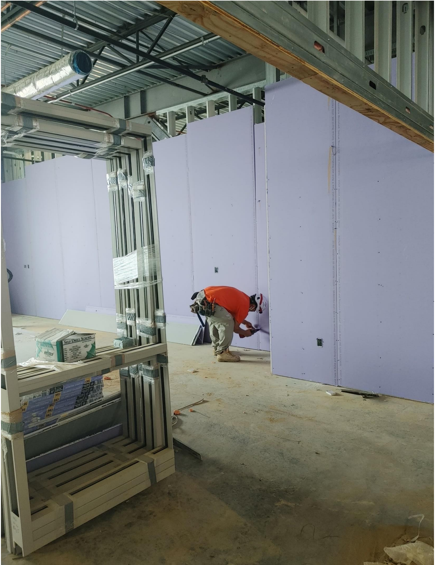
Photo 6 - Sheetrock is being installed in Area B.
