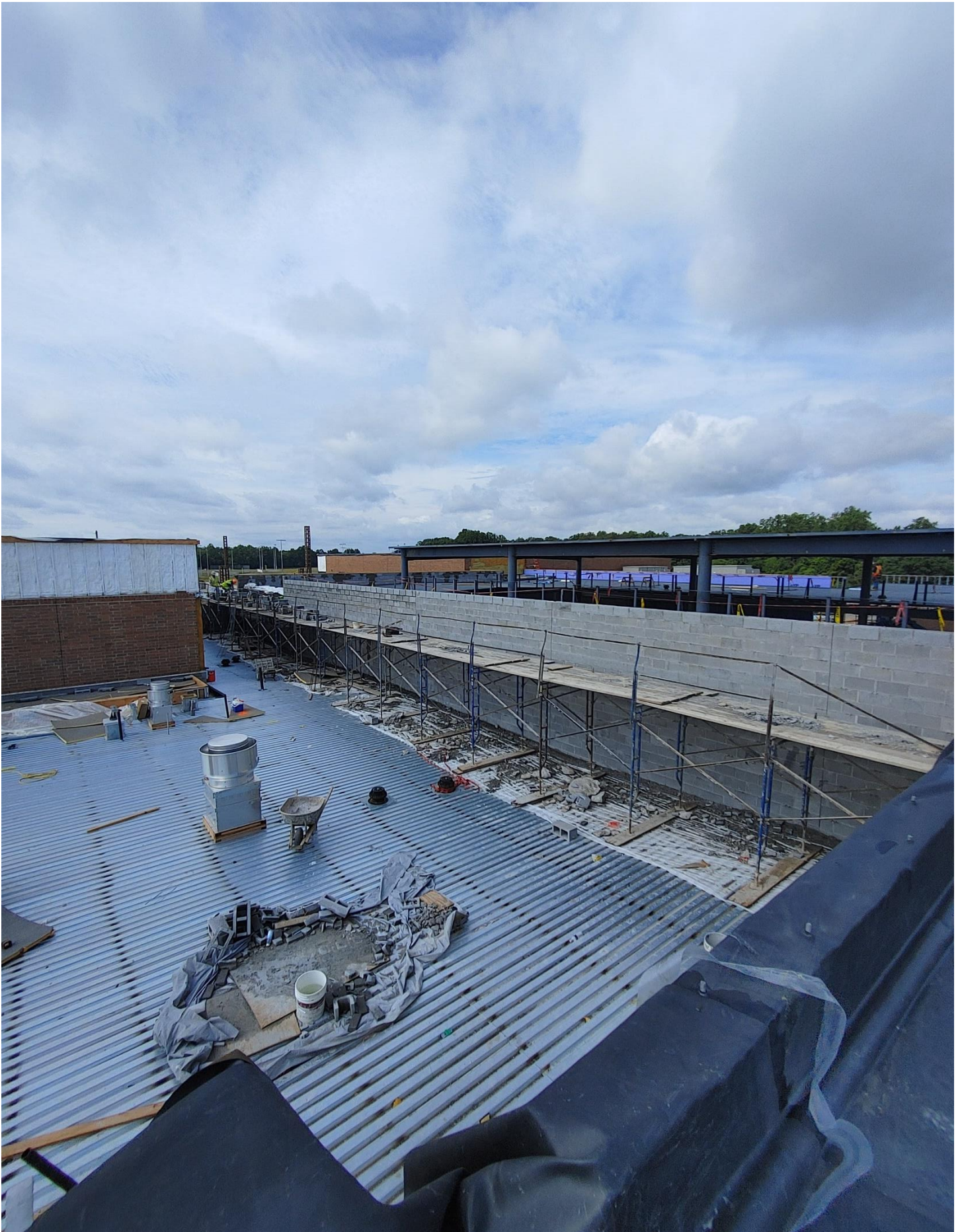
Photo 2 - Masons are laying block between Area D and C.
