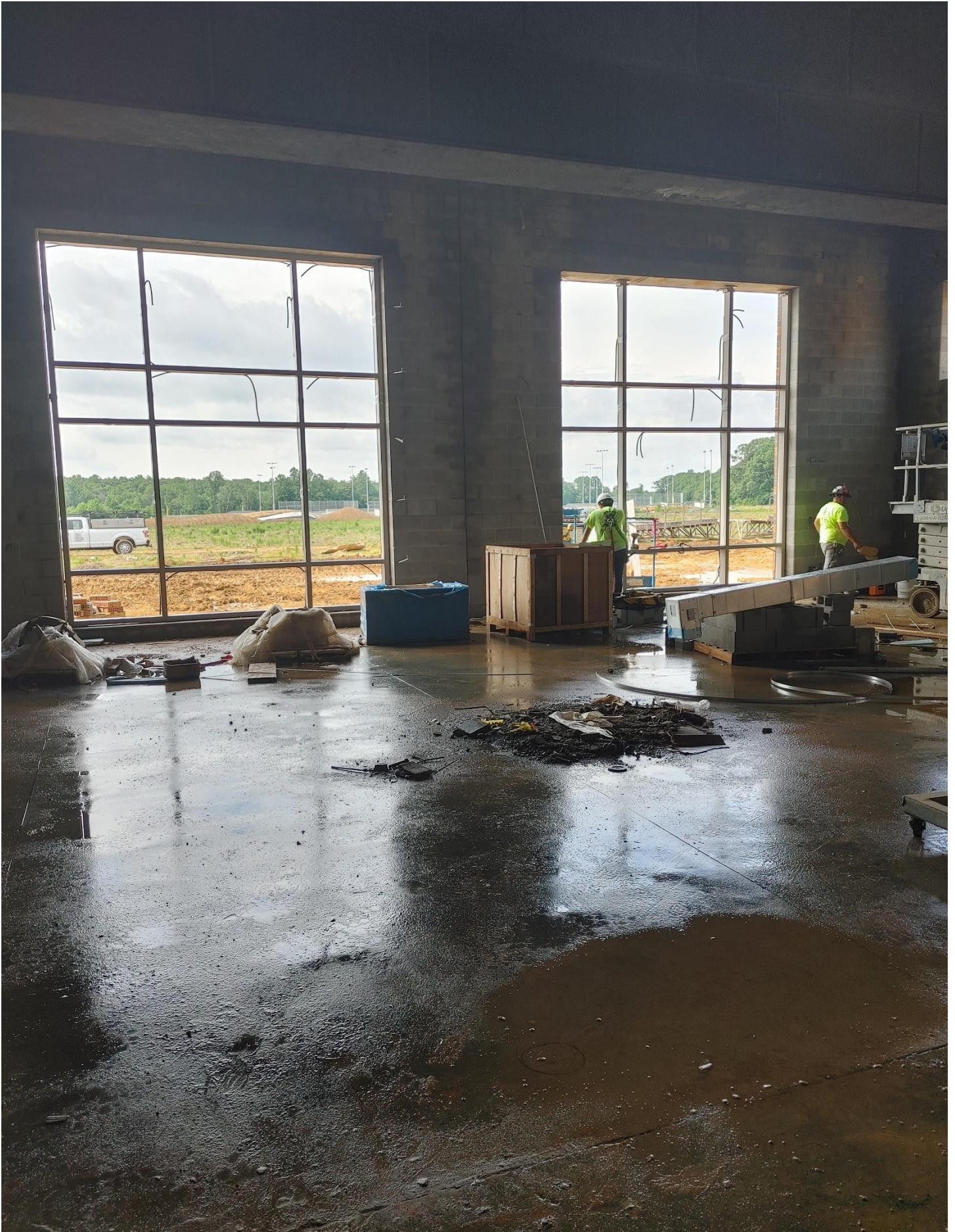
Photo 10 - Storefront frames are being installed in Area D.
