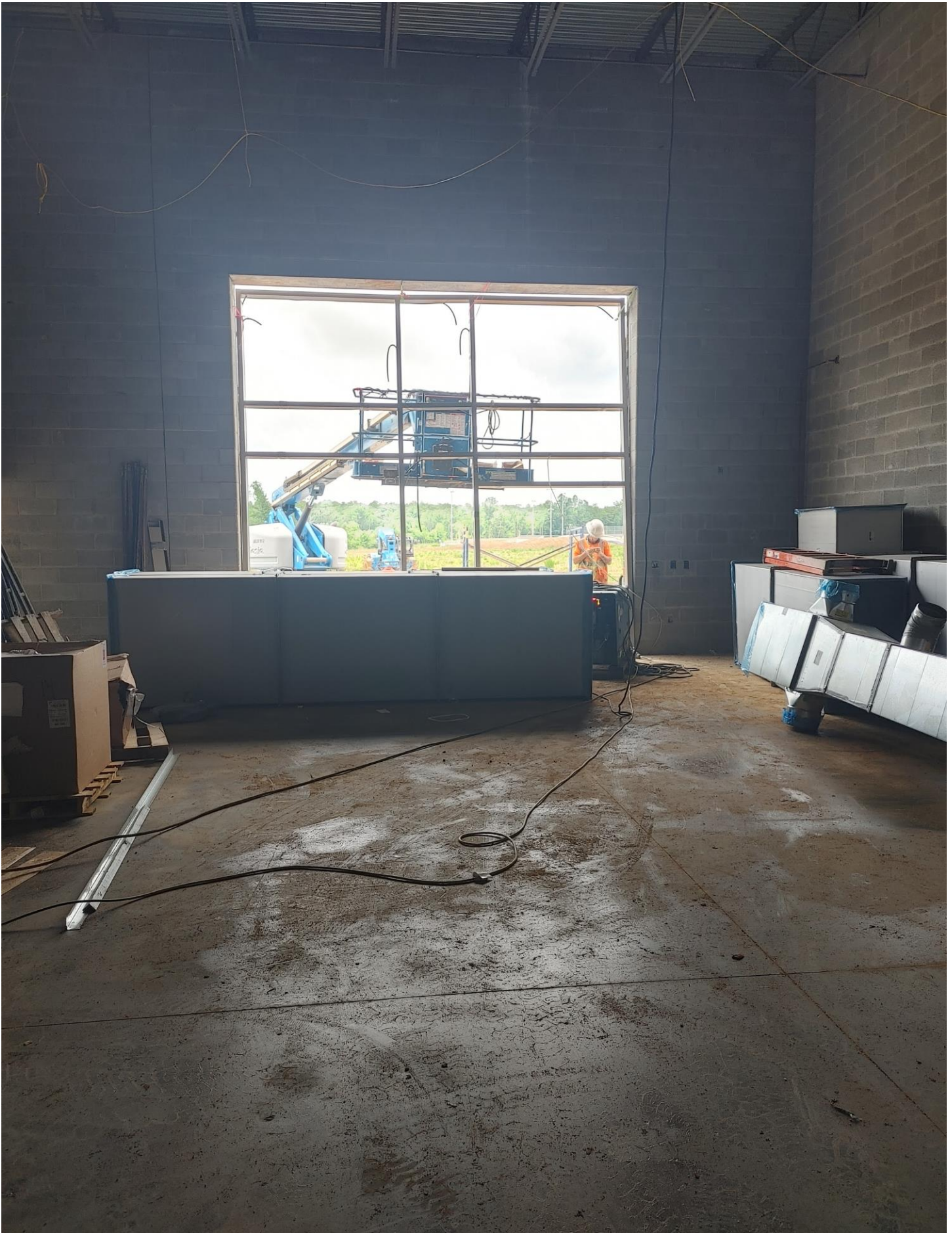
Photo 5 - Storefront being set on the South side of Area D.
