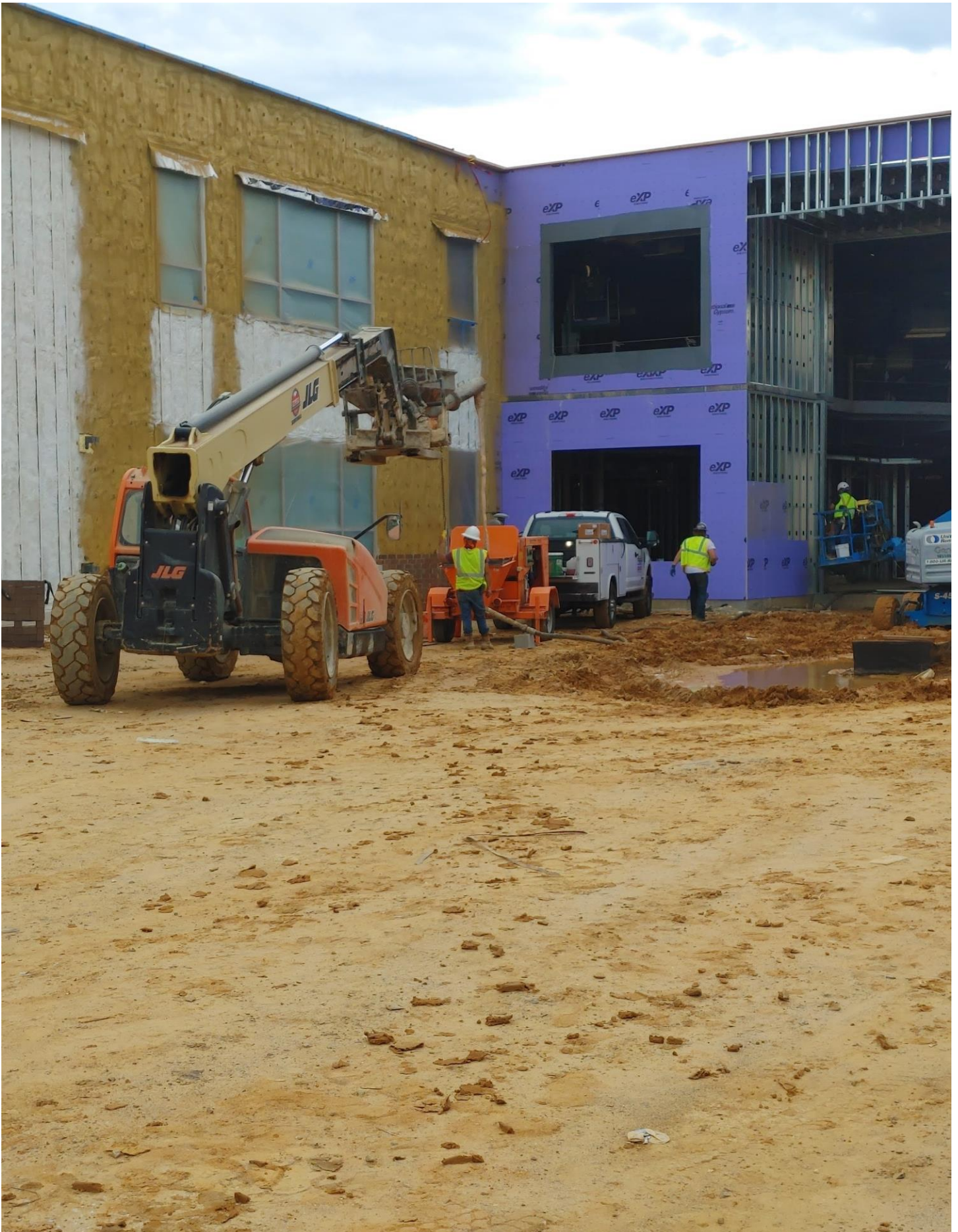
Photo 10 - The Masons are grouting block in Area C.
