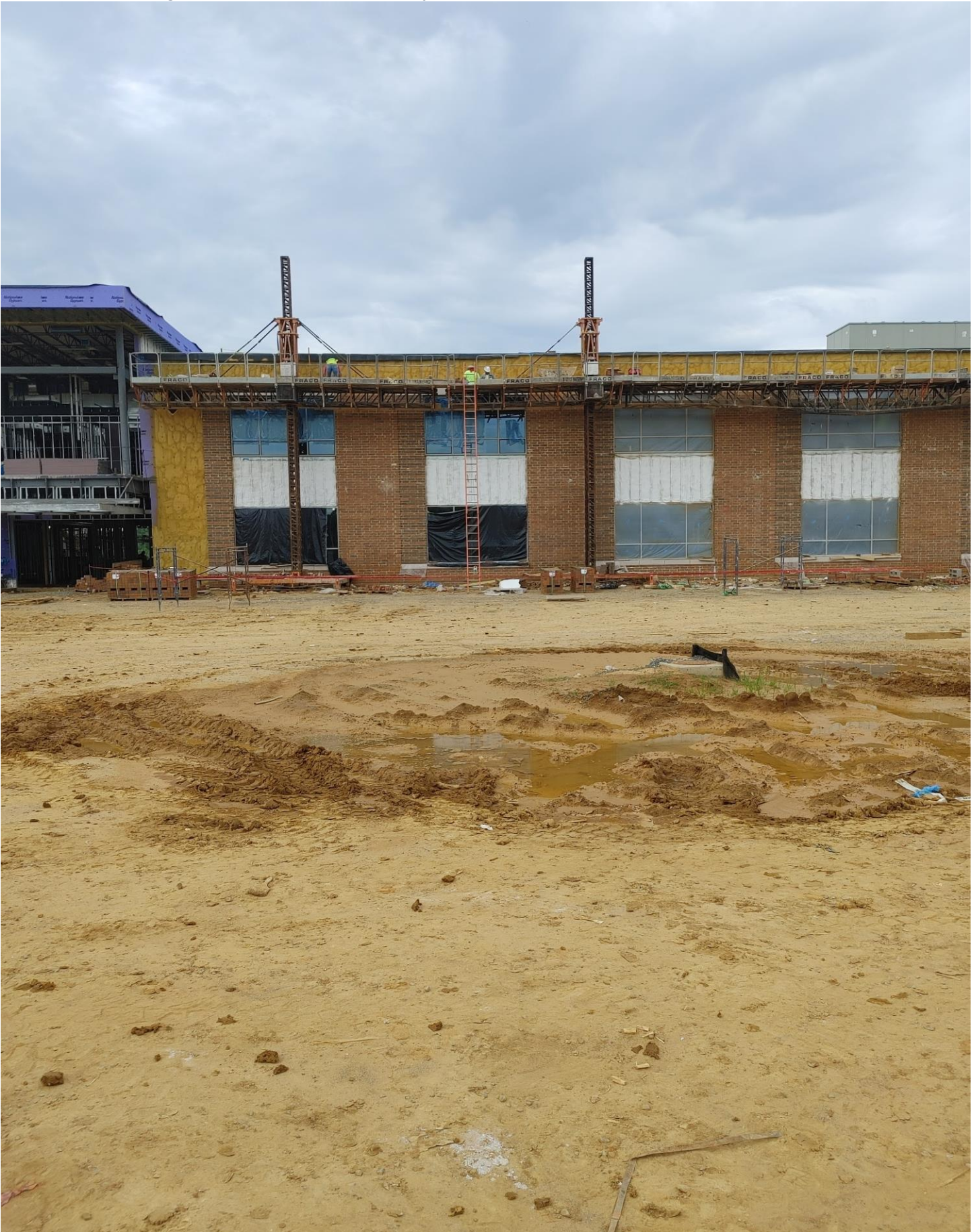
Photo 12 - Brick is being laid on the North side of Area B.
