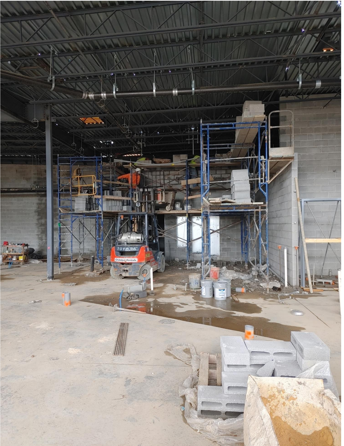
Photo 7 - Block continues to be laid in the Kitchen.
