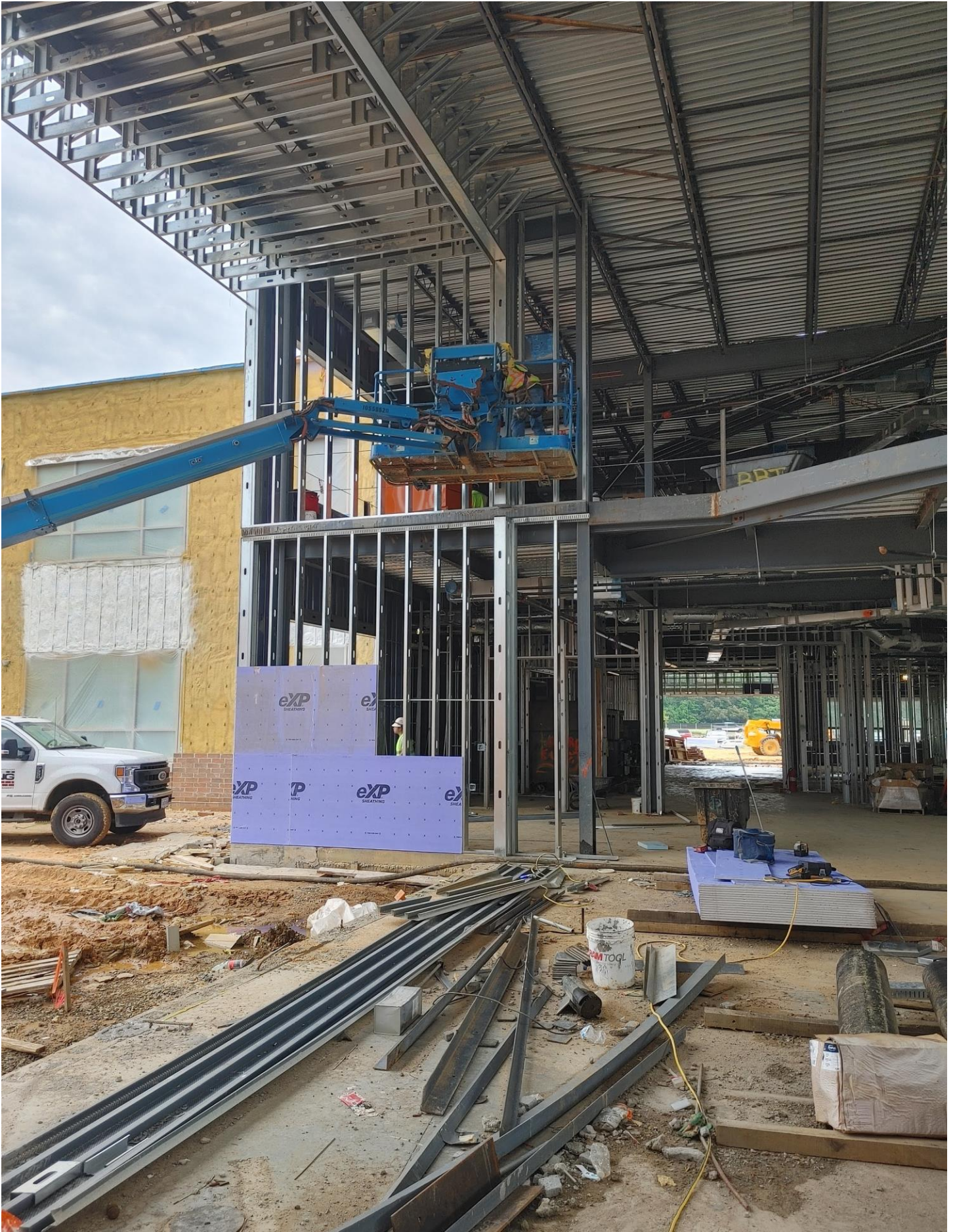
Photo 4 - Walls being framed in Area C.
