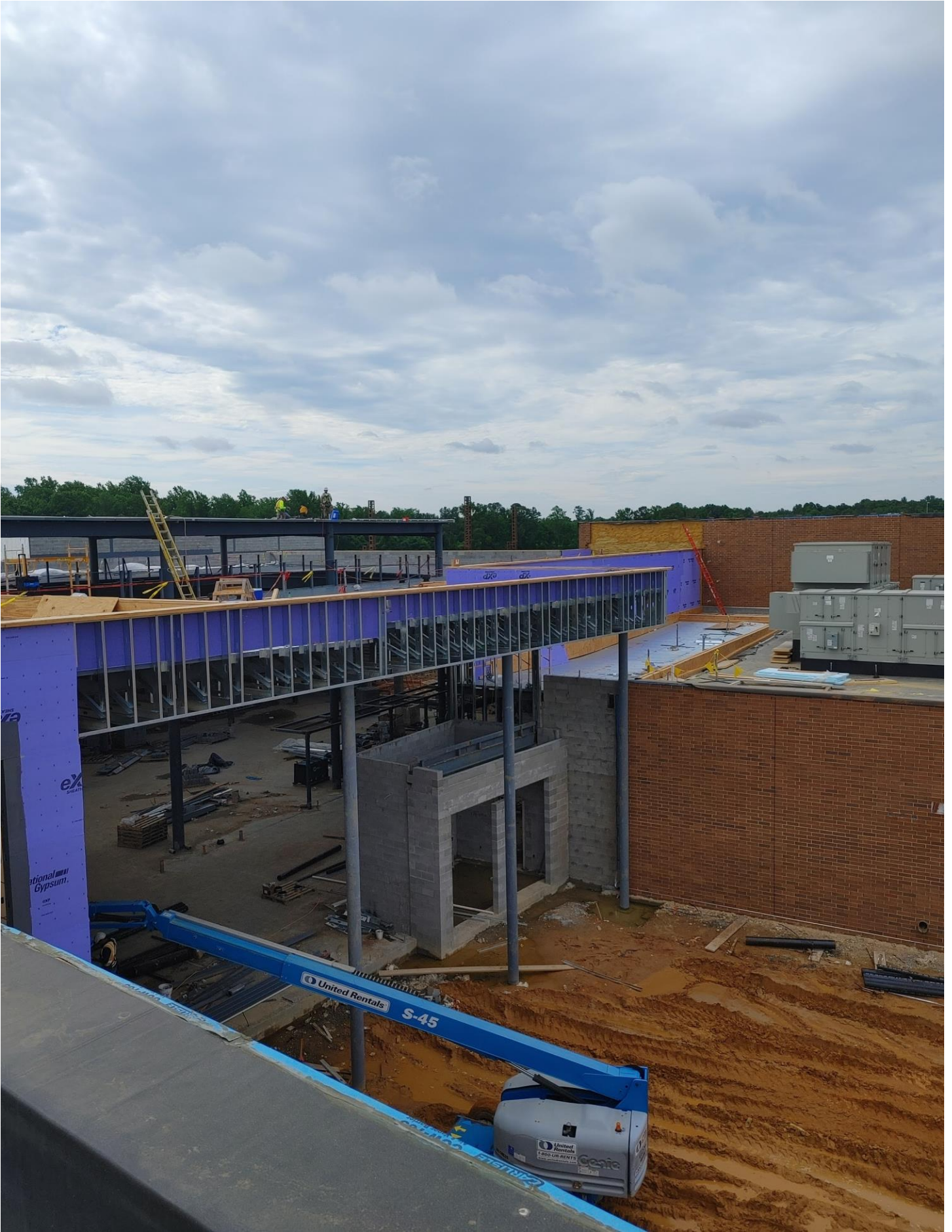
Photo 3 - Parapet Walls are being constructed
