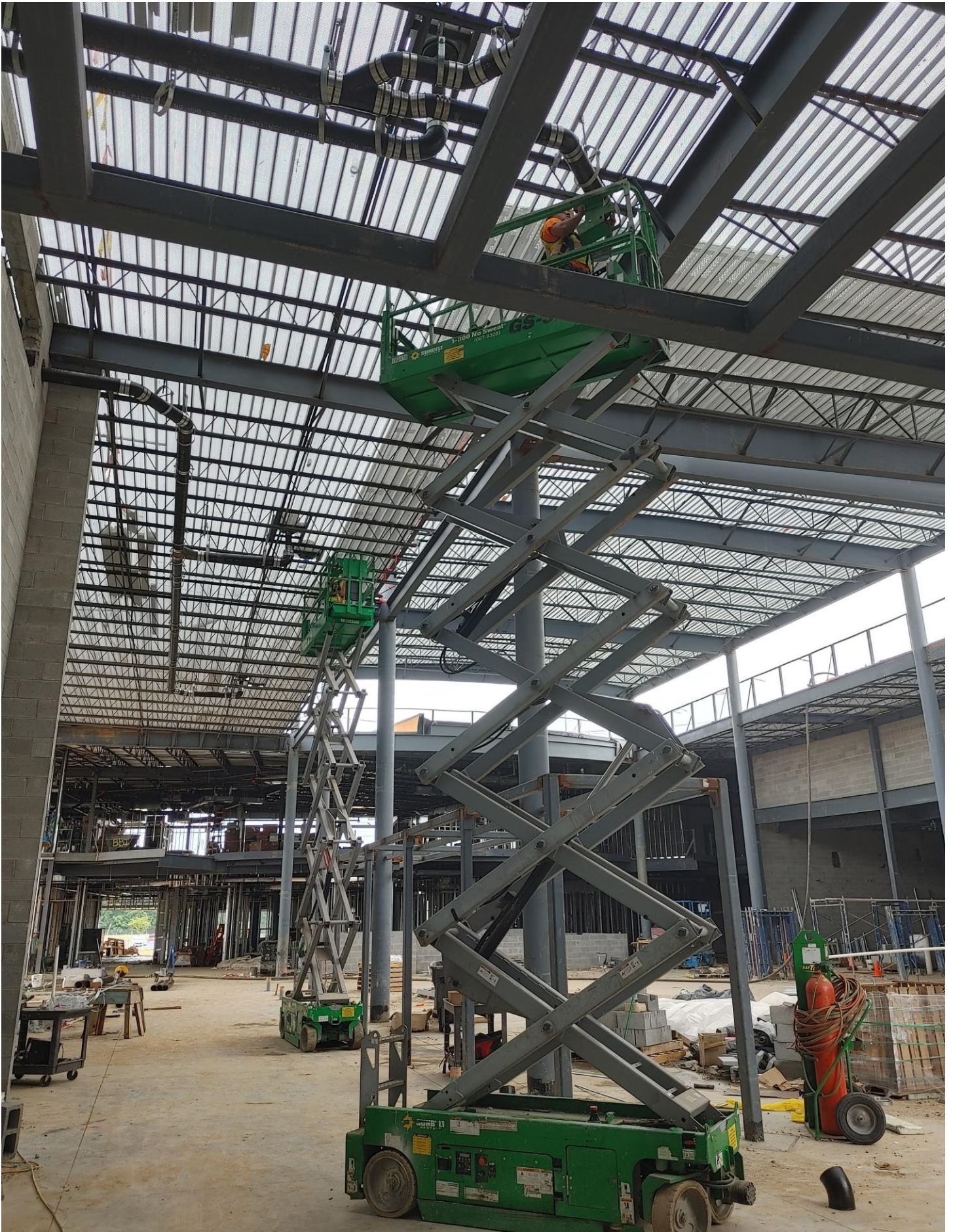
Photo 6 - Roof Drains being installed in Area C.
