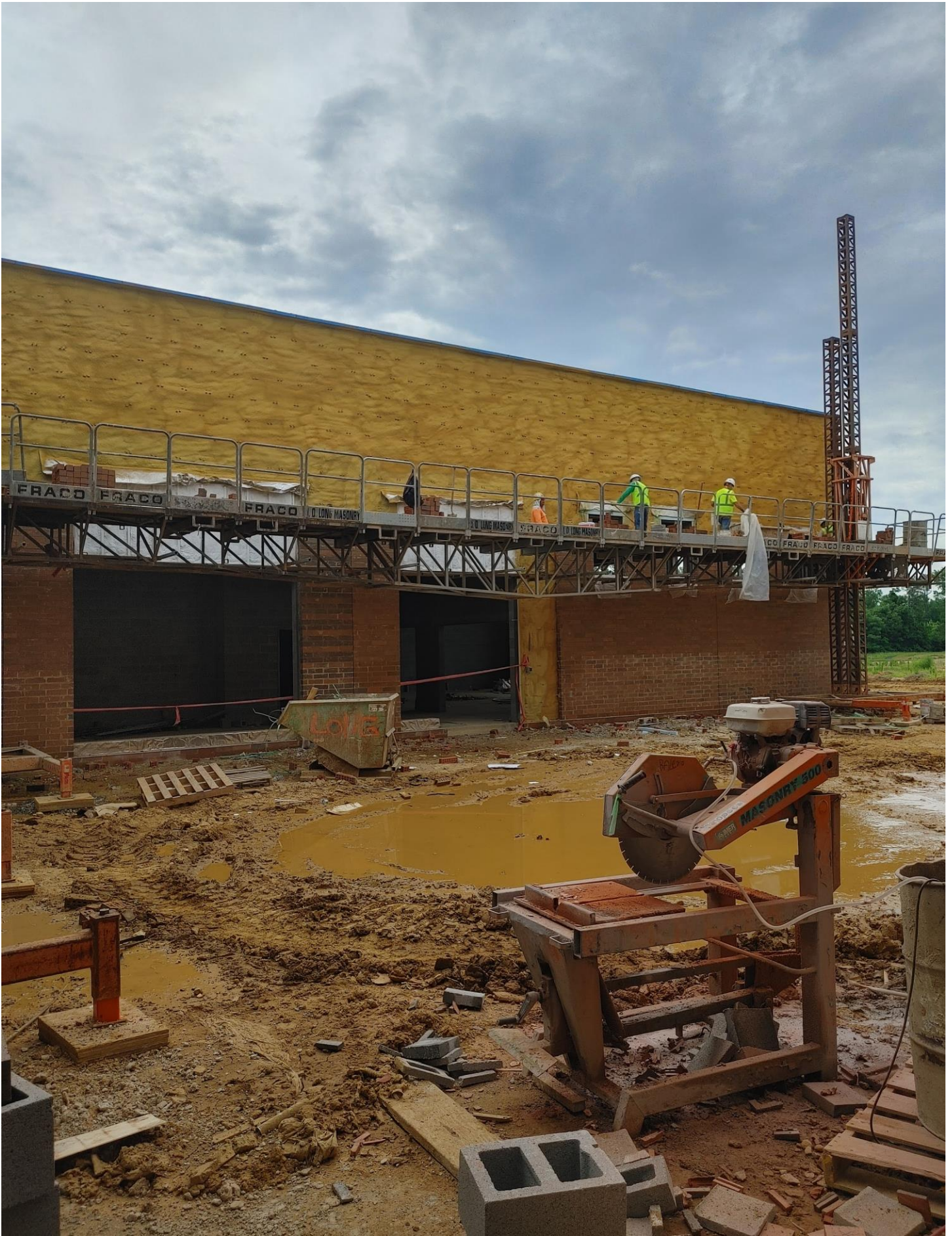
Photo 5 - Brick is being laid on the West side of Area D.
