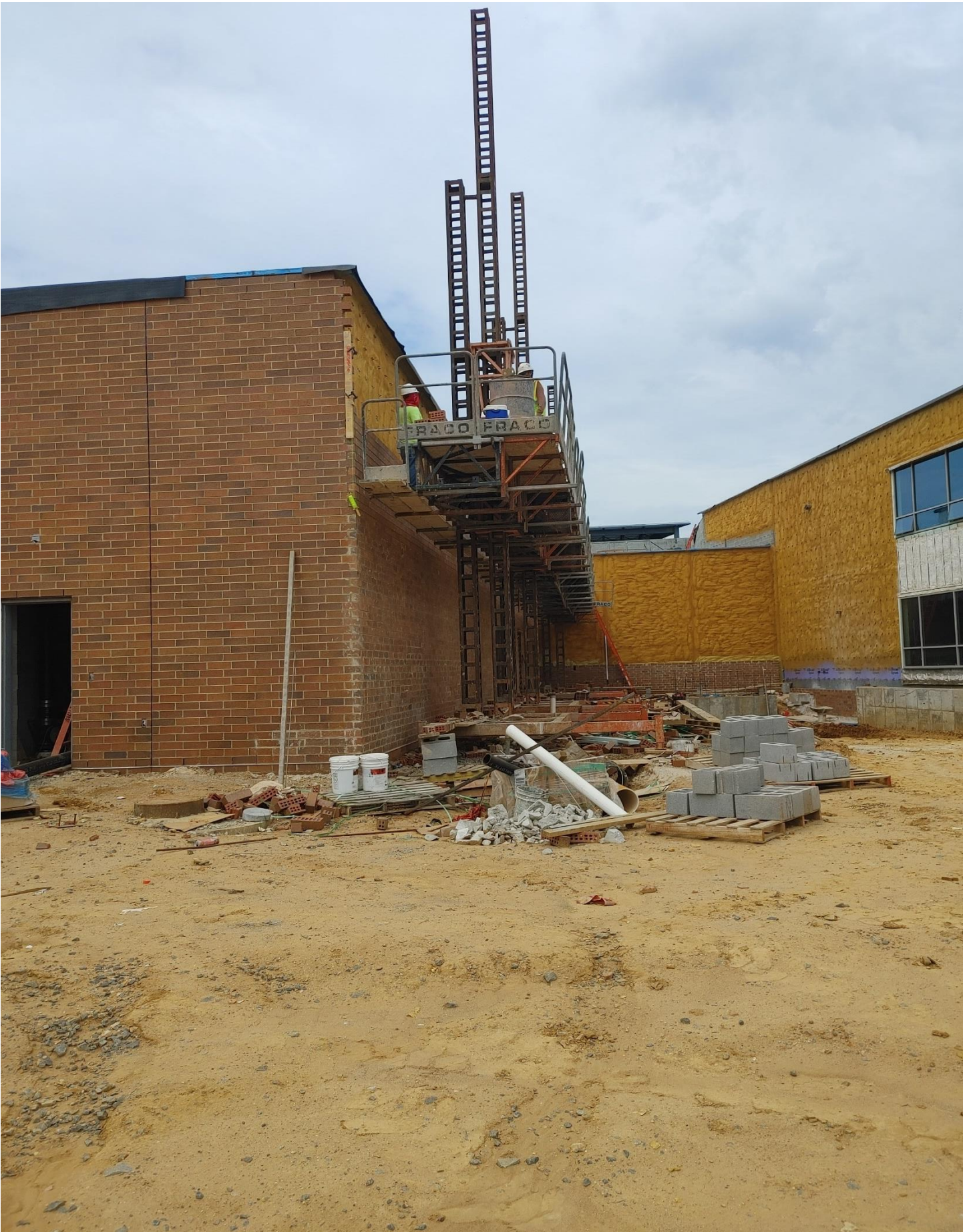
Photo 5 - Brick is being laid on the North side of Area D.
