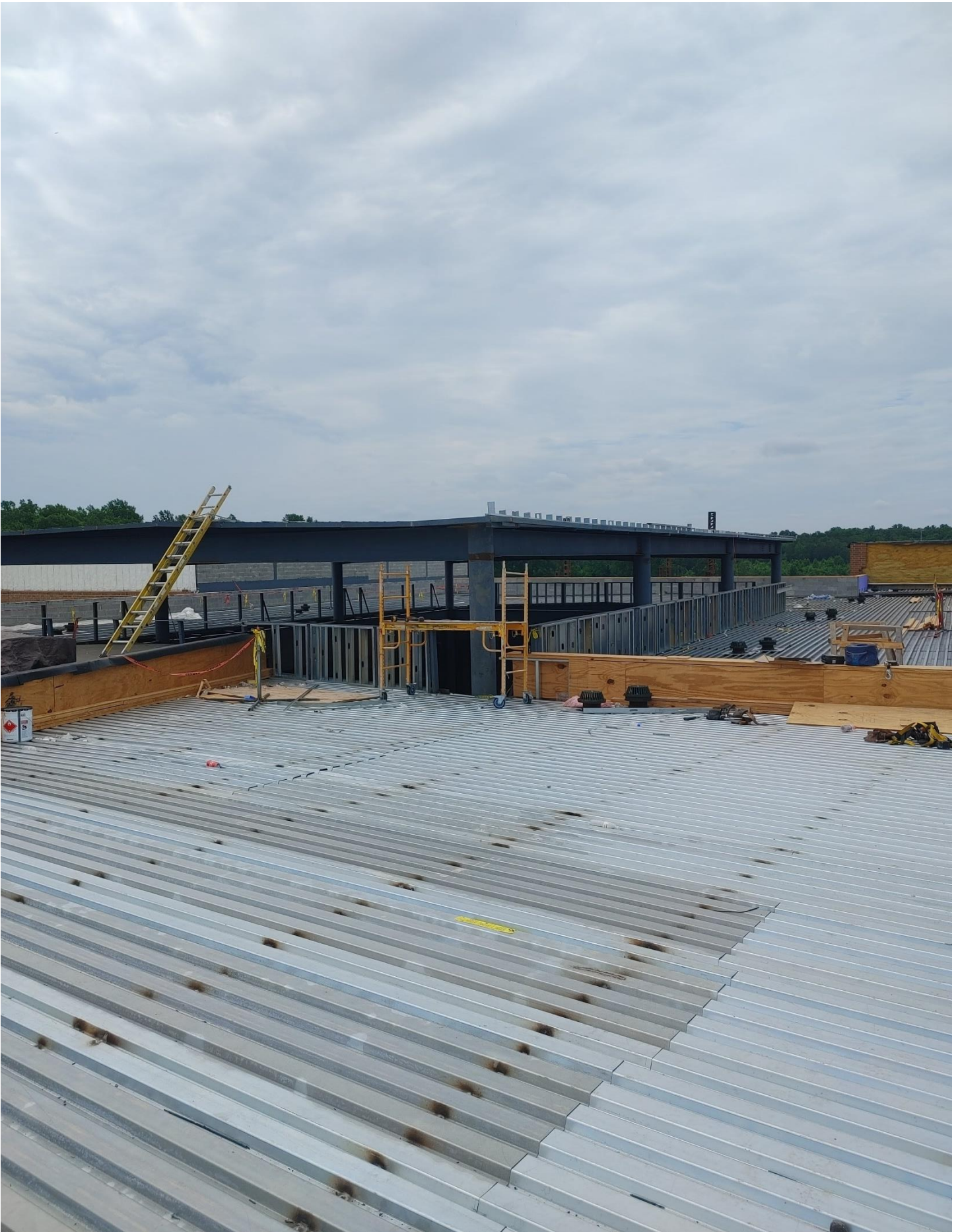
Photo 6 - Parapet walls are being framed in Area C.
