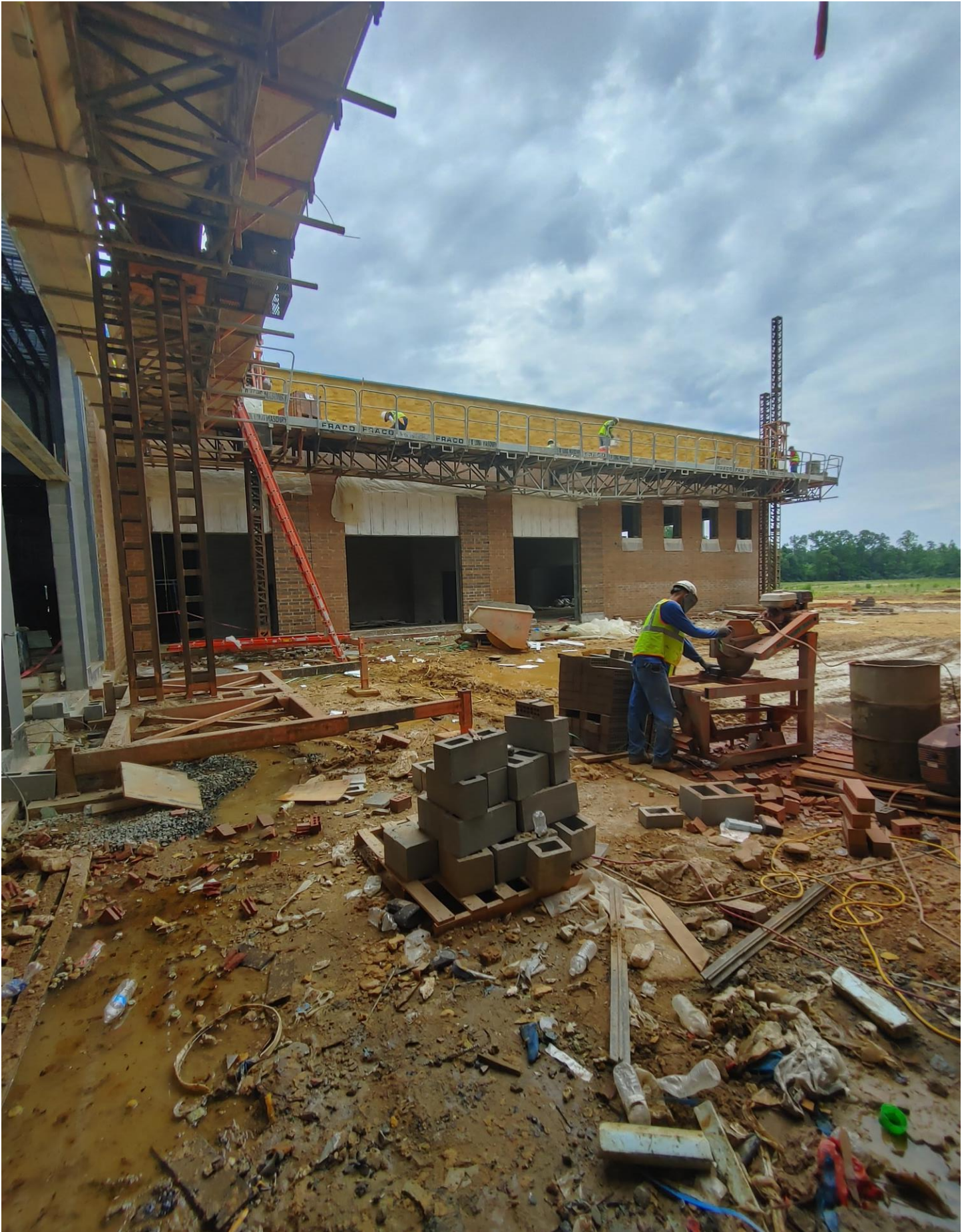
Photo 3 - Brick is being laid on the West side of Area D.
