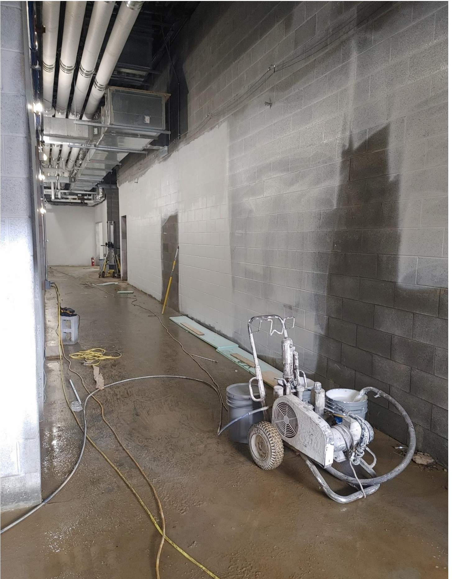
Photo 4 - Block sealer is being sprayed and back rolled in Area E.
