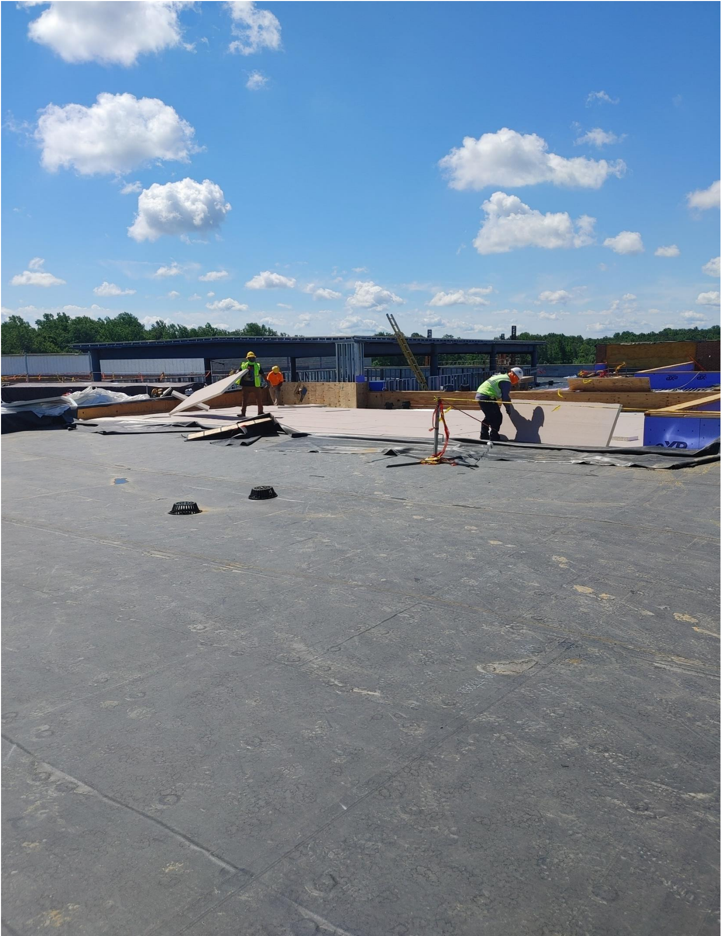
Photo 7 - Roofers are working on the Roof of Area A.
