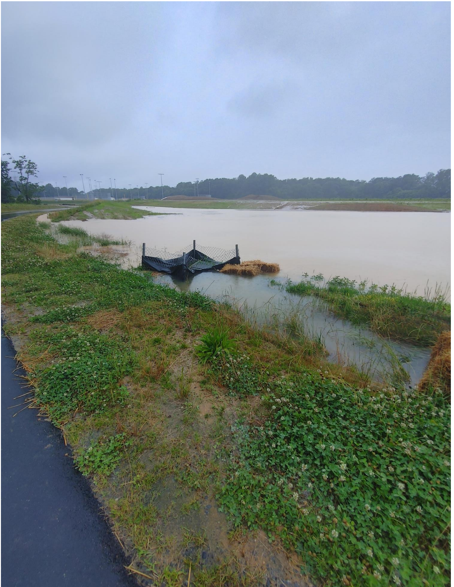
Photo 1 - Retention Pond along County Park Road overflowed its bank on 06/11/2021
