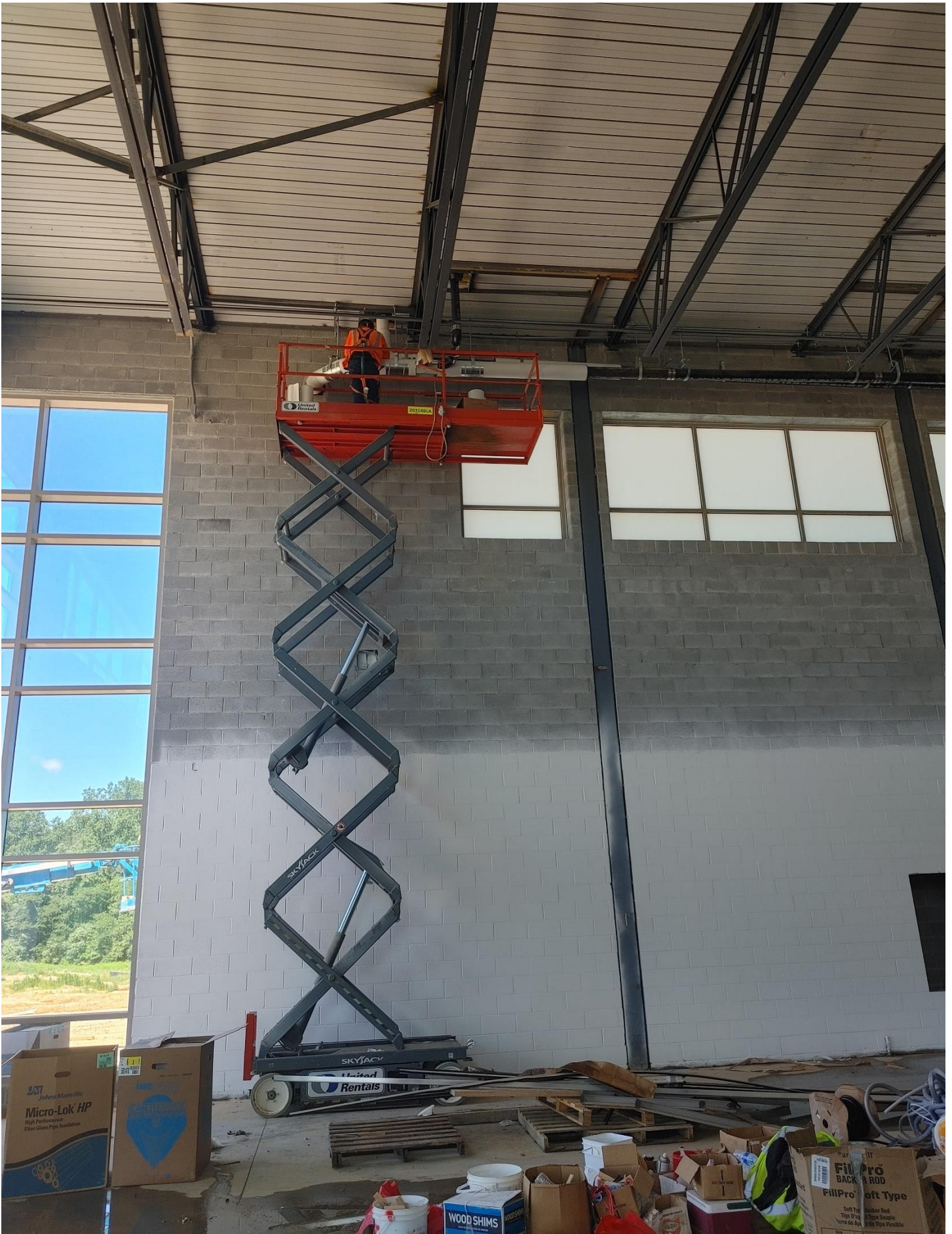
Photo 10 - Roof Drain Pipe is being insulated in Area E.
