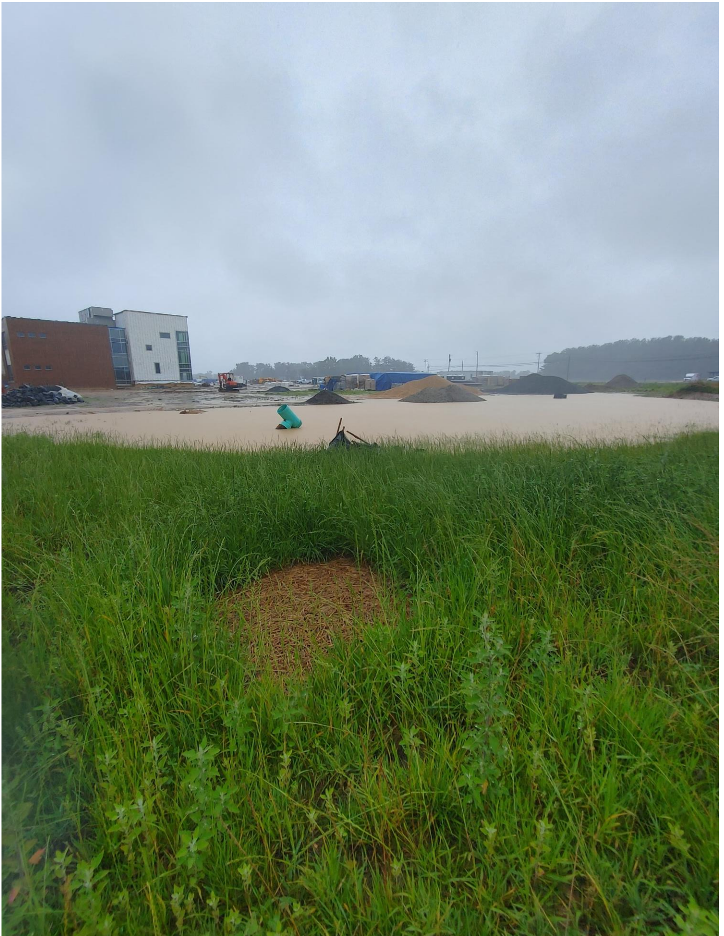
Photo 4 - Retention Pond on the Eastside of the High School.
