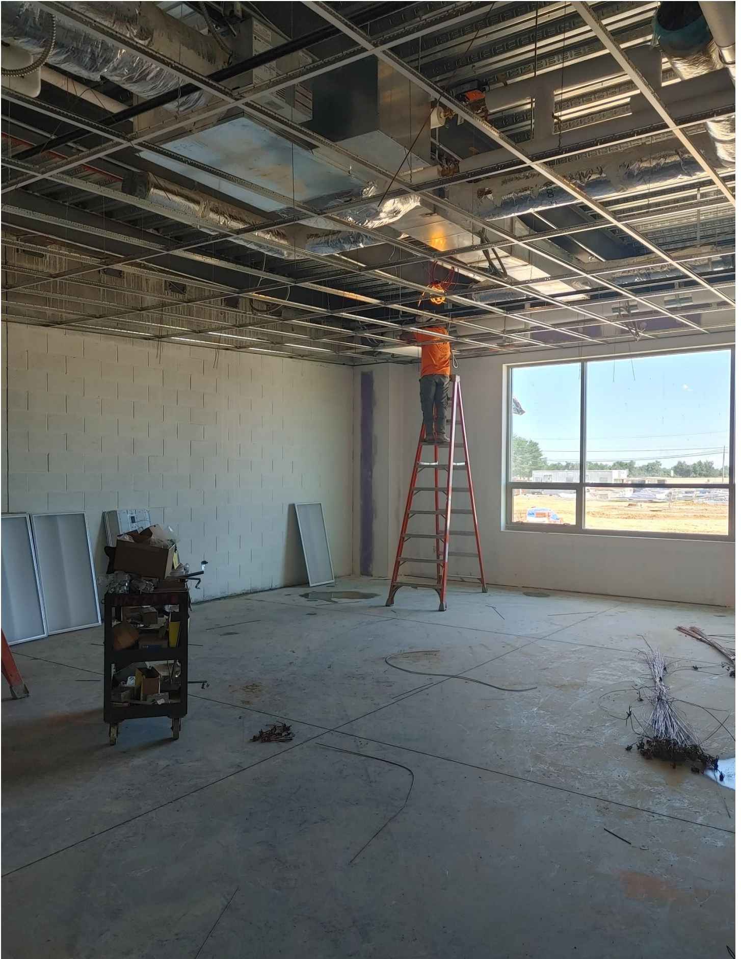
Photo 5 - Electricians installing Light Fixtures in Area A.
