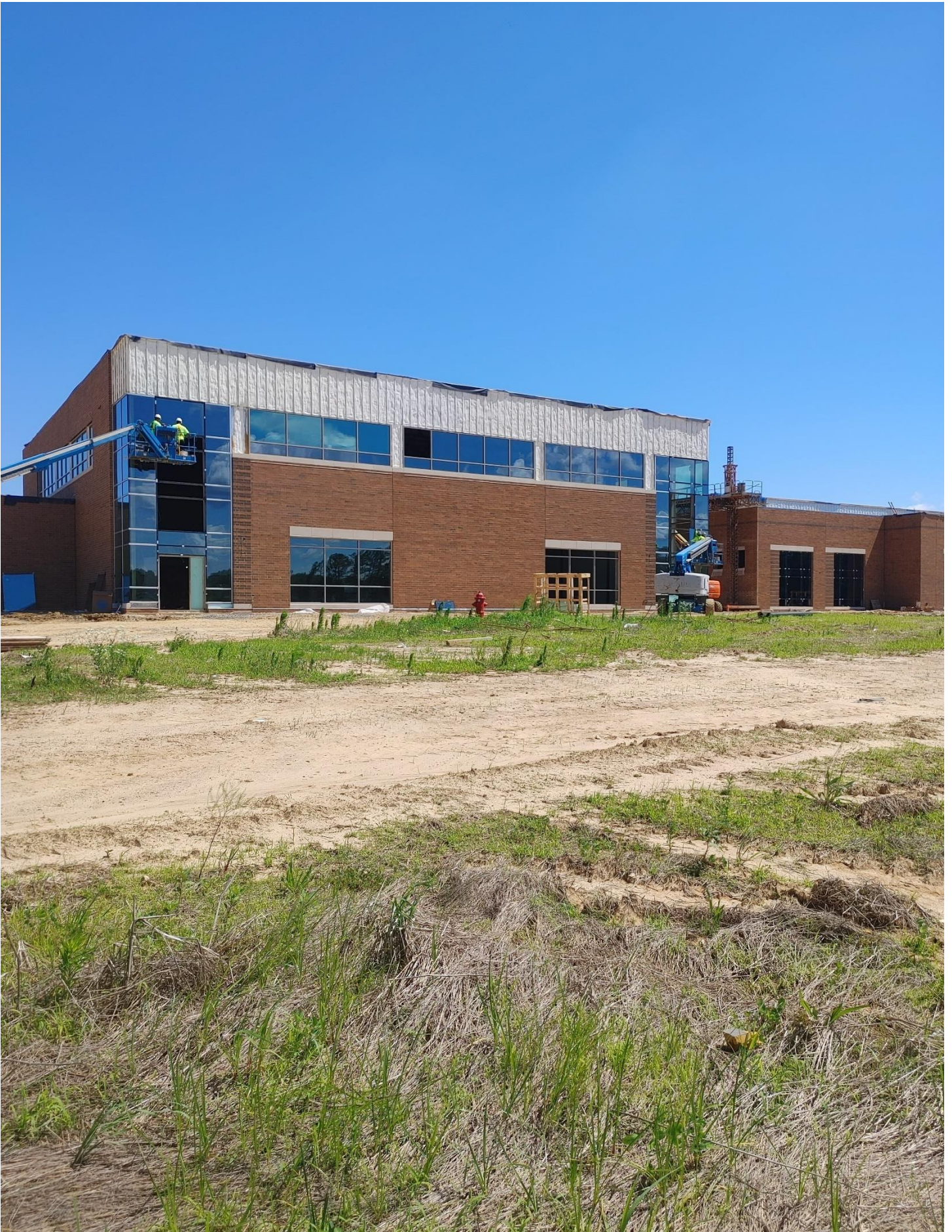
Photo 12 - FG&M Installing glass on the Southwest and Southeast corners of the Gym.
