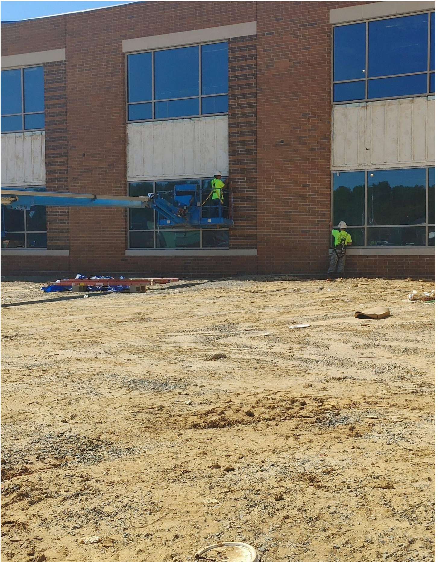
Photo 5 - FM&G installing Backer Rod around windows in Area A.
